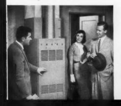
**4.** independent cooling, for use with hot water heat or where there is no central heating, is provided by this TRANE Climate Changer Fan-coil unit. Fits into just 5 square feet in attic, basement, utility room or garage. Ideal for use with TRANE Baseboard and other wet heat systems in homes or small commercial buildings. Comes in 2, 3, 5 and 7½-ton models.
