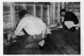
4. BASEBOARD PIGTAILS drop through holes; baseboard, backplate are seated. End fittings soldered to copper tubing.
