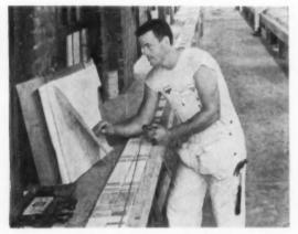
**2** Patternmaker transfers blueprint dimensions and instructions to a series of 16 foot long plywood pattern strips, marking strips for both top and bottom of walls at same time.
