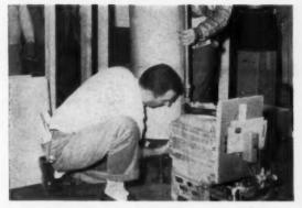
1. HOT WATER TANK is nippled to the boiler. Only two union connectors necessary. This job took 10 min.
