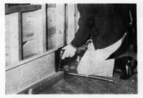
3. WITH OFFSET DRILL, floor is cut for baseboard drop. Baseboards had fittings soldered to ends in the shop.
