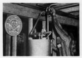
2. A 3/4" HYDRO-FLEX return loop is connected to balancing and purging valve. All vents are eliminated.
