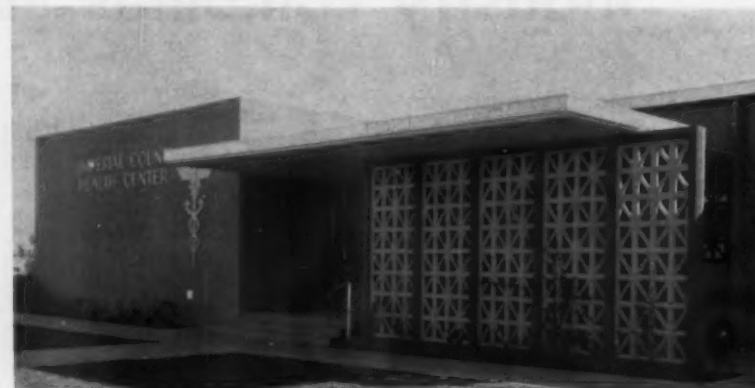
Completed building has light-weight, well-insulated wall
