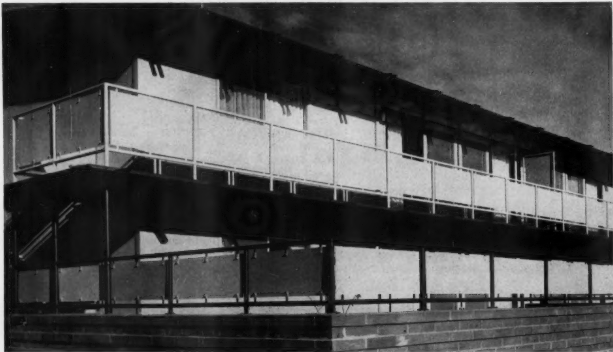
Built mainly of plywood, these apartments are part of the Tsunoda Garden Apartments located at Mountain View, Calif. Premier
