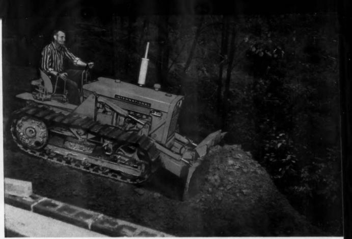
Fast, sure response of T-340 controls enables operator to work close to edge of bank with complete safety. Light-treading
