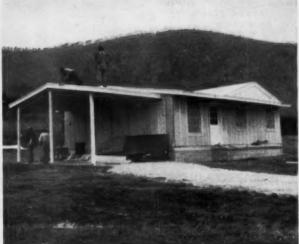
**4:30** Houses are erected and closed-in by seven-man crews in 8 hours, and are ready for interior finishing. Prime-coat painting of the exterior components safeguards them from inclement weather.
