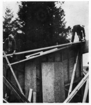
Decking spans box beam and side walls
