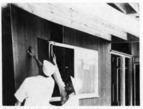
Hardboard siding nailed right to studs
