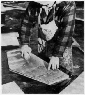
Specially-engineered template speeds fastening To mark nailing pattern on gusset plate blank, spray-paint bomb and template engineered by DFPA are used. Builder does as much detail work as possible in shop to keep quality high.
