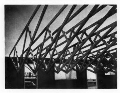
Laborers position 28' Sanford roof trusses—21 to a house—for Builder John Long of Phoenix, Ariz. They're spaced approximately where they will be spiked to the plate.
