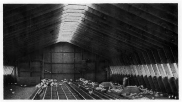
There's a growing demand for rigid frame poultry buildings; they offer plenty of ventilation Big benefit of rigid frame poultry building is ventilation for birds. Using pulleys, endless rope, and cleats similar to those used in boats, window system was developed by builder. Structure measures 40x100°; it's located on farm near Yelm, Wash.
