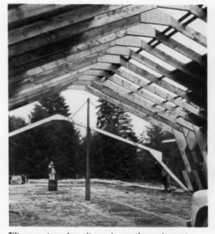
Tilt-up system doesn't require costly equipment Frames go up fast and easy with this system. Other ways include walk-up "bleacher" mounted on back of flatbed truck and Army surplus boom welded on pickup truck.
