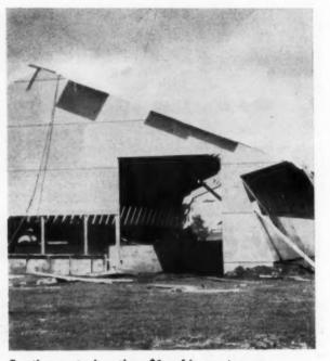
**Erection costs: less than \$1 psf in most areas** End walls of rigid frame building are quickly framed conventionally. Minimum framing was used at opposite end of this building; owner plans to add another 100' to it later.
