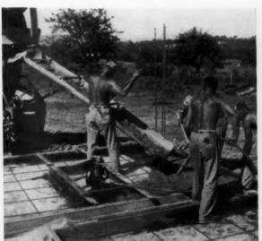
**Reinforce** 4" x 10' x 10' panels with 5 #3 bars Sand casting bed is used, if floor isn't handy. Grade, spread 3" to 6" layer of sand. Screed to level; place film. Reinforcing rods go both directions in forms. Cast in alignment for tilt-up.
