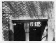
CLOSE - UP of Keymesh Lath that serves as base for  $7/_8$ " machine-applied marble-chip concrete. Wall is 3" of sprayed perlite concrete.
