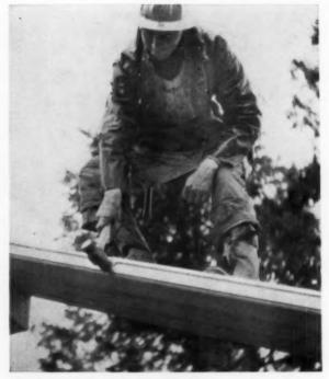
Decking is pre-drilled for spiking
