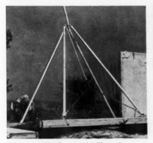
Light tractor, tilting frame used to lift panels Simple pipe frame, with telescoping legs for different-sized panels, and tractor pulls panels into place. Forms are stripped before erection. For slight panel adjustment, pry bar is used.
