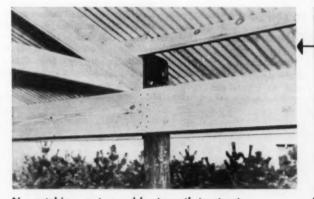
No-notching system adds strength to structure
