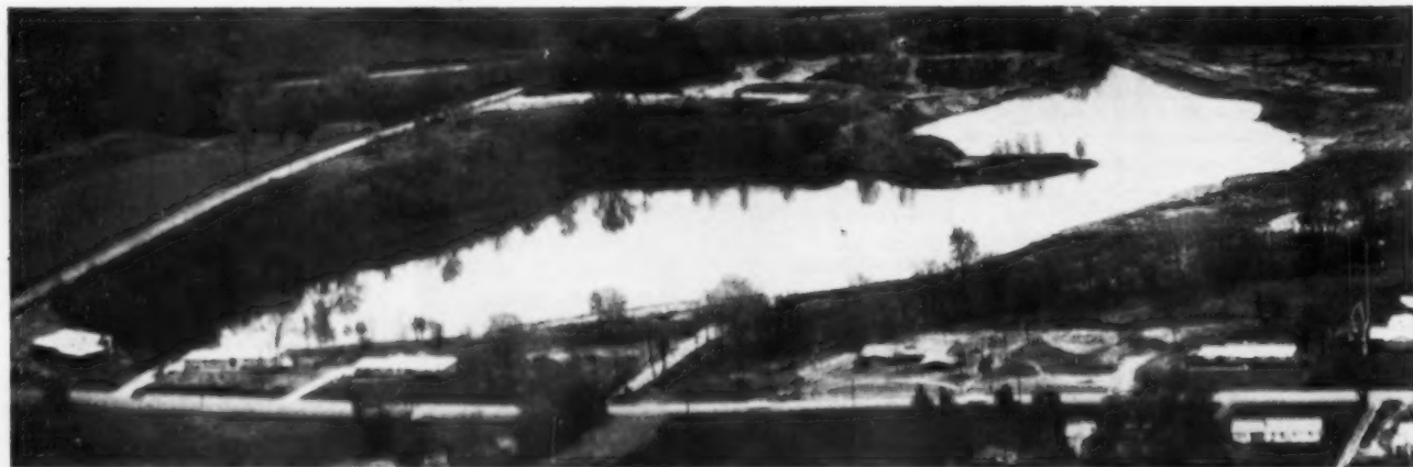
HELICOPTER VIEW OF WESTCHESTER ESTATES IN 1961. 21 of the 32 lake sites were sold before utilities were completed.
