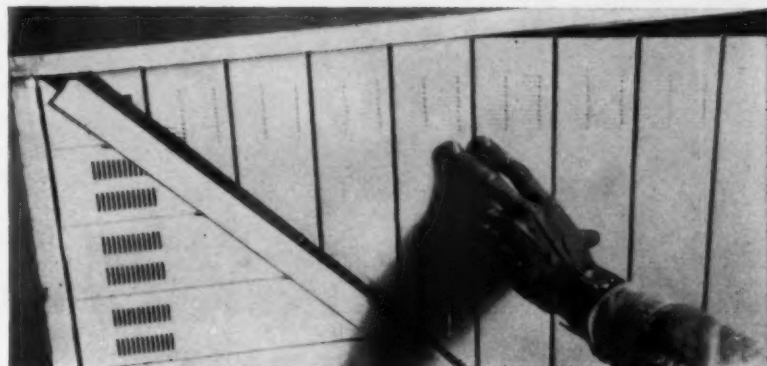
Panels are mitered at site for attractive corner treatment
