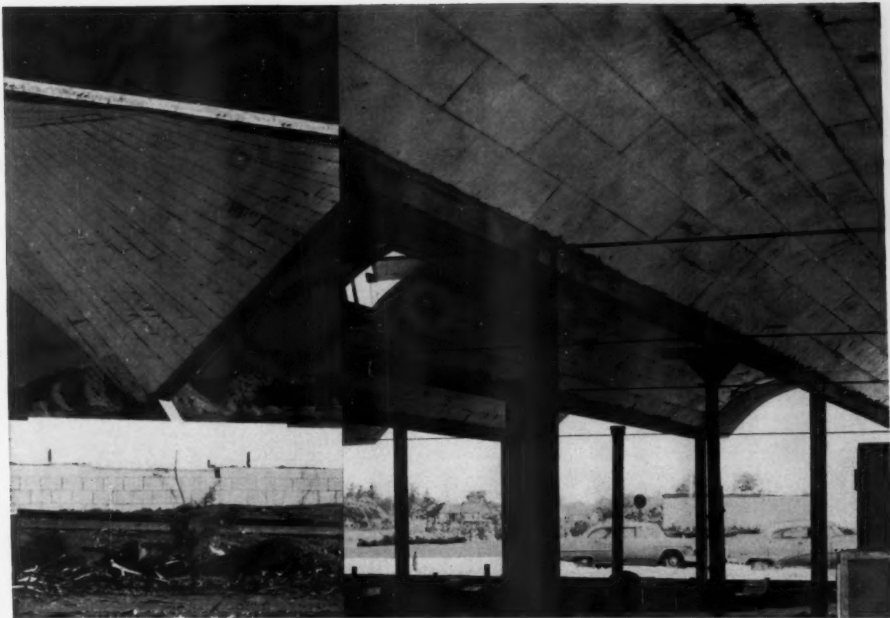
Hyperbolic paraboloid (above) and barrel-vault roof (right) show Styrofoam insulation form liner ready for plastering.
