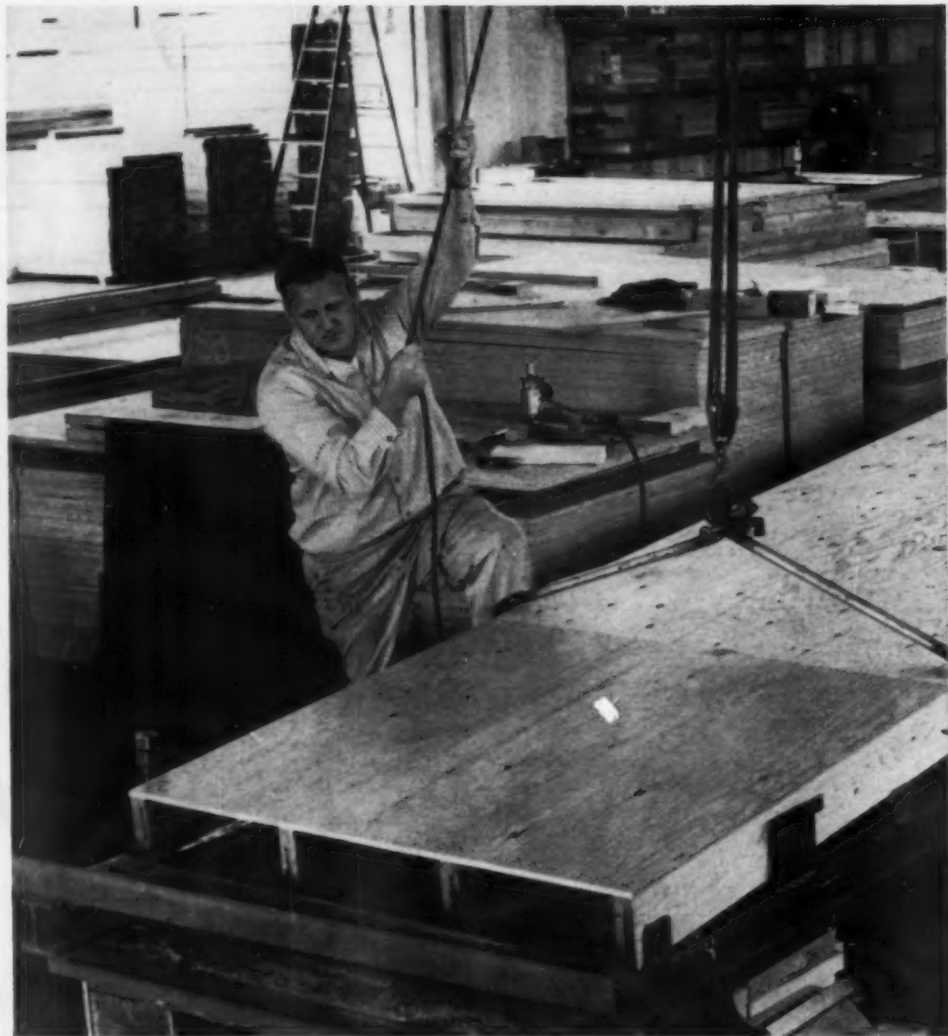
Bell & Valdez' floor panels also can be used for carport roofs
