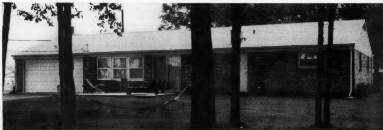
Orientation allows plenty of privacy for outdoor living at the rear where terrace is located.
