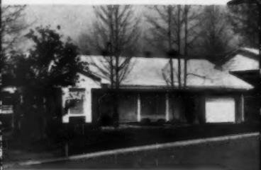
Downspout Conductor Drainage
