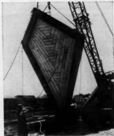
1½-inch Styrofoam serves as form liner, permanent insulation and base for plaster in this lightweight tilt-up panel.
