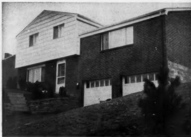
SAME HOUSE, SAME BUILDER: BUT $1,500 LESS. The only difference in this home (built in Whitehall, just outside of Pittsburgh) are the cost-saving features that were permitted by updated plumbing and building codes. Average price: $21,000.
