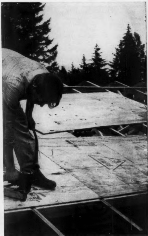
Automatic stapler speeds top-out time
