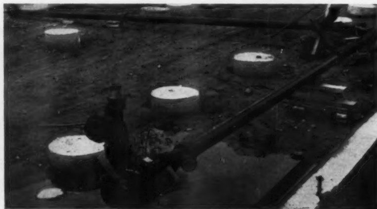
Pre-fabricated plumbing runs cut cost of labor for Bell
