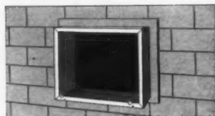
Galvanized steel sleeve is cemented right into wall during construction.
