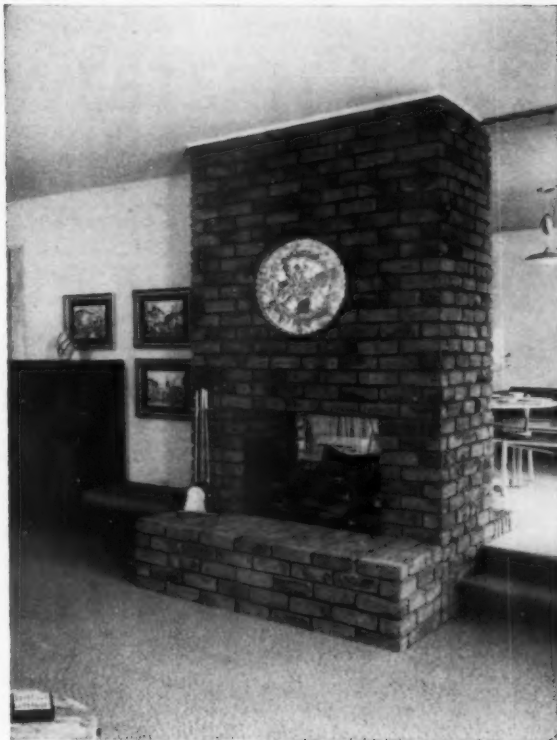
Brick adds rugged texture and contrast to the simple, flat wall surfaces in this house; hearths of various heights were designed to fit naturally into the different floor levels of two rooms and keep carpeting safe from embers. Two-way opening is a money-saver, warms both rooms and eliminates the need for two separate fireplaces and chimney flues.
