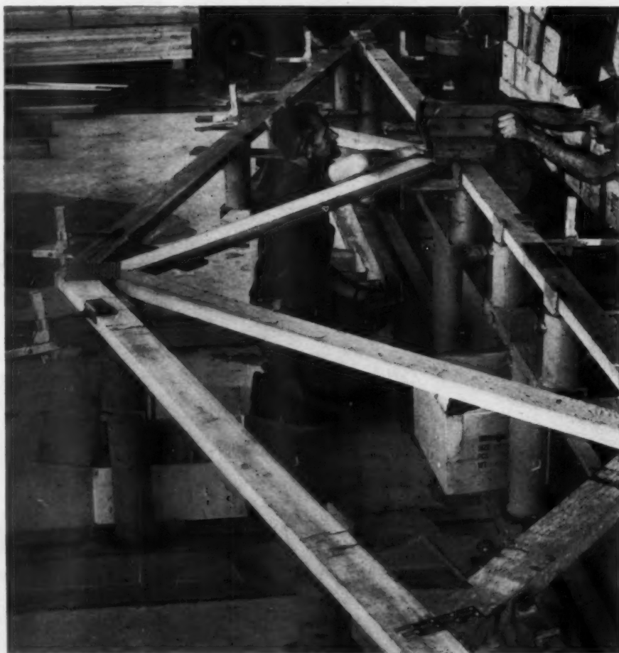
Truss production: 100 daily, fabricated by two-man crew
