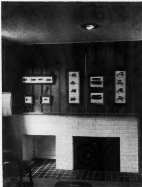
Simplified traditional design combines fireplace and wood box into single unit. Brick facing has been painted white, to contrast with the warm tones of the surrounding butterfly-jointed pine paneling. A molded wood strip frames the unit; hearth is square ceramic tile. Door, at back of wood box, opens into garage to allow storing of wood from outside.
