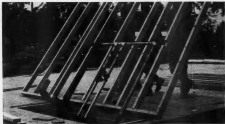
Plumbing wall is tip-up; connects to under-floor runs
