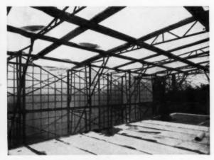
English-designed enclosure system utilizes scaffolding and wood frames for support
