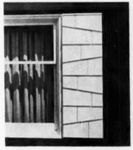
For this design, butts of shingles are trimmed on slight angle; direction changed.
