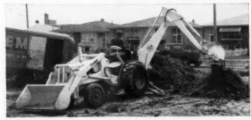
If you need footings for slabs on grade, or dig your own septic systems, or want to handle trenching for sewer and water lines . . . See Case 530 Utility Backhoe-Loader. Hoe cuts over 16' from pivot, digs 14' deep, excavates fast because exclusive foot-pedal swing control allows bucket operation while swinging.
