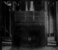
3 Face masonry and hearth completed, chimney section started.
