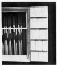
Double-crossed shingles give deep shadow lines. Joints are spaced 1/4" apart.
