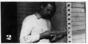
TIES IN ... Many wall sections were left unfinished for other work to progress. For continuous reinforcement, Keywall was used. Bill Revers of Crouch-Walker, shows the Keywall "tails" to be tied in later. Only Keywall can be tied in. Only Keywall is flexible enough to accommodate variations in mortar joint levels.
