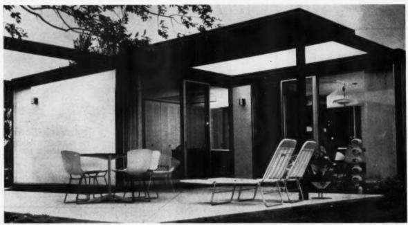
MODULAR PRINCIPLE of design allows flexibility in arrangement of colored aluminum panels and fixed or sliding glass walls.
