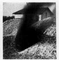
Oil drums can be substituted for pipe to heat sand
