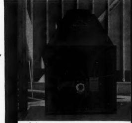
Base laid, firebrick hearth installed, fireplace form positioned.
