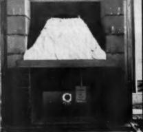
2 Form wrapped with insulation, concrete block installed to 8" above chimney base, face masonry started.
