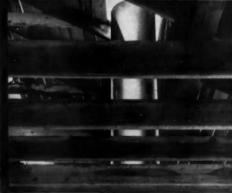
Chimney section extended thru roof, ready for exterior housing installation.
