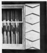
This shutter is made from machine-grooved shakes; butts are retrimmed on an angle.
