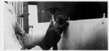
**CLIPS** are nailed to sheathing or studs, fit into groove along butt edges of siding. Snug assembly is achieved, yet system permits natural ventilation.
