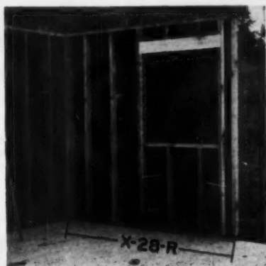
Panel 28-R is 8" wide. When six are used—side by side—48" wide sheathing can be fastened on, saving time. Windows, partitions can be located in any position.
