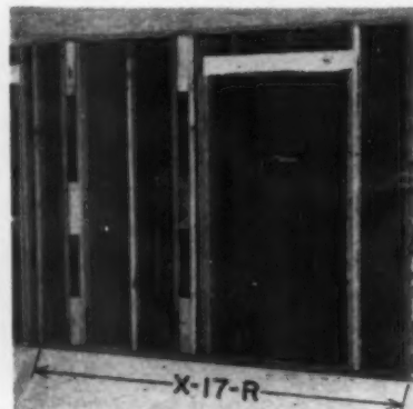
Panel 17-R measures 9'4". It is framed for one 3-0 door and two partitions. Note partition nailers. Unit utilized two pieces of sheathing; waste is reused.
