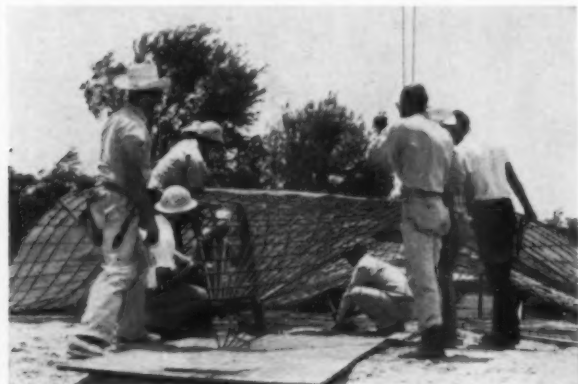
Workmen assemble geometric framework on ground
