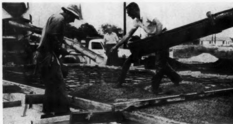
Solid concrete wall is poured flat, tilted up into place
