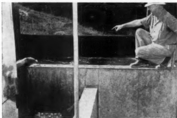
Builder Mikkelson kneels on settlement basin wall, part of small tract sewage system
