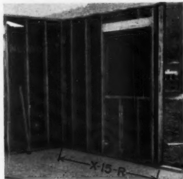
Panel 15-R has one window. From exterior framing lines, studding 16" o.c., can use vertical, horizontal siding, providing it is in multiples of 16".
