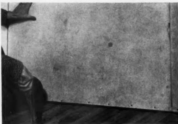
Wall panels installed on top of finished floor
