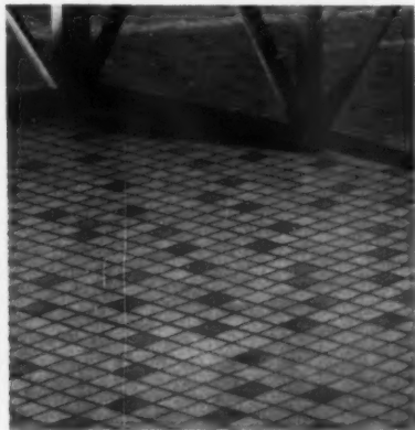
WROUGHT IRON RAILING enhances entryway floor which is laid in 1"x1" mosaic tile blocks. All units in new line have smooth, all-purpose joining edge.
