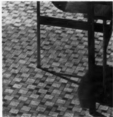
FAMILY ROOM FLOOR is laid in 2"x2" blocks, 2"x1" random blend strips and 1"x1" accent blocks. Clearline and Texline tiles come in 45 color styles.
