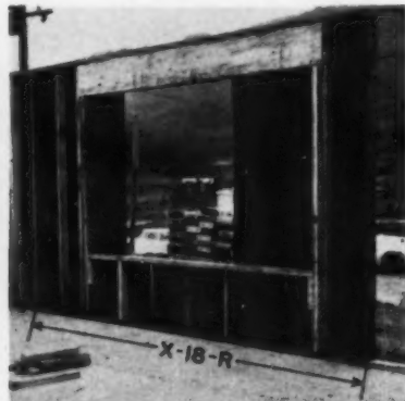
Panel 18-R is framed for large window, which determined smaller size for 19-R. Too, if 18-R had been made any larger, it would have been hard to handle.
