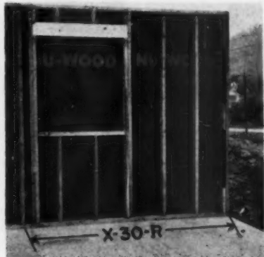
Panel 30-R has one window and corner post. Two pieces of sheathing 48" wide were used. Studding is on 16" centers. Centers are carried through openings.
