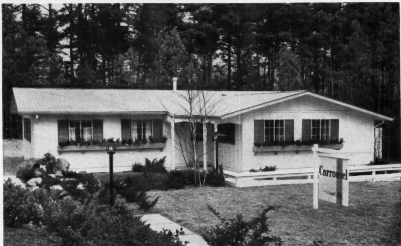
Asbestos cement, prefinished with acrylic coating, covers all outside walls, trim and battens, eliminates repainting up to 30 years.
