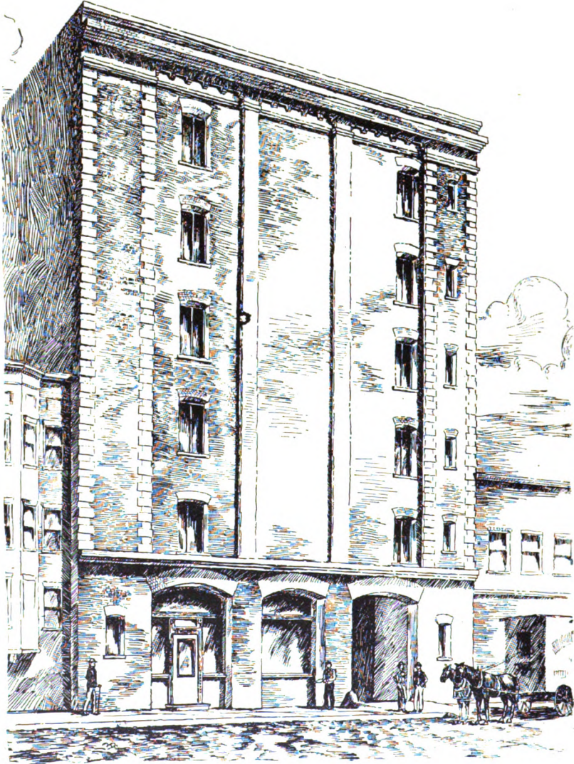
Reinforced Concrete Storage Warehouse for Bekins Company, San Francisco First structure of kind to be built in California. Ralph W. Hart, Architect.
