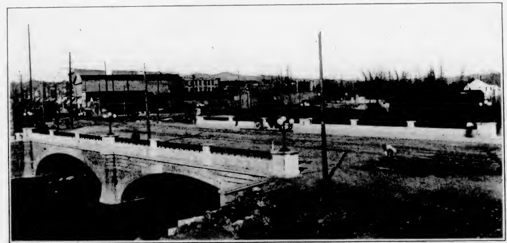
Reinforced Concrete Bridge, Reno City, Nev.
