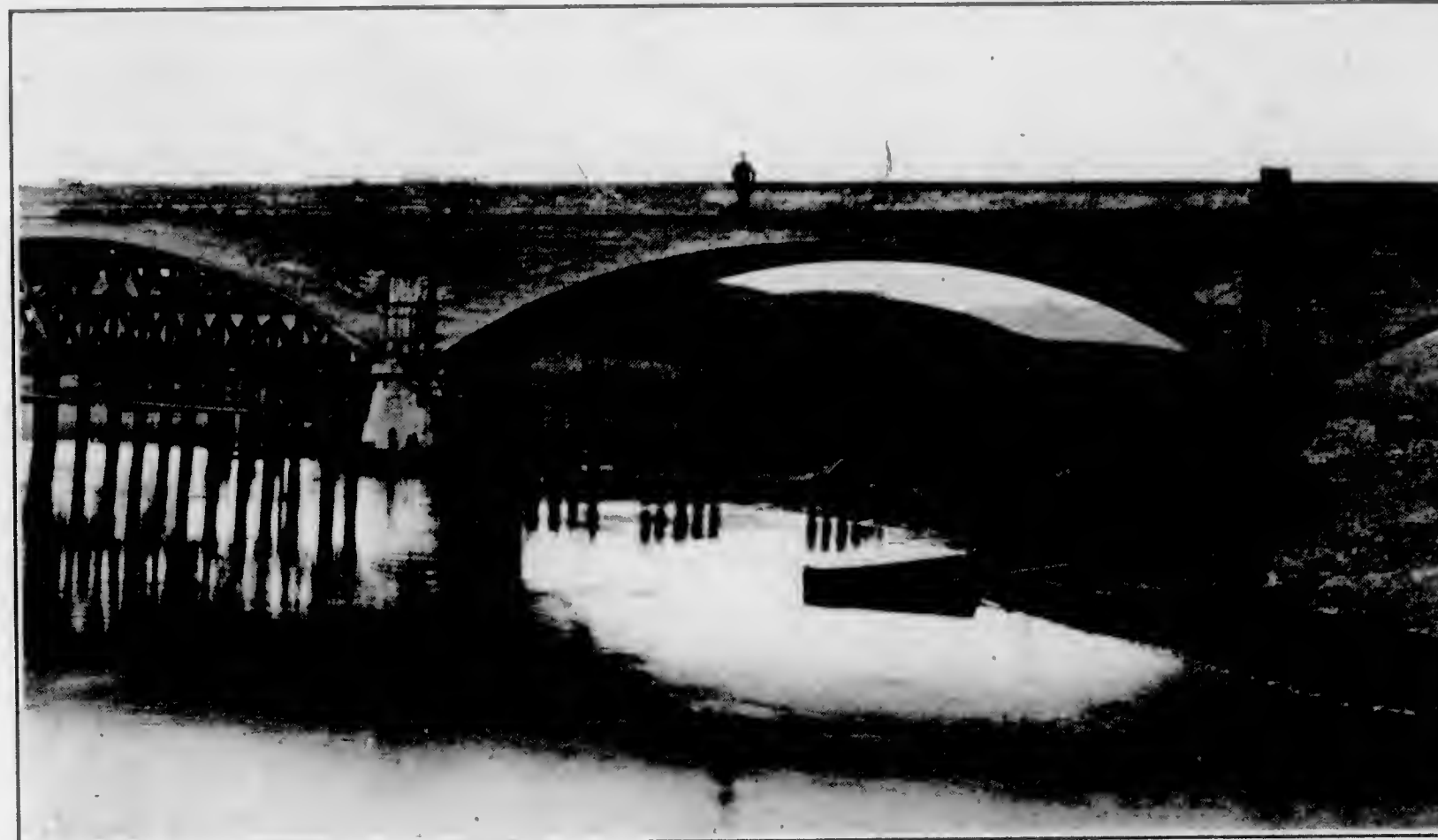
Concrete Bridge at Pollasky, Cal., Ten 75-foot Spans, Reinforced with Corrugated Bars, Designed by Jno. B. Leonard, C. E.
