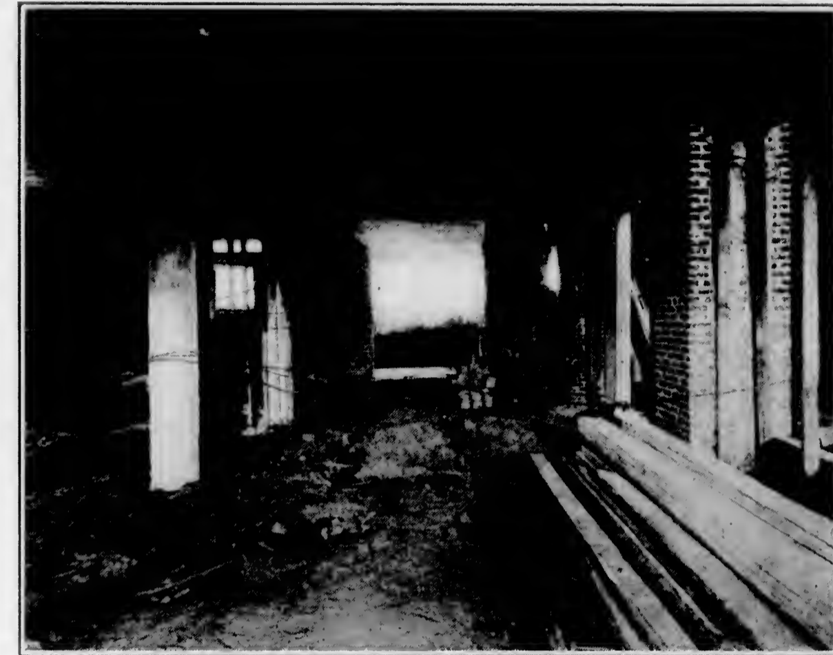
View Showing Tile Construction, Basement Marysville Public Library C-425
