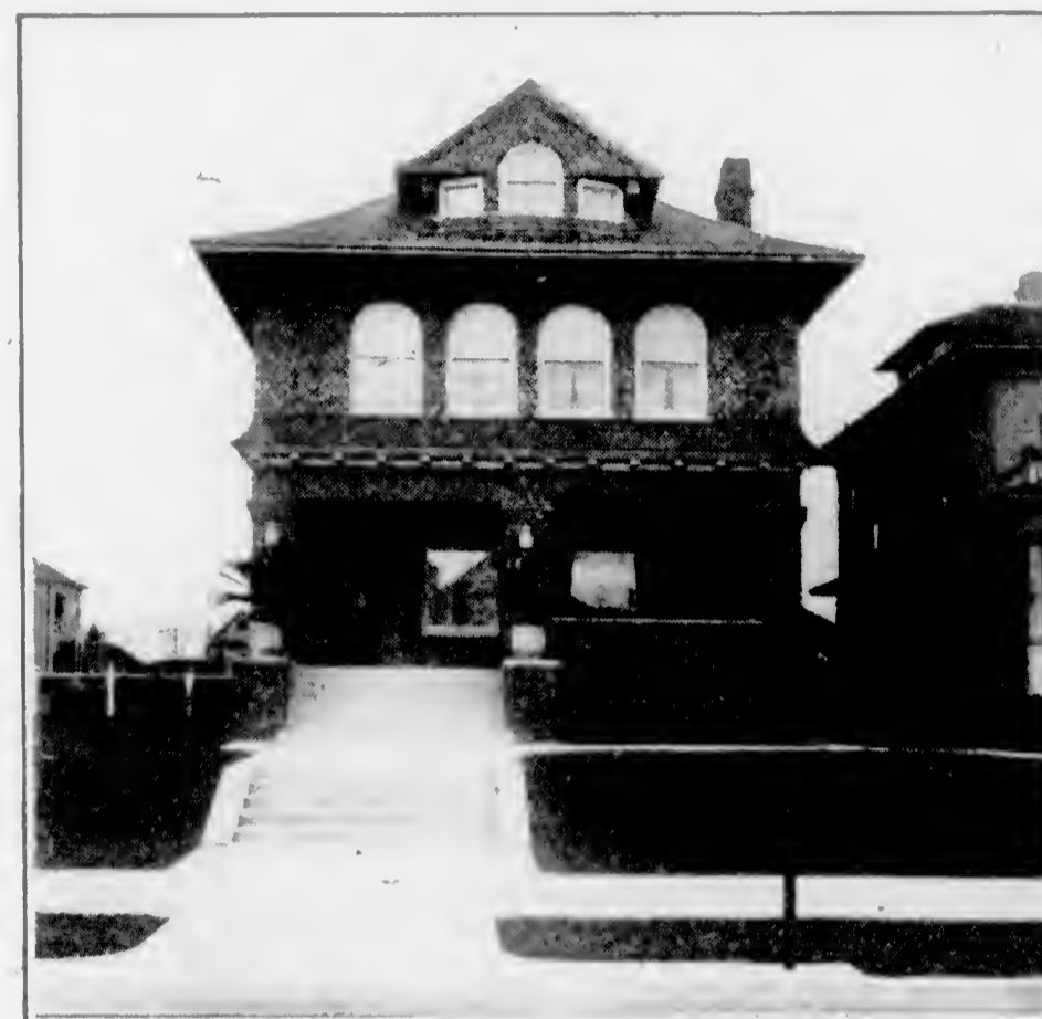
Keyes Residence, Sacramento Hook & Son, Builders C-405 Electrical Work by Electrical Supply Co.
