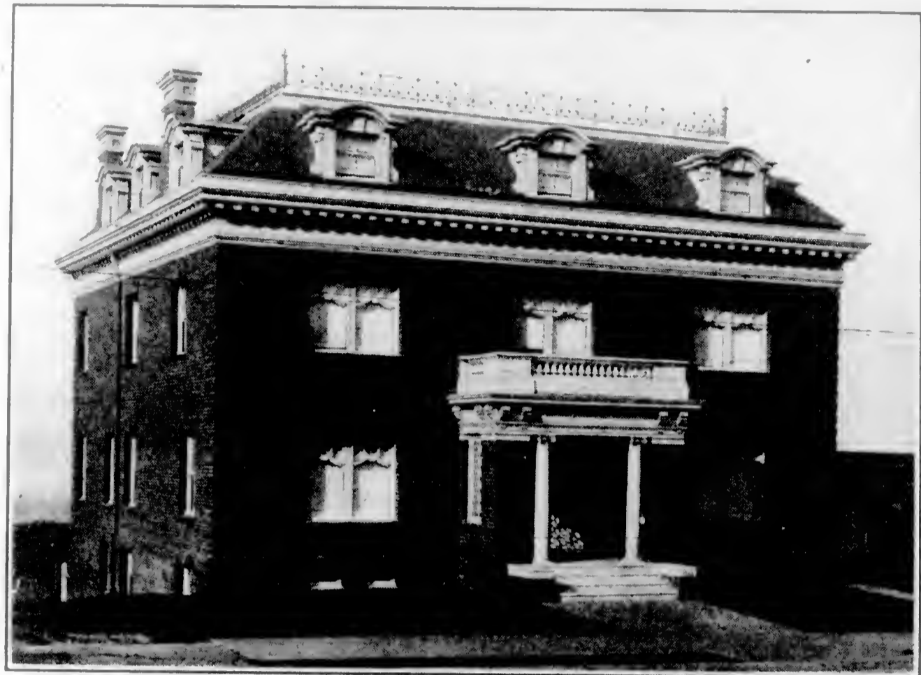
Residence of Mr. Leon Kauffman, San Francisco Edgar A. Matheson, Architect C-357
