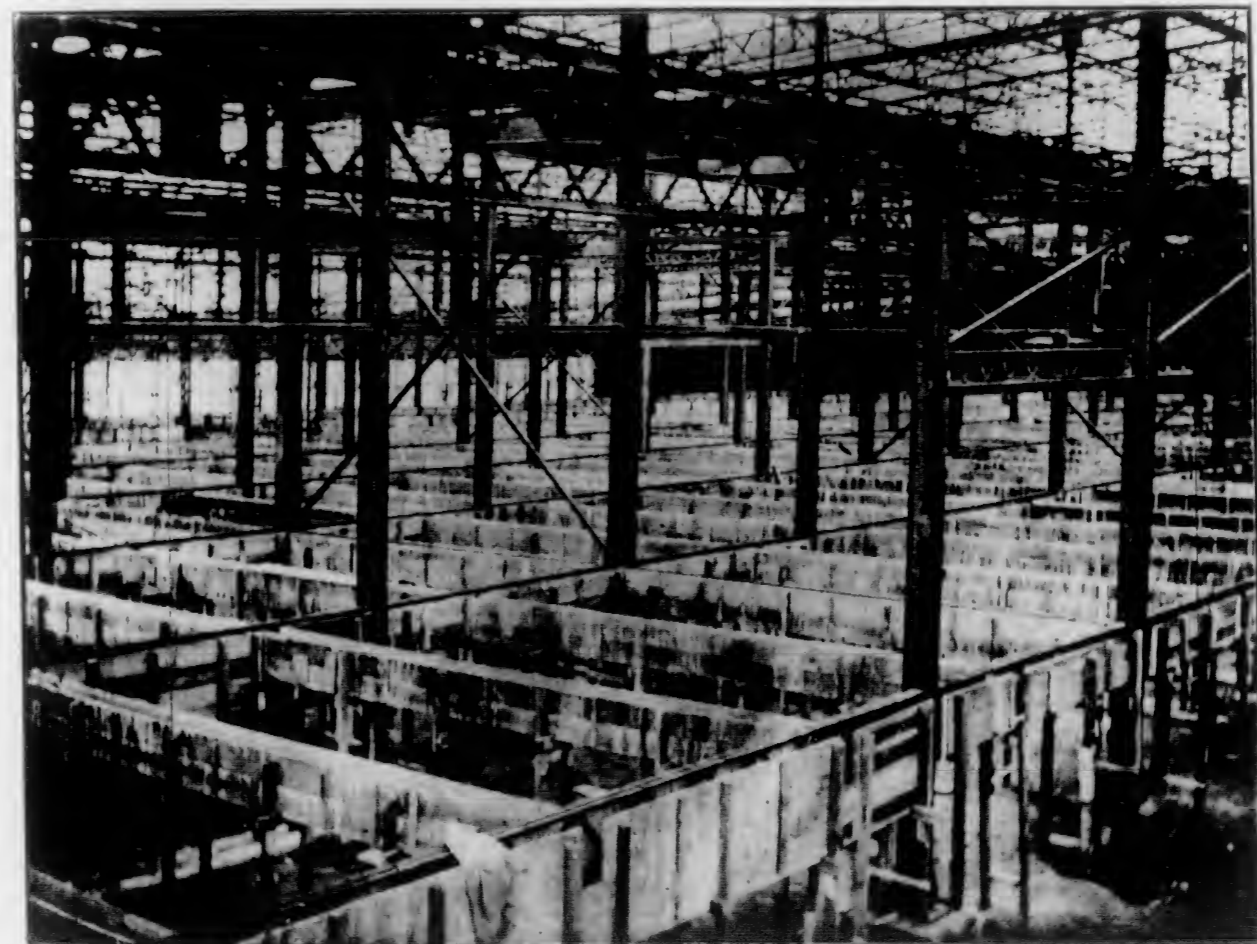
UTAH COPPER COMPANIES WORKS, GARFIELD, UTAH.
