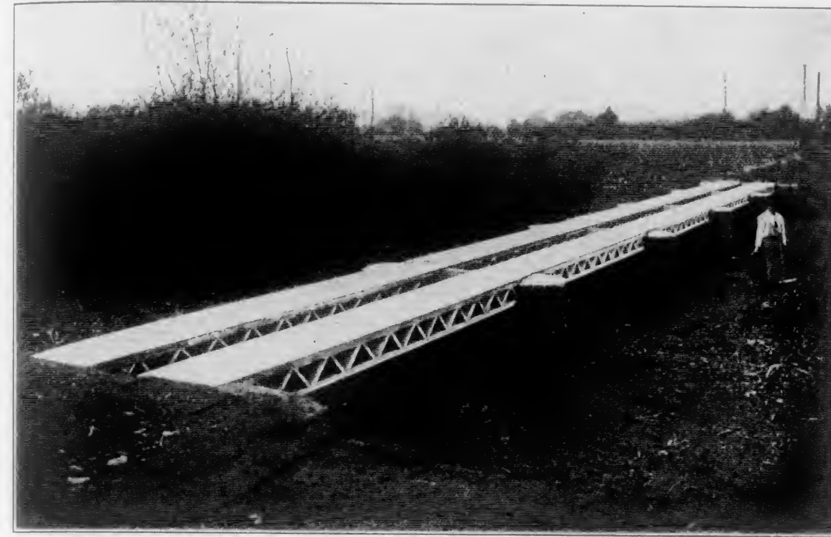
A Railroad Bridge of Reinforced Concrete
