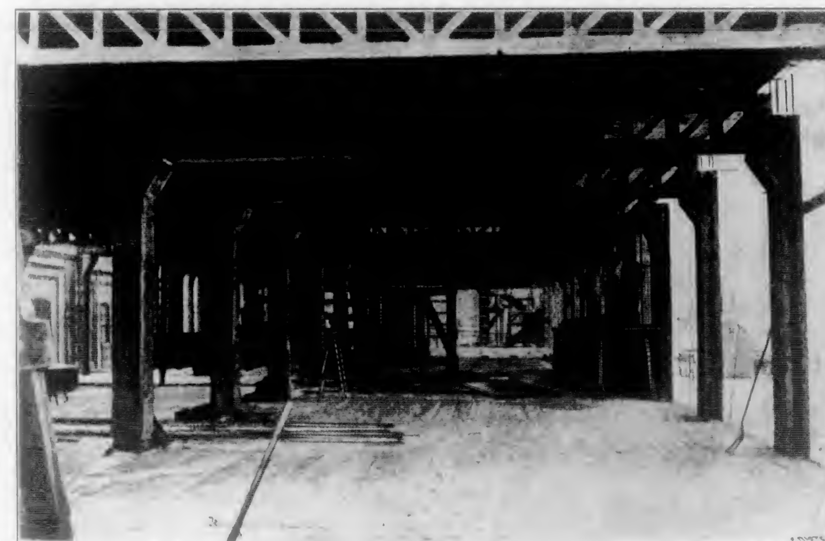
View Showing Inside Floor Near Completion Factory Building, Reading, Pa.
