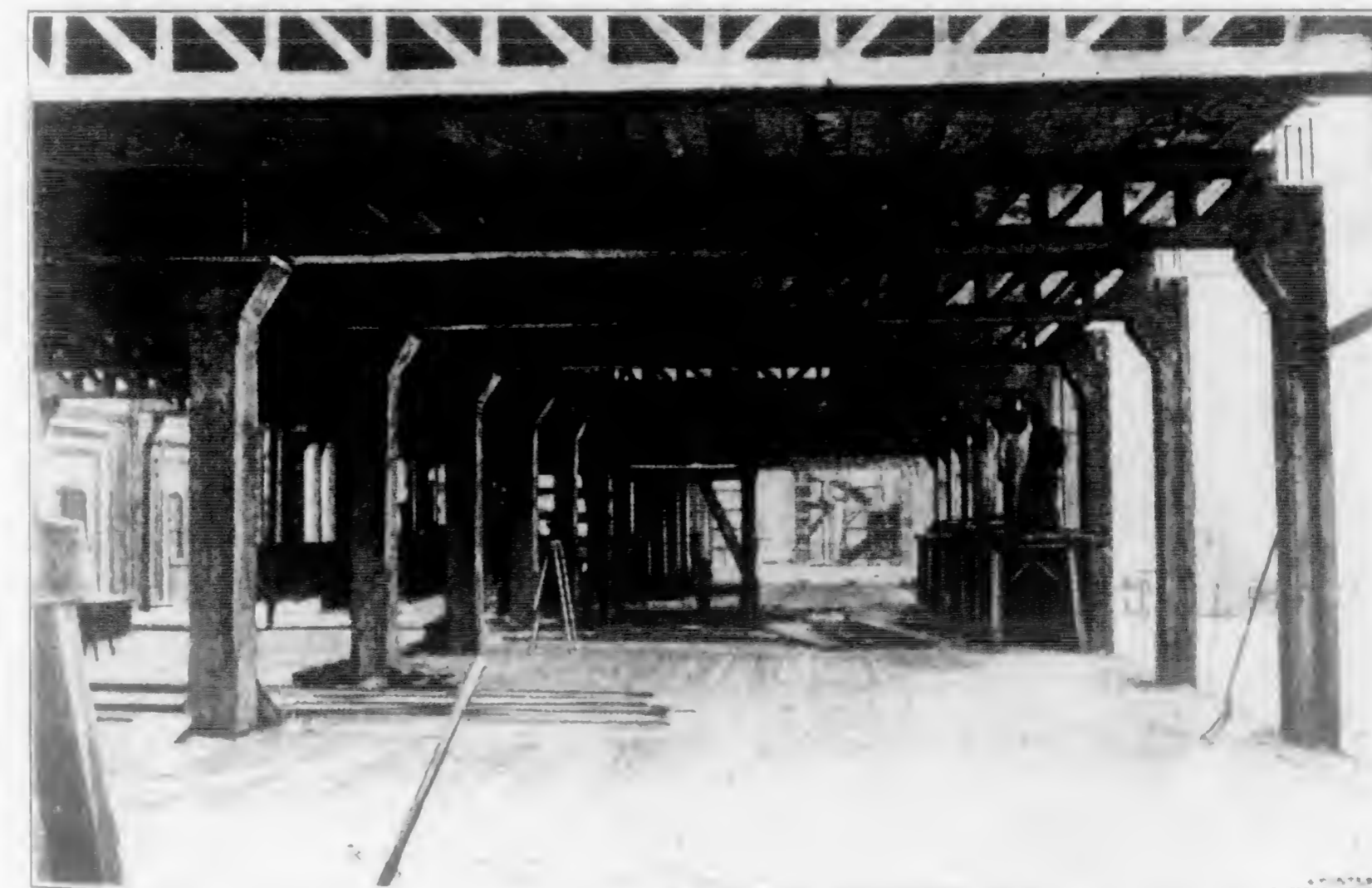
View Showing Inside Floor Near Completion Factory Building, Reading, Pa.
