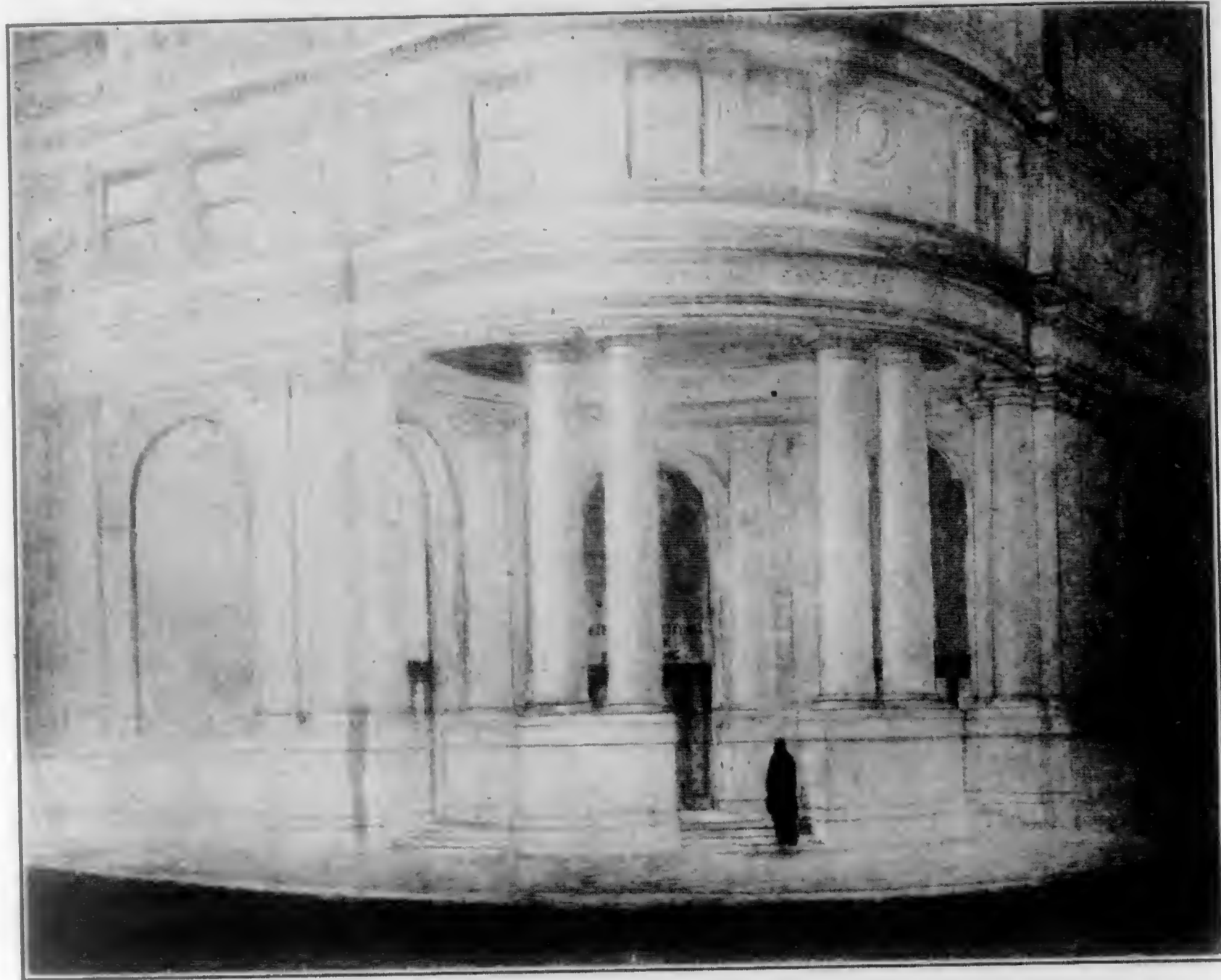
Entrance First National Bank Building D. H. Burnham & Company, Architects Equipped with Otis Elevators
