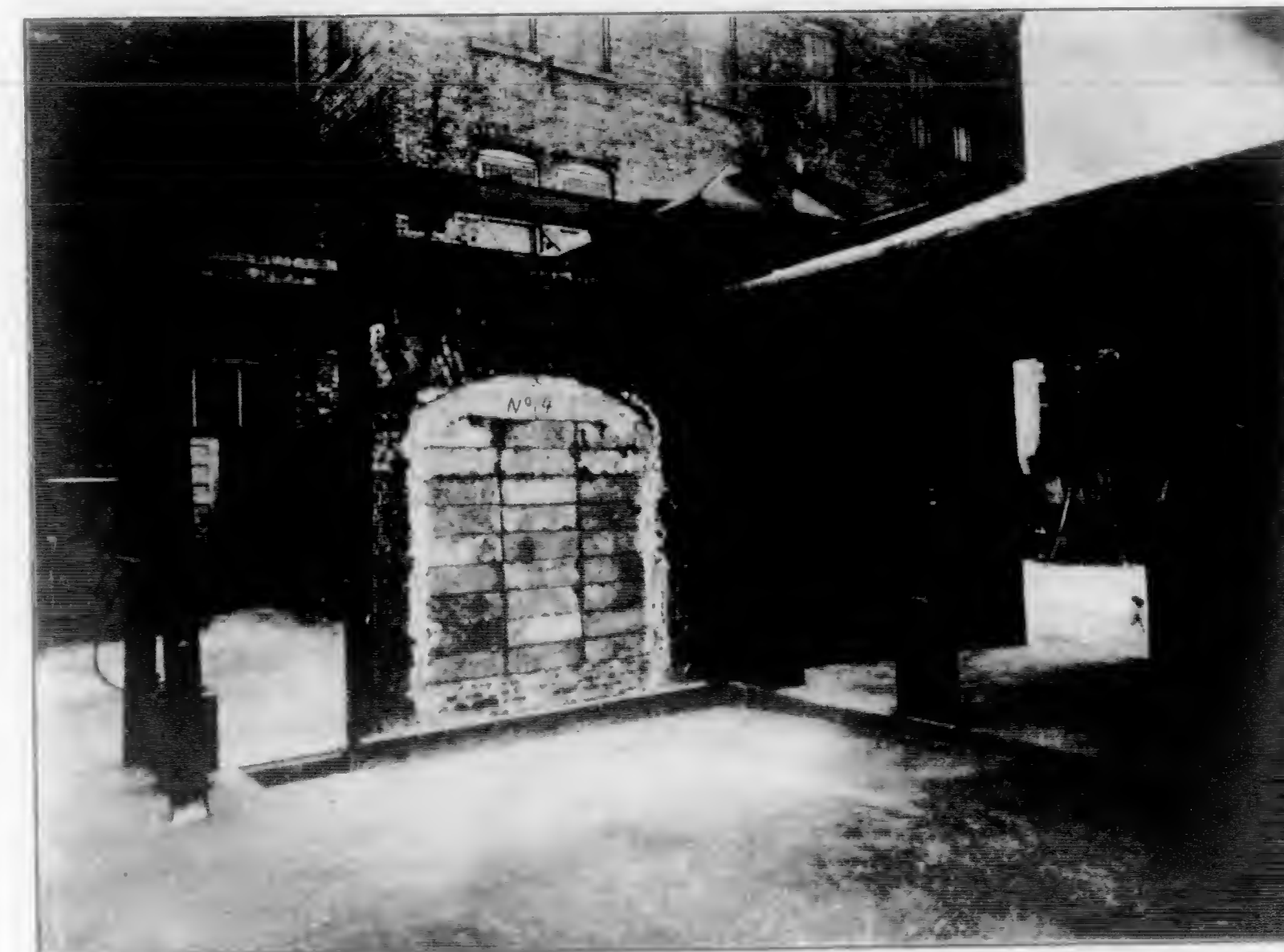
Fig. 5. Testing Fireproofing Qualities of Concrete
