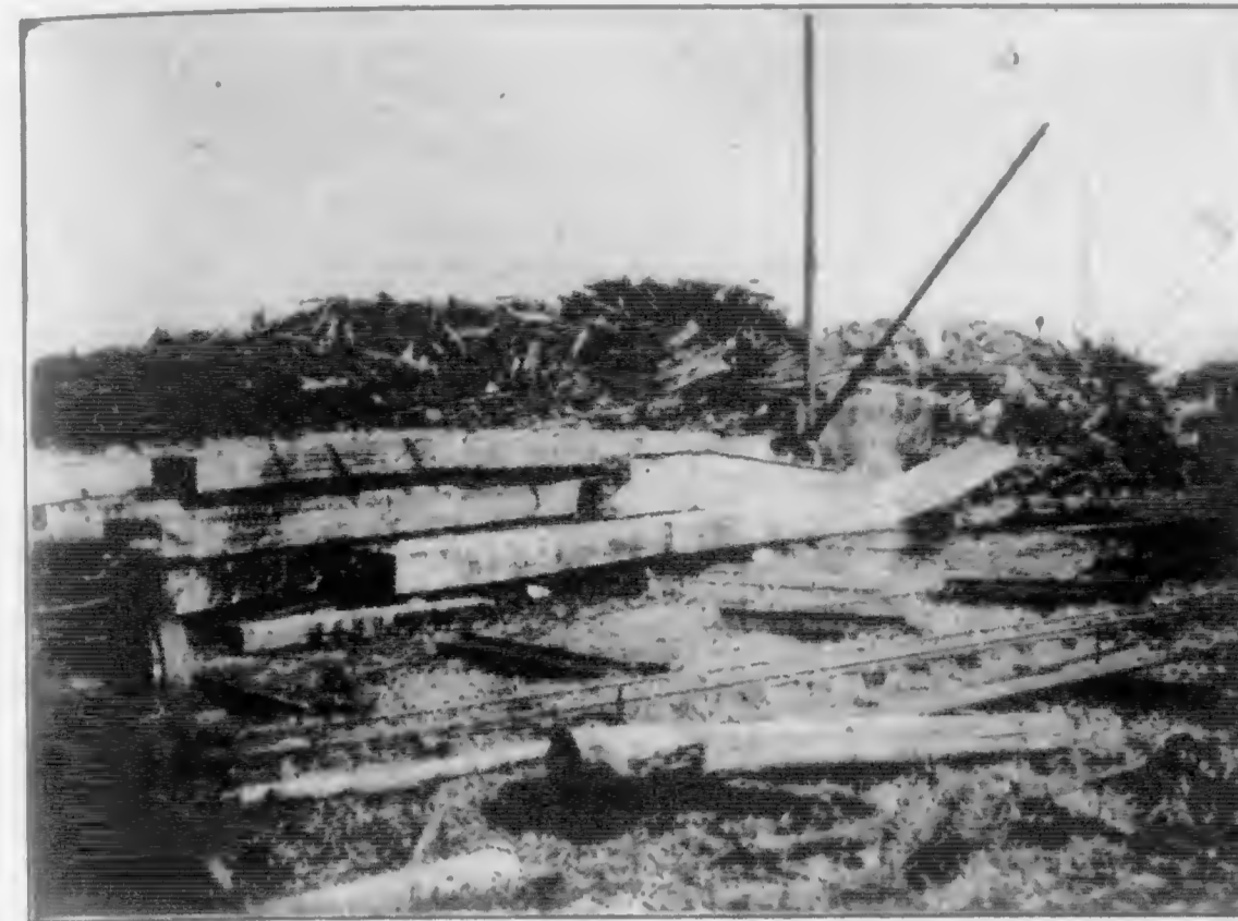
Fig. 5. Another View of Fig. 4 Showing Old Palace Hotel Girders in the Foreground
