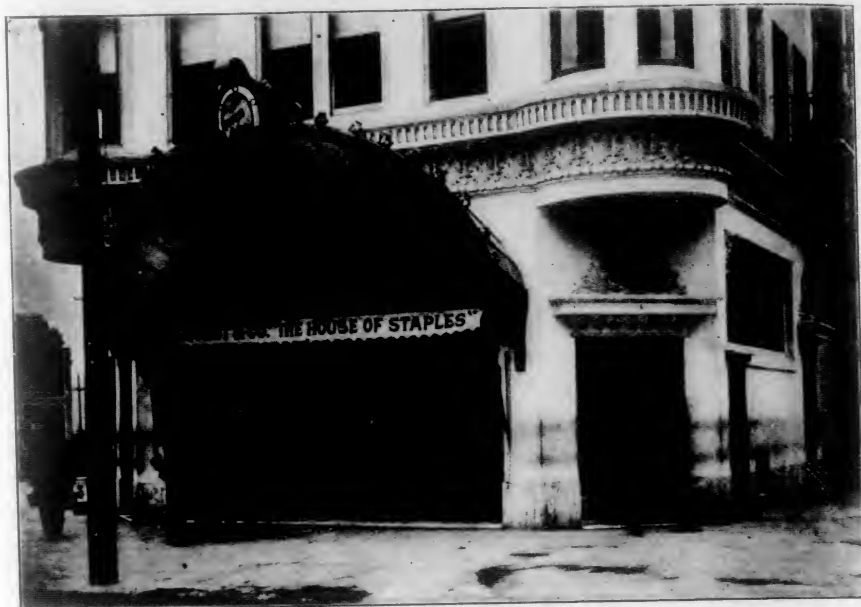
Detail of Flannery Building Art Metal Canopy by Chr. Deterding Ornamental Plastering by D. Ross Concrete Work by Victor Stanquist Clark
