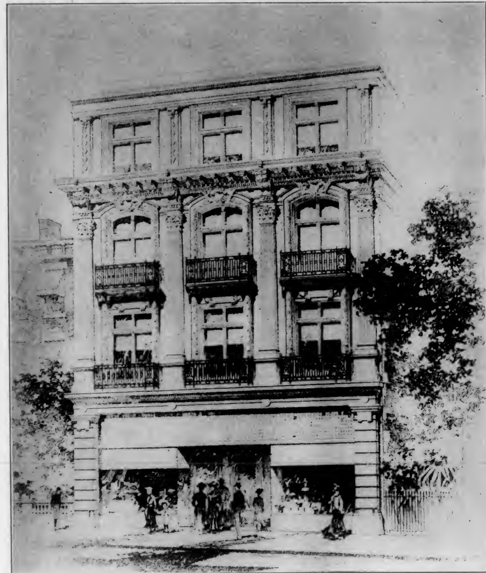
Building for F. M. Green, San Francisco Houghton Sawyer, Architect
