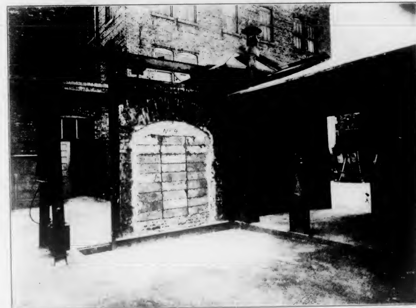
Fig. 5. Testing Fireproofing Qualities of Concrete
