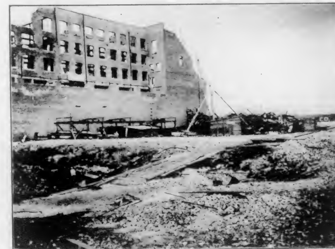
Fig. 2. Showing Wall of Emporium Building; Also, Steel Pile and Work Shop at a Distance
