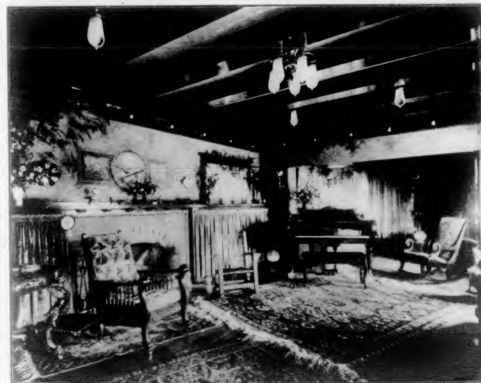
Living Room, Residence of Mr. Frank K. Wilson, Los Angeles Hunt and Eager Architects
