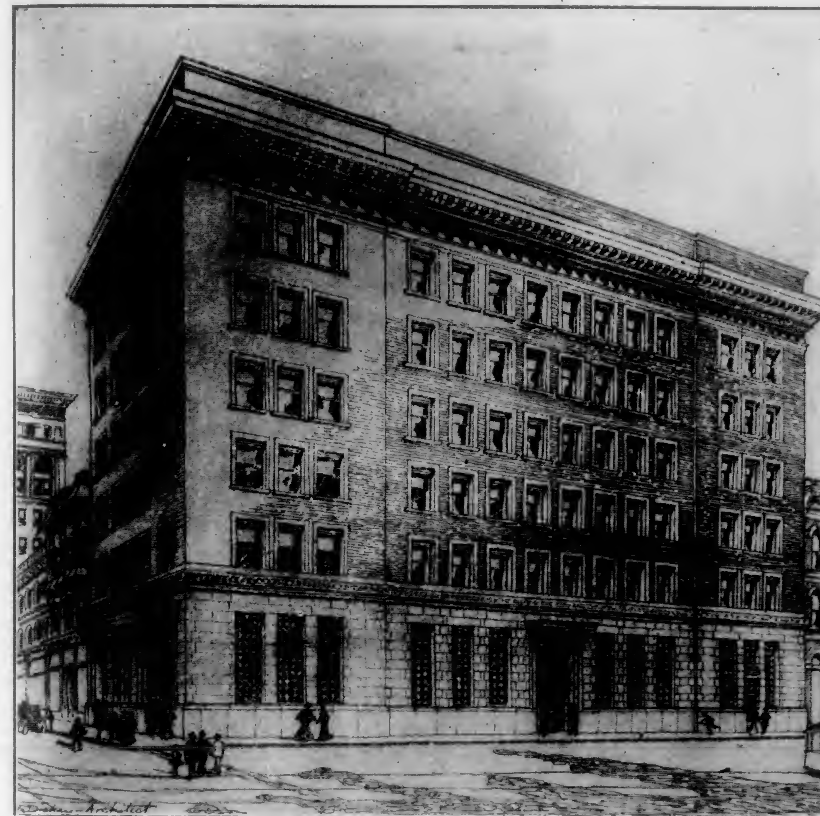
Six-Story Steel and Brick Building of the Oakland Bank of Savings—C. W. Dickey, Architect
