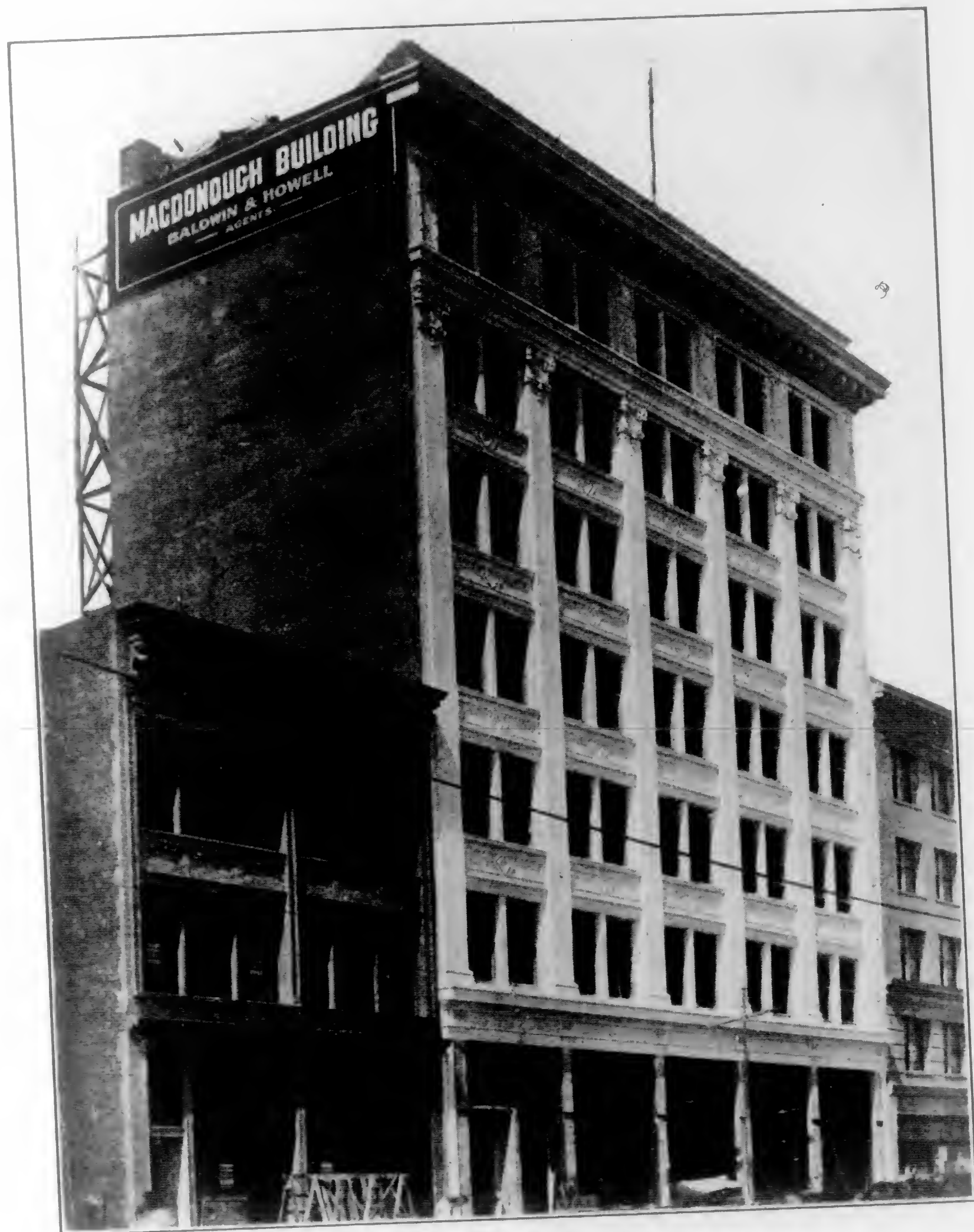
The Macdonough Building, San Francisco William Curlett, Architect John B. Leonard, Engineer Equipped with Otis Elevators Thompson-Starrett Co., Contractors
