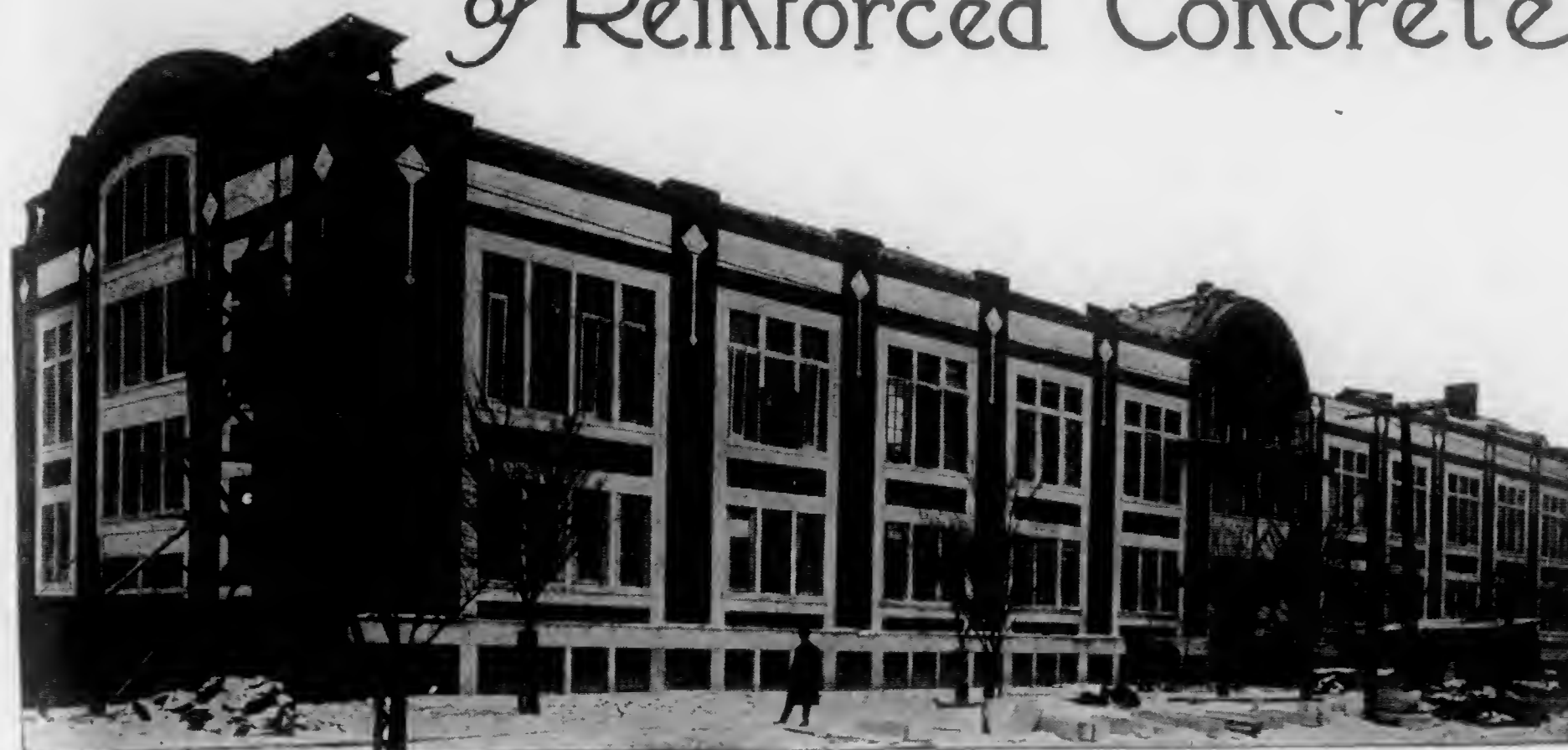
The Administration Building of the Geo. N. Pierce Manufacturing Plant at Buffalo taken during the process of construction. This immense plant, having over 325,000 square feet of floor space, was built throughout according to the Kahn System of Reinforced Concrete.
