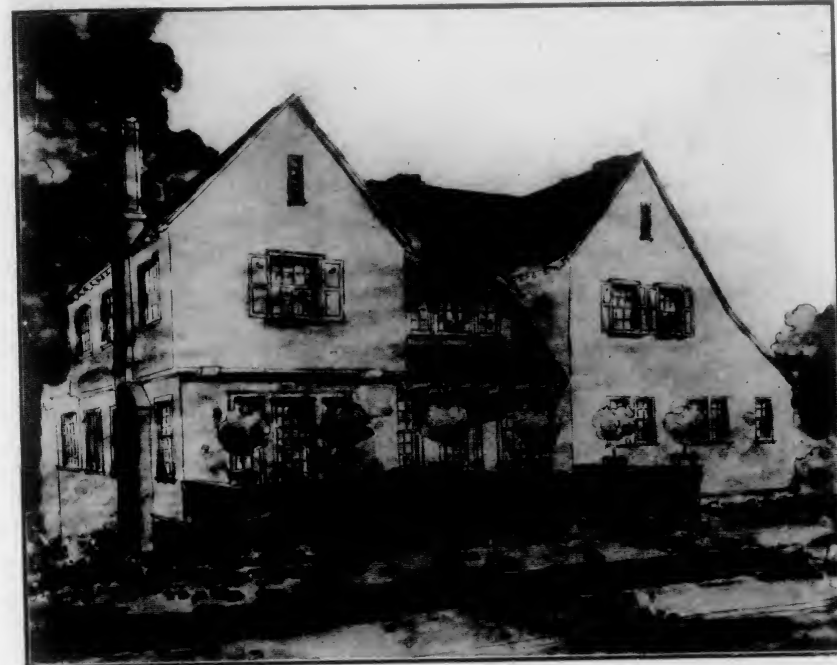
RESIDENCE OF MR. F. A. WEBSTER, OAKLAND. C. W. DICKEY, Architect
