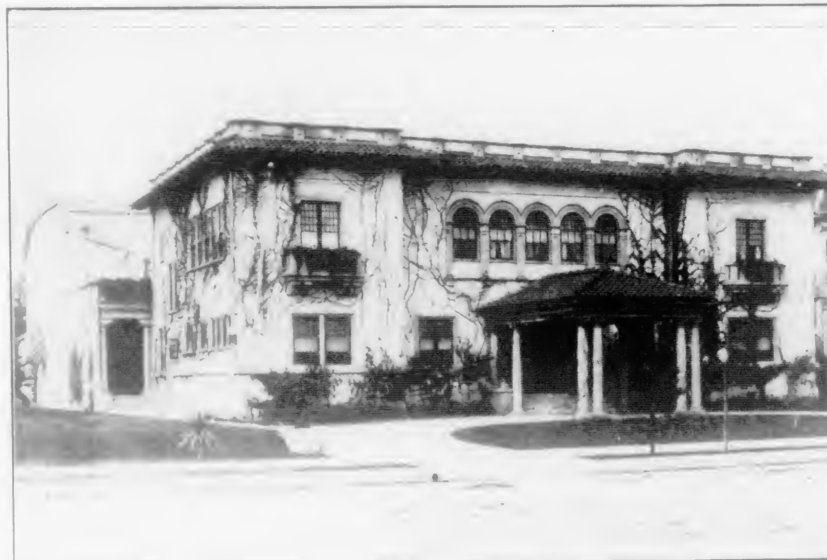
Elks Club Building, Los Angeles Hunt and Fager Architects
