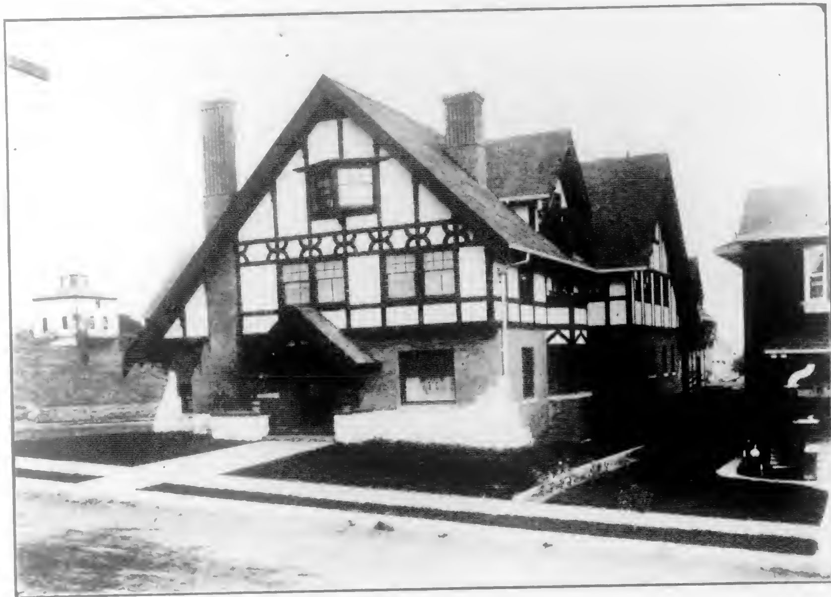
Residence of Mr. F. J. Stanton, Los Angeles Hunt and Eager, Architects
