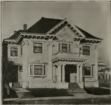
Four Six-Room Flats for Mrs. R. McCall, Oakland C. W. McCall, Architect
