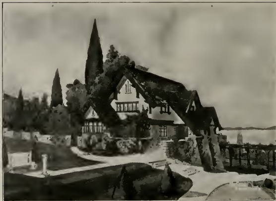
Study of House and Grounds for Mr. W. A. Stephenson, Piedmont C. W. McCall, Architect
