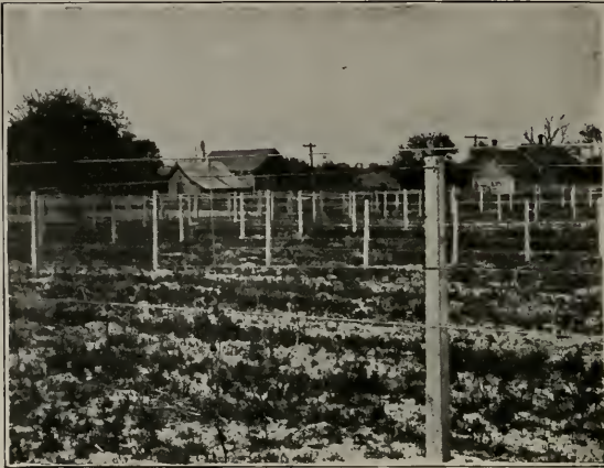
Concrete Posts for Fence and Vineyard Use
