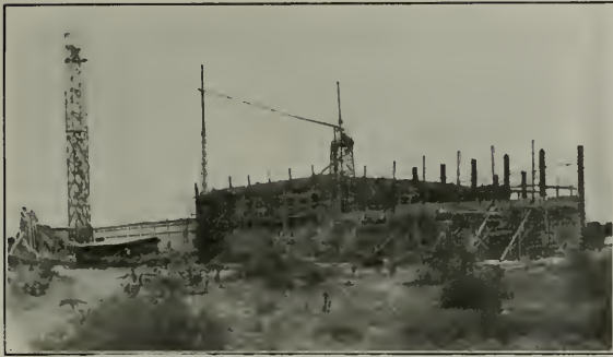
Freezing Ice Plant for Santa Fe Railroad, San Bernardino, California Showing Gravity System Delivering Concrete 302 Feet From the Mixing Plant
