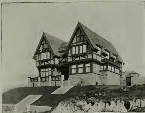
Residence of Mr. George Hatch, Oakland, California
