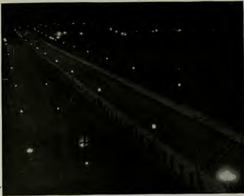
Fig. 2—Night Scene on the Harrisburg Bridge. Note the Absence of Shadows Along the Entire Bridge. Compare the Effect of the Diffused Light with the Concentrated Glare and Surrounding Blackness as Indicated by the White Spots Which Are Arc Lamps in the Railroad Yards in the Background.
