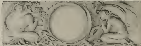
Figures Executed in Ornamental Plaster in Bank of Italy Building, San Francisco. Shea & Lofquist, Architects
