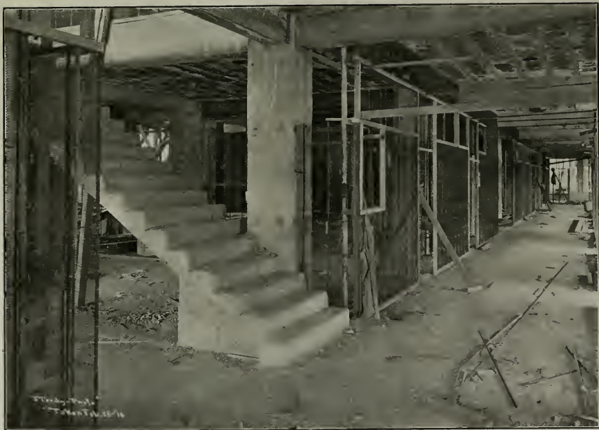
Photo Showing Metal Partitions Before Plastering
