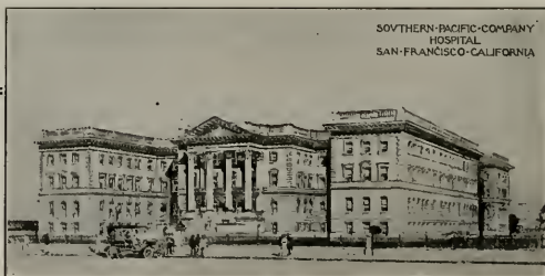
This cut shows the new Southern Pacific Co.'s Hospital, D. J. Patterson, Architect, as it will look when the west wing is completed. The main building, east wing, annex, and the power house are all faced with "Golden Gate Sandstone" brick, made of sand and lime at Antioch. The new wing will require 250,000 of these brick for the facing. You know the Southern Pacific Co. buys the best of materials, hence our brick were specified. We also manufacture at Stockton all kinds of Clay-Faced brick—Enamel, Mat Glazed, Buff, and Fire. GOLDEN GATE BRICK CO., 660 Market St.
