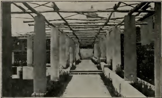
Concrete Pergola in Southern California
