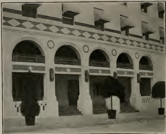
Hotel Sacramento. Detail of Main Entrance
