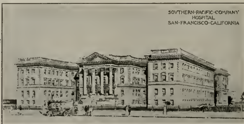
This cut shows the new Southern Pacific Co.'s Hospital, D. J. Patterson, Architect, as it will look when the west wing is completed. The main building, east wing, annex, and the power house are all faced with "Golden Gate Sandstone" brick, made of sand and lime at Antioch. The new wing will require 250,000 of these brick for the facing. You know the Southern Pacific Co. buys the best of materials, hence our brick were specified. We also manufacture at Stockton all kinds of Clay Pressed brick—Enamel, Mat Glazed, Buff, and Fire.
