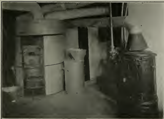
Furnace Room in Residence of Dr. Murray L. Johnson, Piedmont, California, Showing Torrid Zone Furnace and Humphrey Automatic Water Heater
