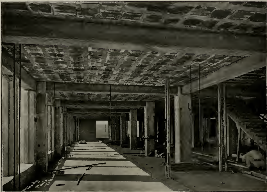
Thomas Higgins Building—Showing Tile Construction After Forms Were Removed on Second Floor
