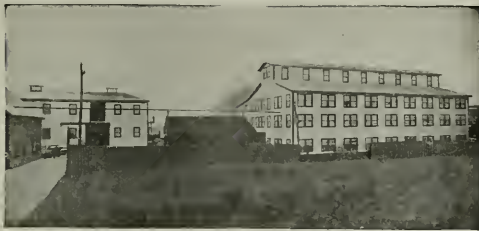
Plant of Woburn Machine Company, Woburn, Mass., showing fire proof and fume-proof roofing and siding of ASBESTOS PROTECTED METAL
