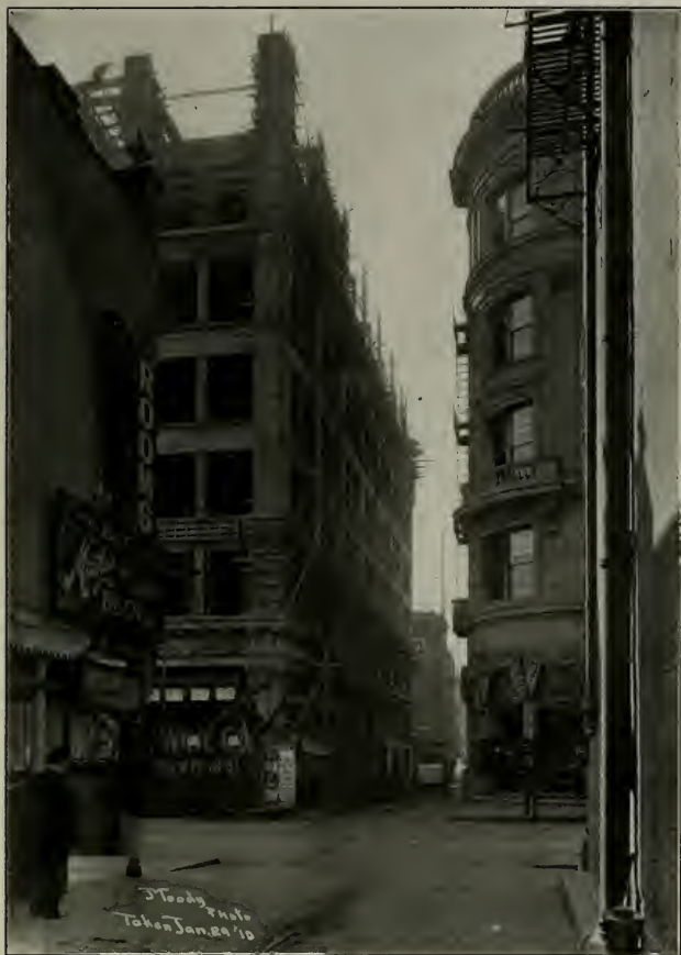
Thomas Higgins Building in Course of Construction
