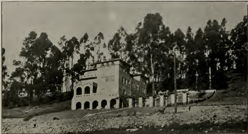
House and Pergola of Mr. R. L. Johns, Piedmont, Cal.
