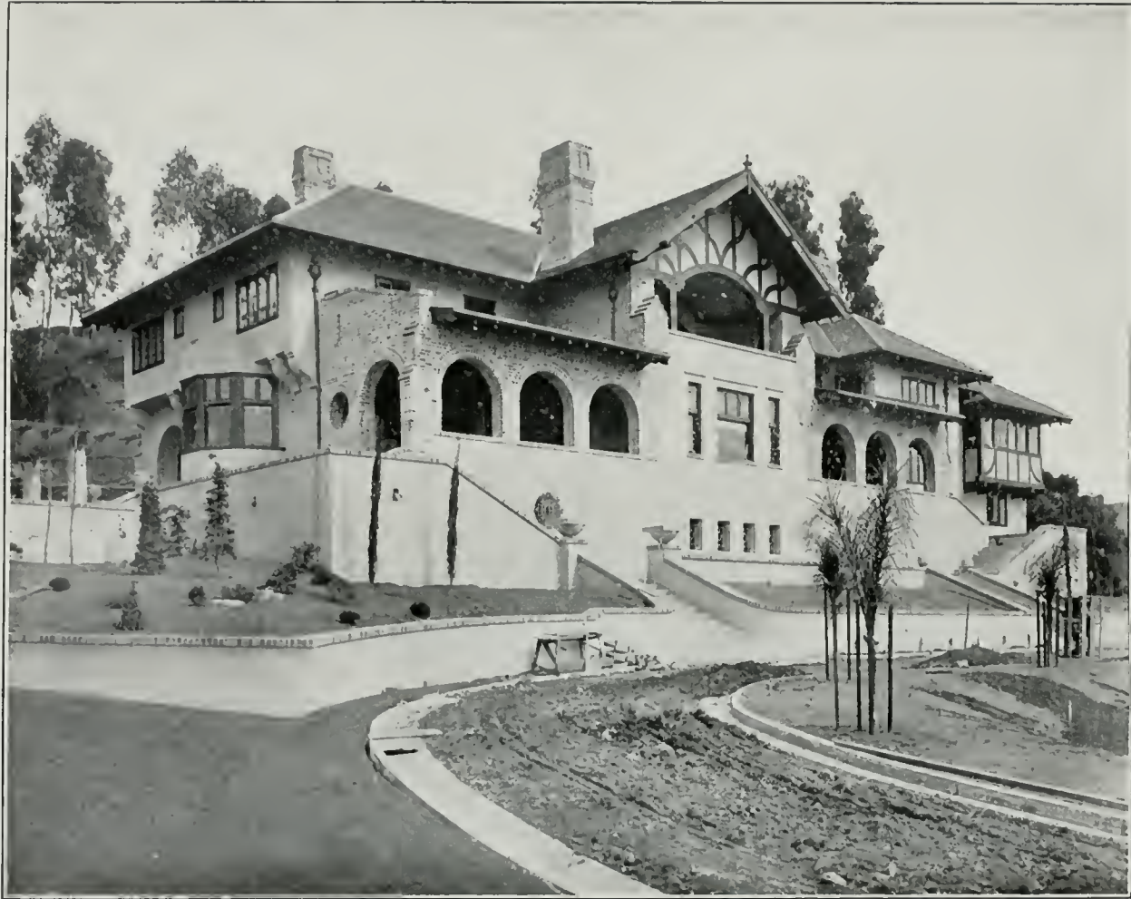
J. L. Groux Residence, Hollywood, Cal. Frederick L. Roehrig, Architect 25,000 Tan Ruffled Brick, 45,000 Shingle Roof Tile, furnished by Los Angeles Pressed Brick Co.
