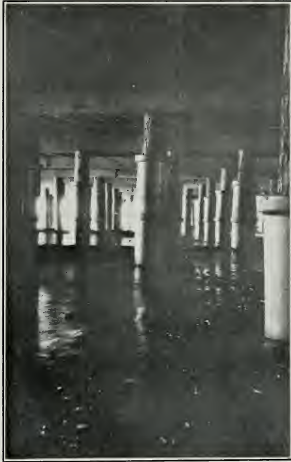
Clay Pipe Used to Protect Piles from Parasites
