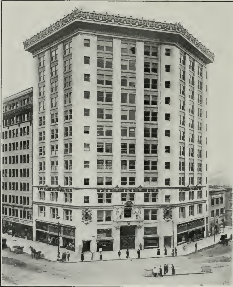
Hearst Building, San Francisco. James C. Green, Architect White Matt Enamel Terra Cotta with Polychrome Treatment at Entrances and Lower Stories
