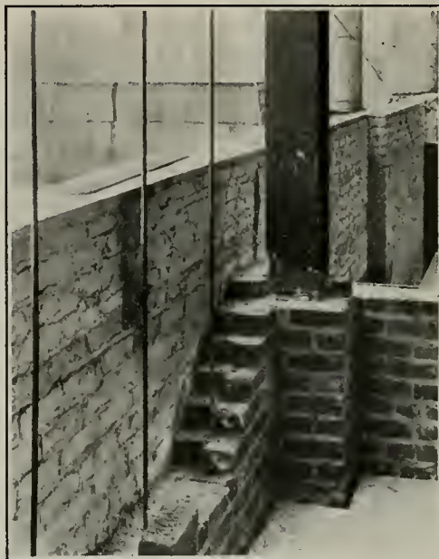
REINFORCED BRICK CURTAIN WALL
