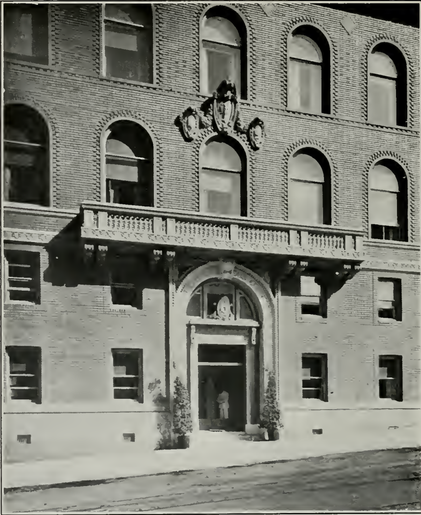
Entrance University Club, San Francisco. Bliss & Faville, Architects Dark Buff Standard Terra Cotta
