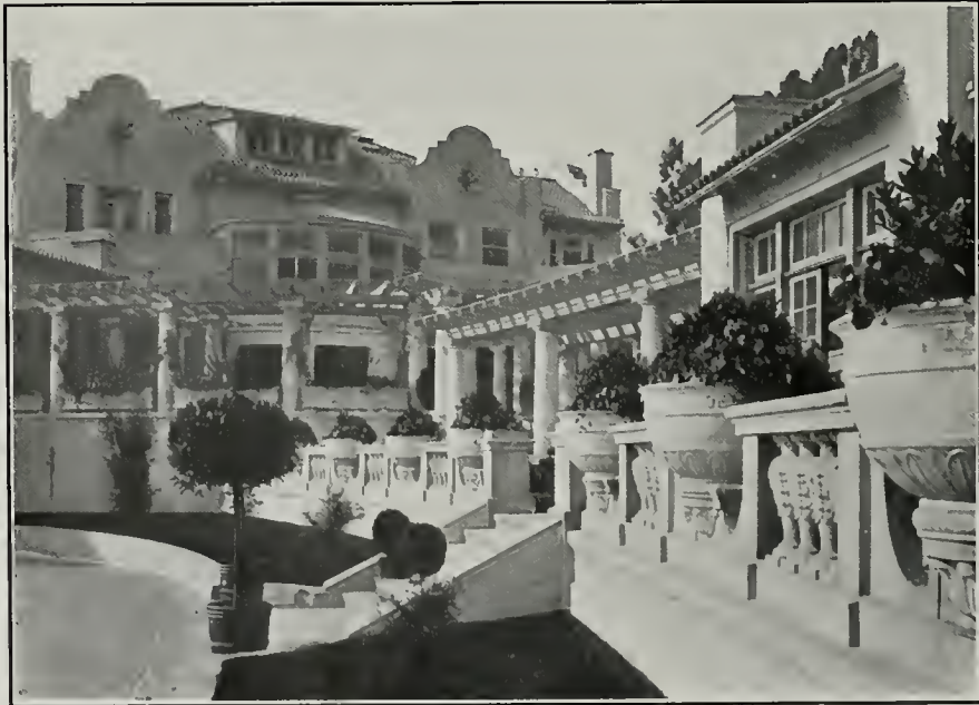
Showing Pergolas and Mission Tile Roof of the Hart Residence, Claremont. C. W. Dickey, Architect
