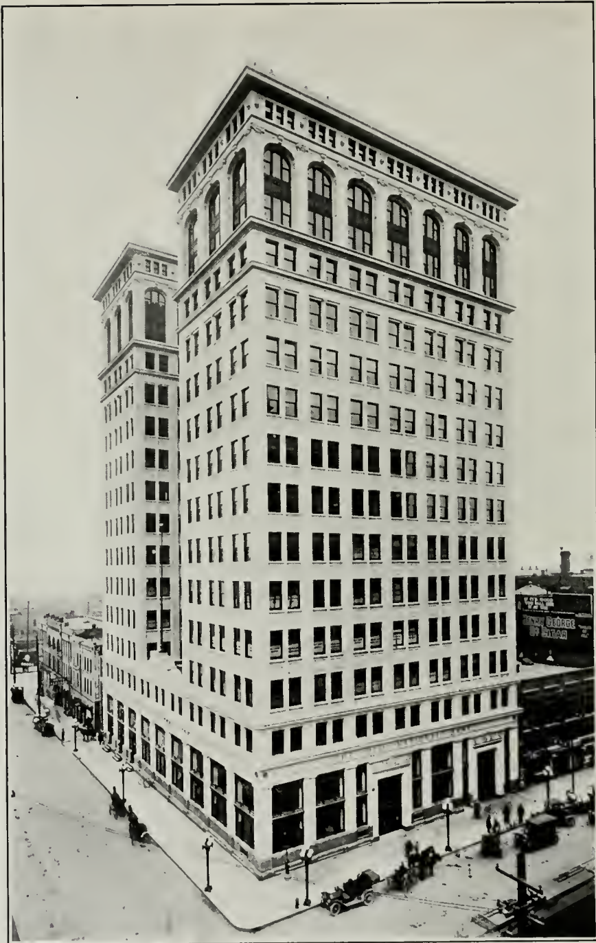
OLD NATIONAL BANK BUILDING, SPOKANE, WASHINGTON D. H. Burnham & Co., Architects Cream White Matt Enamel Terra Cotta
