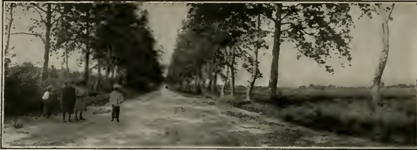
Oakland Road, California. Richmond Road Oil used as a binder.
