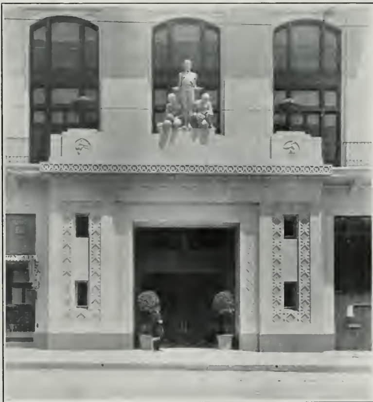
Entrance to Los Angeles Athletic Club Building. Parkinson & Bergstrom, Architects Architectural Terra Cotta by Gladding, McBean & Company
