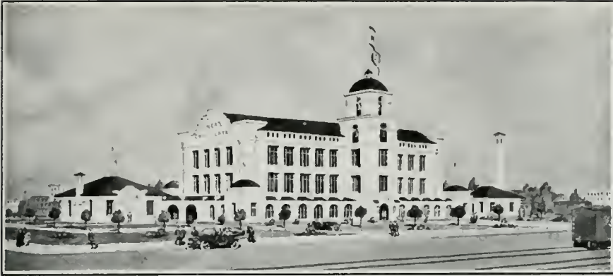
California Mission Style of Architecture Followed in Design for Eastern Chocolate Factory Sidney B. Newsom, Architect
