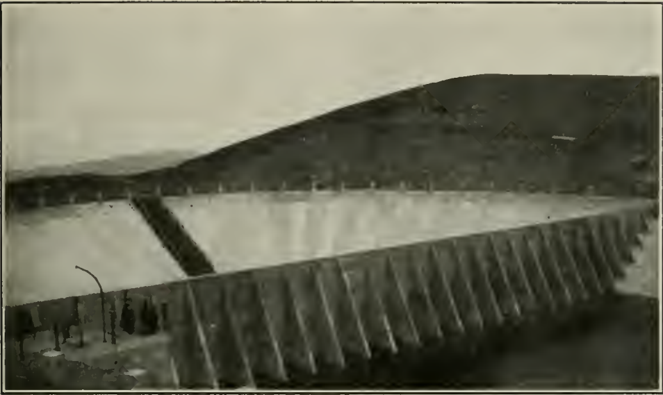
Twin Peaks Concrete Reservoir, San Francisco
