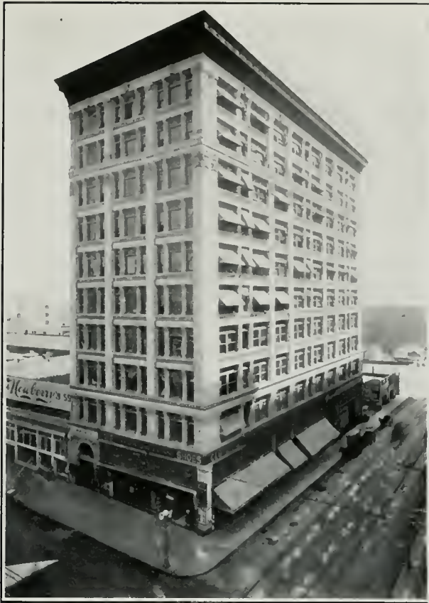
Kerckhoff Building, Los Angeles. Morgan & Walls, Architects Cream White Matt Enamel Terra Cotta
