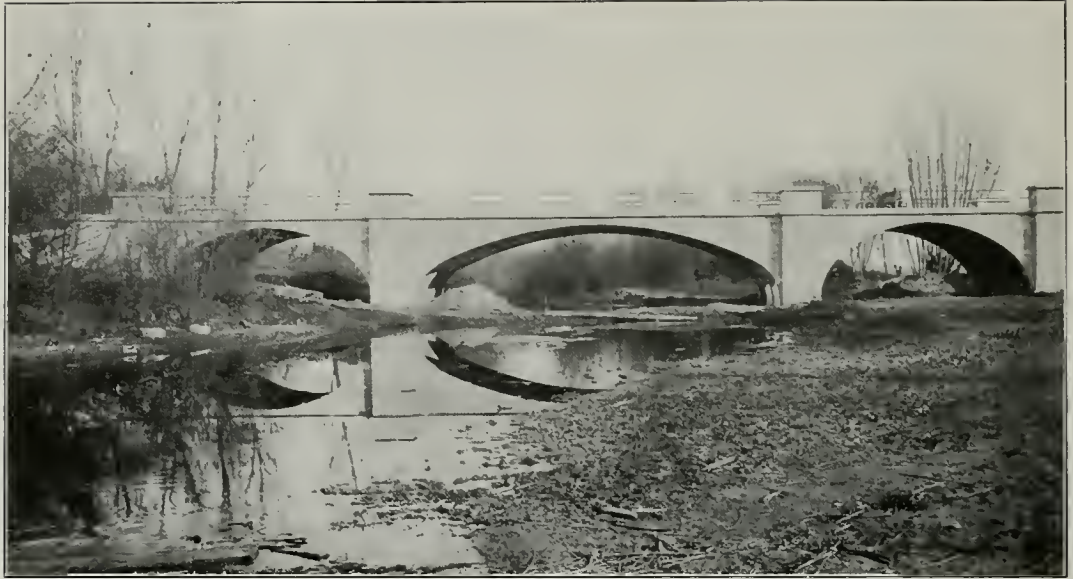
Reinforced Concrete Bridge, Santa Clara County, California Designed by J. G. McMillan, C. E.
