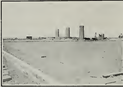
General View of Plant
