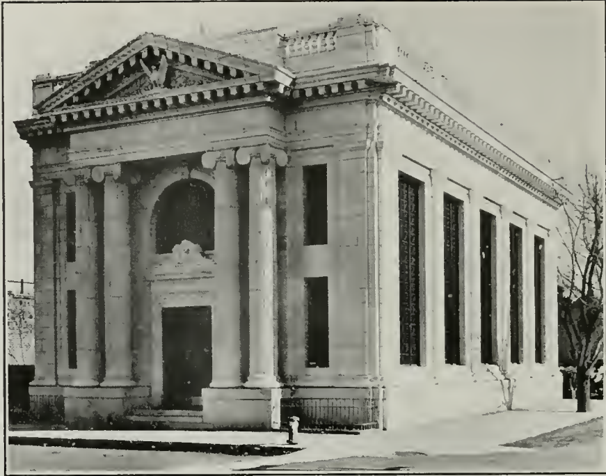
Citizens Bank of Winters, California. Walter H. Parker, Architect Exterior of White Matt Glazed Architectural Terra Cotta Executed by N. Clark and Sons Photo by Walter H. Scott
