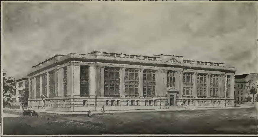
Girls' High School Building, San Francisco, in which the California Air Purifying Co.'s Air Washer and Cooler have been installed.
