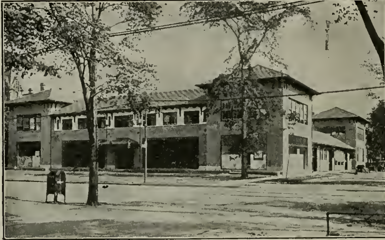
Ferrosinclave was used for Roof of this Garage
