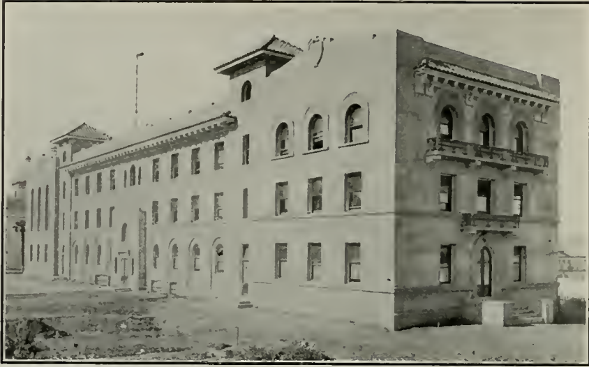
One of the Completed Santa Clara University Buildings, Built of Reinforced Concrete. W. D. Shea, Architect
