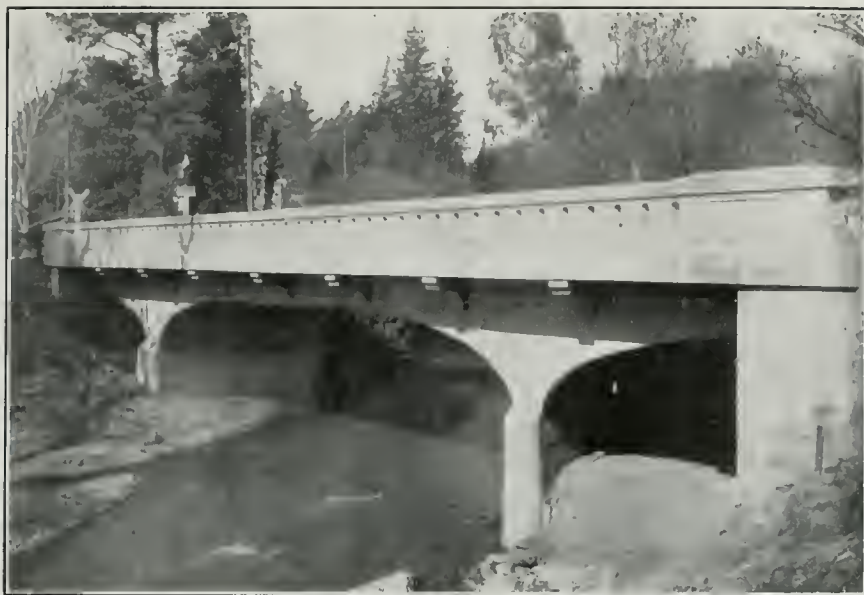
Reinforced Concrete Girder Bridge, City of Ross, Marin County, California
