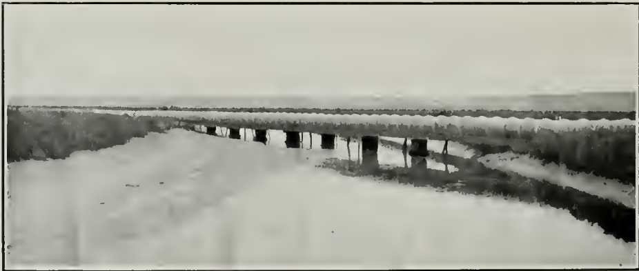
Cut Shows Vitrified Clay Pipe Line Built Above Ground
