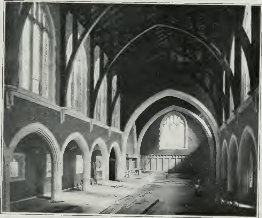
Interior St. Pauls Church Finished in Richmond Red Pressed Brick
