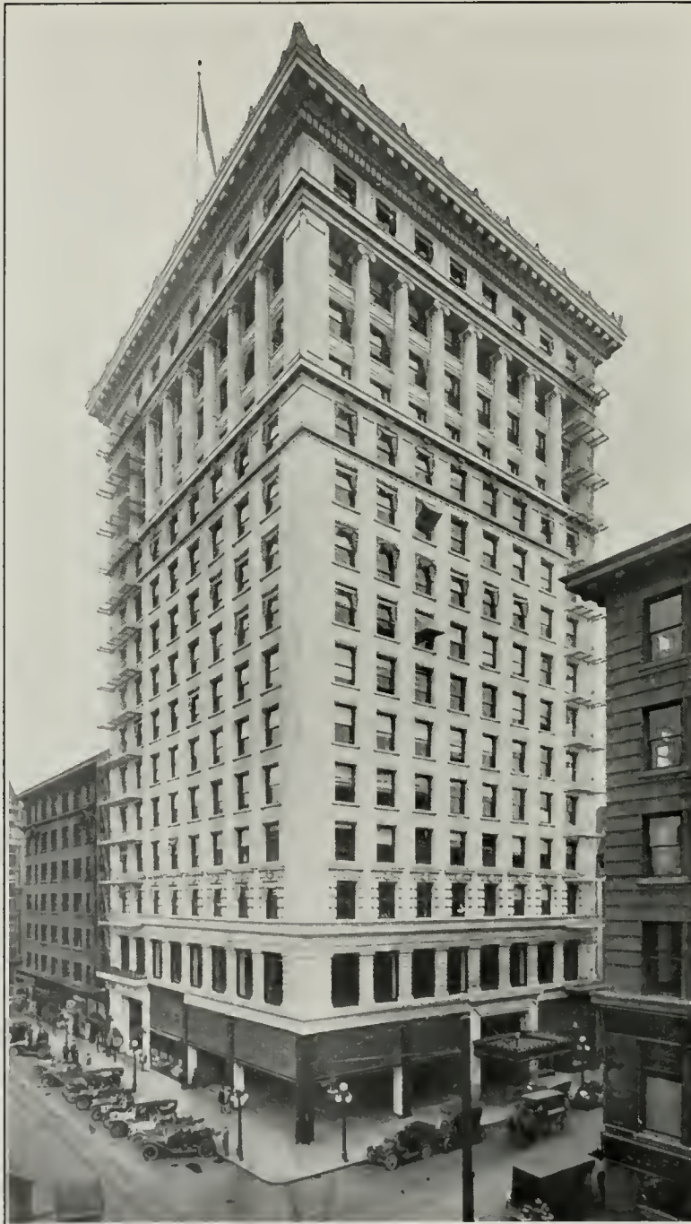
Yeon Building, Portland, Oregon. Reid Bros., Architects White Matt Enamel Terra Cotta
