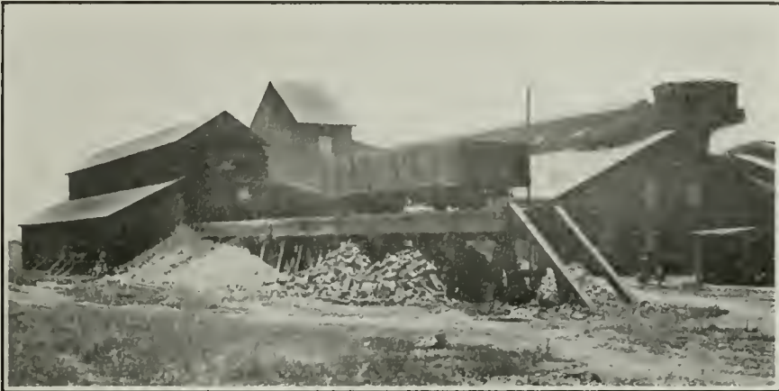
General View of LIVERMORE FIRE BRICK COMPANY'S Factory Livermore, California
