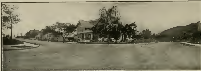
Claremont Court, Berkeley, Cal. Richmond Road Oil used as a binder.
