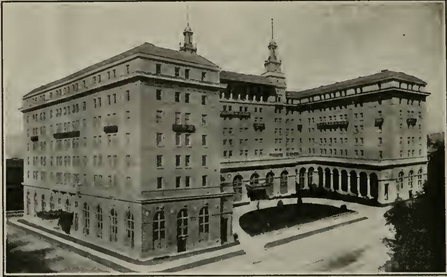
View of the Oakland Hotel, in which two large size Double Deck "New Era" bread and pastry ovens have just been installed. Jarvis Oil Burner used to operate.
