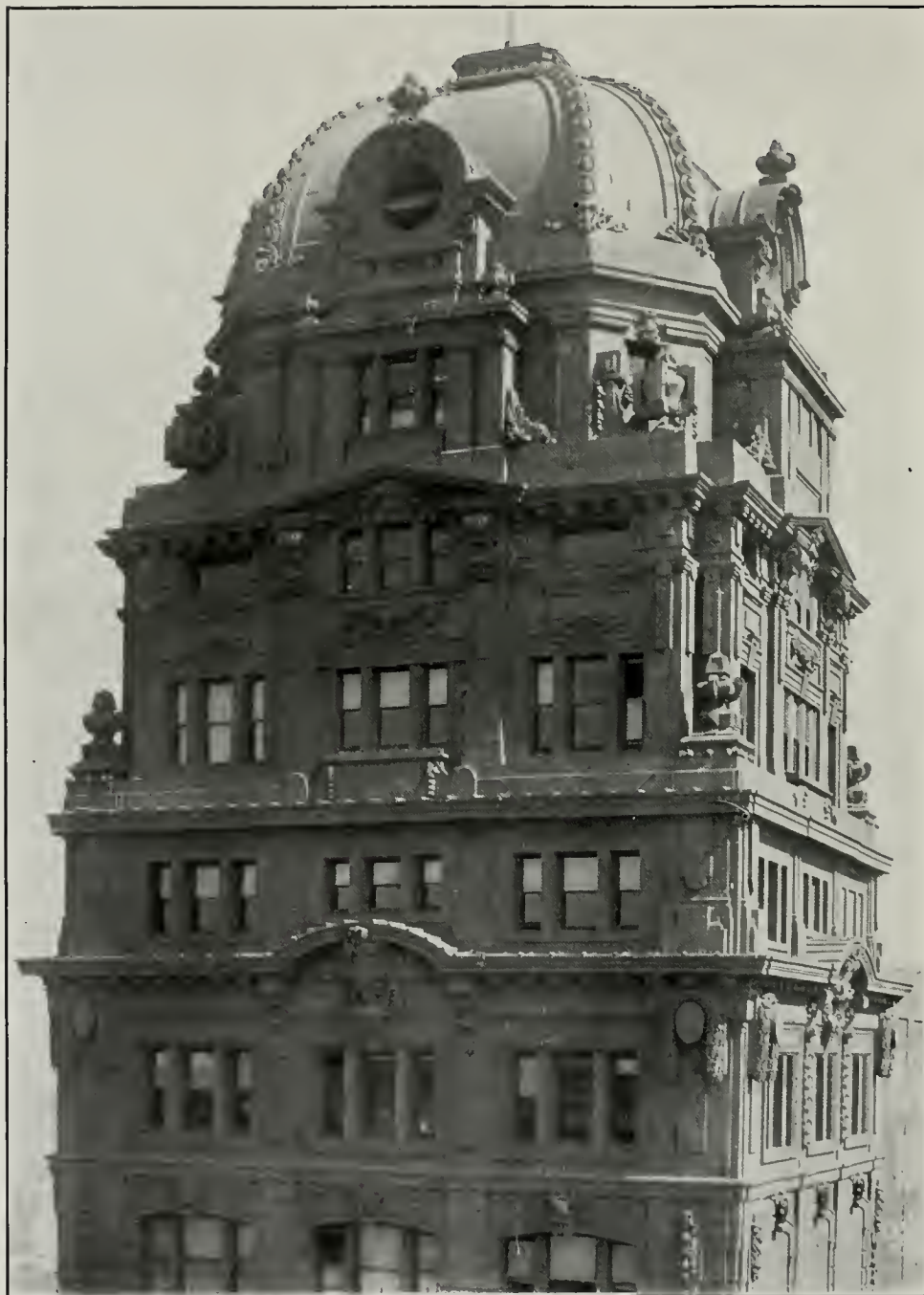
Detail of Upper Stories and Dome of Humboldt Bank Building, San Francisco Frederick H. Meyer and Smith O'Brien, Architects Terra Cotta by Steiger Terra Cotta and Pottery Works
