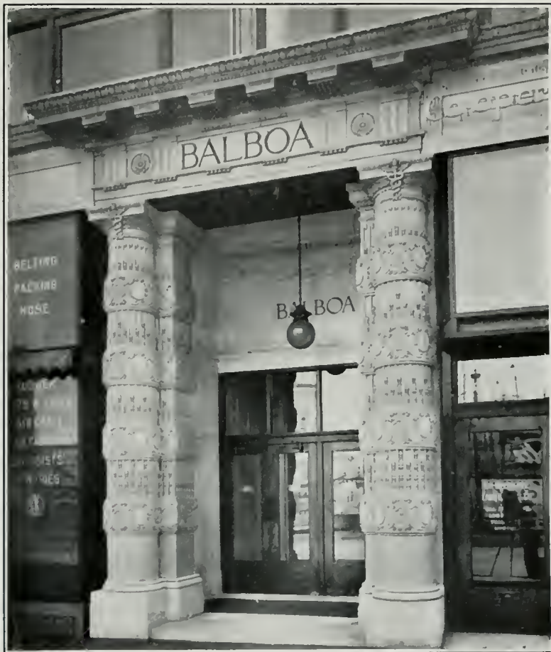
Entrance Balboa Building, San Francisco. Bliss & Faville, Architects Standard Terra Cotta in Dark Buff
