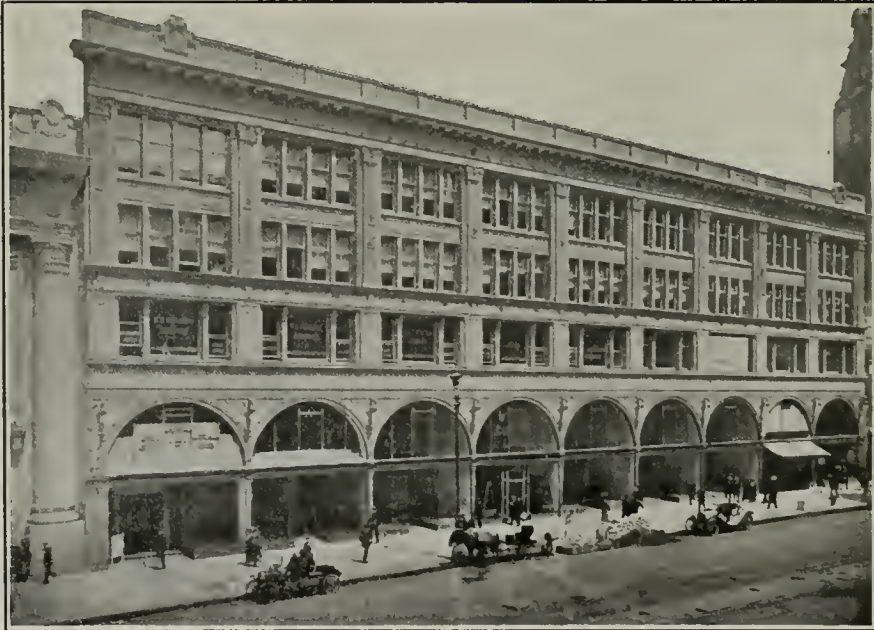
BANKERS INVESTMENT BUILDING
