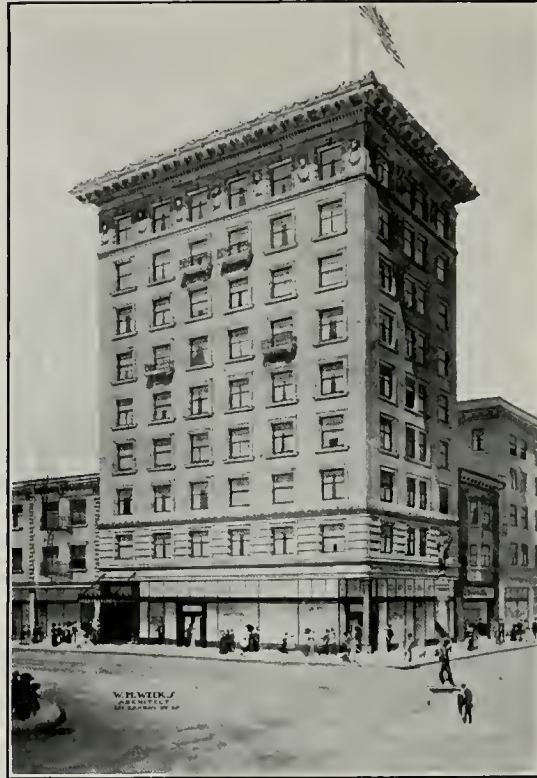
St. Francis Realty Co. Building, San Francisco. William H. Weeks, Architect Exterior Finished in White Matt Glazed Terra Cotta and Cream Pressed Brick by N. Clark and Sons
