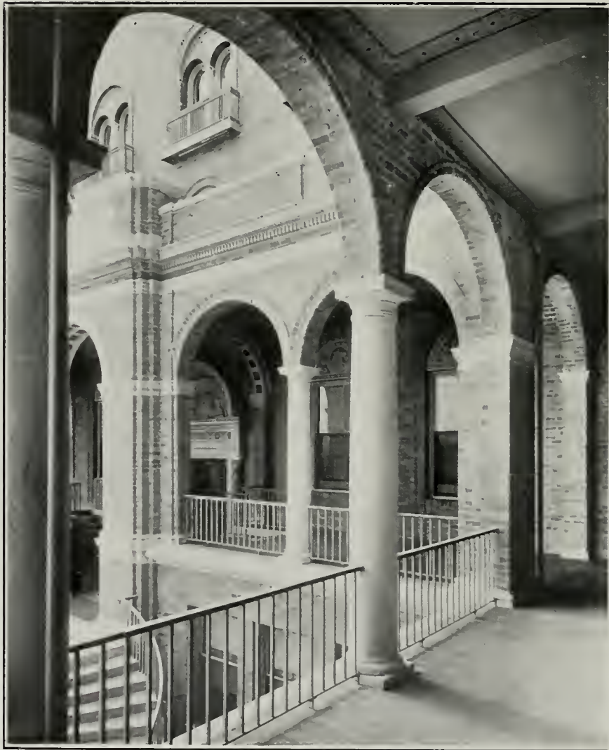
Colonnade and Portico Entrance, Children's Hospital, San Francisco Bliss & Faville, Architects
