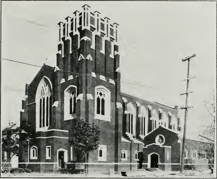
St. Pauls Episcopal Church, Oakland. Benj. G. McDougall, Architect Richmond Red Ruffled Brick
