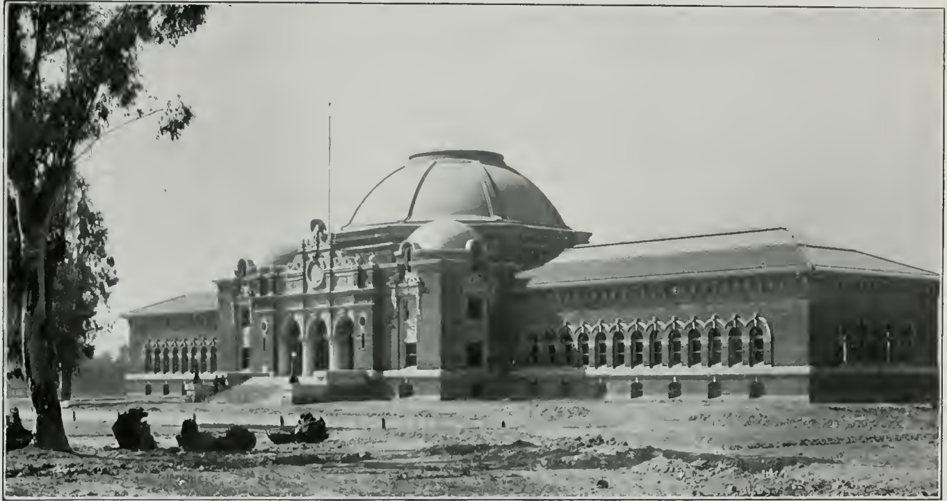
County Museum Building, Exposition Park, Los Angeles, California. 200,000 Red Ruffled Brick—1,500,000 Hollow Common Brick—110 Squares of Red Spanish Roofing Tile furnished by Los Angeles Pressed Brick Co.
