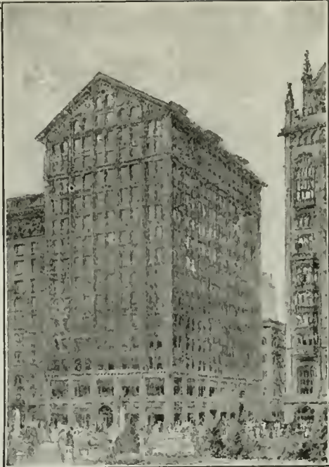
THE NEW MONROE BUILDING, CHICAGO Basement Waterproofed with Ceresit
