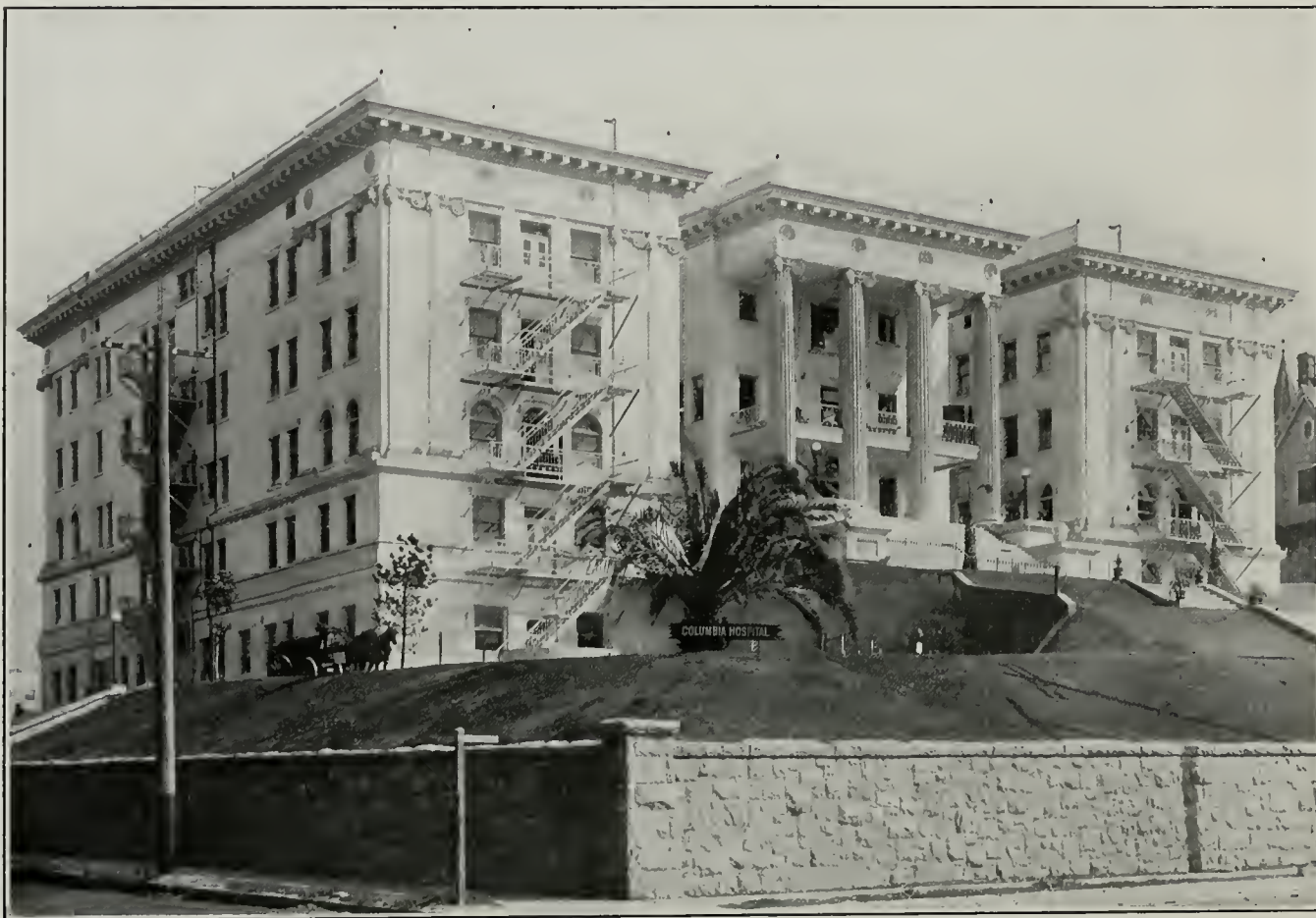
Columbia Hospital Building, Built by General Osteopathic Association, Los Angeles, Cal. Norman F. Marsh, Architect. About 1000 Tons of Hollow Tile and 175,000 Enameled Brick furnished by Los Angeles Pressed Brick Co.
