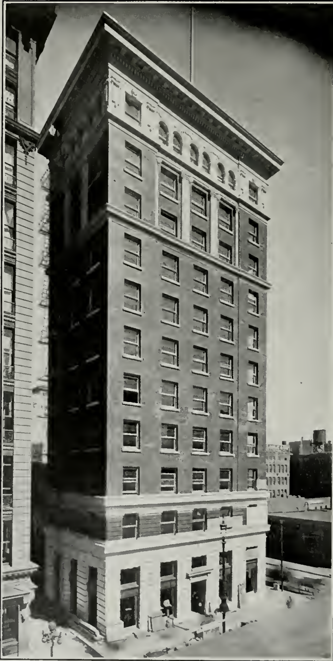
California Pacific Building, San Francisco. Reid Bros. Architects Finished in Richmond Red Pressed Brick furnished by United Materials Company
