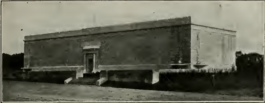
Spring Valley Water Co., Sloat Boulevard Pumping Station Willis Polk, Architect
