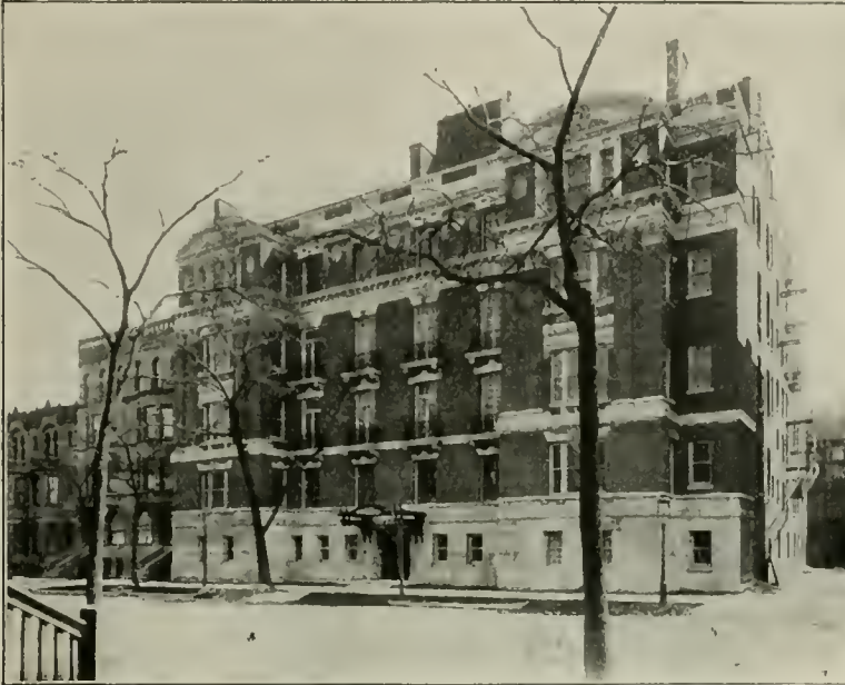
NEW APARTMENT BUILDING, CHICAGO. FLOOR OF LAUNDRY ON FIFTH FLOOR. Waterproofed with CERESIT Waterproofing.
