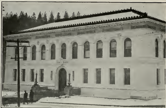
El Dorado County Court House, Placerville, California Clarence C. Cuff, Architect
