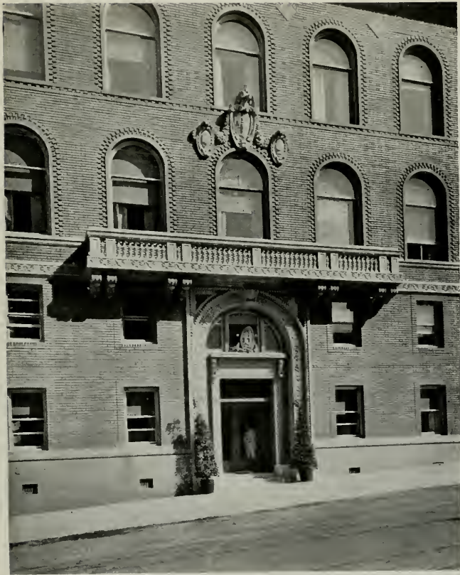
DETAIL, UNIVERSITY CLUB BUILDING SAN FRANCISCO
