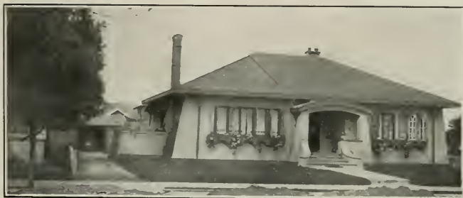
Good Design for a Plaster Bungalow, San Jose William Binder, Architect
