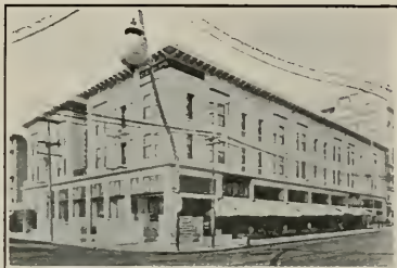
St. Albans Apartments, San Francisco. Reid Bros., Architects.
