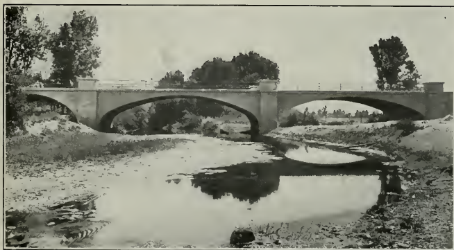
Concrete Bridge on the San Jose-Oakland Road Over Coyote Creek. Three 70-Foot Spans J. G. McMillan, Engineer
