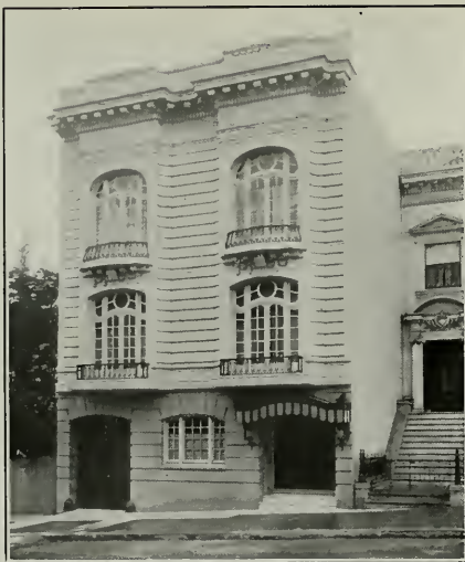
Double Residence for Dr. J. E. Artigue, San Francisco Righetti & Headman Architects
