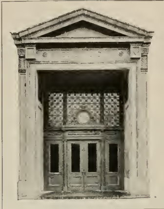
Cast Iron Entrance and Bronze Doors. Lincoln High School, Portland, Oregon EXECUTED BY
