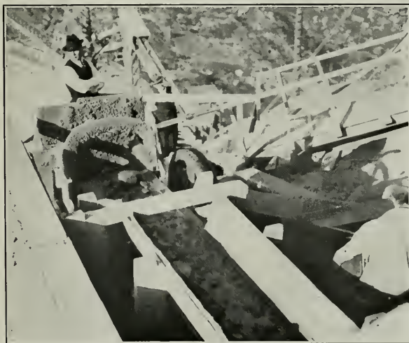
Belt Conveyor Discharging Wet Concrete—Speed 400 Feet Per Minute
