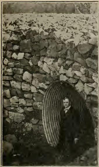
Ingot Iron Culvert
