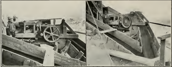
Belt Conveyor at Rest, Showing Wet Concrete on Belt
