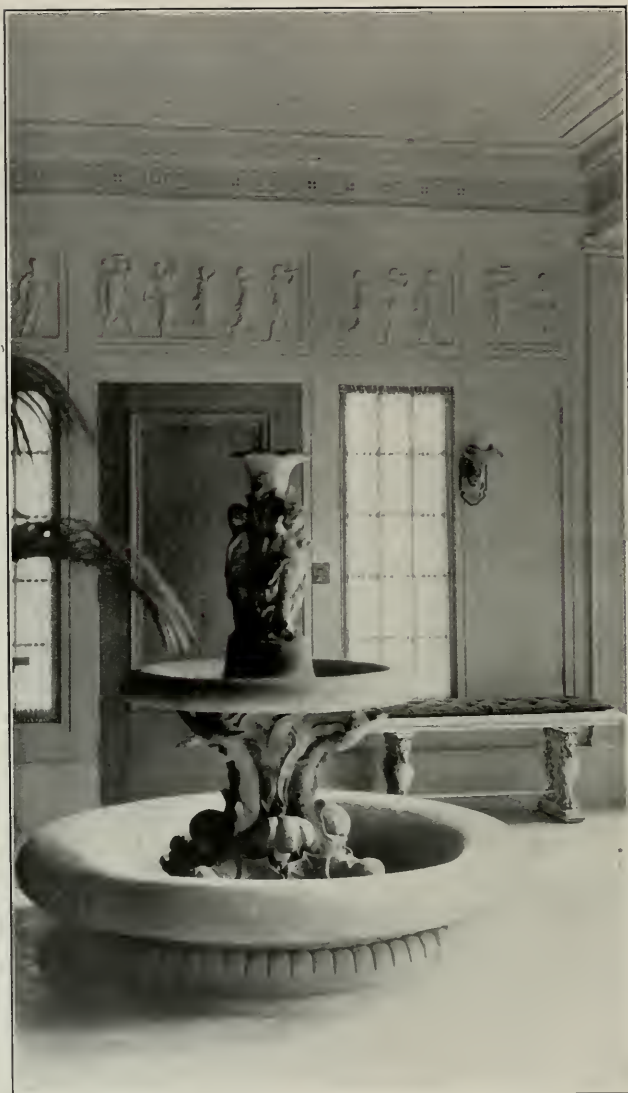
ENTRANCE COURT. RESIDENCE OF MR. J. B. CROWLEY West Clay Park, San Francisco Righetti & Headman, Architects
