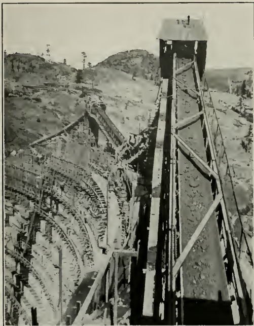
Belt Conveyor at Close Range
