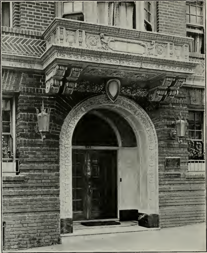
Detail Entrance Angelus Apartments Righetti & Headman, Architects
