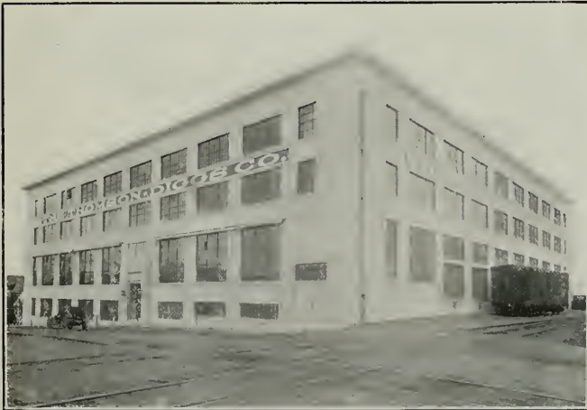
Reinforced Concrete Warehouse for the Thomson-Diggs Company, Sacramento Clarence C. Cuff, Architect
