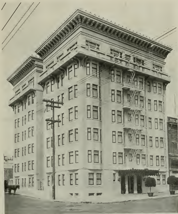
McKENZIE APARTMENTS, BUSH STREET AND VAN NESS AVENUE, SAN FRANCISCO
