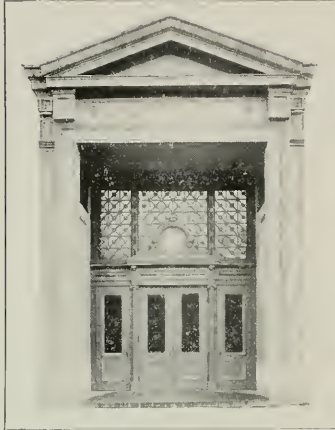
Cast Iron Entrance and Bronze Doors. Lincoln High School, Portland, Oregon EXECUTED BY
