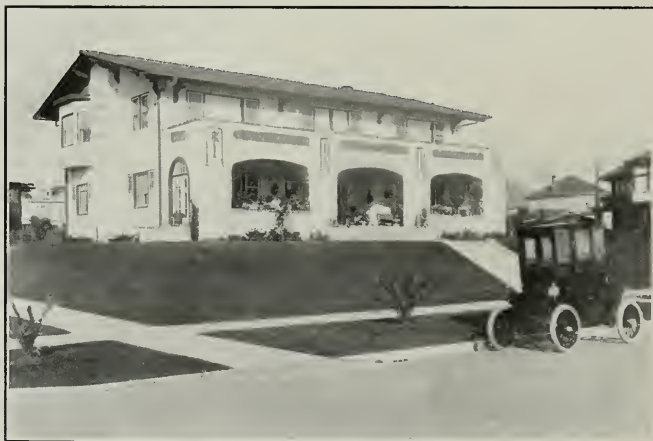
House of Mr. D. W. Cormichael, Sacramento Clarence C. Cuff, Architect
