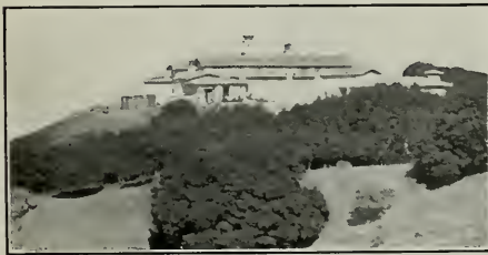
Henry W. Taylor Residence in the Berkeley Hills
