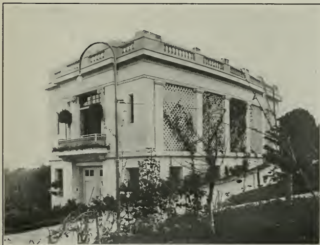
Concrete Garage for Mr. A. Schilling on Shore of Lake Merritt, Oakland Bluzome & Company, Builders
