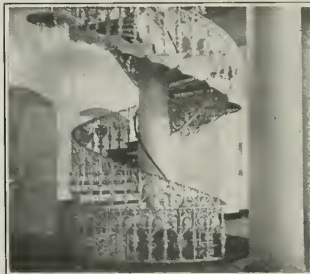
Circular Iron Stairs in Hall of Records, San Francisco Erected 1876
