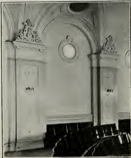
Corner of Ball Room and Auditorium, Native Sons' Building
