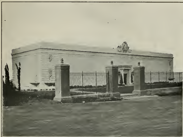
Pumping Station for the Spring Valley Water Company, Sloat Boulevard, San Francisco Built by Bluxome & Company
