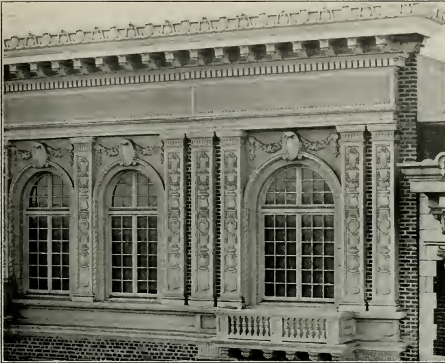
Detail Upper Story, Metcalfe Hotel, San Francisco
