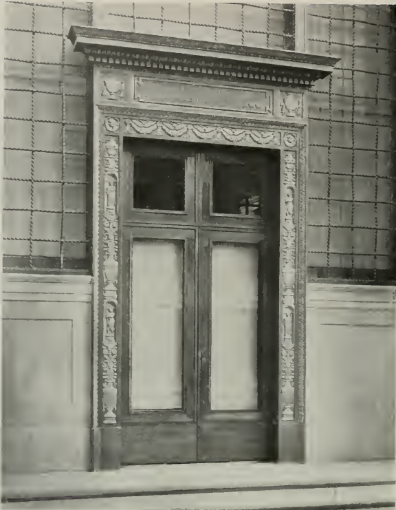
ENTRANCE DETAIL, LIVERPOOL AND LONDON AND GLOBE INSURANCE COMPANY'S BUILDING
