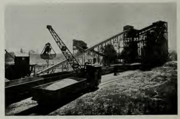
(Fig. D)-Port of plant of Niles Sand, Grovel & Rack Company, showing bunkers, loading facilities and locomotive crane in operation
