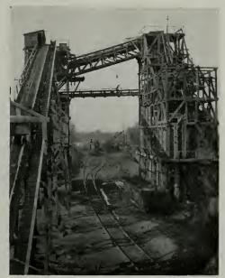
(Fig. A)-View of plant, showing belt-conveyor and storage bins
