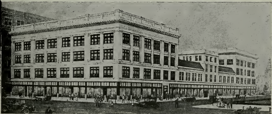
STORE AND OFFICE BUILDING, FOURTH AVENUE AND GUTHRIE STREET, LOUISVILLE ARTHUR LOOMIS AND JULIUS HARTMAN, ARCHITECTS
