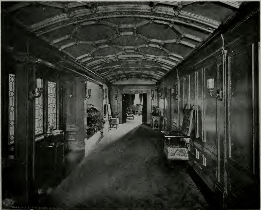
HALL, RESIDENCE OF MR. ALEX. D. KEYES Smith O'Brien, Architect
