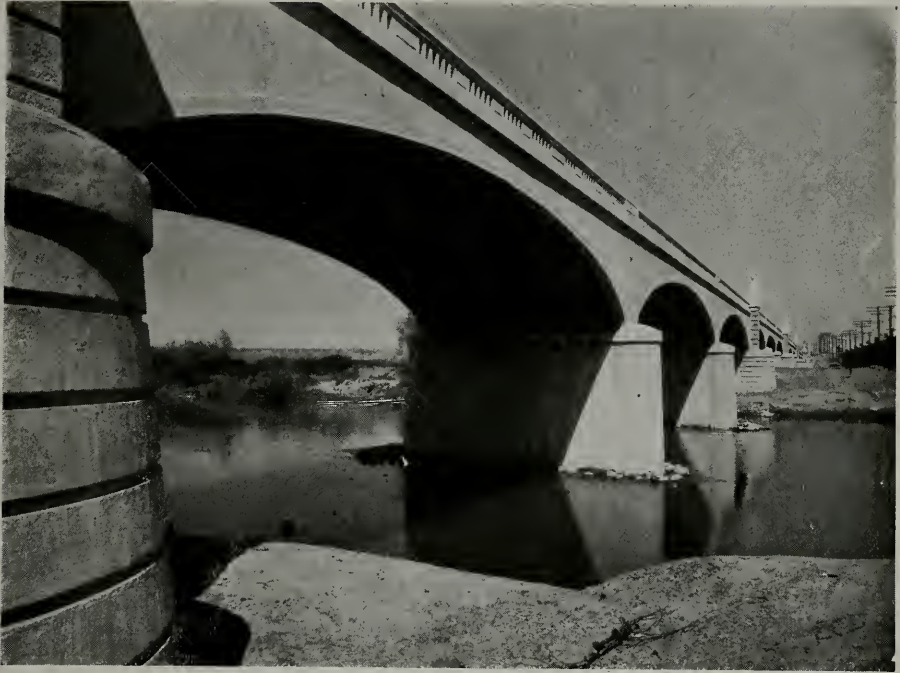
MODESTO BRIDGE, SHOWING RIVER SPANS (Not arches, but cantilevers)
