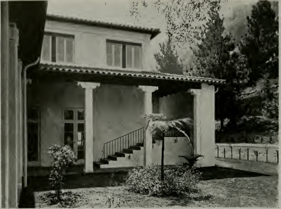
MAIN STAIRWAY TO SECOND STORY, RESIDENCE OF MAJOR J. H. H. PESHINE, SANTA BARBARA Myron Hunt, Architect
