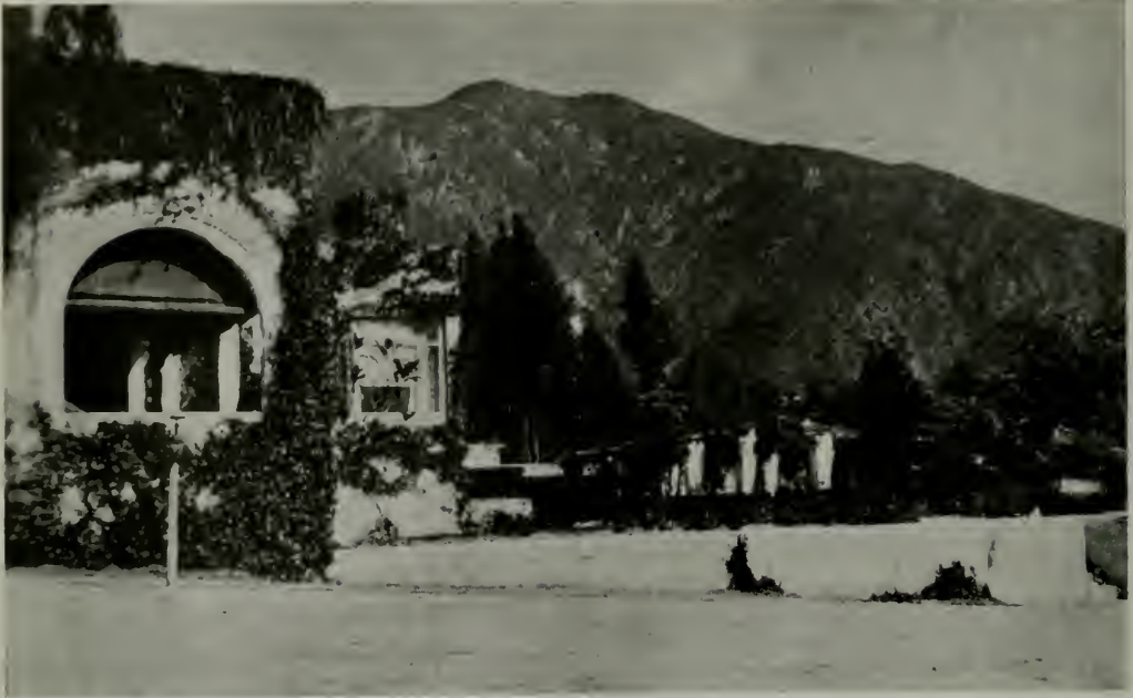
GARDEN APARTMENTS, SIERRA MADRE Irving J. Gill, Architect
