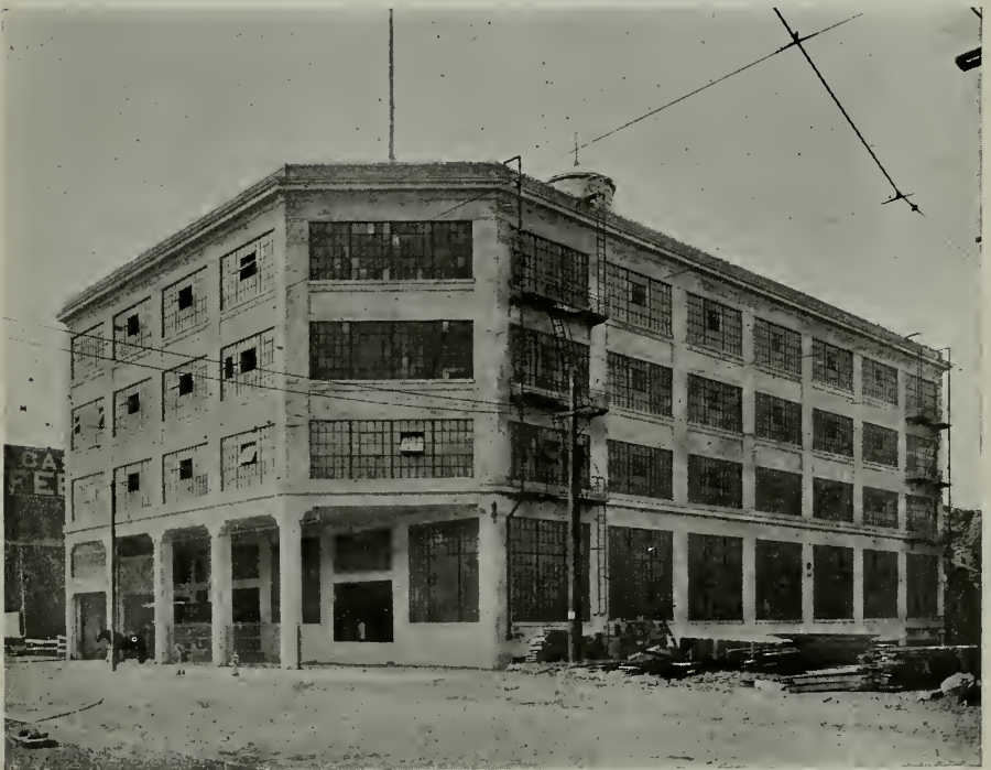
BUILDING FOR PACIFIC COAST ENVELOPE COMPANY, SAN FRANCISCO W. H. Crim, Jr., Architect
