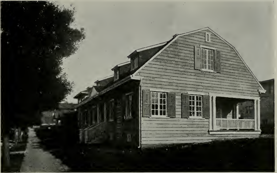
RESIDENCE OF MR. J. BAUME, BERKELEY James W. Plachek, Architect
