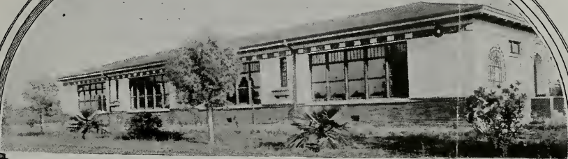
Jackson School, Fresno, California—Ernest J. Kump, Architect JOHNS-MANVILLE STUCCO USED
