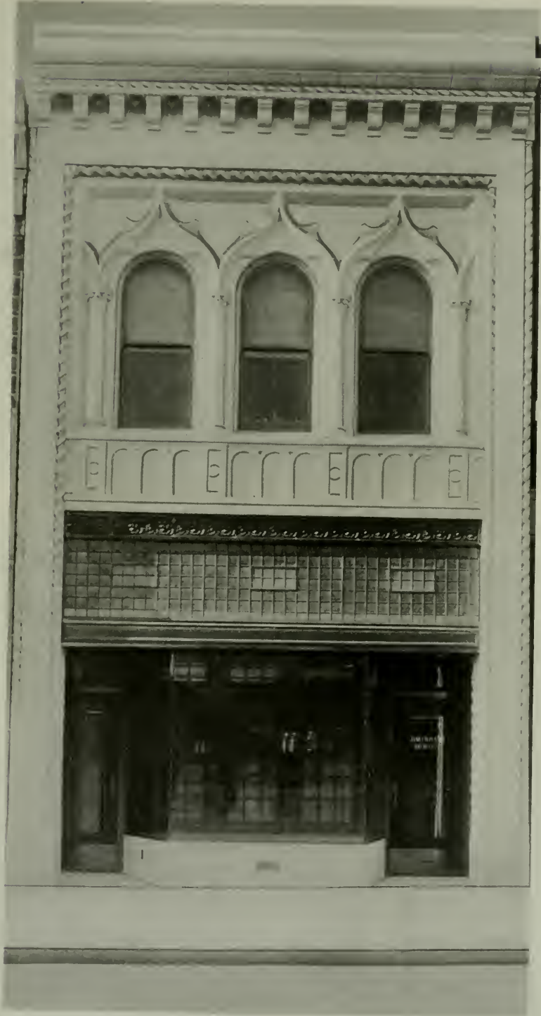
BUILDING FOR FORMER MAYOR W. H. HEYWOOD, BERKELEY JAMES W. PLACHEK, ARCHITECT
