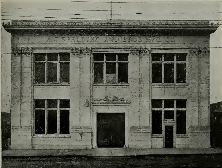
BUILDING FOR A. G. SPAULDING BROS. CO., SAN FRANCISCO W. H. Crim, Jr., Architect
