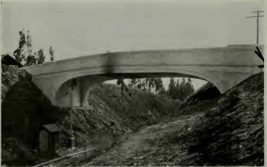
CANTCRETE BRIDGE, PEYTON, CALIFORNIA
