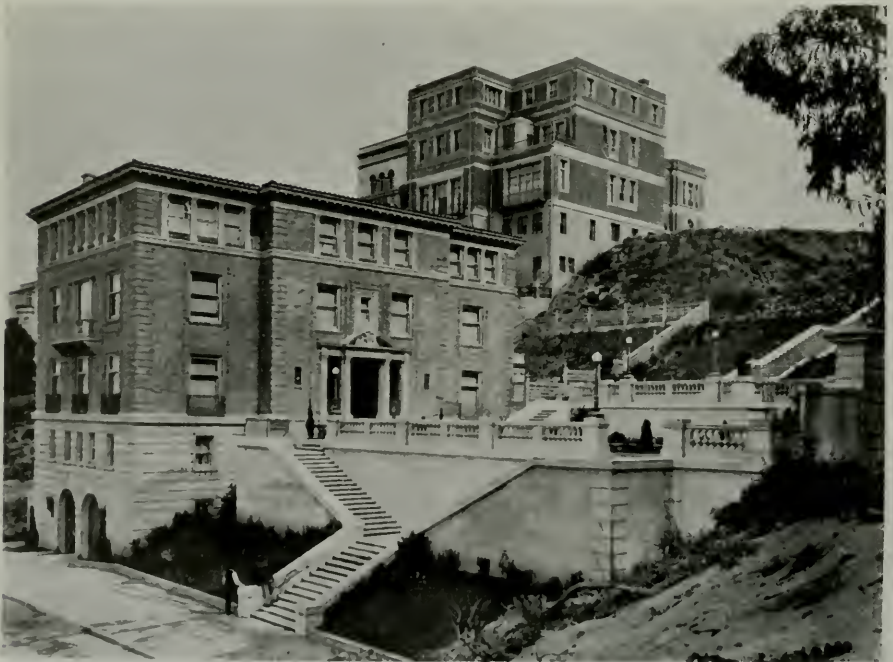
RESIDENCE OF MR. JOSEPH J. TYNAN, SAN FRANCISCO Louis M. Upton, Architect
