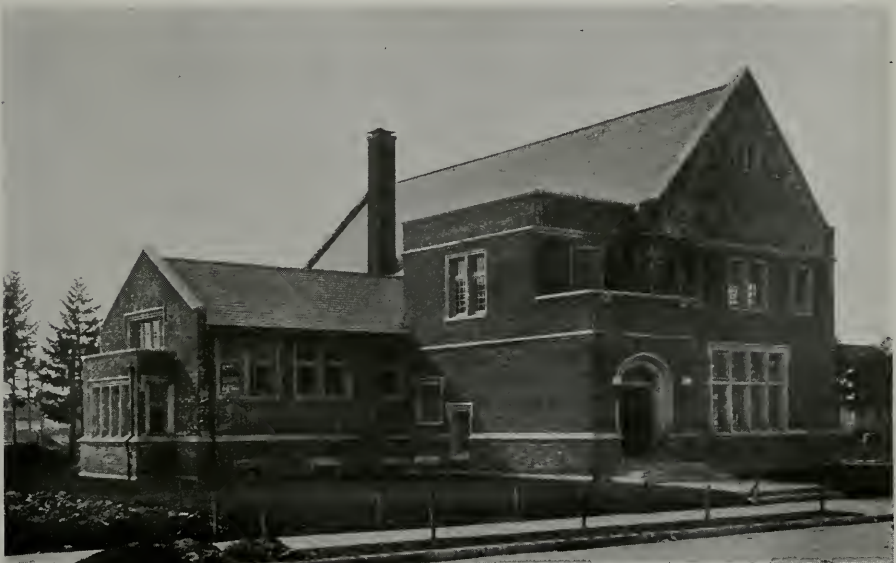
NORTH BRANCH LIBRARY
