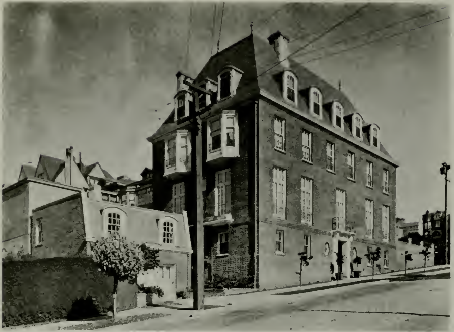
RESIDENCE OF MR. FRANK KING, SAN FRANCISCO Bakewell & Brown, Architects
