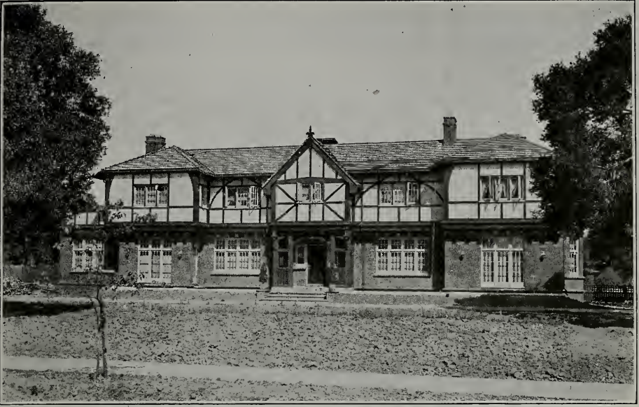
RESIDENCE OF MR. W. E. PALMER, PALO ALTO, CALIFORNIA CHARLES E. HODGES, Architect
