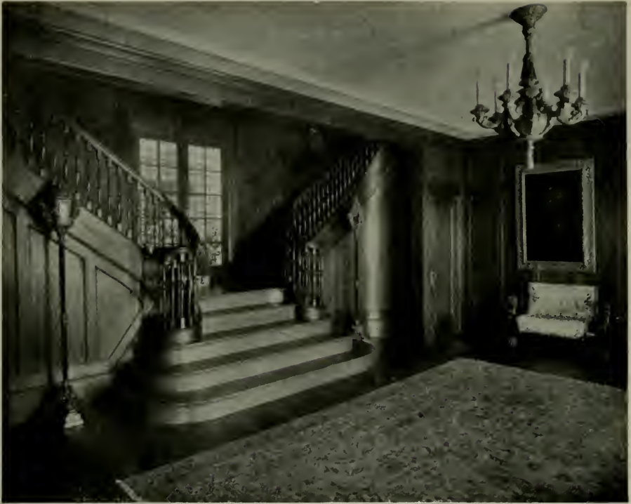
STAIRCASE, RESIDENCE OF MR. HARRY R. WILLIAR, SAN FRANCISCO W. H. Crim, Jr., Architect
