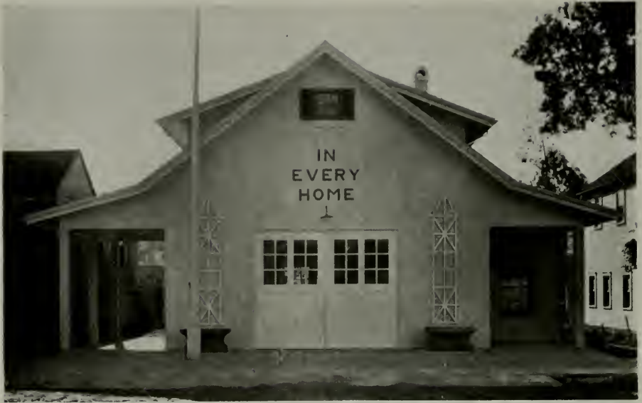
FIRE HOUSE FOR SPERRY FLOUR COMPANY, STOCKTON Joseph Losekann, Architect.
