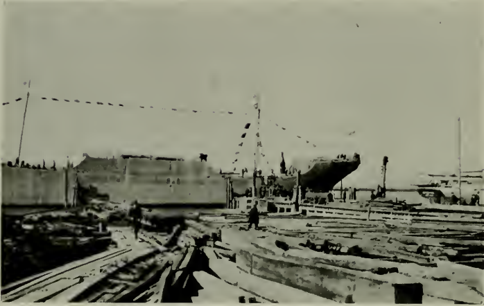
FIG. 3—Atlantis tied up to pier after launching.
