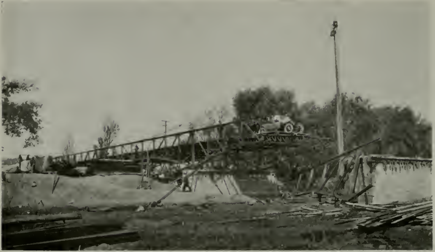
BRIDGE OVER PAJARO RIVER, SHOWING CANTILEVERS BEFORE ENCASEMENT WITH CONCRETE.
