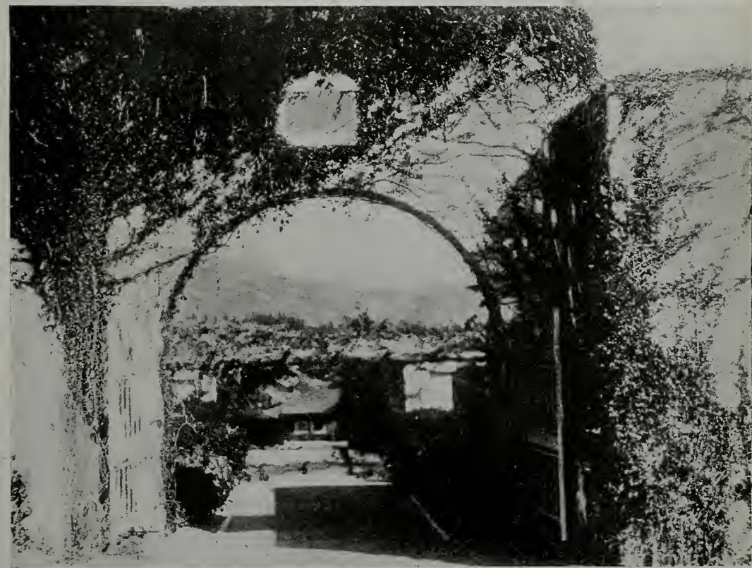
GARDEN APARTMENTS, SIERRA MADRE IRVING J. GILL, ARCHITECT
