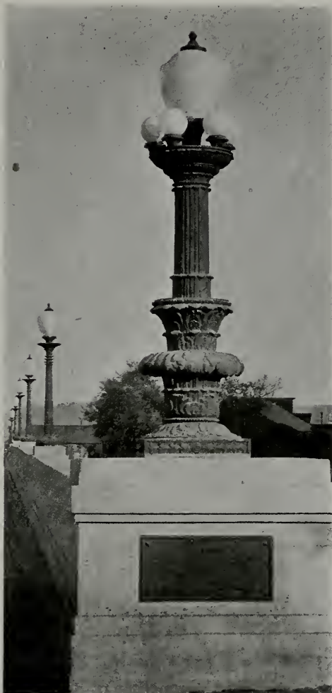
ELECTROLIER, WATSONVILLE BRIDGE
