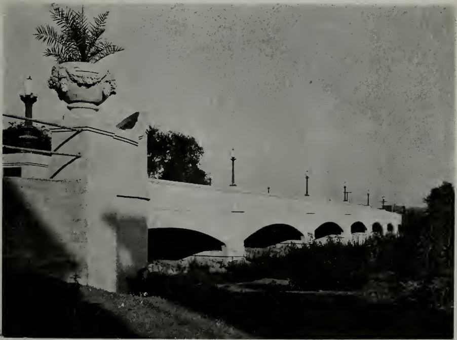
WATSONVILLE BRIDGE, OVER PAJARO RIVER, WATSONVILLE, CAL. Leonard & Day, Consulting Engineers
