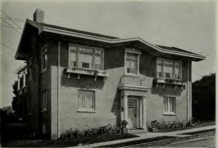
RESIDENCE OF MR. LESLIE D. ROBINSON, BERKELEY James W. Plachek, Architect
