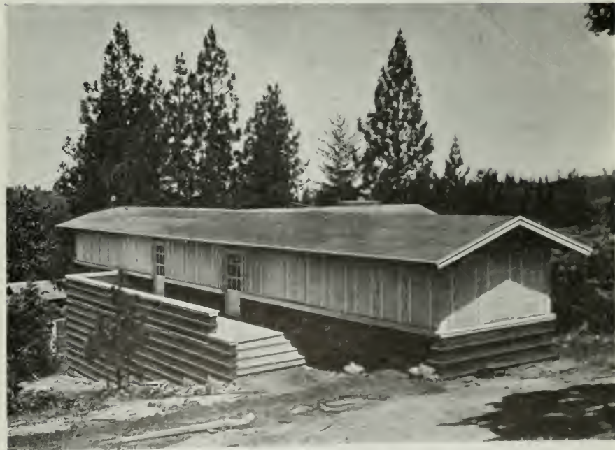
Typical Sleeping Porch Ward WEIMAR JOINT SANATORIUM, WEIMAR PLACER COUNTY R. A. Herald, Architect
