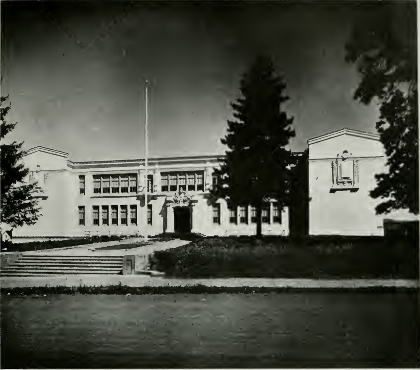
Healdsburg School, Wm. H. Weeks, Architect Robert Dalziel, Jr., Plumbing Contractor
