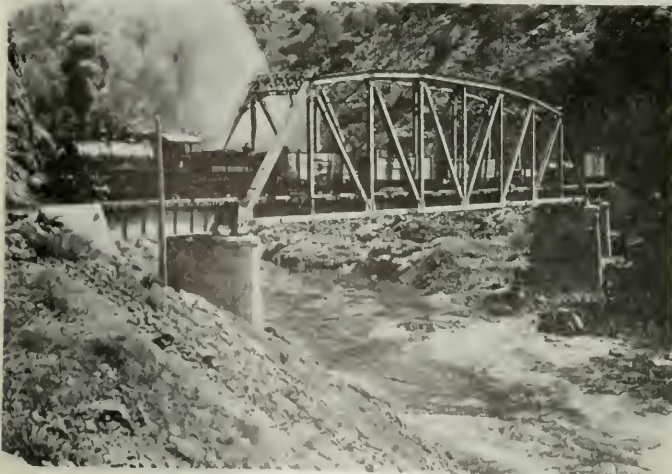
HETCH HETCHY RAILROAD OVER TUOLUMNE BRIDGE.
