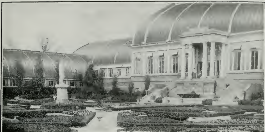
PALM HOUSE, MISSOURI BOTANICAL GARDENS, ST. LOUIS, MO. Designed by Pierson U-Bar Co., erected by Hitchings & Co., Elizabeth, N. J.
