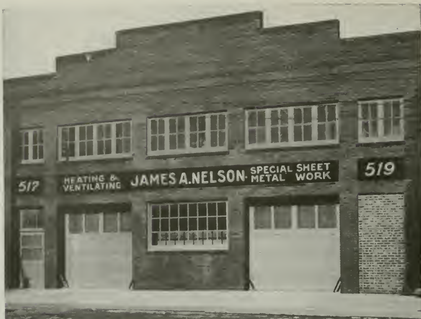
NEW FACTORY AND SHEET METAL SHOPS OF JAMES A. NELSON, SAN FRANCISCO
