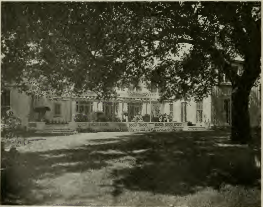
HOUSE OF MR. CHAS. R. McCORMICK, ATHERTON, CALIFORNIA Lewis P. Hobart, Architect
