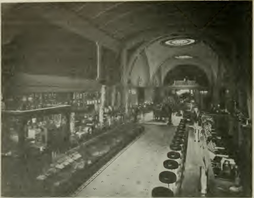
INTERIOR, HUNNECUTT STORE, SAN FRANCISCO Alfred Kuhn, Architect
