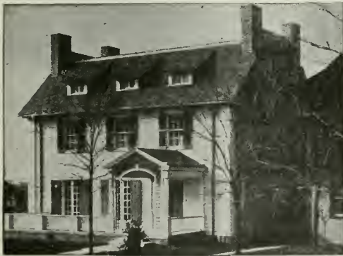
Walls finished with Cabot's Old Virginia White Roof finished with No. 36 Dark Gray Creosote Stain Walter Boschen, Architect, St. Joseph, Mo.
