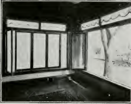
Sash open inside. Screens or storm windows applied outside. Windows easily cleaned.
