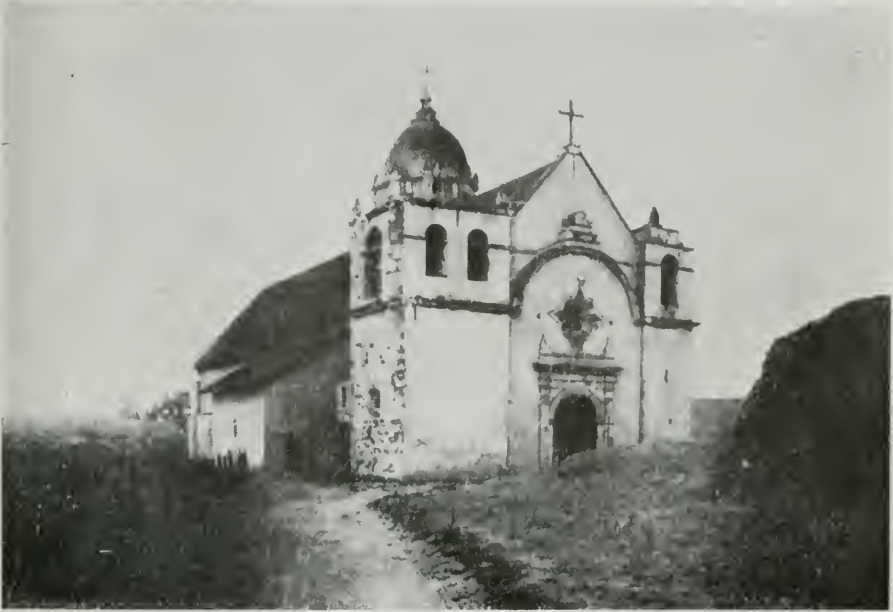
SAN CARLOS MISSION, CARMEL—PRESENT CONDITION
