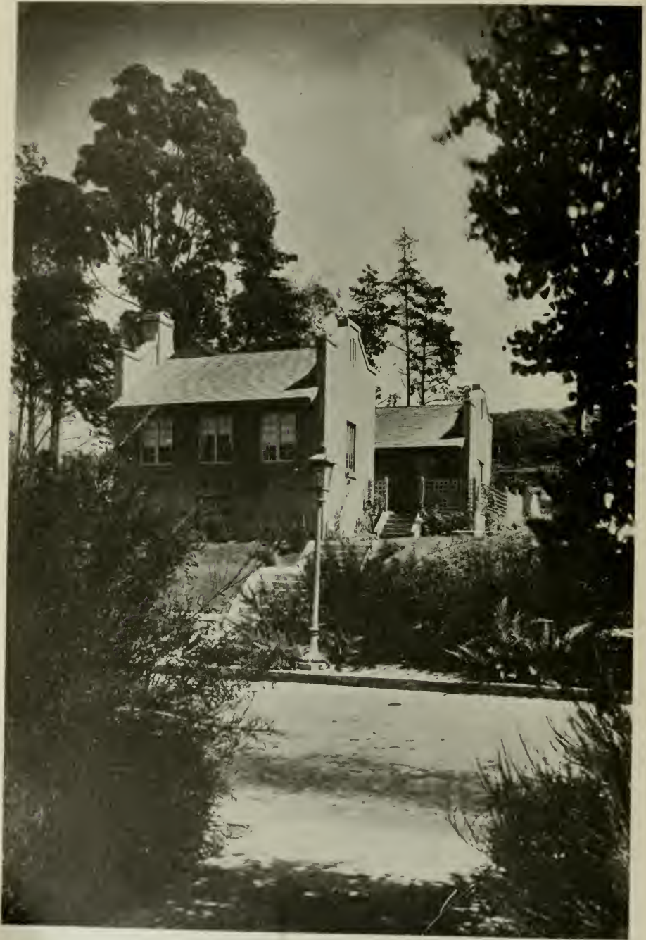
HOUSE OF MR. HENRY N. CLIFT, ST. FRANCIS WOOD, SAN FRANCISCO HEIMAN & SCHWARTZ, ARCHITECTS
