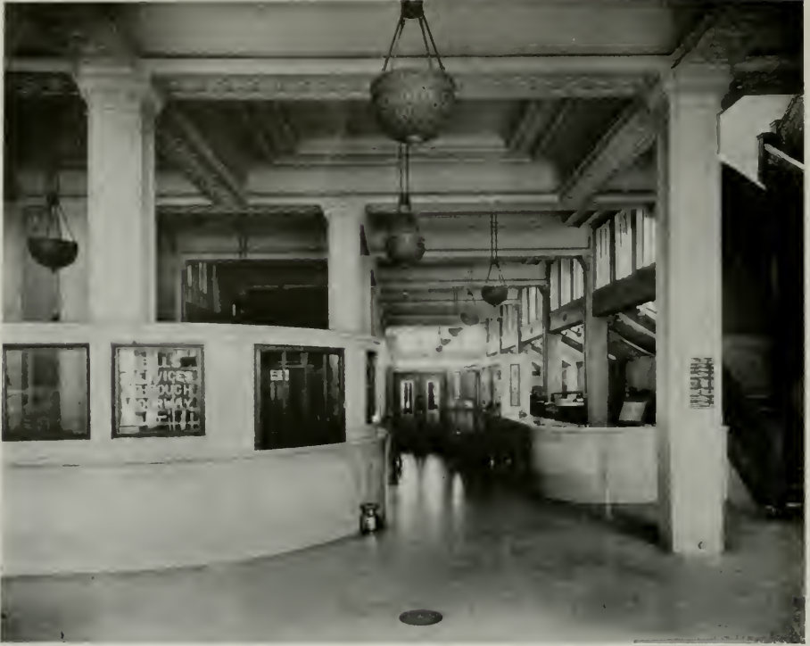
MAIN FLOOR, PACIFIC GAS AND ELECTRIC CO. ANNEX, SAN FRANCISCO Edgar A. Mathews, Architect
