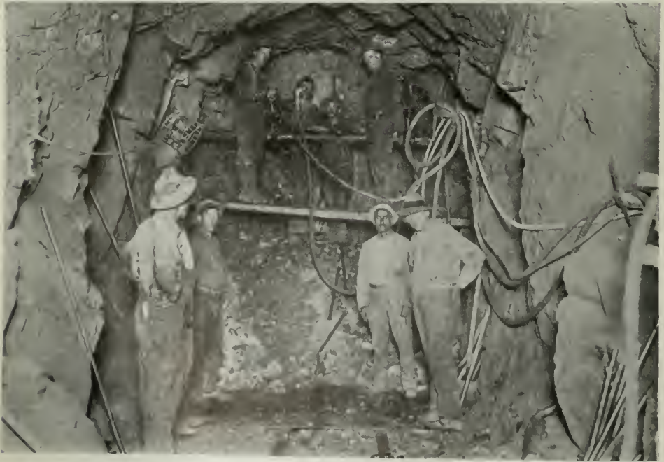
FACE OF PRIEST TUNNEL, HETCH HETCHY WATER SUPPLY PROJECT
