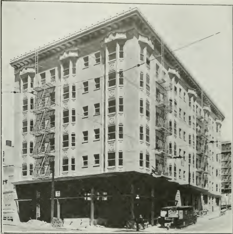
APARTMENT HOUSE, TAYLOR AND GEARY STREETS, SAN FRANCISCO FOR I. ROSENBERG - JOSEPH CAHEN, ARCHITECT
