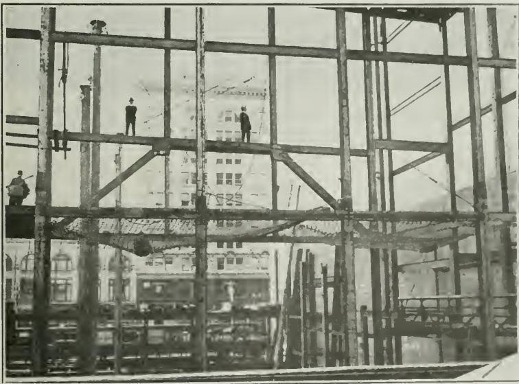
SAFETY NETS TO CATCH FALLING WORKMEN
