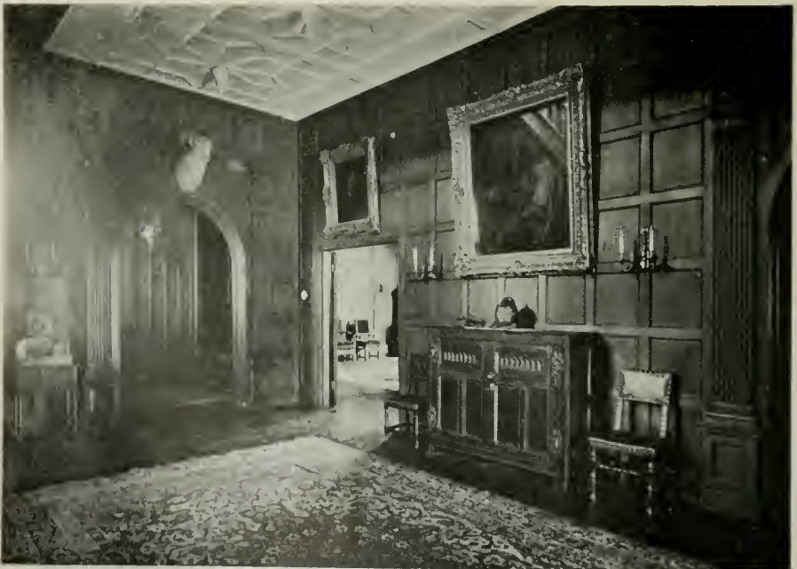
MAIN STAIR HALL, MORGAN HOUSE
