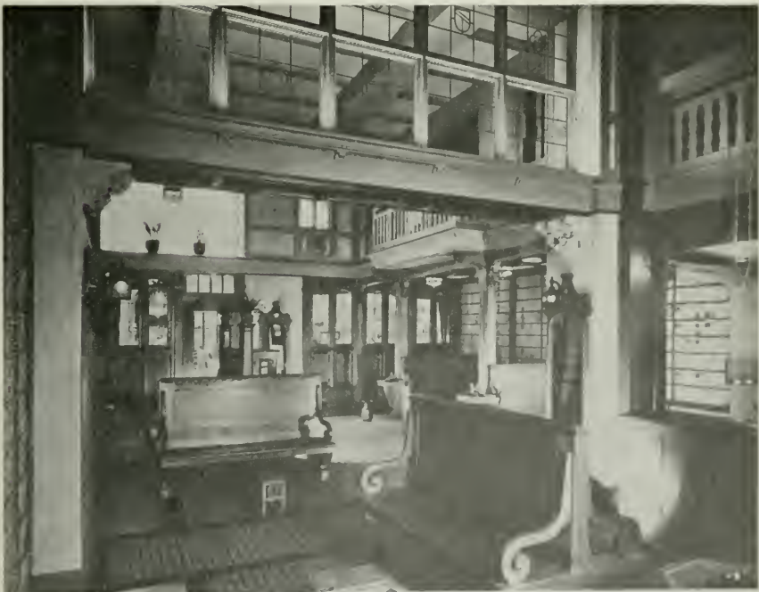
GENERAL VIEW, WERNER SHOE STORE Alfred Kuhn, Architect
