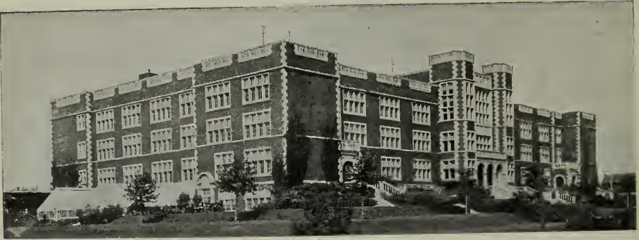
CENTRAL HIGH SCHOOL, MINNEAPOLIS, MINN.
