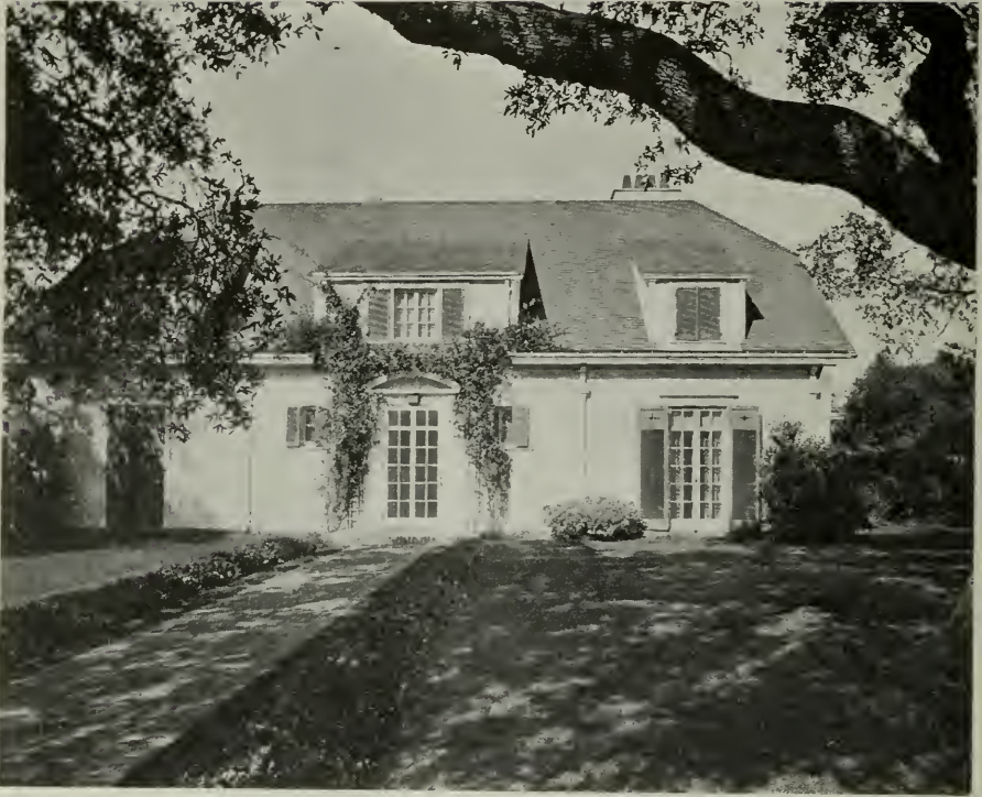
RESIDENCE OF MRS. MARY KEELEY 908 OAK GROVE AVENUE, PASADENA ROBERT D. FARQUHAR, ARCHITECT
