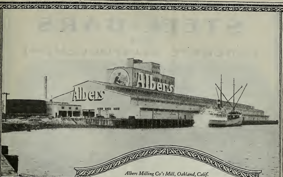
Albers Milling Co's Mill, Oakland, Calif. Covered with a PABCO 10 Year Roof.
