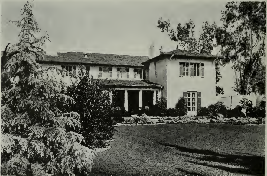
LOOKING TOWARD THE HOUSE, FULLER GARDEN, PASADENA Paul G. Thiene, Landscape Architect
