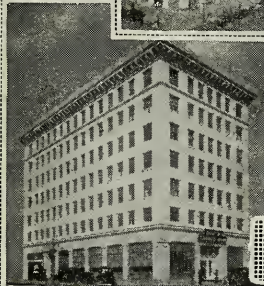
CITIZENS SAVINGS BLDG. PASADENA, CAL.
