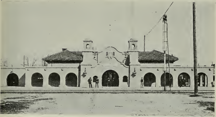
PASSENGER STATION, MODESTO, CALIFORNIA Engineering Department, Southern Pacific Company, Architects
