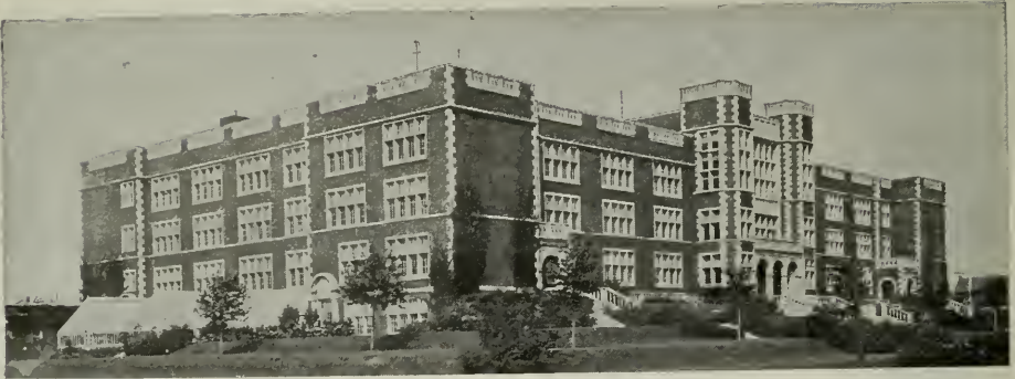
CENTRAL HIGH SCHOOL, MINNEAPOLIS, MINN.
