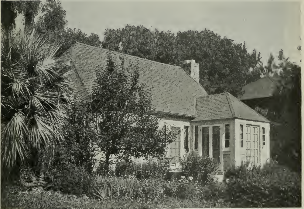
SIDE VIEW, LYON RESIDENCE, HOLLYWOOD Pierpont and Walter S. Davis, H. F. Withey, Architects
