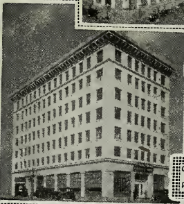
CITIZENS SAVINGS BLDG. PASADENA, CAL.
