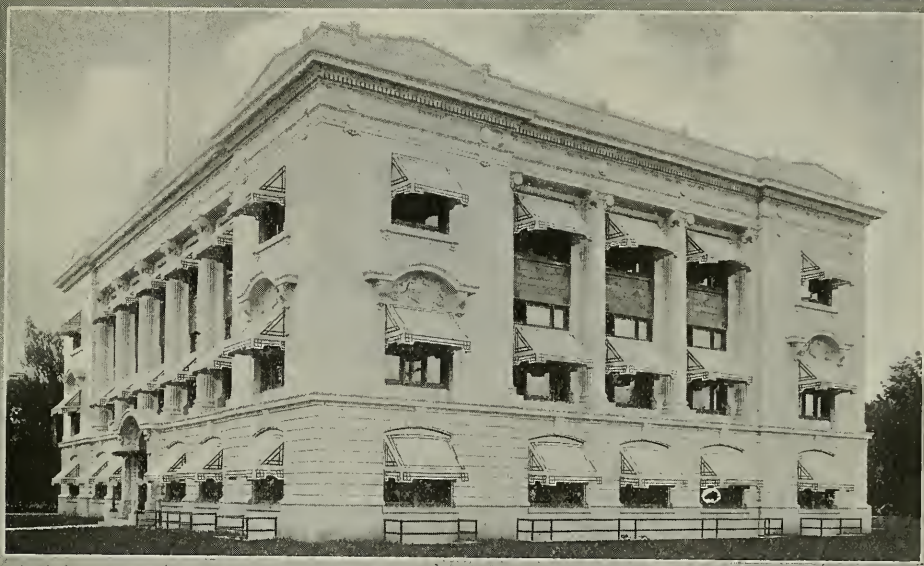
State Supreme Court and Library Building, Salem, Oregon Architect W. C. Knighton, formerly State Architect, Portland, Oregon
