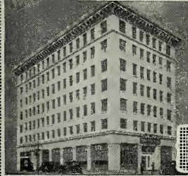
CITIZENS SAVINGS BLDG. PASADENA, CAL.
