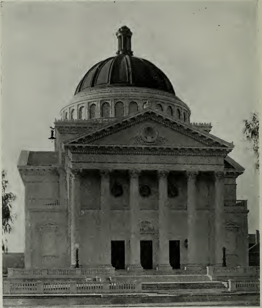
SECOND CHURCH OF CHRIST SCIENTIST, WEST ADAMS ST. A. F. ROSENHEIM, ARCHITECT
