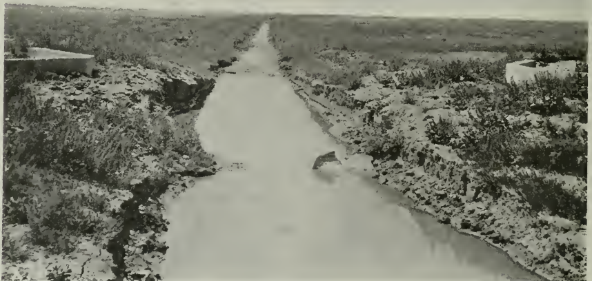
2. Location of corrugated siphon carrying drainage water under irrigation canal. No trouble from expansion and contraction although firmly anchored at both ends.
