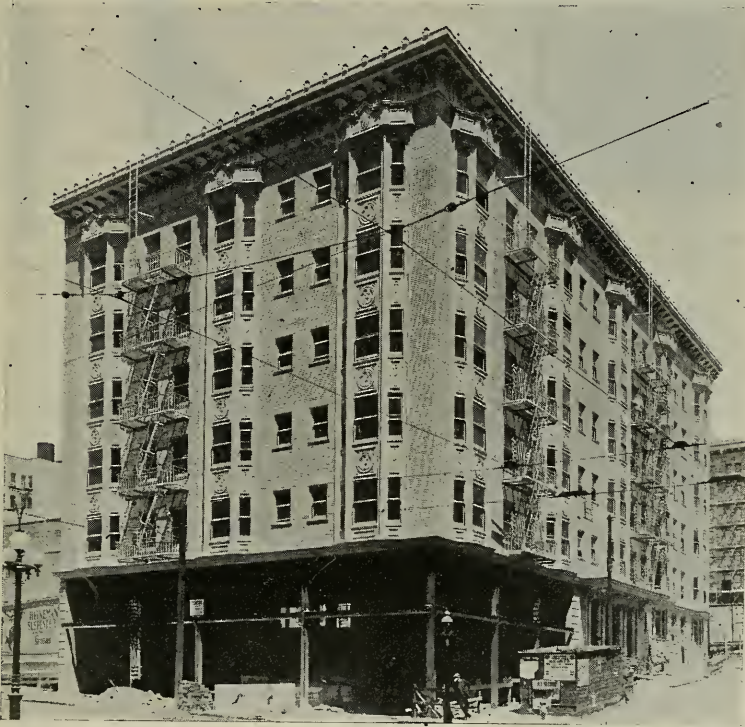
Apartment House, Taylor and Geary Streets, San Francisco, for Mr. I. Rosenberg. Mr. JOSEPH CAHEN, Architect.
