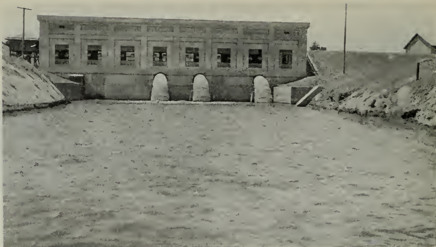
IRRIGATION PUMP HOUSE AT THE NORTHWEST CORNER OF DISTRICT NO. 1500
