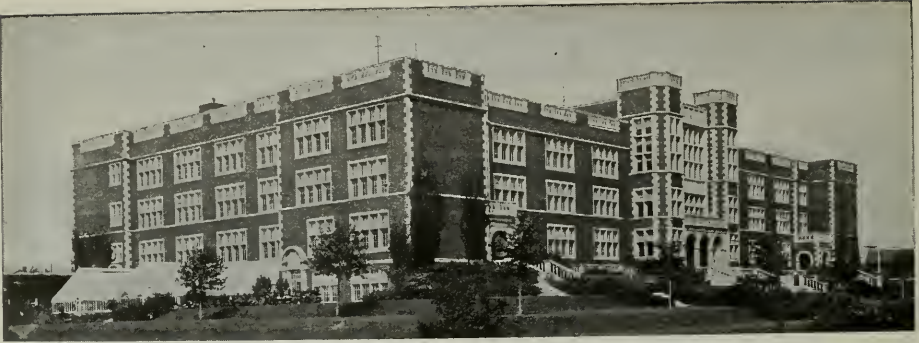
CENTRAL HIGH SCHOOL, MINNEAPOLIS, MINN.
