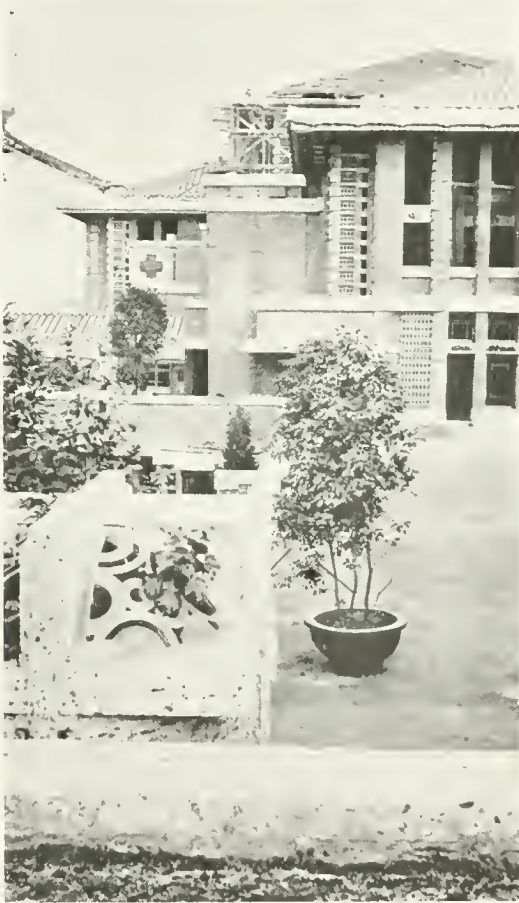
On the roof of the center unit, viewing the rear superstructure, containing the banquet hall and the theater
