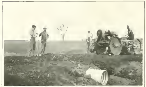
Installing Armeo Culverts Carmichael Colony Road Day
