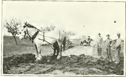
Making the Horses Dig the Trenches
