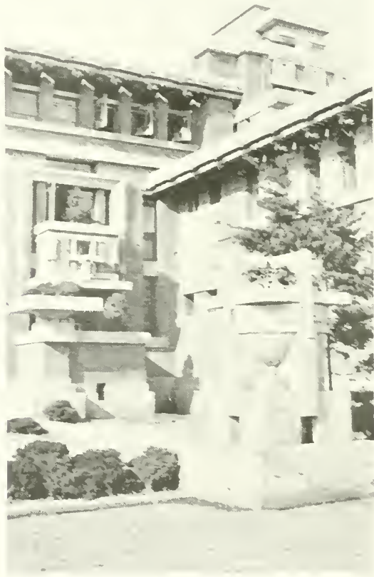
Perforated cornices, with applied copper ornament, overhang every facade. Groups of windows are almost absorbed with brick and stone
