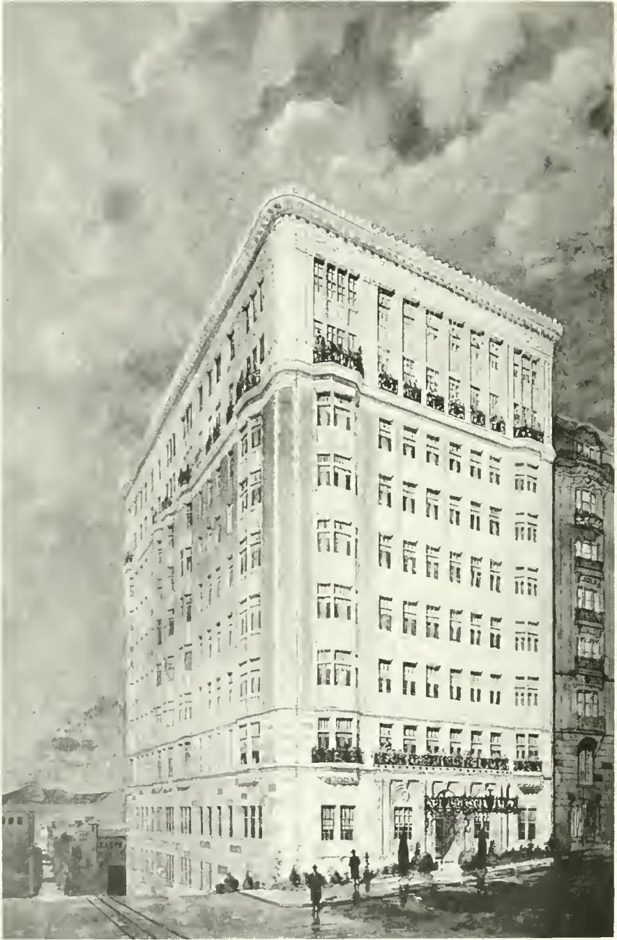
FRANCESCA APARTMENTS, SAN FRANCISCO KENNETH MAC DONALD ARCHITECT MAURICE C. COUCHOT ENGINEER
