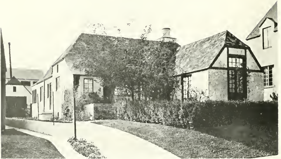
ESTATE OF MR. THOMAS D. NICKOLS, LOS ANGELES Pierpont and Walter S. Davis, Architects
