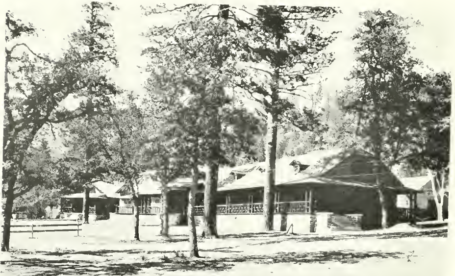
THE CLUB HOUSE, PIT RIVER No. 1 DEVELOPMENT
