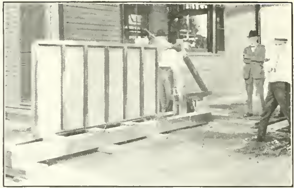
Test Conducted by Armour Institute, showing superiority of Metal Lath over other forms of construction.
