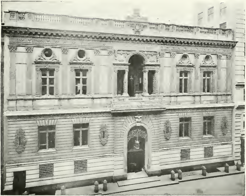
The Century Club, New York City, McKim, Mead & White, Architects. Terra Cotta used for wall finish of lower story above base and ornamental treatment up to and including parapet balustrade.
