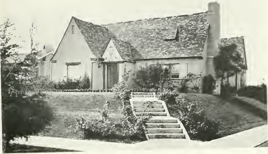
HOUSE FOR MR. MAX CROTINER, LOS ANGELES Pierpont and Walter S. Davis, Architects
