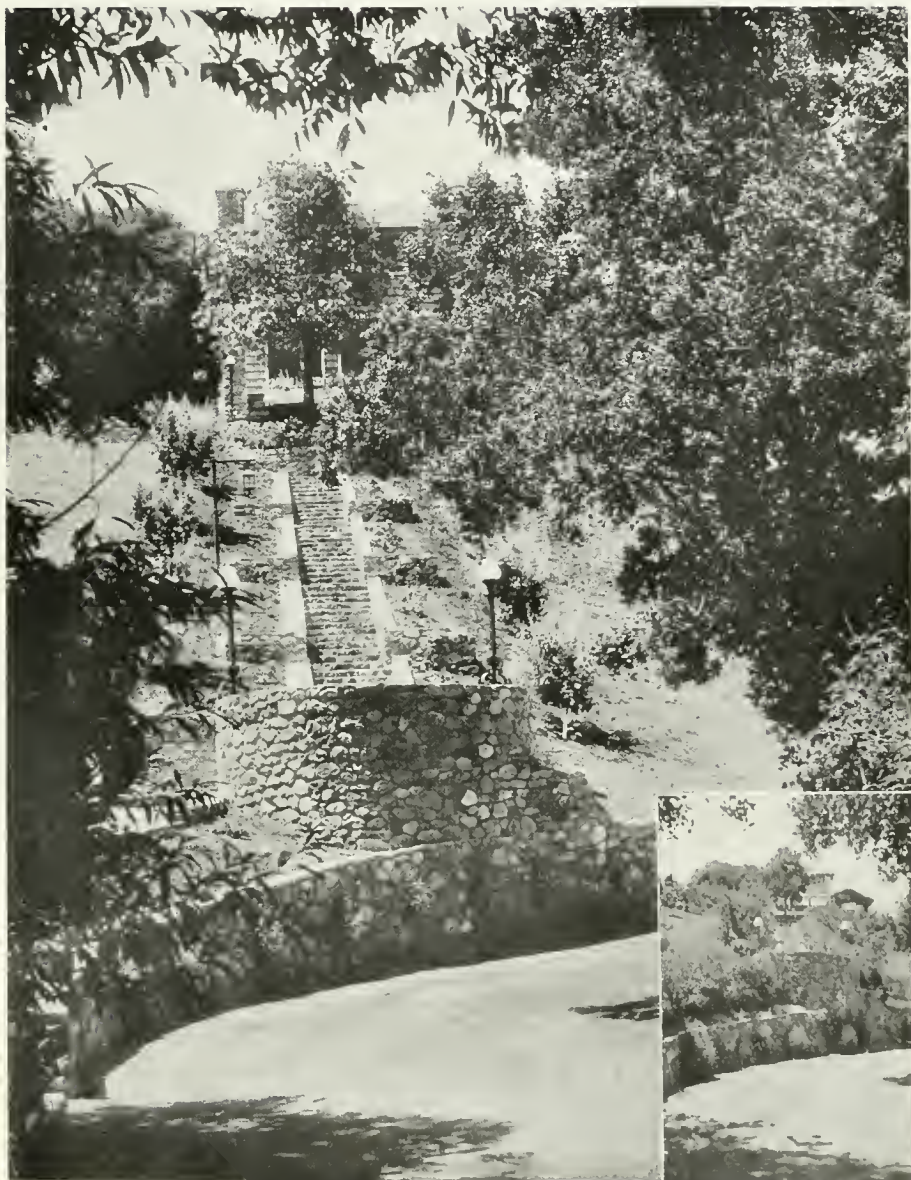
RUBBLE STONE STAIRWAY, LITTLE BROOK FARM, LOS GATOS EMERSON KNIGHT LANDSCAPE ARCHITECT AND ENGINEER
