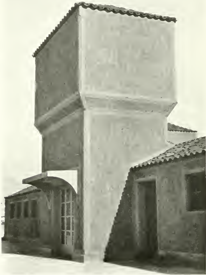
ELEVATOR HOUSE ON ROOF. BUILDING FOR THEO. H. DAVIES & CO. Louis Christian Mullgardt, Architect
