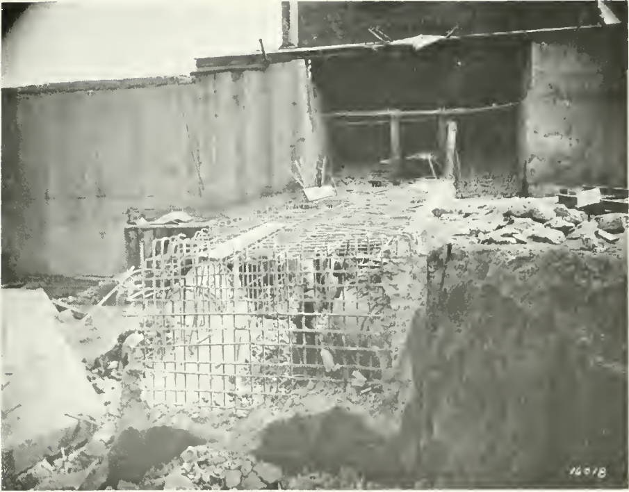
SECTION OF VENTURI VAULT BEING DEMOLISHED BY PAVING BREAKERS
