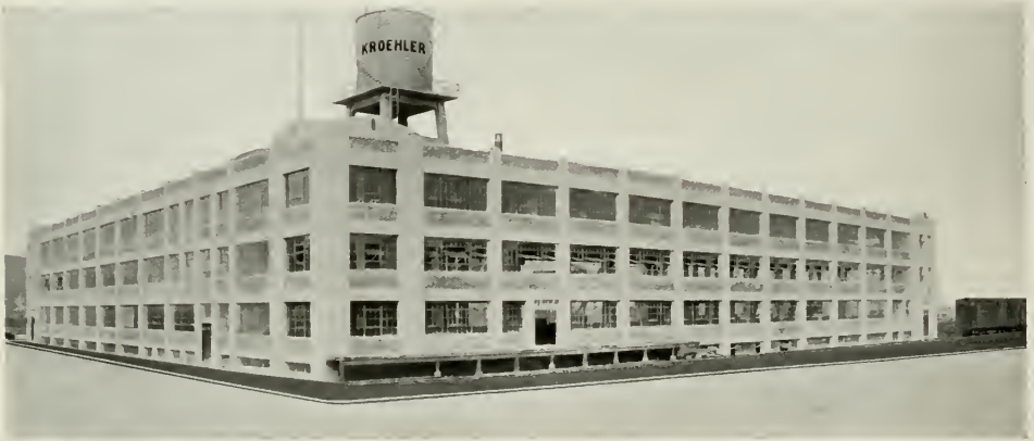
BUILDING FOR KROEHLER MANUFACTURING COMPANY, SAN FRANCISCO N. H. Nishkian, Engineer
