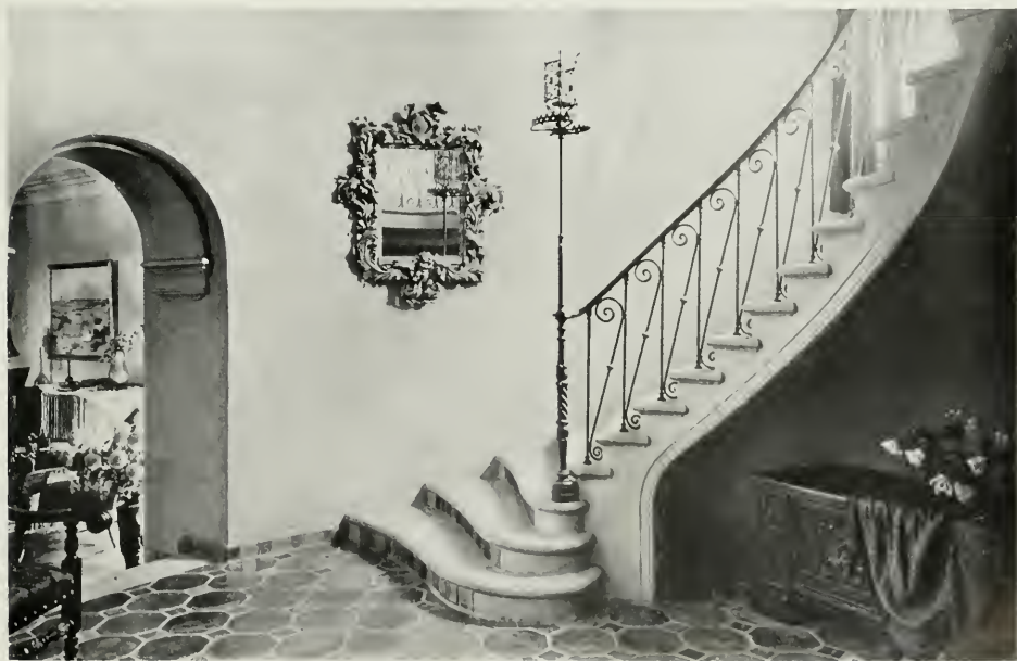
CONCRETE FLOOR, HOUSE OF FRED R. JOHNSON, BEVERLY HILLS.
