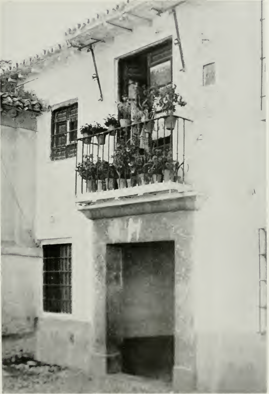
DELIGHTFUL TREATMENT OF AN ENTRANCE TO A HOUSE IN GRANADA
