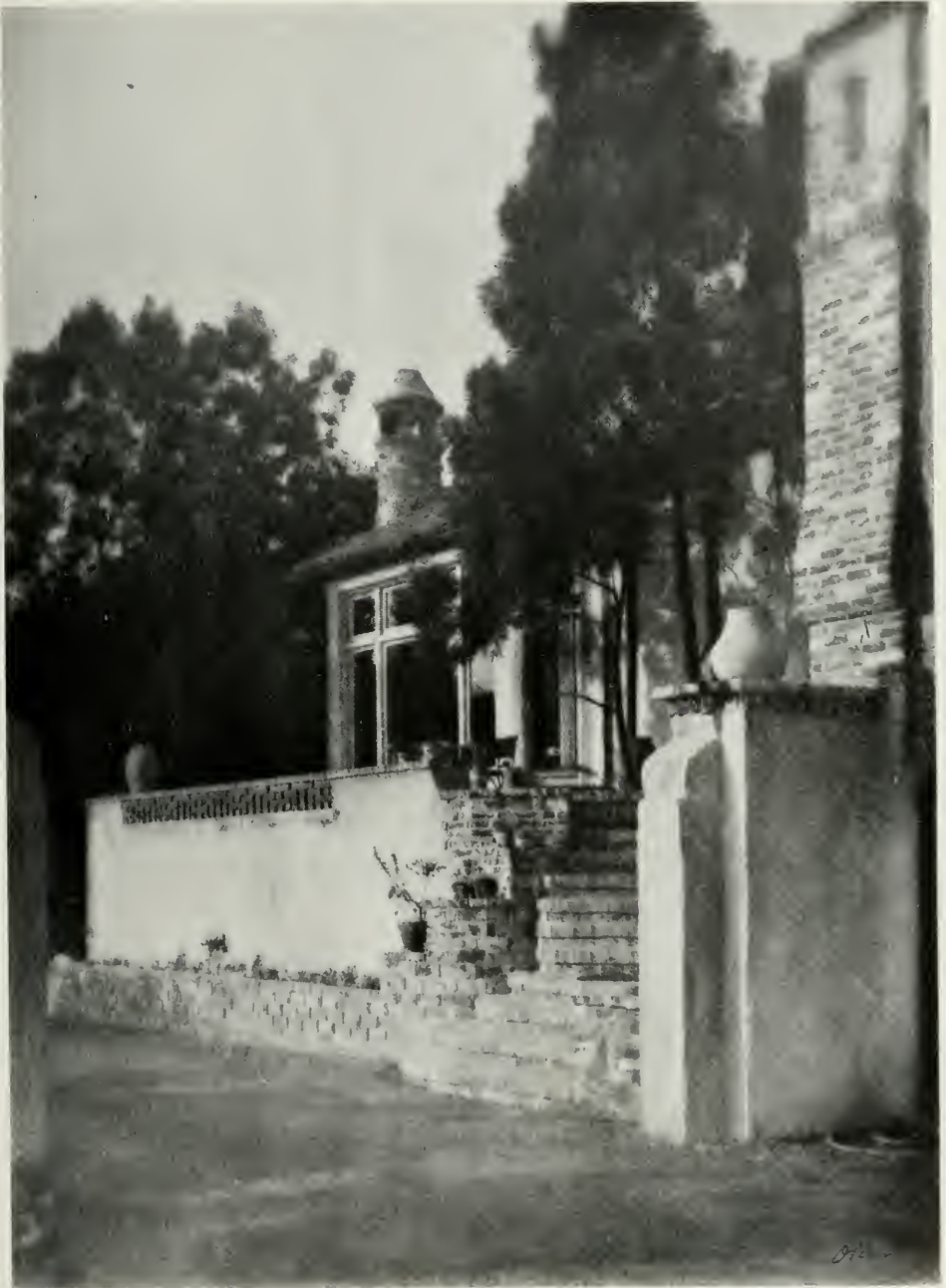
PORCH, HOUSE FOR DR. DEXTER RICHARDS, CLAREMONT, BERKELEY W. R. YELLAND, ARCHITECT
