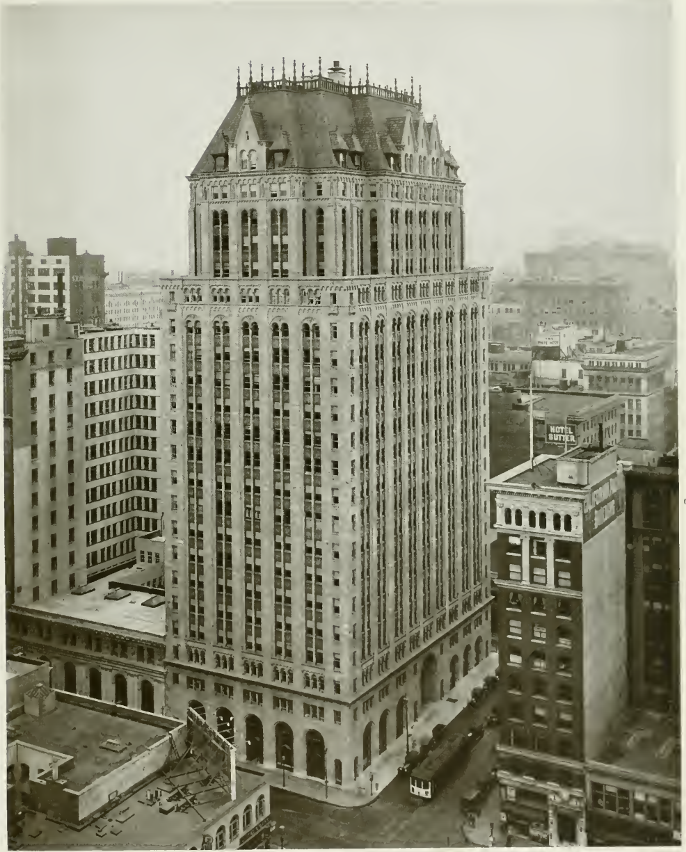
HUNTER-DULIN BUILDING, SAN FRANCISCO SCHULTZE AND WEAVER, ARCHITECTS
