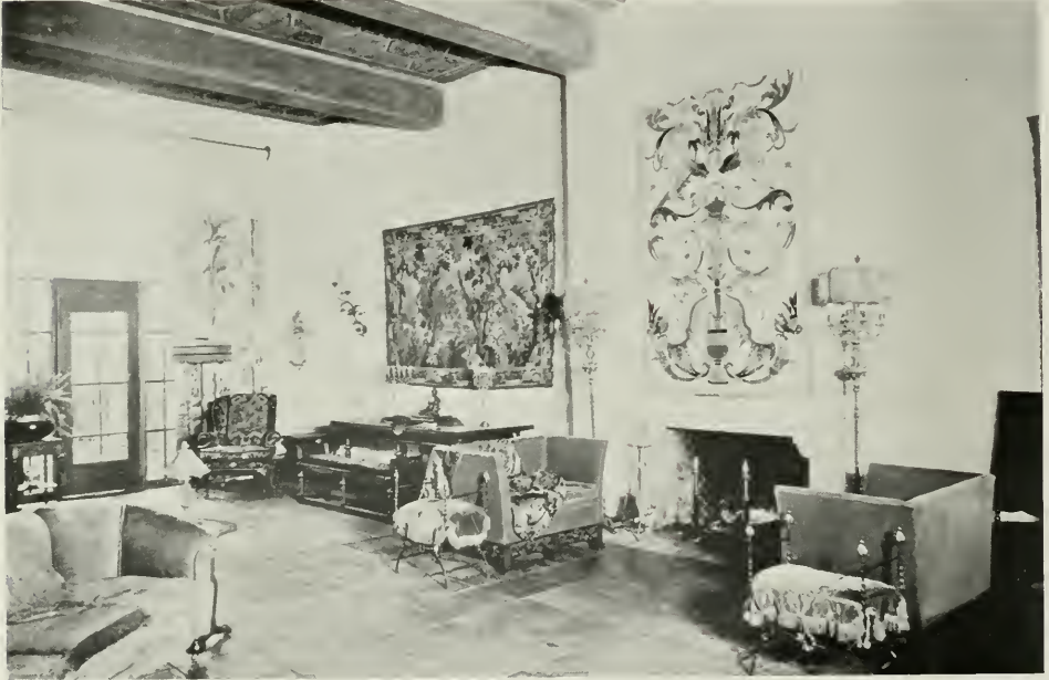
GATCH-HILL STUDIO, LOS ANGELES, CALIFORNIA (CONCRETE FLOOR)
