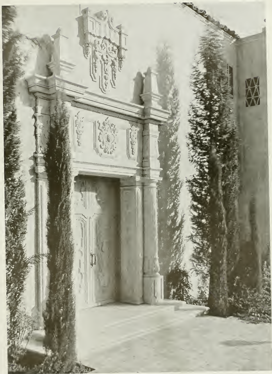
HOUSE FOR MR. AND MRS. W. H. PETERS, PASADENA, CALIFORNIA MARSTON, VAN PELT & MAYBURY, ARCHITECTS
