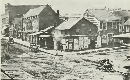
1861—SITE OF THE PRESENT RUSS BUILDING
