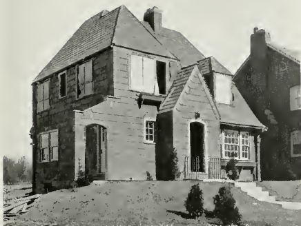
EXTERIOR OF FRAME DWELLING AFTER FIRE SWEEPS INTERIOR
