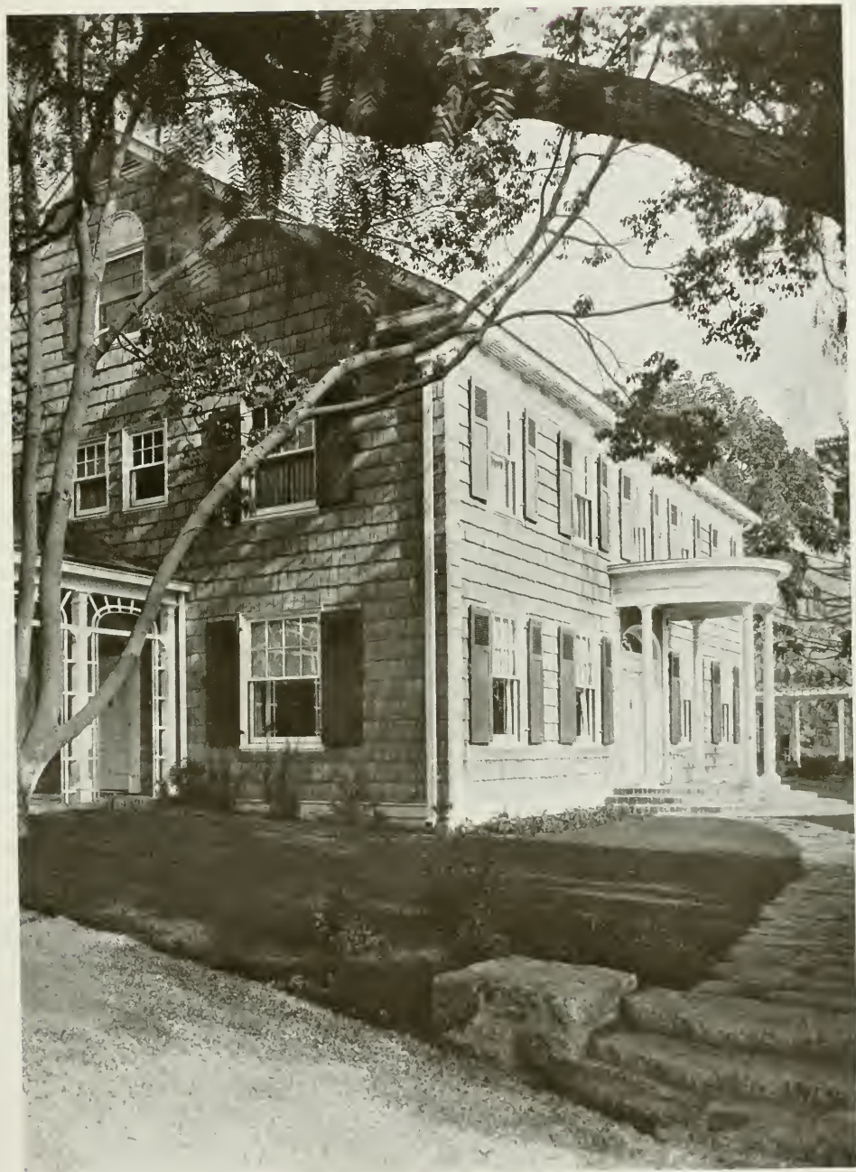
HOUSE FOR MR. GEORGE L. EASTMAN, HOLLYWOOD, CALIFORNIA WILLIAM LEE WOLLETT, ARCHITECT
