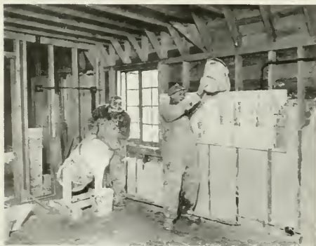
APPLYING CELLULAR GYPSUM TO SIDE WALLS OF FRAME DWELLING
