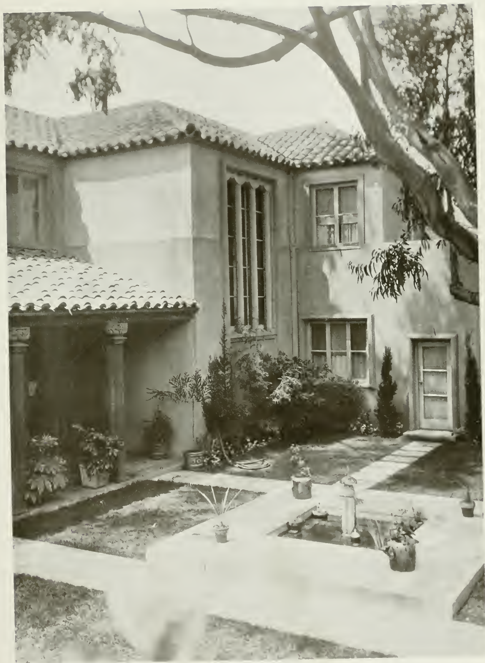
PATIO, HOUSE OF DR. HUBERT HEITMAN, CLAREMONT, BERKELEY W. H. RATCLIFF, JR., ARCHITECT
