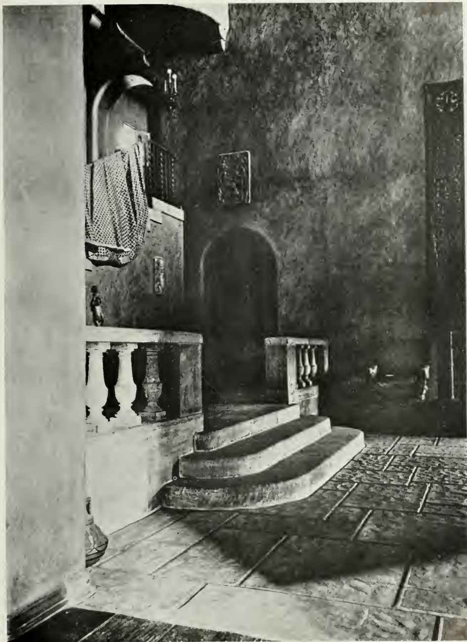
CONCRETE BALCONY AND FLOOR, HOUSE OF W. H. HANSON, FLINTRIDGE HARWOOD HEWITT, ARCHITECT
