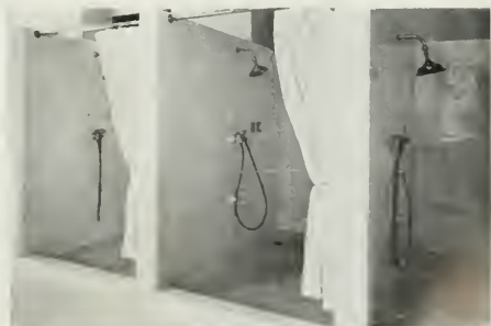
SHOWERS IN GYMNASIUM, RUSS BUILDING, SAN FRANCISCO
