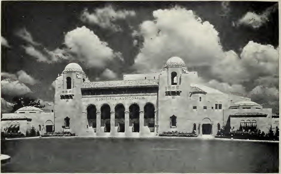
Municipal Auditorium, San Antonio, Texas. - Atlee B. and Robt. M. Ayers, Geo. Willis and organization, and Emmett T. Jackson, Architects
