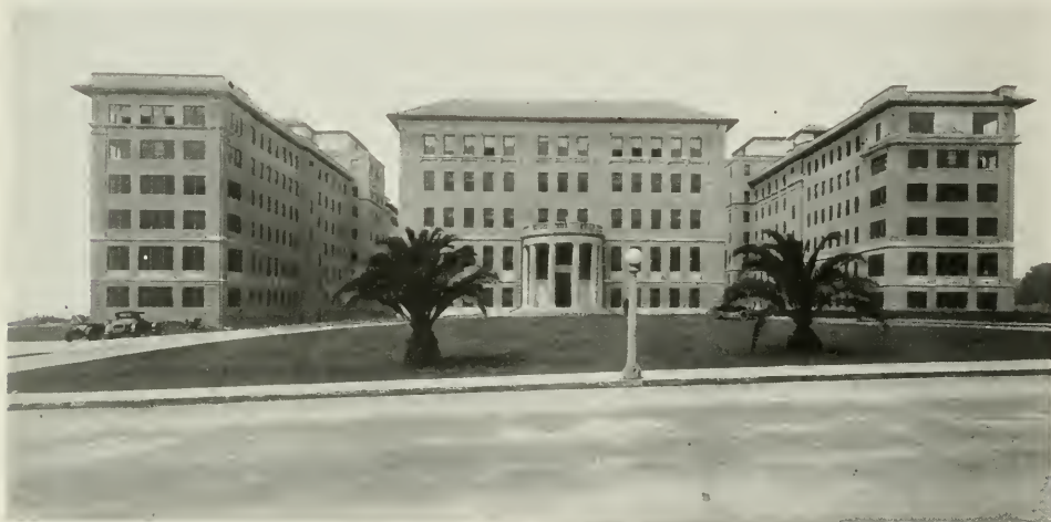
JAMES W. WADSWORTH HOSPITAL, SAWTELLE, CALIFORNIA
