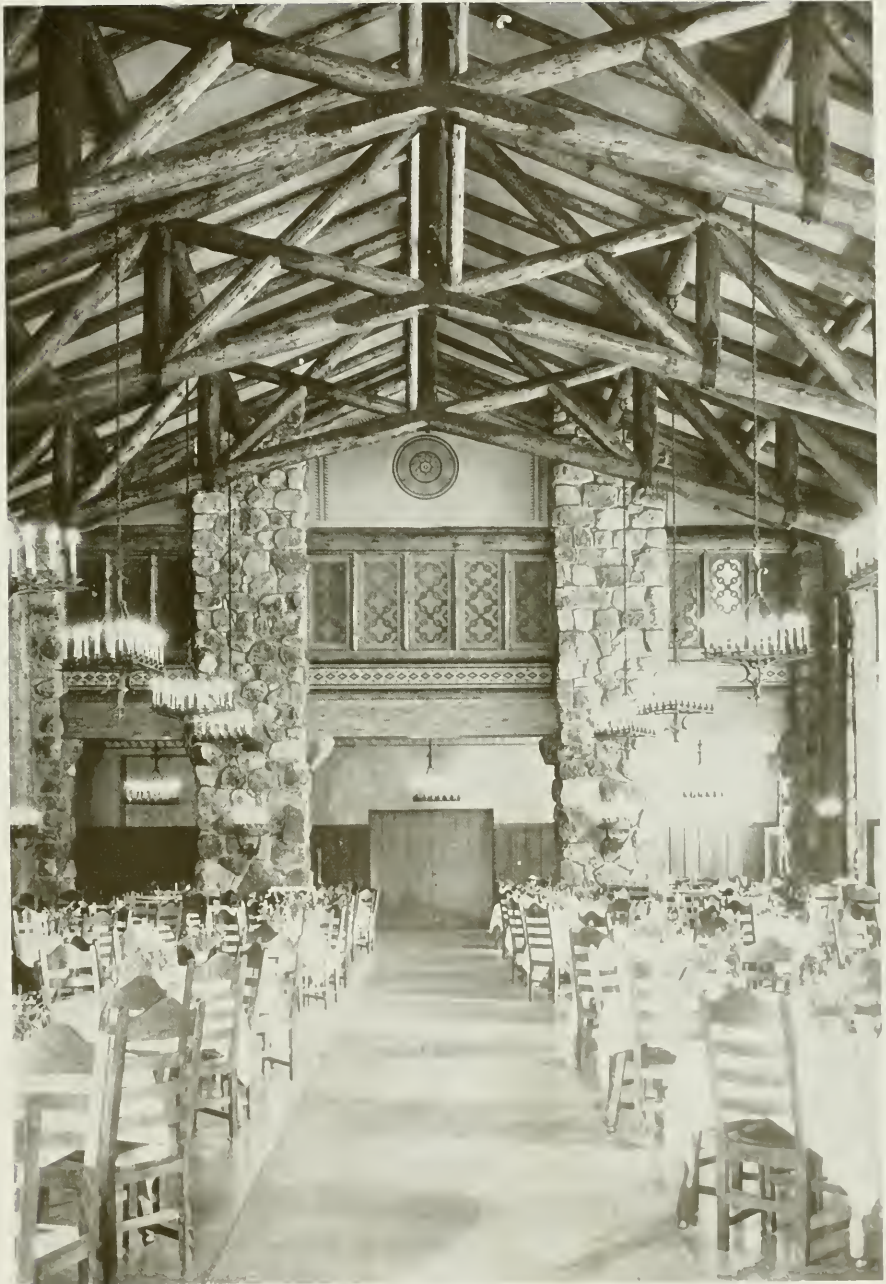
DINING ROOM, AHWAHNEE HOTEL, YOSEMITE VALLEY, CALIFORNIA GILBERT STANLEY UNDERWOOD, ARCHITECT
