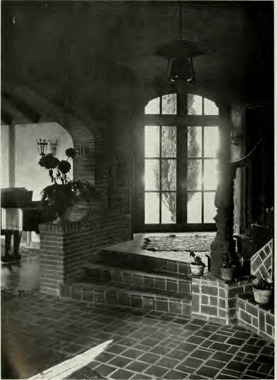
STAIR HALL, HOUSE FOR DR. DEXTER RICHARDS, CLAREMONT, BERKELEY W. R. YELLAND, ARCHITECT
