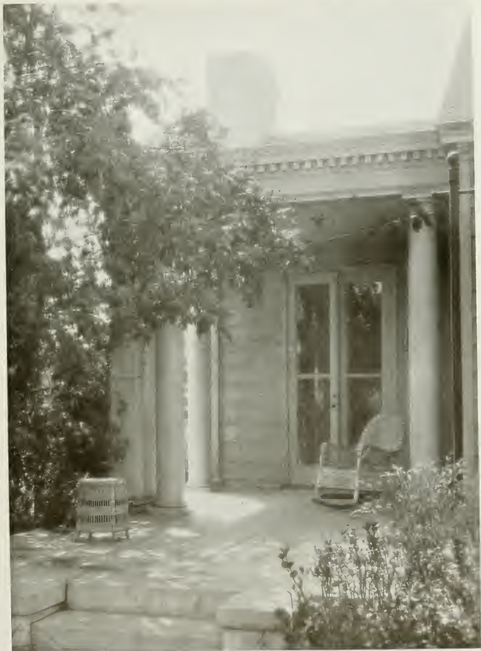
HOUSE FOR MR. W. S. WAITH, BEVERLY HILLS, CALIFORNIA MYRON HUNT AND H. C. CHAMBERS, ARCHITECTS
