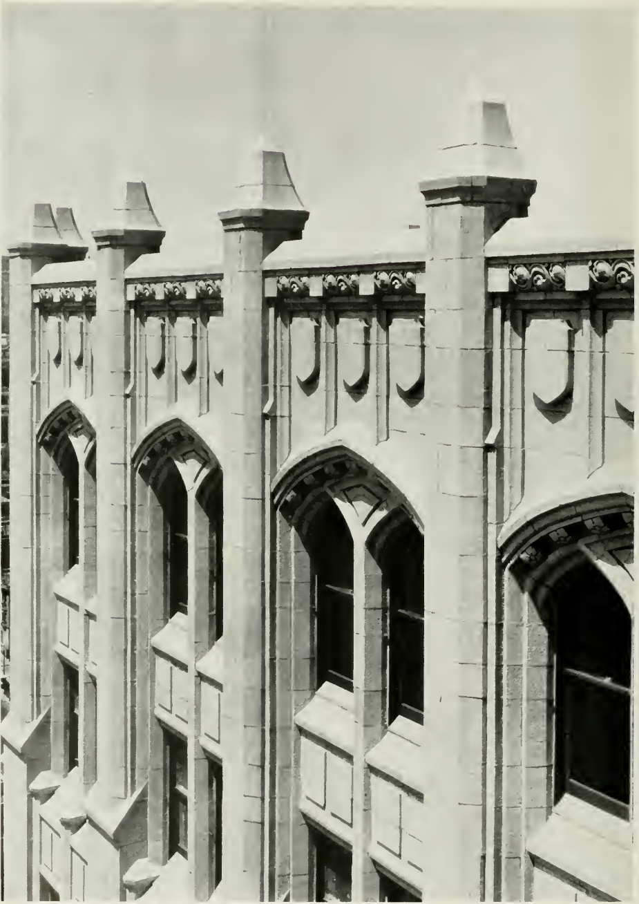
DETAIL OF UPPER STORIES, RUSS BUILDING, SAN FRANCISCO
