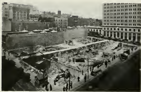
CLEARING THE SITE FOR THE NEW RUSS BUILDING. JULY, 1926
