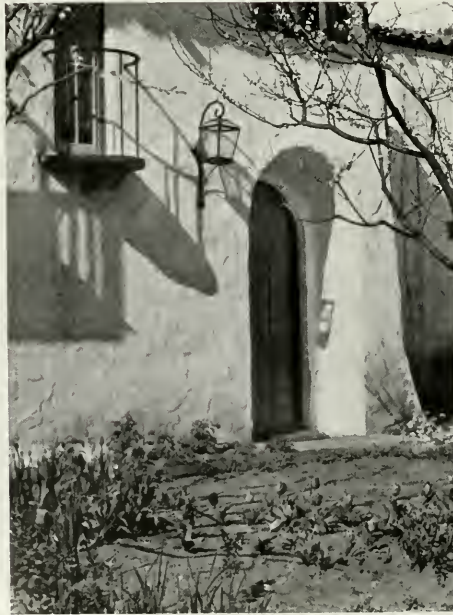
HOUSE OF MR. H. F. SWIFT, BERKELEY, CALIFORNIA Roland I. Stringham, Architect
