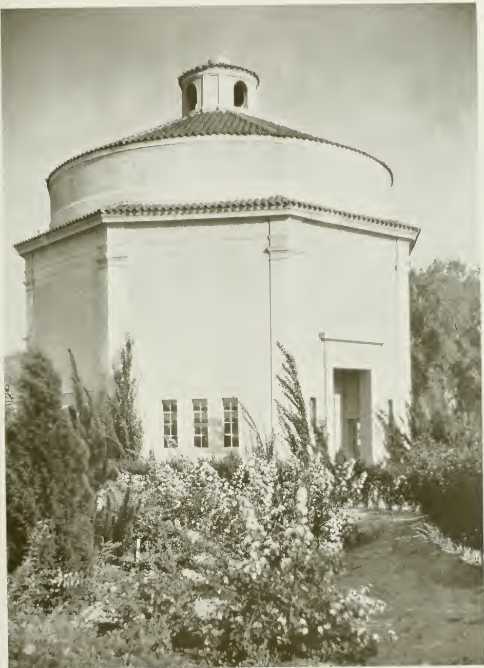
HEAD HOUSE, MUNICIPAL FILTRATION PLANT, SACRAMENTO
