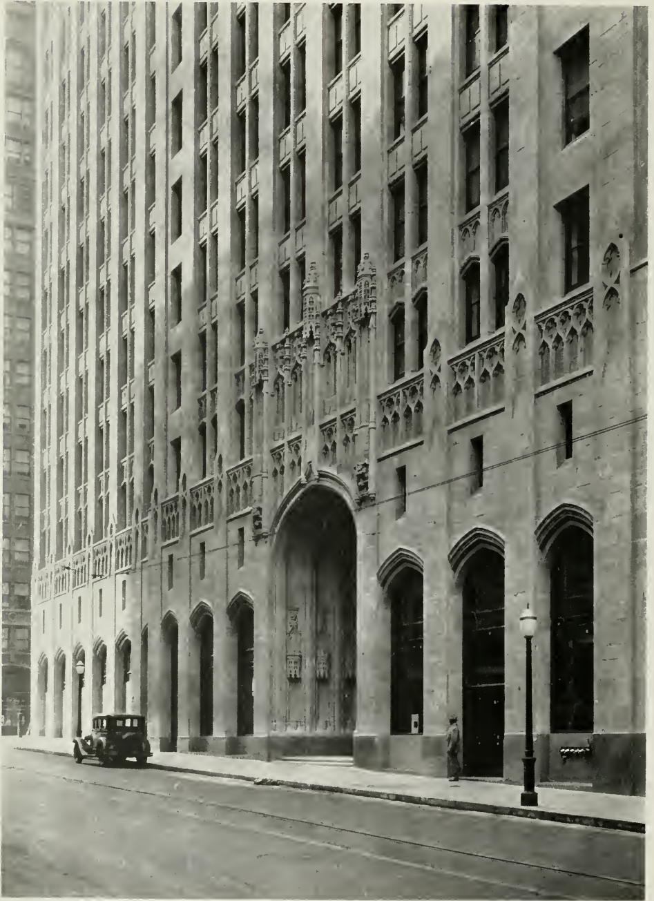
DETAIL OF LOWER FLOORS, RUSS BUILDING, SAN FRANCISCO
