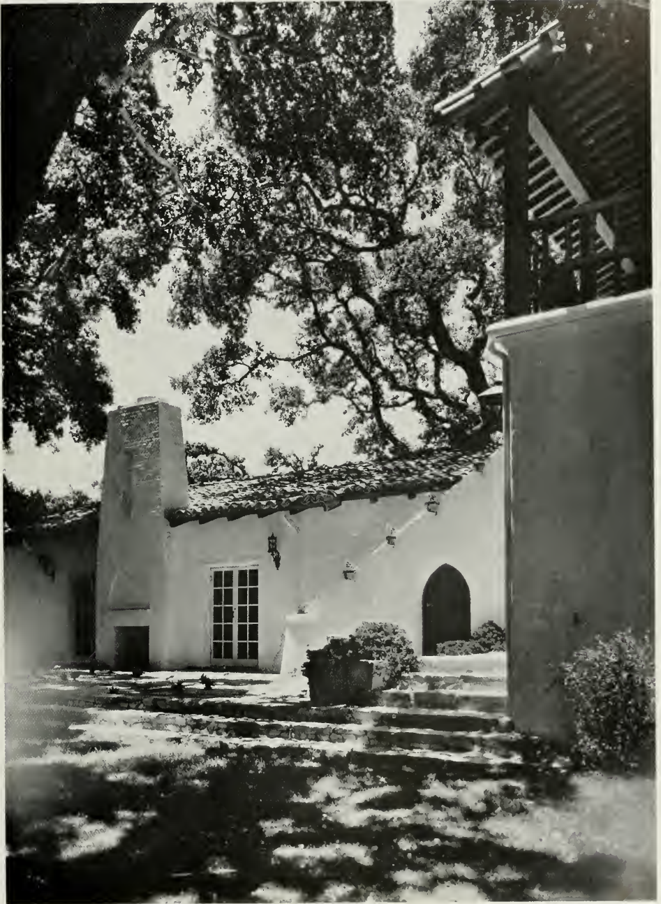
HOUSE FOR MRS. ALMA NEIMAN, HILLSBOROUGH, CALIFORNIA SIDNEY B., NOBLE AND ARCHIE T. NEWSOM, ARCHITECTS
