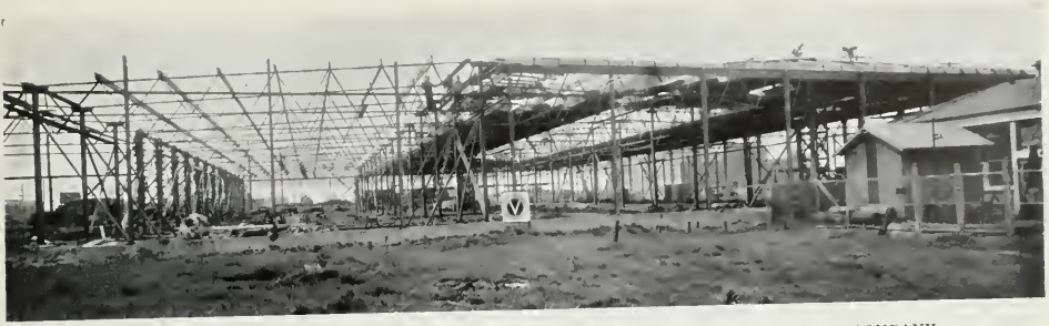
STEEL FRAME (ALL ELECTRICALLY WELDED) SHOP BUILDING FOR ASSOCIATED OIL COMPANY
