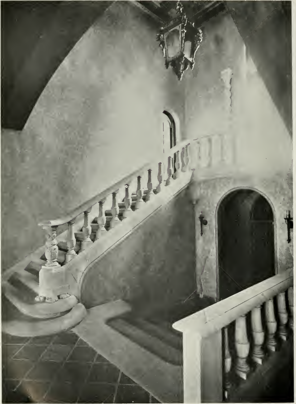
CONCRETE FLOOR AND CAST STONE STEPS, HOUSE OF JAS. SCHULTZ
