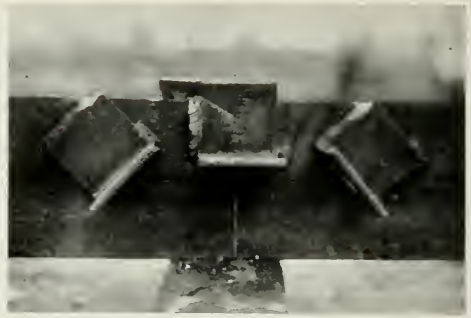
CLIPS FOR CROSS BRACING ON BOTTOM CHORD
