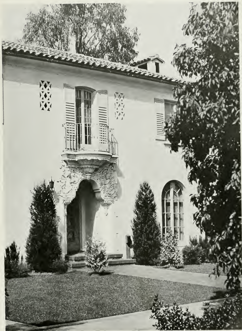
HOUSE FOR MR. JOHN HEPBURN, SAN FRANCISCO, CALIFORNIA B. COOPER CORBETT, ARCHITECT
