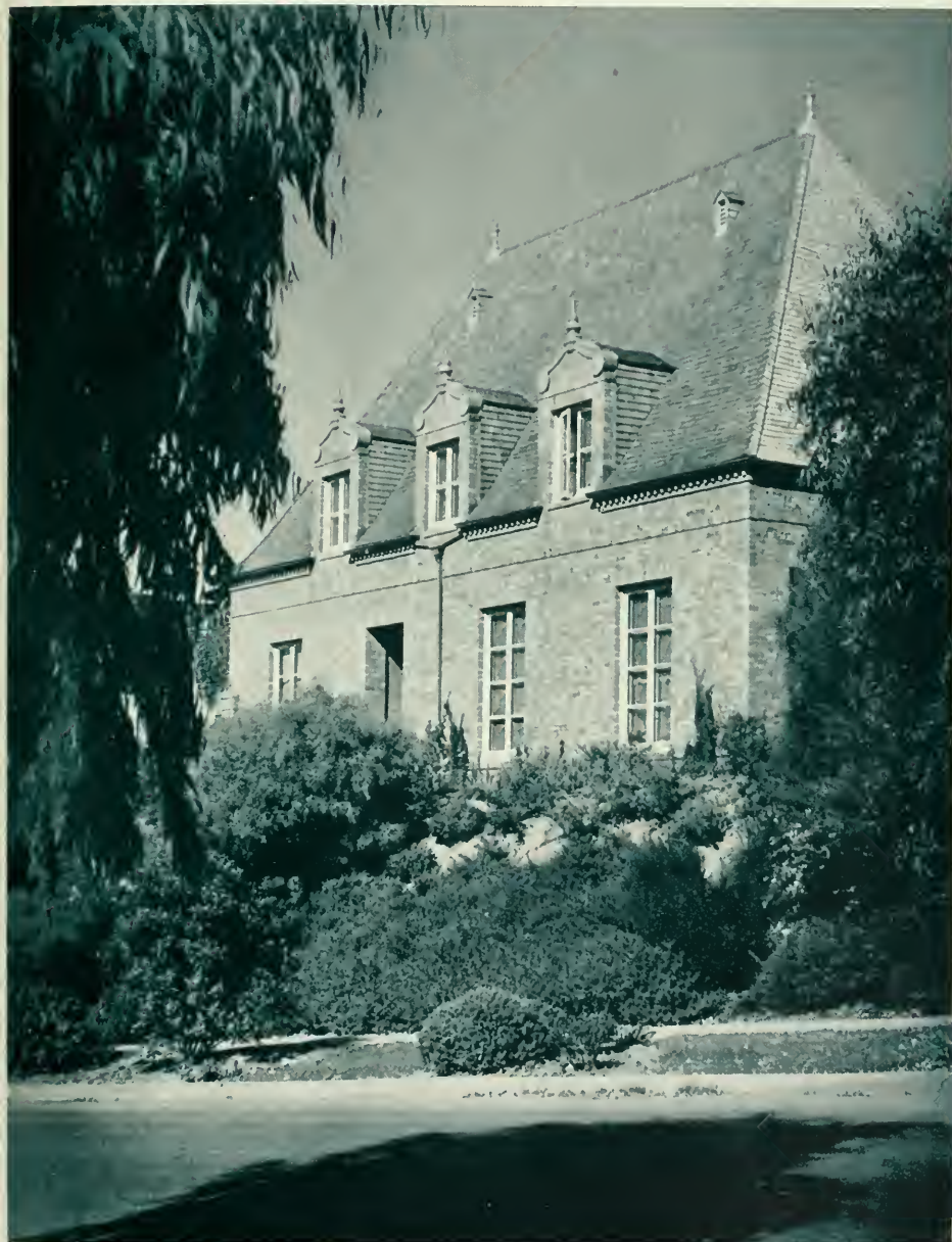
HOUSE FOR MR. A. MEYERS, ST. FRANCIS WOOD, SAN FRANCISCO WILLIAM I. GARREN, ARCHITECT
