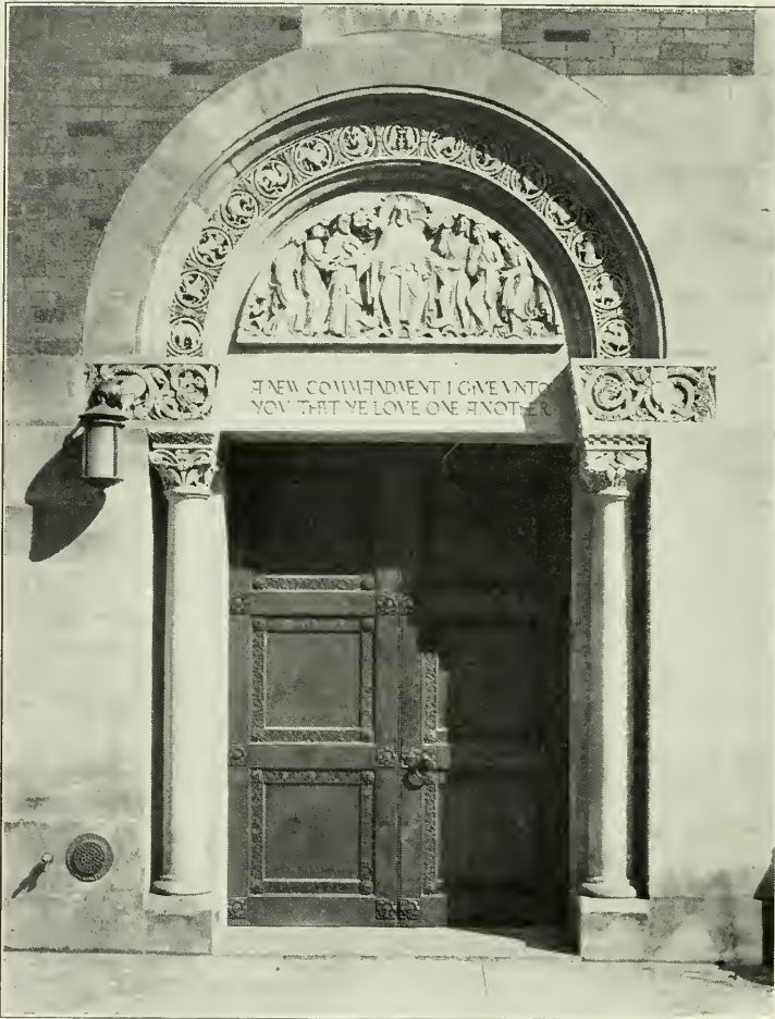
Detail side entrance, St. Bartholomew Community House, New York City. B. G. Goodhue Associates, Architects. Variegated Indiana Limestone base and trim
