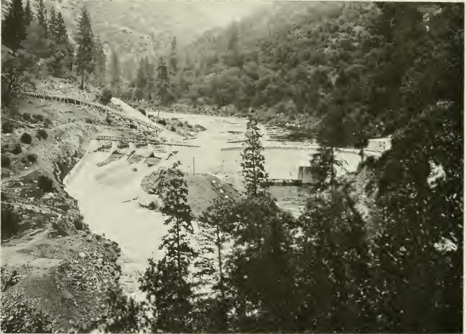
EARLY INTAKE DIVERSION DAM ON TUOLUMNE RIVER
