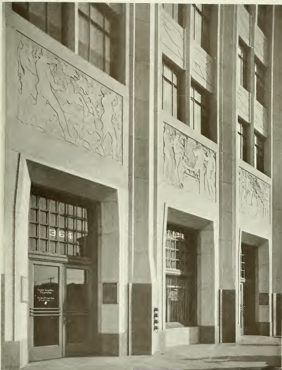
DETAIL OF LOWER STORIES, INCOME SECURITIES BUILDING, OAKLAND FREDERICK H. REIMERS, ARCHITECT
