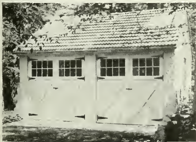
STUCCO GARAGE WITH TILE ROOF
