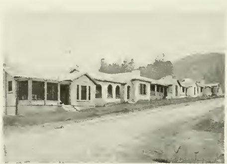
MOCCASIN POWER PLANT OPERATORS' COTTAGES Constructed of Concrete and Tile, Electrically Heated and Lighted
