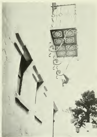
DETAIL, SHOPPE BUILDING, CARMEL
