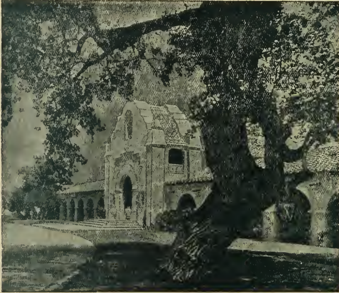
Front view of Agua Caliente Hotel, Tia Juana Hot Springs, Mexico. Wayne B. McAllister of American Building Company, designer and superintendent of construction. Fernando Rodriguez, general contractor. A. A. Barbarosa, plastering contractor. Monolith Waterproof Portland Cement furnished by Squires-Belt Company.
