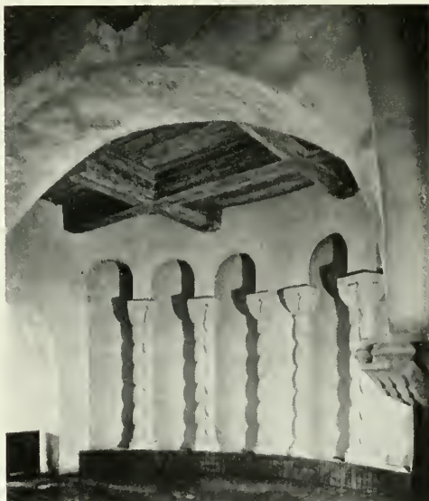
DETAIL, EARLE C. ANTHONY BUILDING
