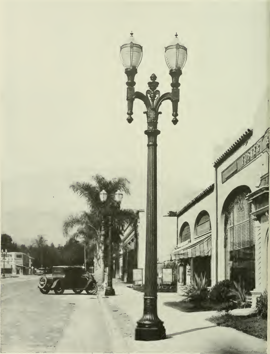
SHOWING ARTISTIC LIGHTING ASSEMBLY FOR COMMERCIAL THOROUGHFARE IN SOUTHERN CALIFORNIA CITY
