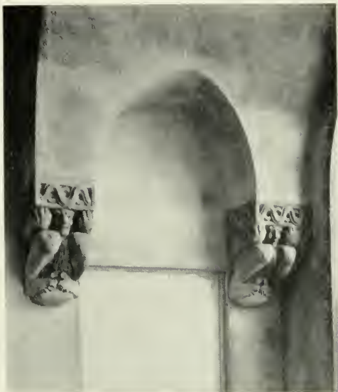
DETAIL, EARLE C. ANTHONY BUILDING
