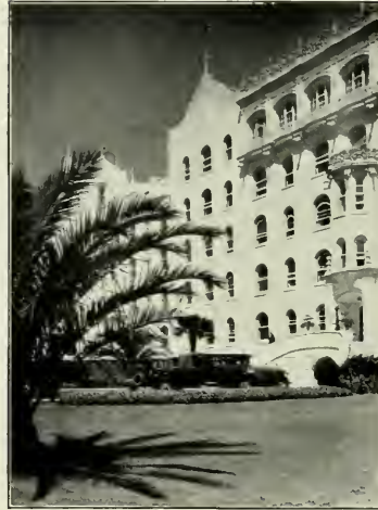
An exterior view of St. Mary's Hospital, San Francisco, Calif. Equipped throughout with McCray Refrigerators
