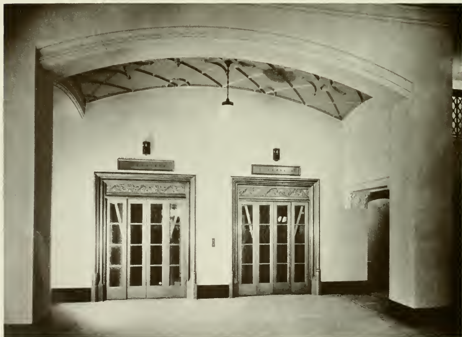
ELEVATOR LOBBY, O'CONNOR-MOFFATT BUILDING, SAN FRANCISCO
