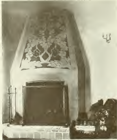
MANTLEPIECE IN FRESCO AND SGRAFFITI William L. Garren, Architect Simeon Pelenc, Decorator
