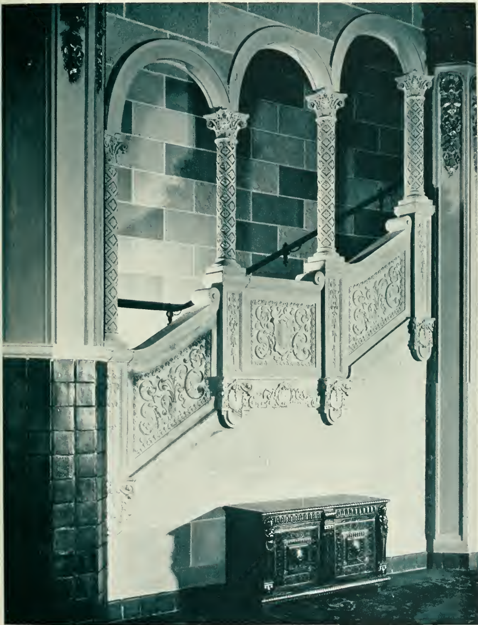
DETAIL OF MAIN STAIRS, WARNER BROS. THEATER, HOLLYWOOD G. ALBERT LANSBURGH, ARCHITECT
