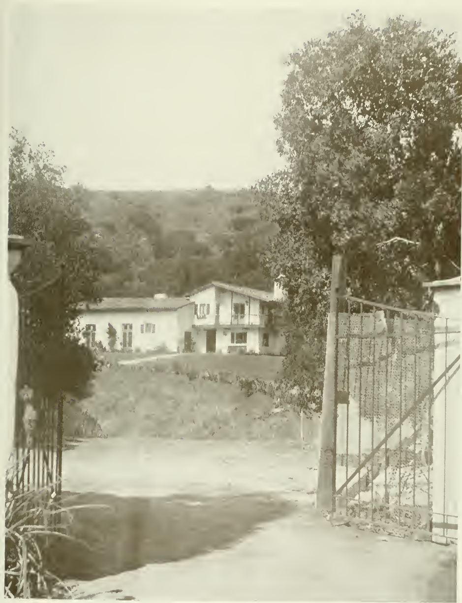
RANCH HOUSE FOR HAROLD W. TUTTLE, LAS TURAS, CALIFORNIA JOHN BYERS, ARCHITECT
