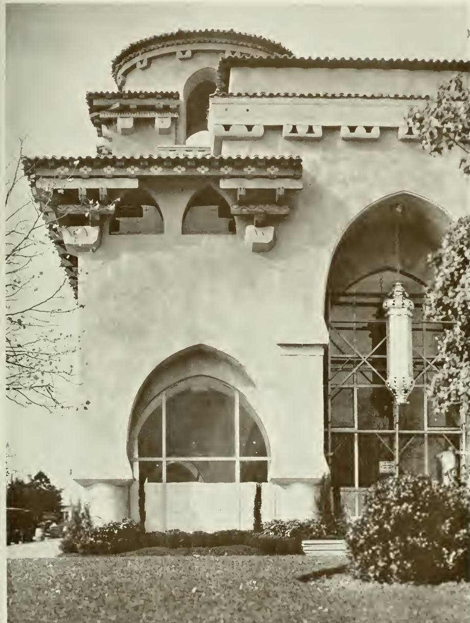
GARDEN VIEW, EARLE C. ANTHONY BUILDING, OAKLAND, CALIFORNIA BERNARD R. MAYBECK, POWERS & AHNDEN, ASSOCIATED ARCHITECTS
