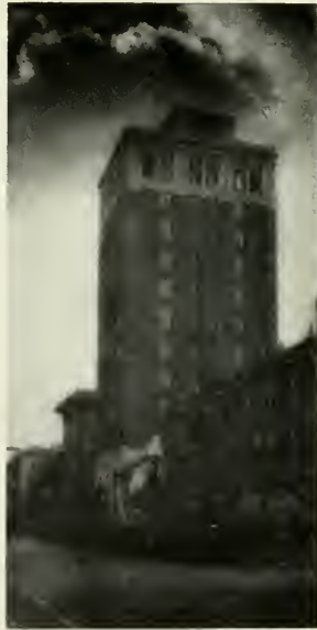
CHAMBER OF COMMERCE BUILDING, BERKELEY W. H. Ratliff, Jr., Architect
