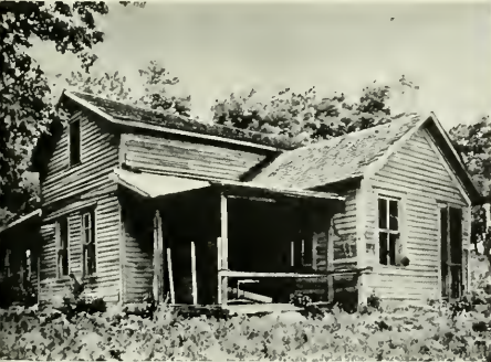
DILAPIDATED FARM HOUSE BEFORE ARCHITECTURAL TREATMENT
