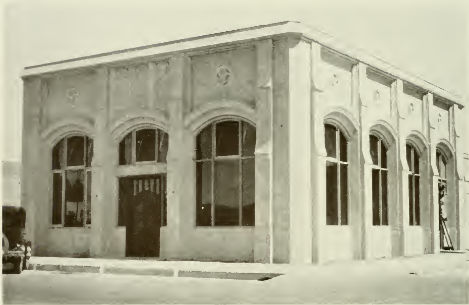
FIRST CORCORAN SECURITIES BUILDING, CORCORAN, CALIFORNIA Chas. D. Vezey & Sons, Builders F. Eugene Barton, Architect
