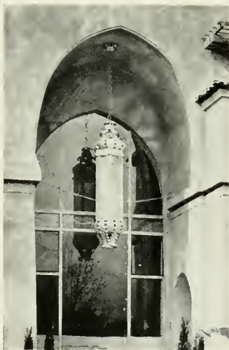
DETAIL, EARLE C. ANTHONY BUILDING OAKLAND
