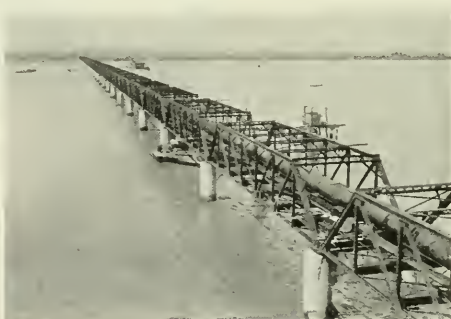
DUMBARTON PIPE BRIDGE, HETCH HETCHY AQUEDUCT
