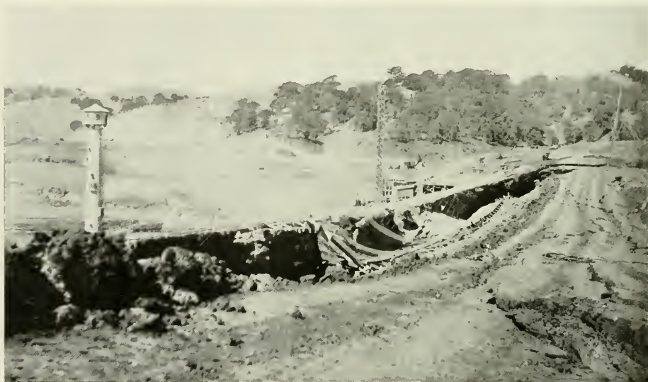
UP-STREAM CREST OF LAFAYETTE DAM, SHOWING SLIPPING OF BODY FROM CONCRETE SKIN
