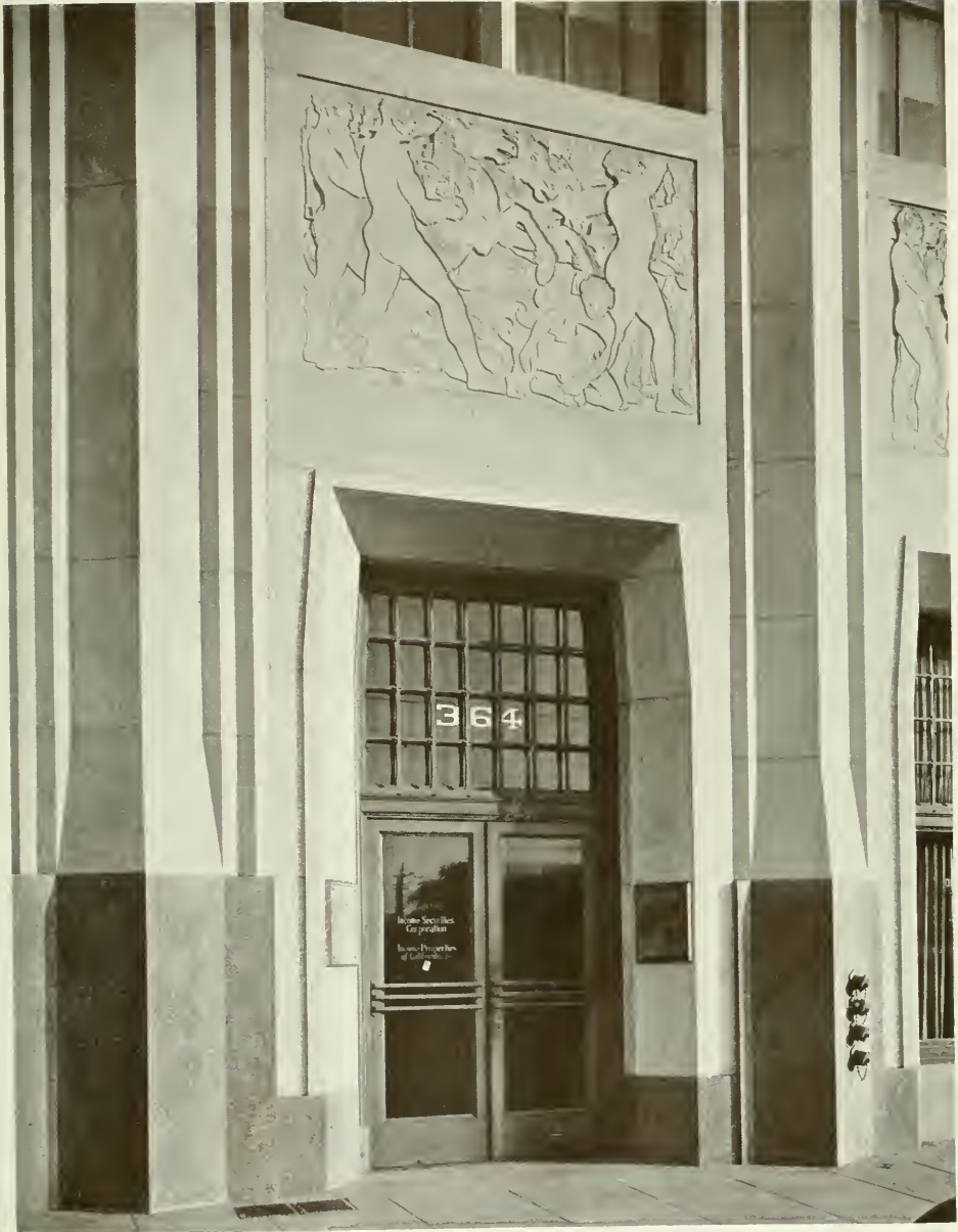
DETAIL OF ENTRANCE, INCOME SECURITIES BUILDING, OAKLAND FREDERICK H. REIMERS, ARCHITECT
