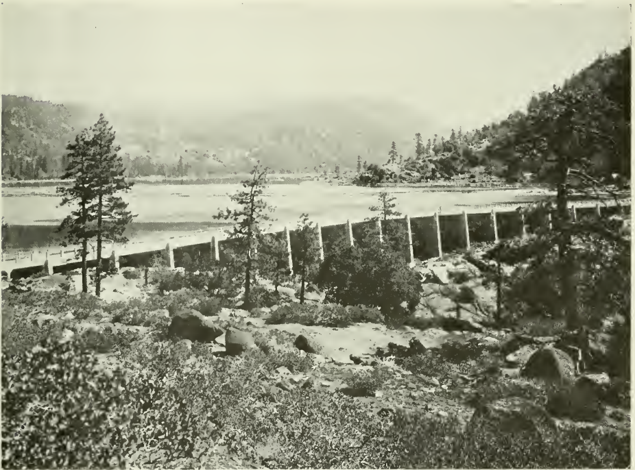
LAKE ELEANOR DAM, HETCH HETCHY PROJECT
