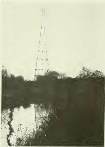
HETCH HETCHY POWER TRANSMISSION LINE TOWERS 208 FEET HIGH, AT CROSSING OF SAN JOAQUIN RIVER, CALIFORNIA
