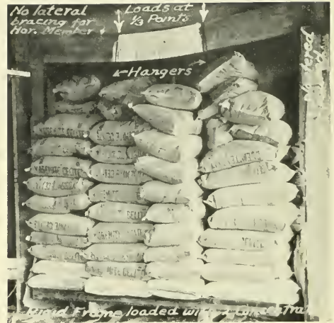
TEST OF FABRICRETE RIGID FRAME
