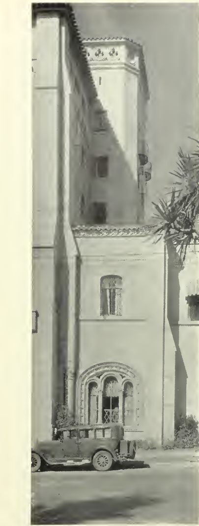
DETAIL, WOMEN'S CITY CLUB Julia Morgan, Architect
