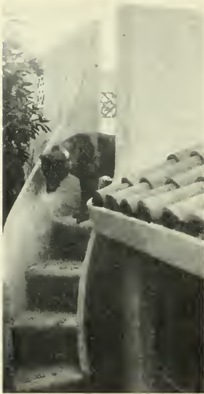
Spiral stair to roof terrace, treads, risers and rails made of stucco. The terrace parapet also of stucco. The terrace parapet also of stucco, is about 11 1/4" thick, 4" high and 8" long, reinforced with netting and 3/8" rods. Tests have proven that it has ample strength.
