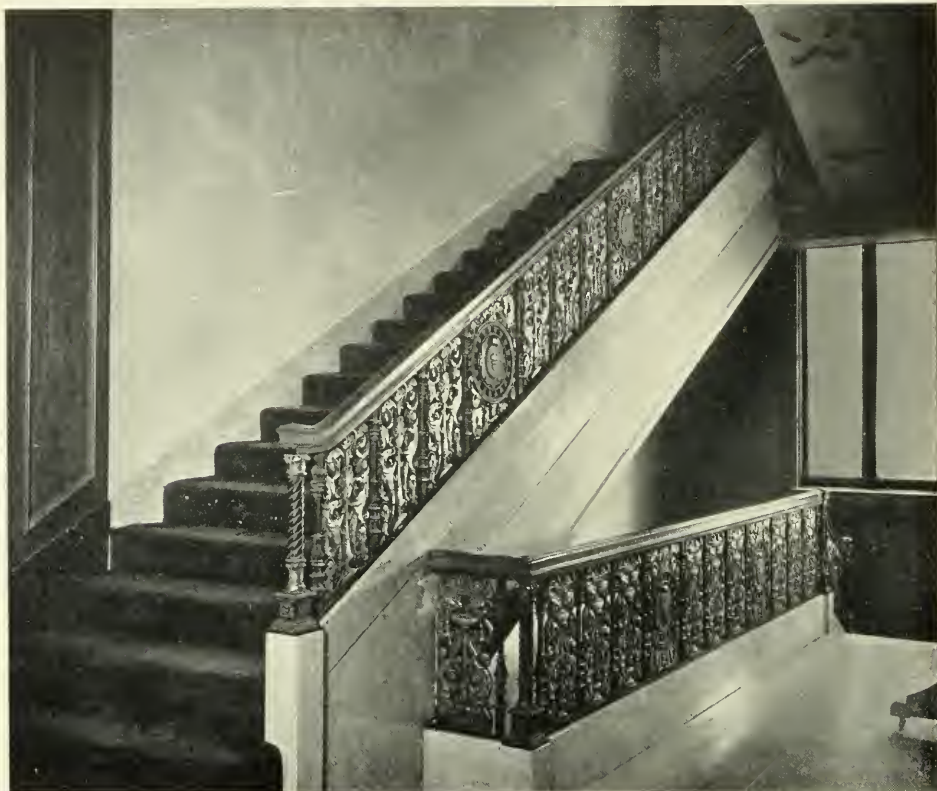
CAST IRON RAIL, MAIN STAIRCASE, SIR FRANCIS DRAKE HOTEL, SAN FRANCISCO Weeks and Day, Architects
