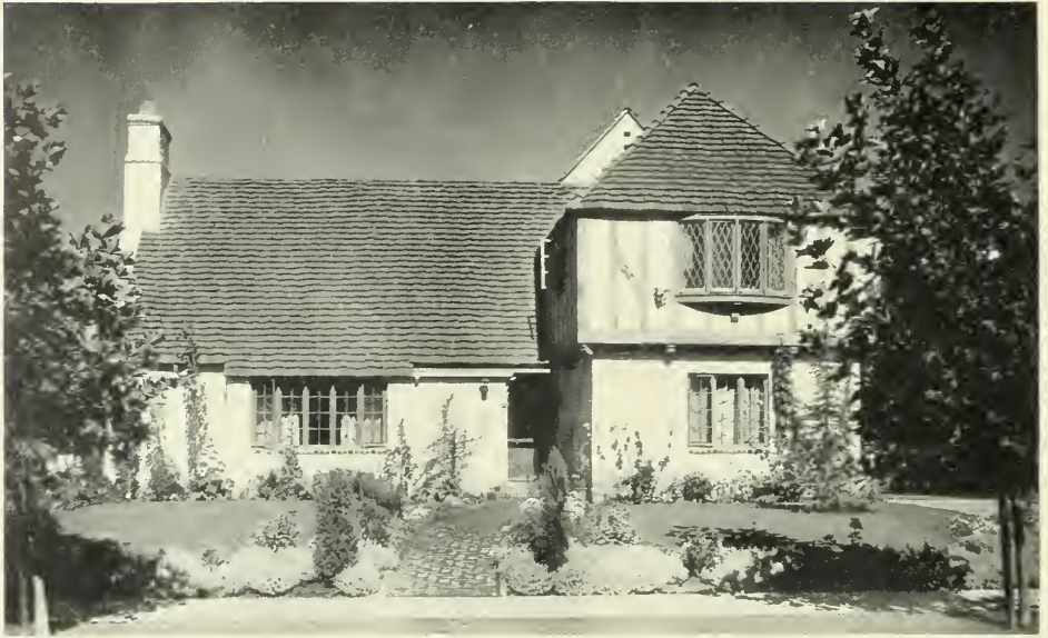
RESIDENCE OF FRANKLIN DONNELL, BEVERLY HILLS, CALIFORNIA H. Roy Kelley, Architect
