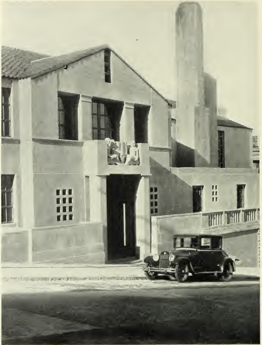
ENTRANCE, TEACHERS STATE COLLEGE, SAN FRANCISCO GEORGE B. McDOUGALL, STATE ARCHITECT
