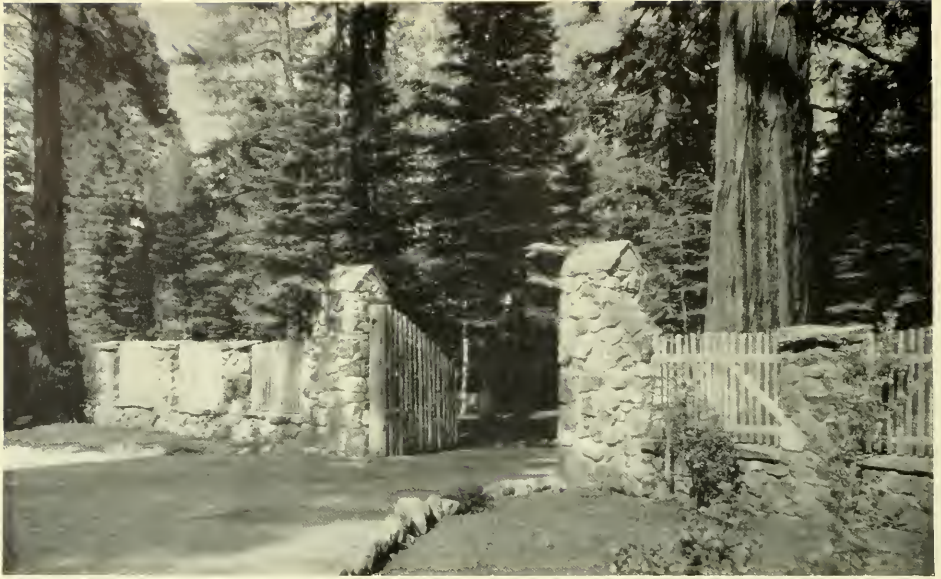
HIGHWAY APPROACH, HOUSE OF MRS. LAURA B. WESTPHAL, LAKE TAHOE Kent and Hass, Architects
