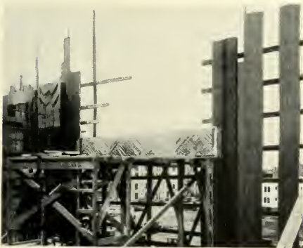
PLASTER WASTE-MOLD SET IN PLACE
