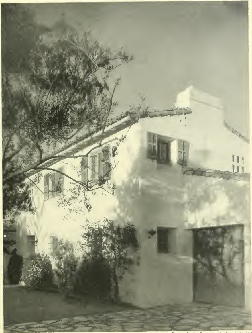
Equipped with Payne gas fired unit furnaces
