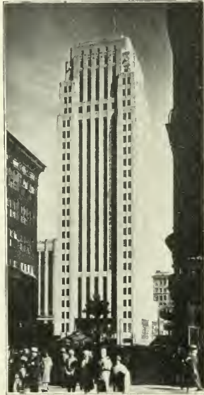
RAND TOWER, MINNEAPOLIS Holabird & Root, Architects
