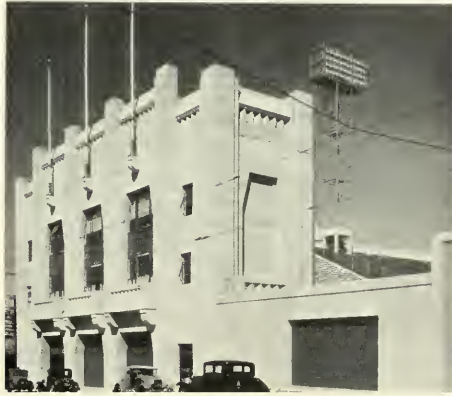
MAIN ENTRANCE AND OFFICE WING Note light tower on right with 48 reflectors
