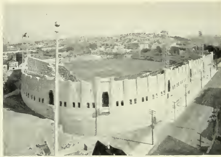
GENERAL VIEW OF STADIUM FROM OUTSIDE
