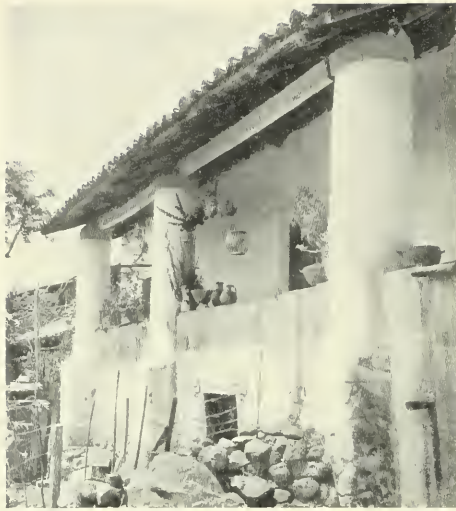
DETAIL, THE GROCER'S HOUSE, TAXCO, MEXICO Door and window trim and column caps are flat painted bands of cobalt blue. Adobe walls on masonry foundation several feet above ground.
