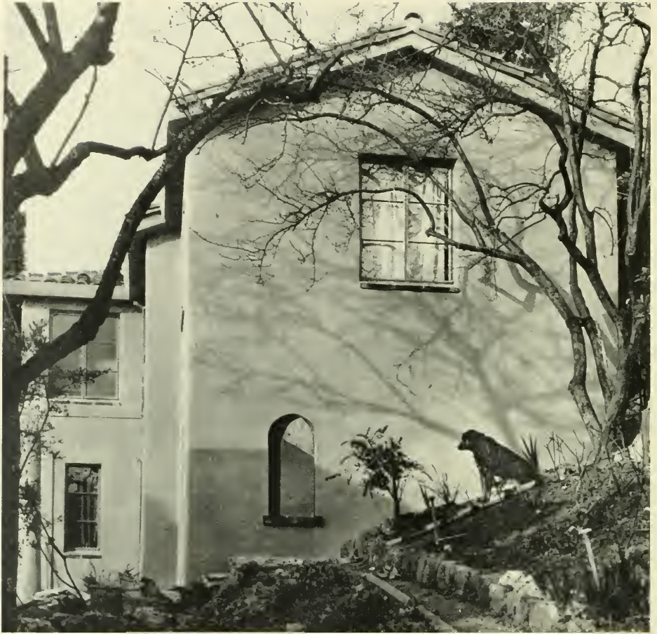
COTTAGE AT 4 MOSSWOOD LANE, BERKELEY, CALIFORNIA NEARING COMPLETION, FEBRUARY, 1931
