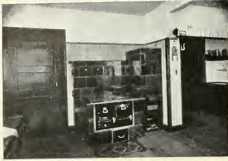
A COMBINATION COOKER AND HEATER Typical Cottage, Gronauerwald, Germany
