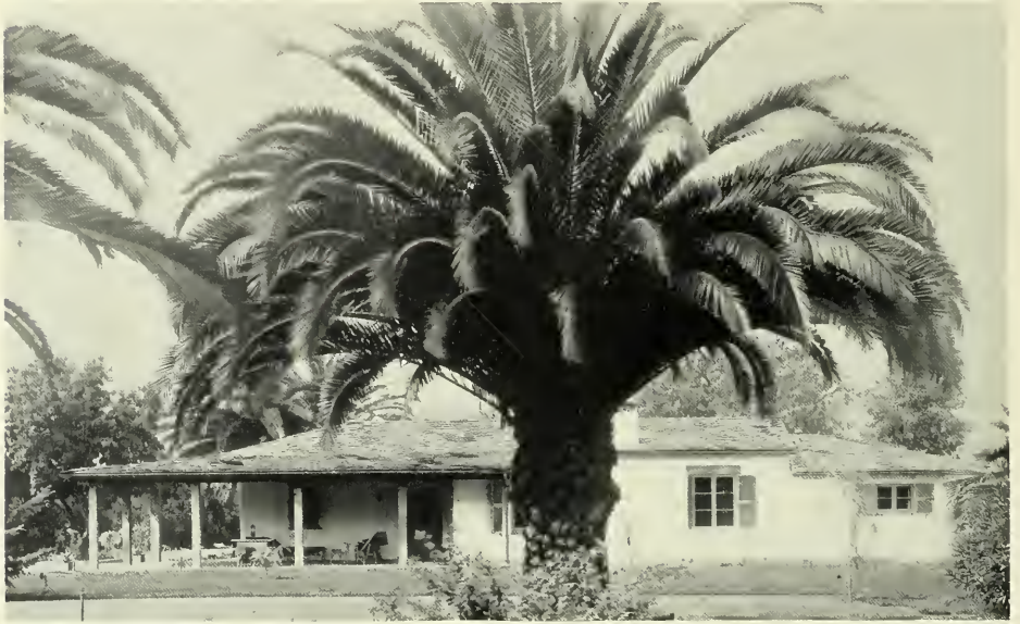
RANCH HOUSE FOR JAMES K. TWEEDY, DOWNEY, CALIFORNIA Roland E. Coate, Architect
