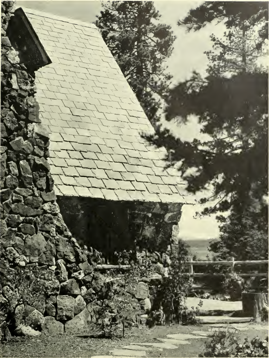
Slate Roof by General Roofing Company
