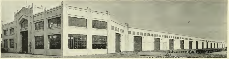
Pier 48—San Francisco
