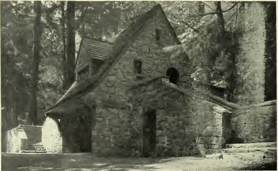
MACLEAY PARK SHELTER, PORTLAND, OREGON Ernest F. Tucker, Architect
