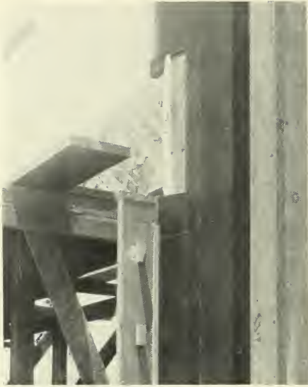
FORMS PARTIALLY LINED WITH FIBRE BOARD
