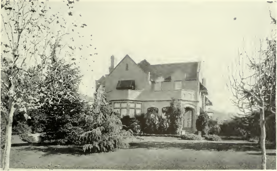
RESIDENCE OF M. B. SKAGGS, PIEDMONT, CALIFORNIA B. J. S. Cahill, Architect
