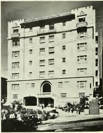
Redstone Apartments in San Francisco. Henry C. Smith, Architect; J. A. Pasqualetti, Owner and Builder. Cabot's Triple-ply Quilt in all partitions.
