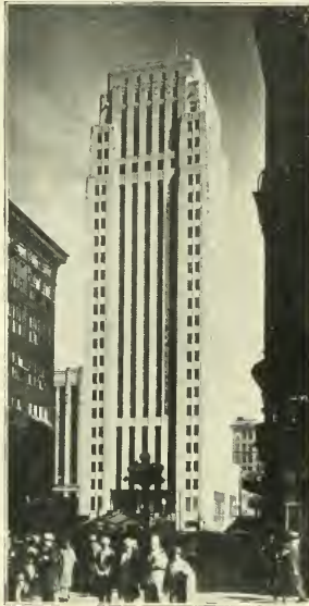
RAND TOWER, MINNEAPOLIS Holabird & Root, Architects
