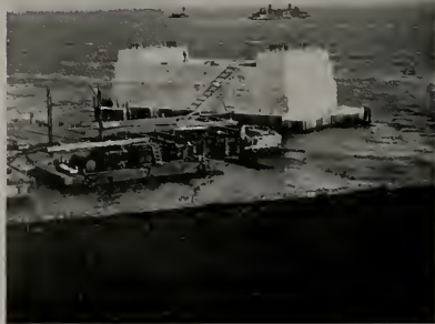
Golden Gate Bridge two years ago. Base of the San Francisco Pier beginning to show its massive proportions
