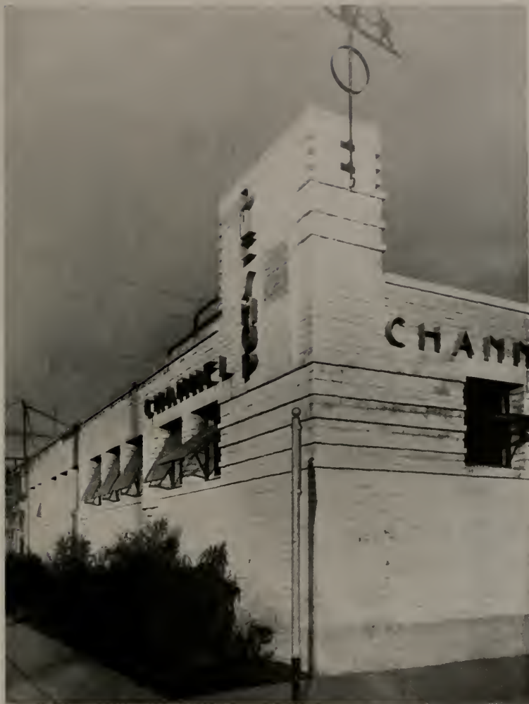
CHANNEL PIE SHOP, SACRAMENTO, CALIFORNIA HARRY J. DEVINE, ARCHITECT
