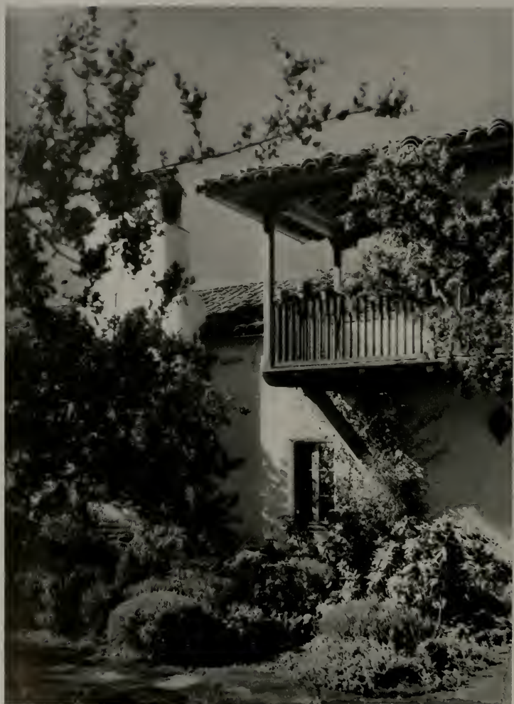
GARDEN VIEW, RESIDENCE OF CLARENCE A. TANTAU, BERKELEY CLARENCE A. TANTAU, ARCHITECT
