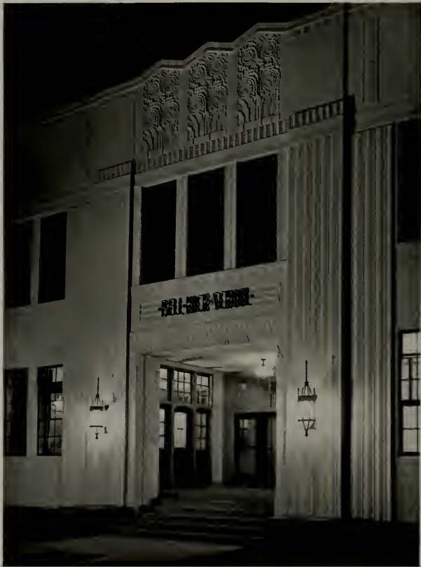
NIGHT VIEW OF ENTRANCE, BELL HIGH SCHOOL, BELL, CALIFORNIA ROBERT F. TRAIN, ARCHITECT
