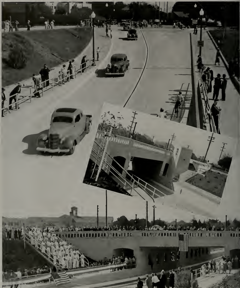
The Embarcadero Underpass at Palo Alto, California. The underpass carries the Embarcadero roadway beneath the tracks of the Southern Pacific railroad and the roadway of Alma Street, both of which are accommodated on the structure above. The top picture shows the wide subway for the Embarcadero lateral swinging down to the underpass with pedestrian ramps on either side. Inset is a view of the structure that carries railroad and Alma Street over the subway. Lower picture is the scene on dedication day.
