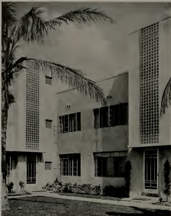
EXTERIOR VIEW OF CLUB BUILDING, SHOWING USE OF GLASS BLOCKS FOR STAIRHALL ILLUMINATION
