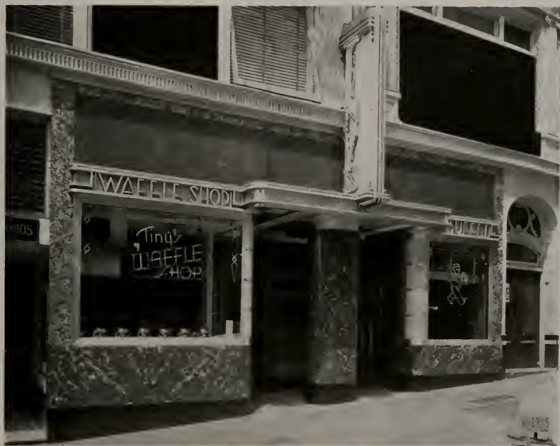
TINY'S WAFFLE SHOP, SAN FRANCISCO, AFTER ALTERATIONS WILLIAMS AND GRIMES, ALBERT R. WILLIAMS, ARCHITECT
