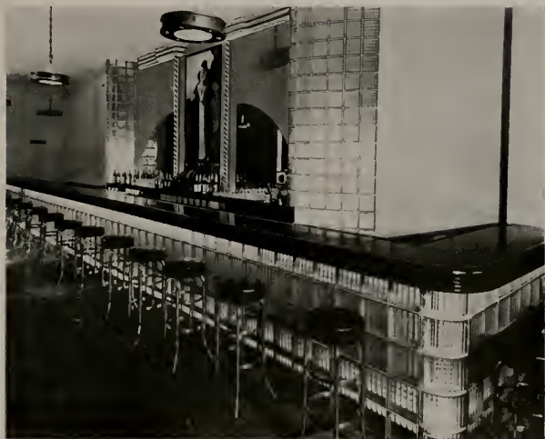
SHOWING APPLICATION OF GLASS BLOCK AS A DECORATIVE MATERIAL. BLOCKS USED IN BAR ILLUMINATED WITH COLORED LIGHTS FROM BEHIND
