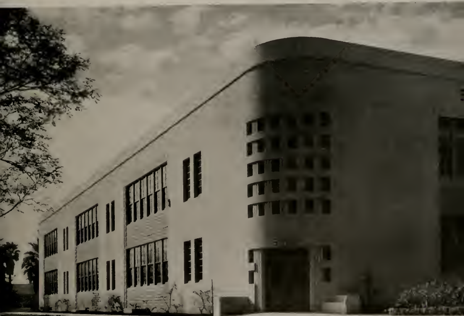
SCIENCE BUILDING, HOLLYWOOD HIGH SCHOOL, HOLLYWOOD, CALIFORNIA Marsh, Smith and Powell, Architects
