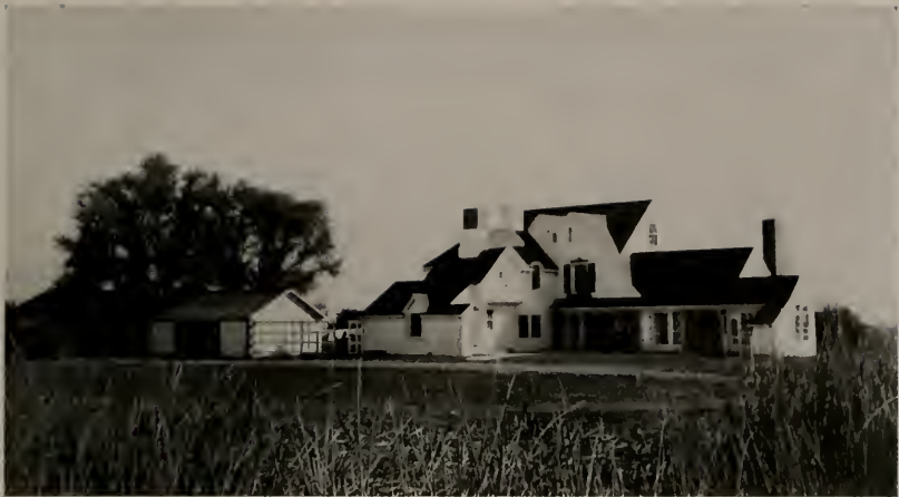
RESIDENCE OF MR. AND MRS. GEORGE WILSON, CLARKSBURG, CALIFORNIA W. R. Yelland, Architect
