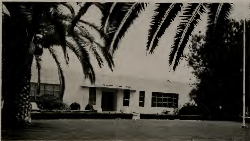
VIEW FROM LAWN, BRADFORD AVE SCHOOL, PLACENTIA, CALIFORNIA T. C. Kistner, Architect
