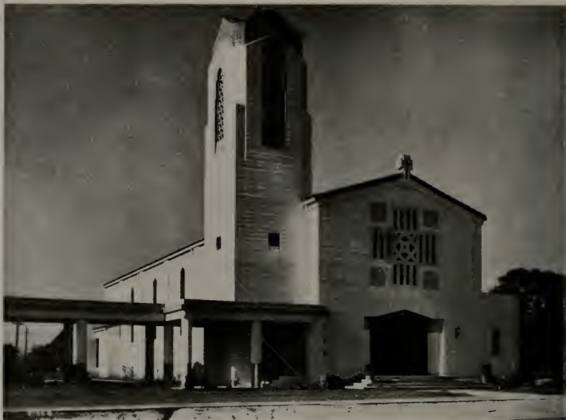
ST. JOSEPH'S CHURCH, NORTH SACRAMENTO, CALIFORNIA Harry J. Devine, Architect
