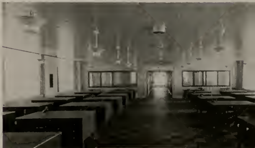
GENERAL OFFICE IN INDUSTRIAL PLANT, SHOWING THE USE OF GLASS BLOCKS FOR HEAT INSULATING FILLERS FOR WINDOW OPENINGS
