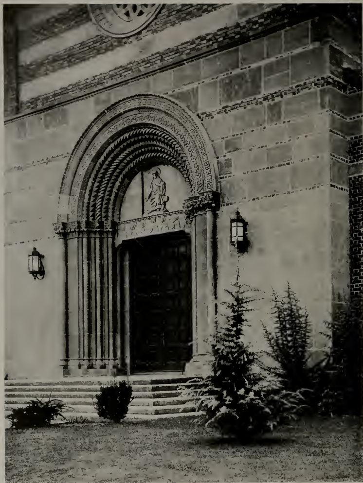
DETAIL OF ENTRANCE, SACRED HEART CHURCH, SACRAMENTO HARRY J. DEVINE, ARCHITECT
