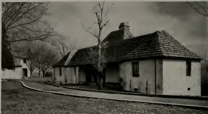
GUEST HOUSE, ESTATE OF MR. AND MRS. P. M. PIKE, SARATOGA HIBBARD, GERITY & KERTON, ARCHITECTS
