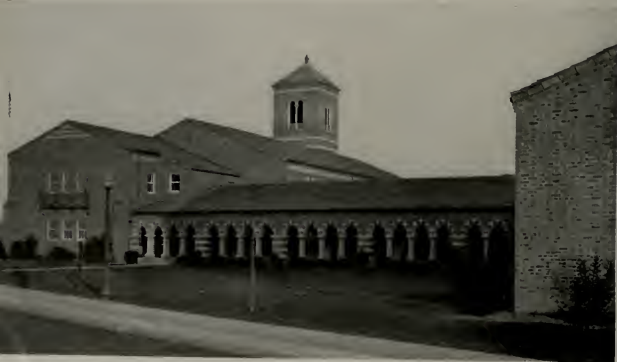
CALIFORNIA JUNIOR HIGH SCHOOL, SACRAMENTO, CALIFORNIA Harry J. Devine, Architect
