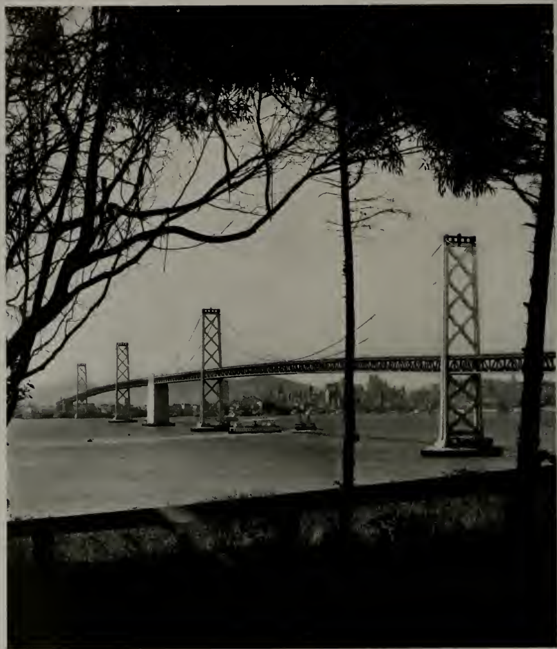
LATE VIEW OF SAN FRANCISCO-OAKLAND BAY BRIDGE
