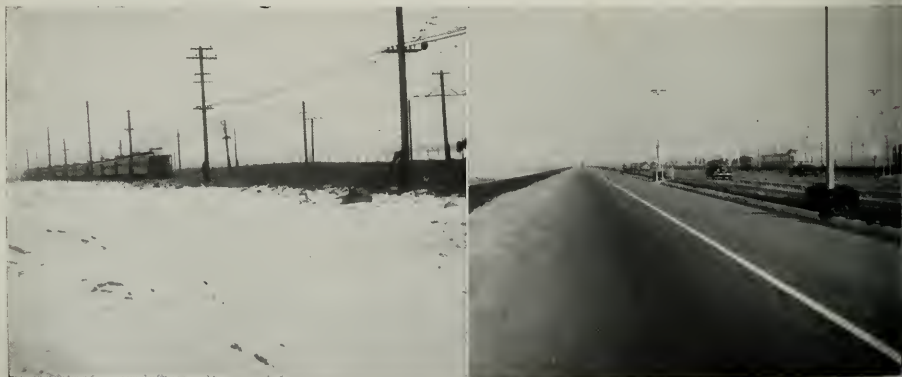
Before—Dredged sand fill between east end of bridge and Toll Plaza. After—Ice plant ground cover on bayside and center strip.
