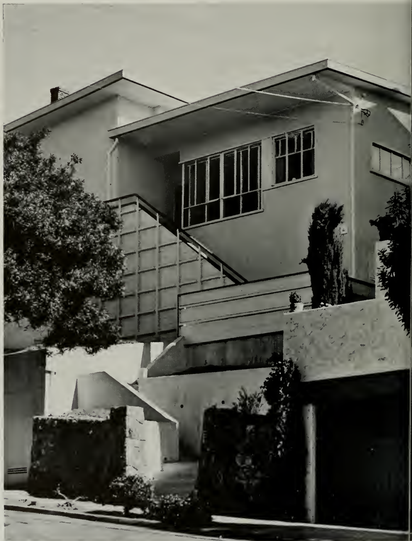
HILLSIDE APPROACH FROM STREET
