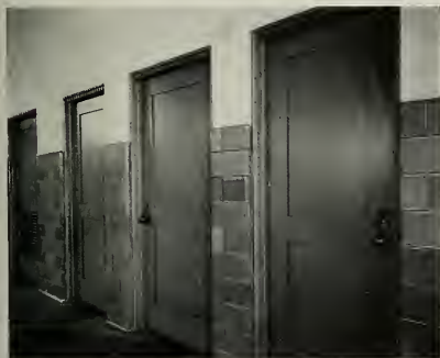
Detail of five-foot wainscoting of Kraftile 6x9's at doors of service rooms of Fresno fire department headquarters. The tile is stain-proof, acid proof and easily cleaned. The larger size of tile facilitates the wainscots design.
