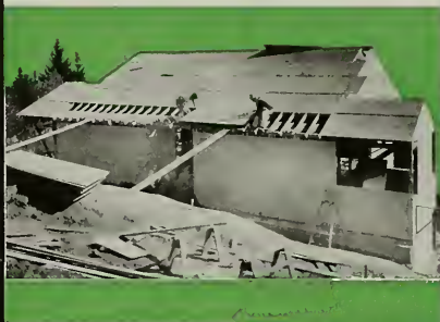
On this Portland, Oregon, home, 5/16" Plyscord was used as wall sheathing, 3/8" as roof sheathing and 5/8" as sub-flooring. (The 5/8" Plyscord was used first as concrete form material.) This house is 40% more rigid than if diagonal board sheathing had been used. Cutting, fitting and nailing were minimized. The 5/8" Plyscord sub-floor, for example, went down in just half the usual time. Richard Sundeleal was the architect.
