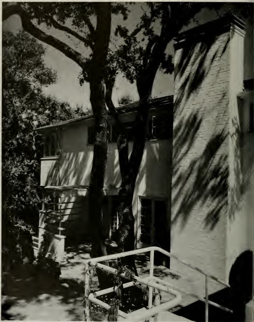
ENTRANCE DETAIL, HOUSE FOR MR. ORTON LUCAS, ORINDA, CALIFORNIA FREDERICK L. CONFER, ARCHITECT
