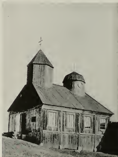
RUSSIAN CHAPEL AT FORT ROSS, SONOMA COUNTY, BUILT OF REDWOOD 121 YEARS AGO AND STILL WELL PRESERVED
