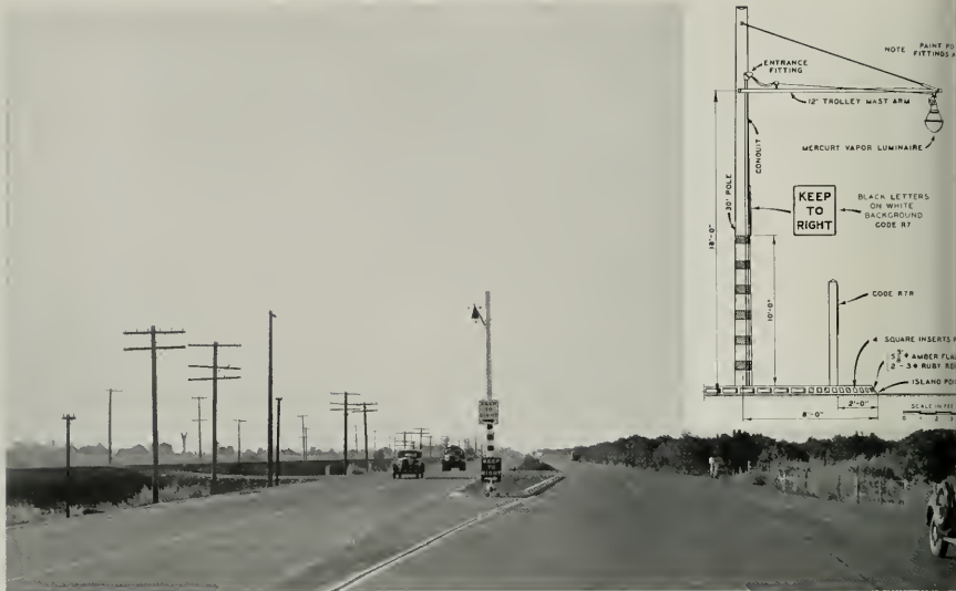
Daylight view of new divisional island lighting equipment on 30-foot pole with 12-foot arm 18 feet above ground.
