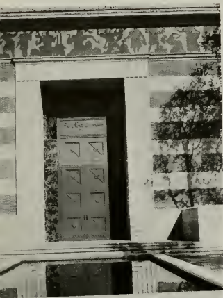
DETAIL OF 15 FT. MAIN ENTRANCE TO HARRIS HALL OF ARCHITECTURE AND FINE ARTS, U. S. C., LOS ANGELES.
