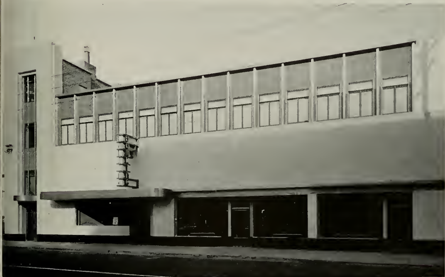
THOMAS KEEN BOWLING ALLEY AND OFFICE BUILDING, BURLINGAME, CALIFORNIA CAHILL BROS., BUILDERS
