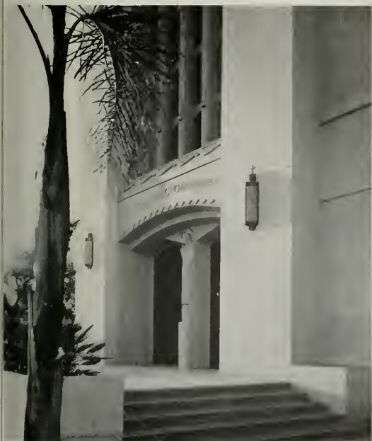
DETAIL OF ENTRANCE, ALL SOULS CHURCH, ALHAMBRA, CALIFORNIA
