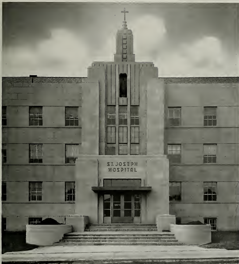
ENTRANCE DETAIL, ST. JOSEPH HOSPITAL, FOR SISTERS OF ST. FRANCIS, LA GRANDE
