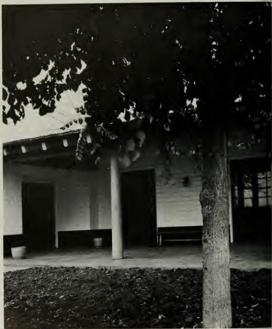
CASTRO VALLEY KINDERGARTEN AND COMMUNITY CENTER NEAR HAYWARD, CALIFORNIA
