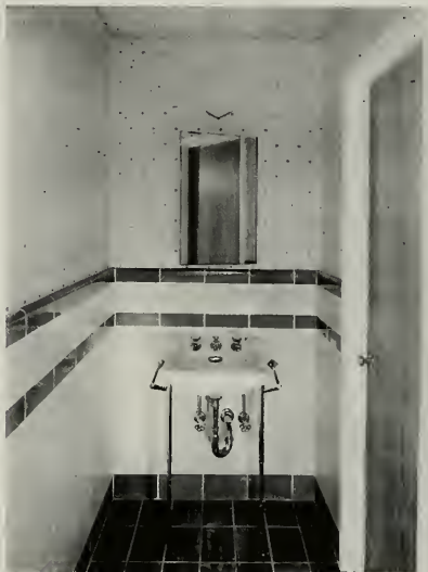
LARGE SIZE TILE USED EFFECTIVELY IN HOME OF R. R. STUART, SAN LEANDRO IRWIN M. JOHNSON, ARCHITECT
