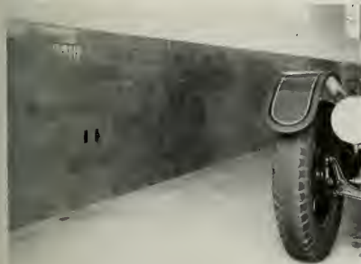
Kraftile was also specified for the equipment room of the Fresno headquarters. The wainscoting has a bullnose top course. Kraftile is considered ideal for such installations. Edward W. Peterson, architect; C. E. McMullen, tile contractor.
