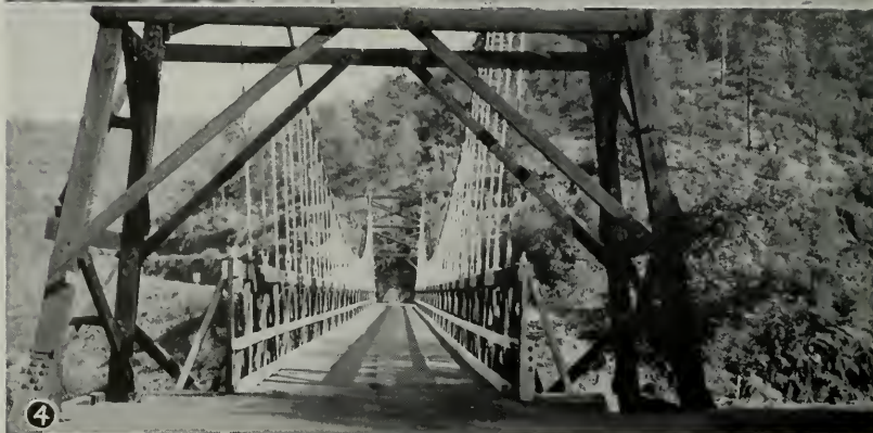
Pictures 1 and 2 show decay in bents of this timber overhead structure evidenced by settlement of the deck. No. 3—A defect in expansion detail of concrete girder structure resulted in disintegration of beam. Note temporary timber supports on shallow footings. No. 4—One-way timber suspension span posted and reinforced by adding additional hangers between originals.
