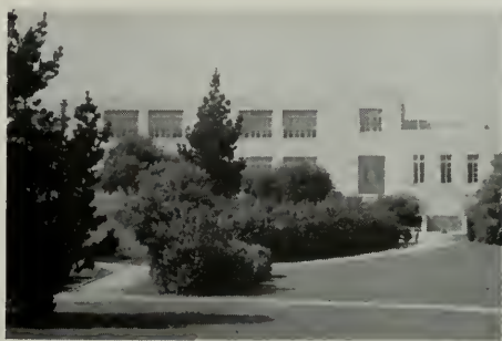
APPROACH TO MAIN ENTRANCE, EL SEGUNDO SCHOOL, EL SEGUNDO, CALIFORNIA
