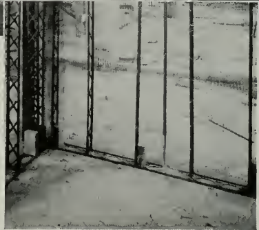
Interior view, showing hollow partition construction
