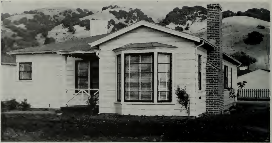
STREET VIEW OF ONE STORY FRAME HOUSE, PAINTED WHITE WITH GREEN TRIM, BRICK CHIMNEY, SHINGLE ROOF AND VENETIAN BLINDS
