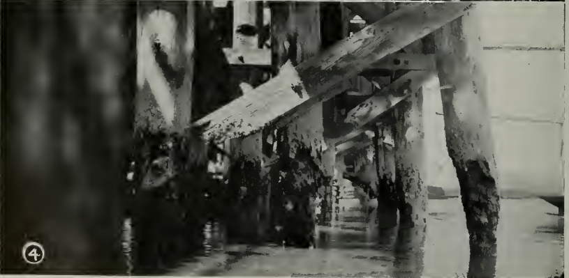
Picture 1—Light, narrow bridge posted and likely to collapse if struck by a vehicle out of control; (2) Inadequate expansion detail in concrete girder span caused serious cracking; (3) Poor concrete in pile coupled with abrasion by floating drift resulted in pronounced weakening; (4) Support piles weakened by marine borers.
