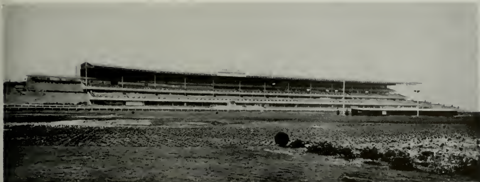
GENERAL VIEW OF THE HUGE GRANDSTAND, ALBANY, CALIFORNIA
