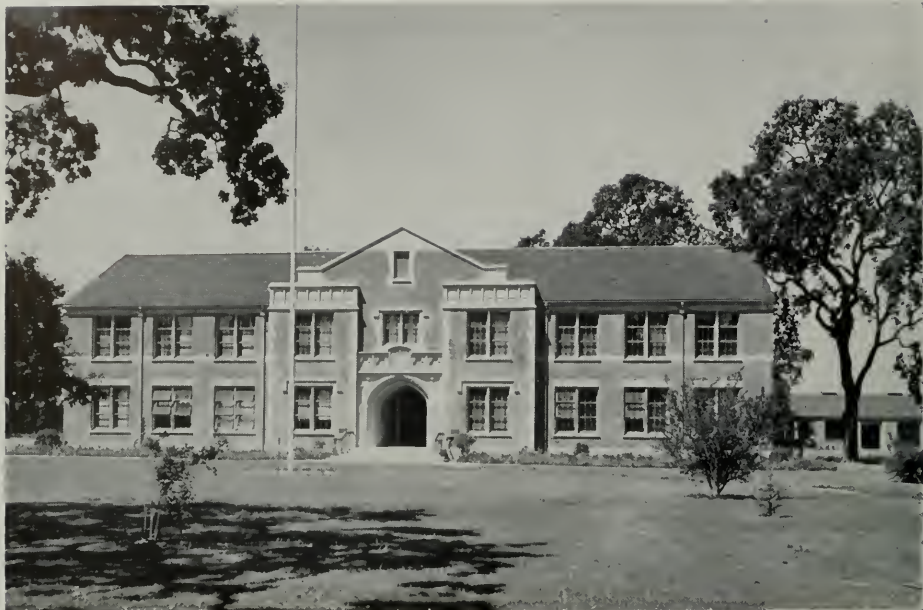
LIBRARY AND ADMINISTRATION BUILDING, SANTA ROSA JUNIOR COLLEGE
