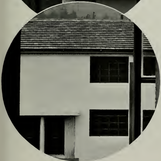
Photos taken from SUNNYDALE HOUSING PROJECT, San Francisco
