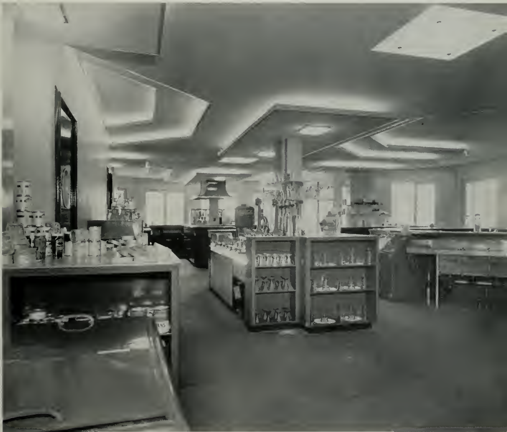
INTERIOR, SHOWING TUBE LIGHTING, NEW CAFE, PORTLAND, OREGON Roi L. Morin, A.I.A., Architect
