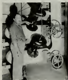
Upper left: Walt Disney (right) and Chief Engineer William E. Garity inspect the Johnson central control panel in the Camera Building. Above: Johnson valves on hot water heating mains in the Central Heating Plant.
