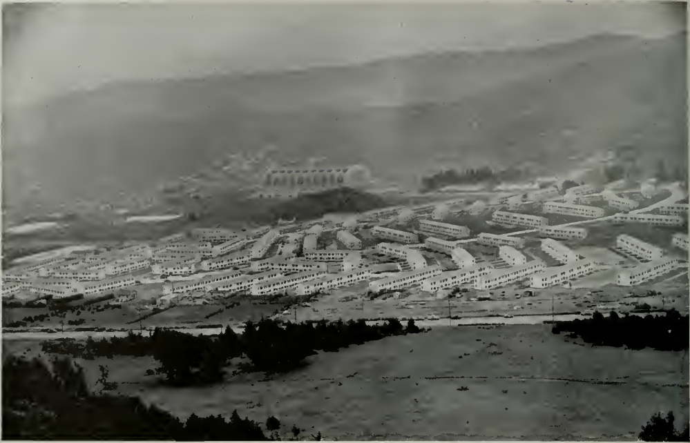
PANORAMIC VIEW OF SNNNYDALE LOW RENT HOUSING PROJECT, VISITACION VALLEY, SAN FRANCISCO
