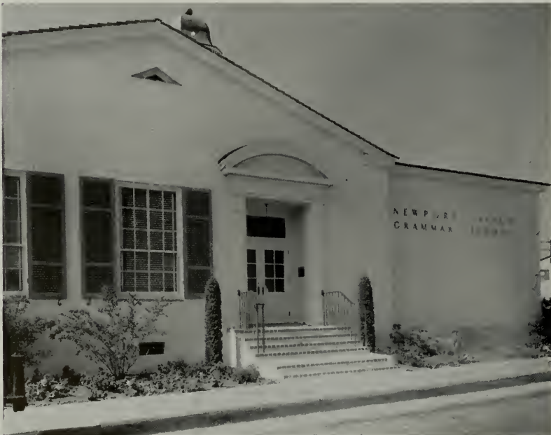
DETAIL OF ENTRANCE
