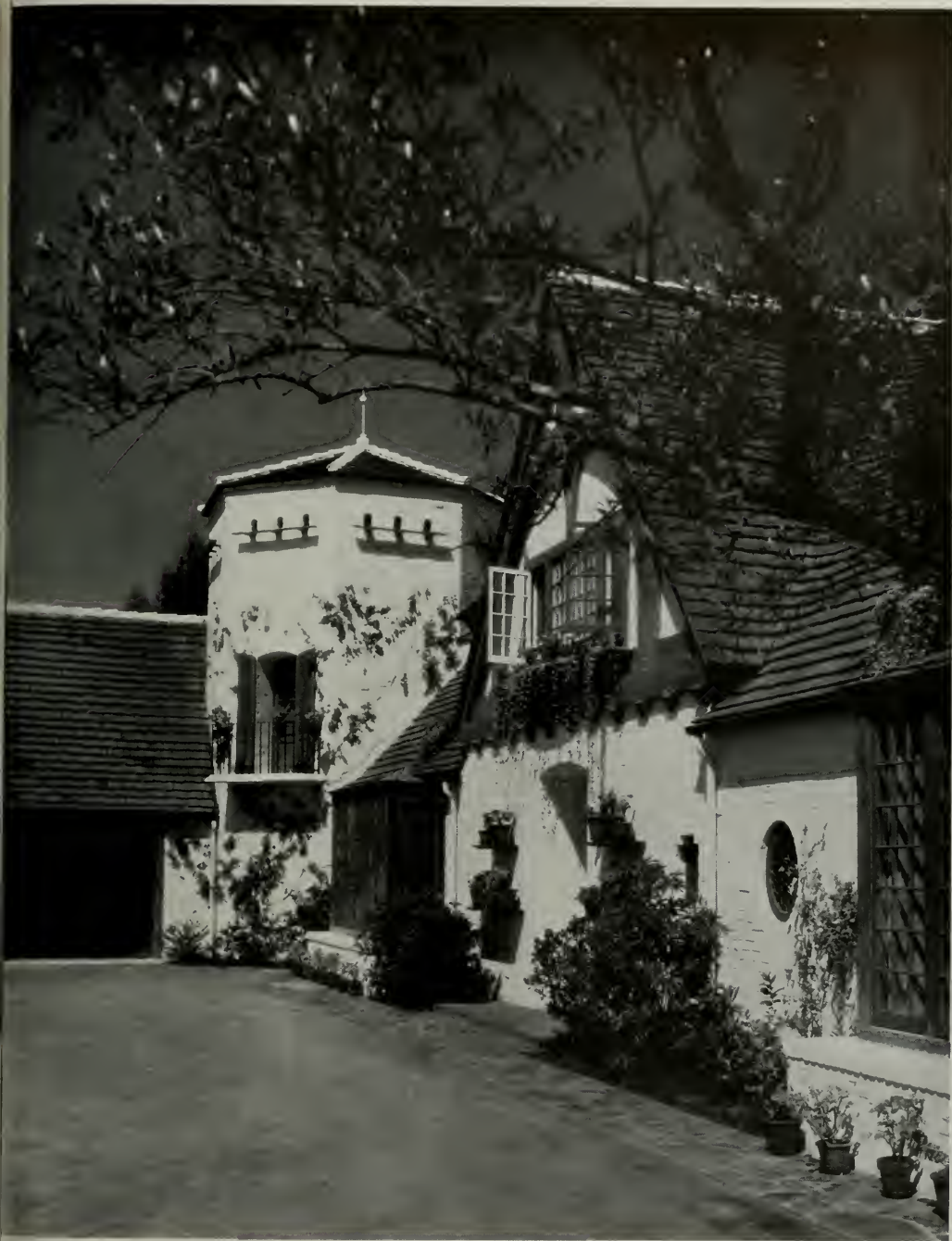
DETAIL OF FRONT, SHIRLEY BURDEN RESIDENCE, BEVERLY HILLS Wallace Neff, Architect
