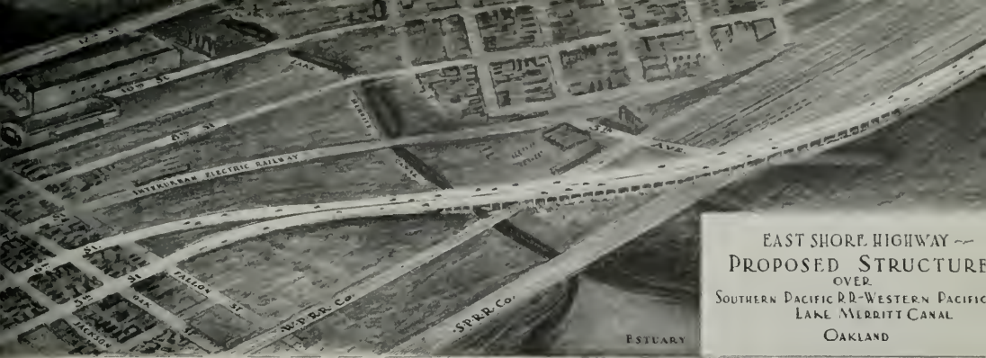
Proposed Divided Highway Structure for East Shore traffic over Lake Merritt Canal and railroad tracks, Oakland
