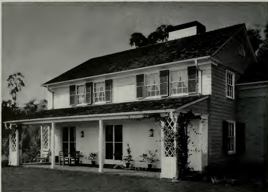
residence for mr. and mrs. charles lane, linda vista, california theodore l. pletsch, architect
