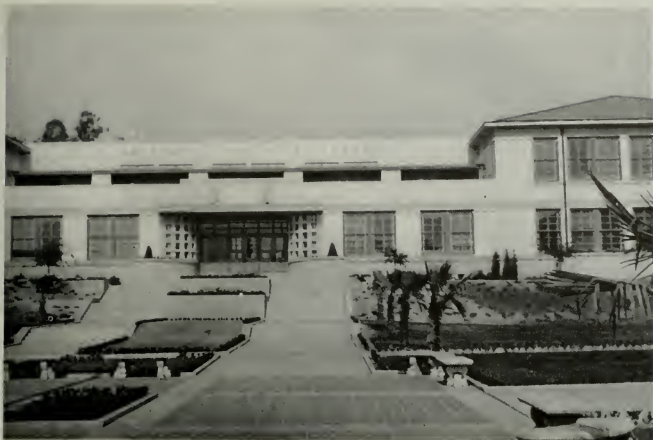
ABRAHAM LINCOLN HIGH SCHOOL, LOS ANGELES, CALIFORNIA Albert C. Martin, Architect
