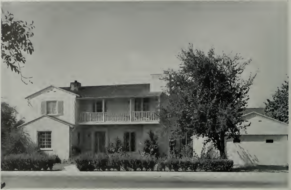
HOUSE FOR MR. AND MRS. LEONARD A. TALBOT, SANTA ROSA, CALIFORNIA C. A. Caulkins, Jr., A.J.A., Architect
