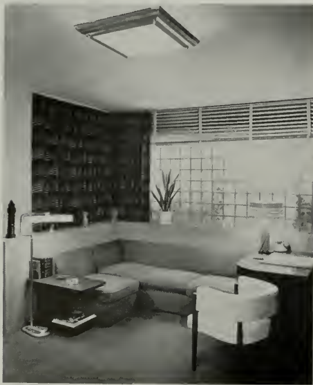
Fig. 5—Fluorescent lamps are incorporated in the modern design of the ceiling fixture and bridge lamp.
