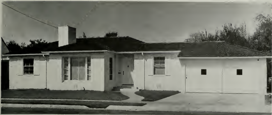
HOUSE FOR MR. AND MRS. J. C. BLACKMAN, SANTA ROSA, CALIFORNIA C. A. Caulkins, Jr., A.I.A., Architect
