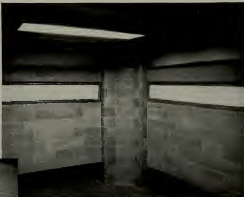
Corner of lunchroom (with glass blocks “blacked out”) shows interesting architectural details possible with Krafftile. Here, 2” thick furring tile is used on interior of the outside walls
