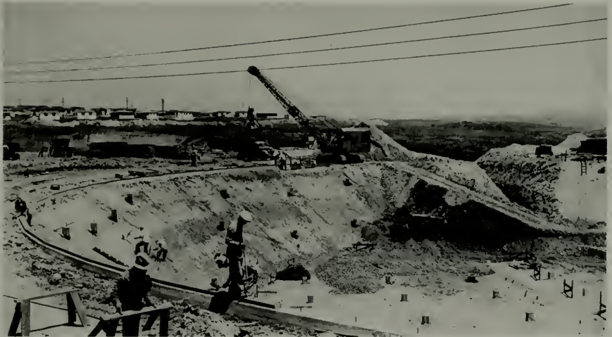
Progress picture of 5,000,000 gallon reservoir for water supply
