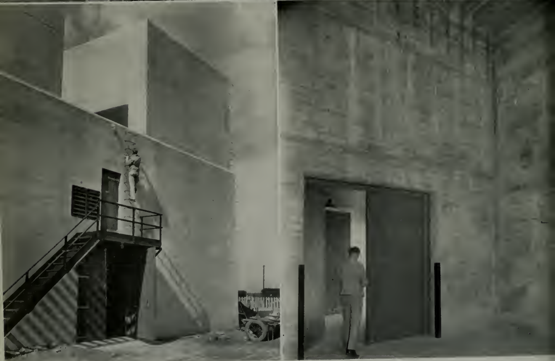
(Top) Exterior view of test stand building. Inlet stacks for the four test cells are on the corners of the structure; outlet stacks in the center each serve two test cells. (Above—left) Exterior view of inlet stacks. (Above—right) Interior view of test cell, showing height from the cell floor that sound-absorbing baffles of Fiberglas pads are installed in an inlet stack.
