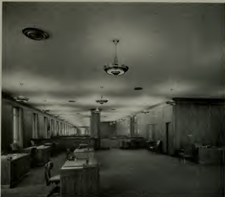
EXECUTIVES' FLOOR, BANK OF AMERICA BUILDING, SAN FRANCISCO
