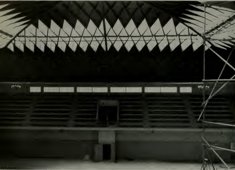
Interior of Union High School Gymnasium, Phoenix, Arizona, showing Lamella type of roof construction.
