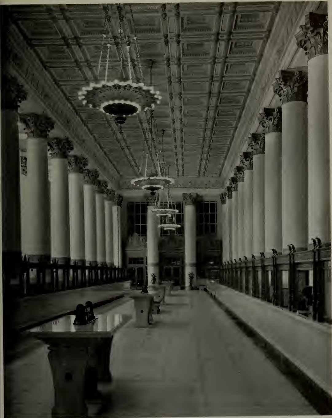
VIEW OF MAIN BANKING ROOM FROM MONTGOMERY STREET ENTRANCE LOBBY
