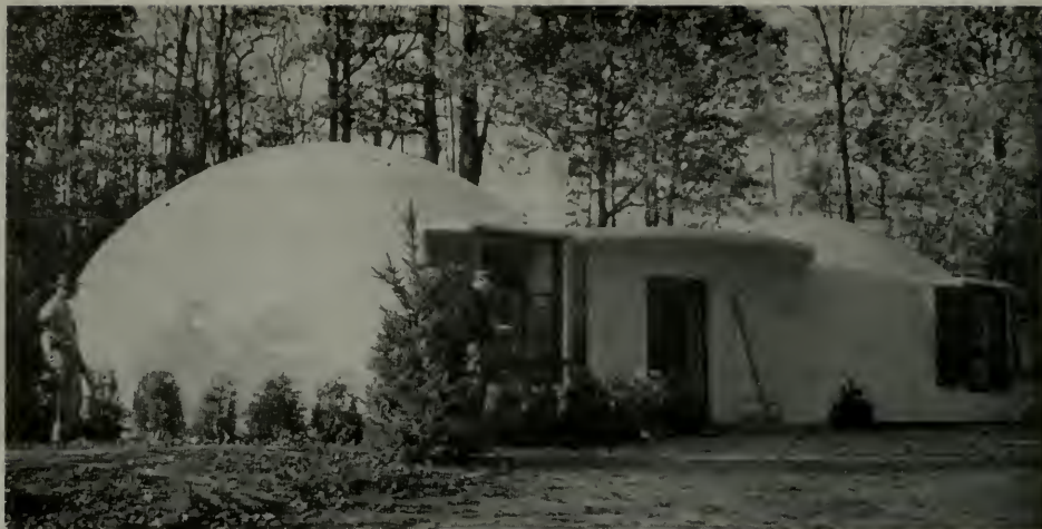
National Defense Homes Corporation of which Jesse Jones is head, is experimenting with this novel type of home at Falls Church, Va., from a patent applied-for design by Wallace Neff, architect, of Los Angeles.
