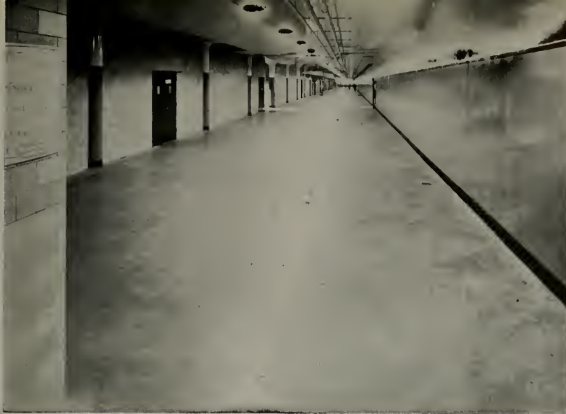
CURTISS-WRIGHT CORPORATION, AIRPLANE DIVISION, BUFFALO, N. Y. Corridor in basement of factory with doors to cafeteria, locker rooms, toilet rooms and stairs.
