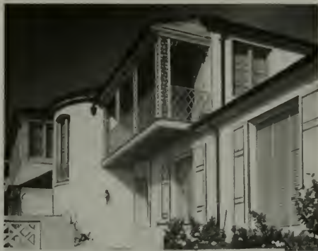
Balcony Detail, Residence of Felix Kahn, Seacliff, San Francisco Farr & Ward, Architects
