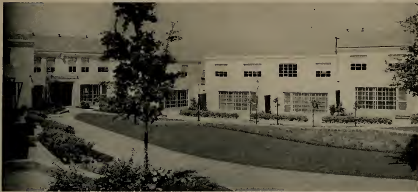
Garden view, row of community apartment houses, Parkmerced, San Francisco
