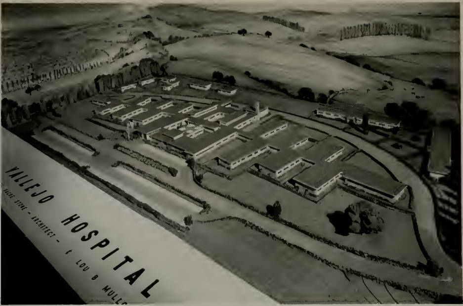
MODEL OF VALLEJO COMMUNITY HOSPITAL, VALLEJO, CALIFORNIA Douglas Dace Stone, Architect, and Lou B. Mulloy; Barrett & Hilp, Builders. Hospital has a normal capacity of 250 beds with provision for an additional 100 emergency beds. All buildings are wood frame and semi-permanent construction.
