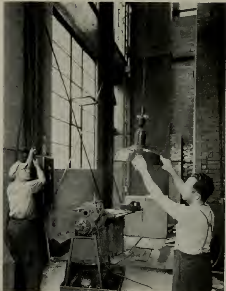
Lowering a luminaire to the floor where it may be cleaned more conveniently is quickly accomplished with the aid of an automatic disconnecting hanger in this high bay area.
