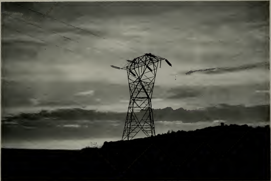
TRANSMISSION TOWER, NEAR PORTLAND, OREGON
