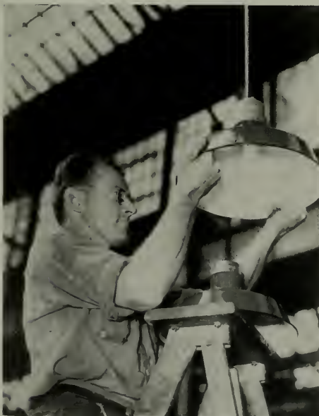
Removable reflectors make it possible for the maintenance man to remove a dirty reflector and replace it with a clean one that is carried as an extra.
