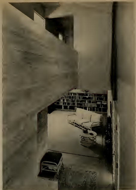
FLUSH FIR SIDING ON STAIR AND BALCONY RAIL IN TWO-STORY HALLWAY
