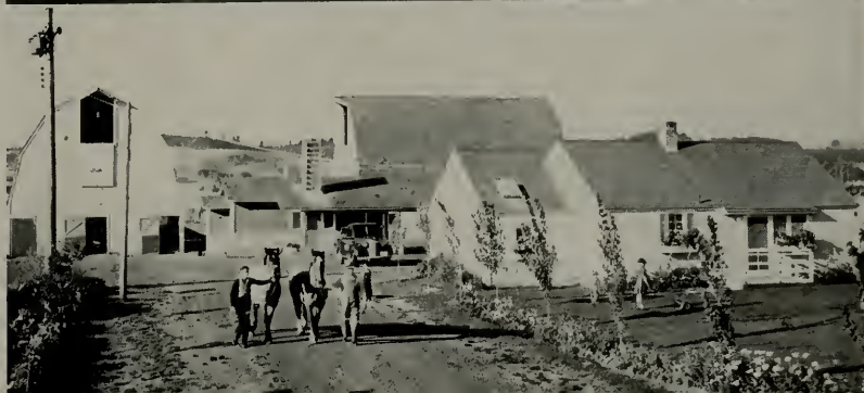
Below: A typical farm unit showing rural use of electric energy.
