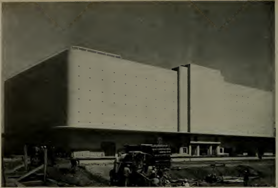
The warehouse, 140 feet by 260 feet, was designed for a fifth story.
