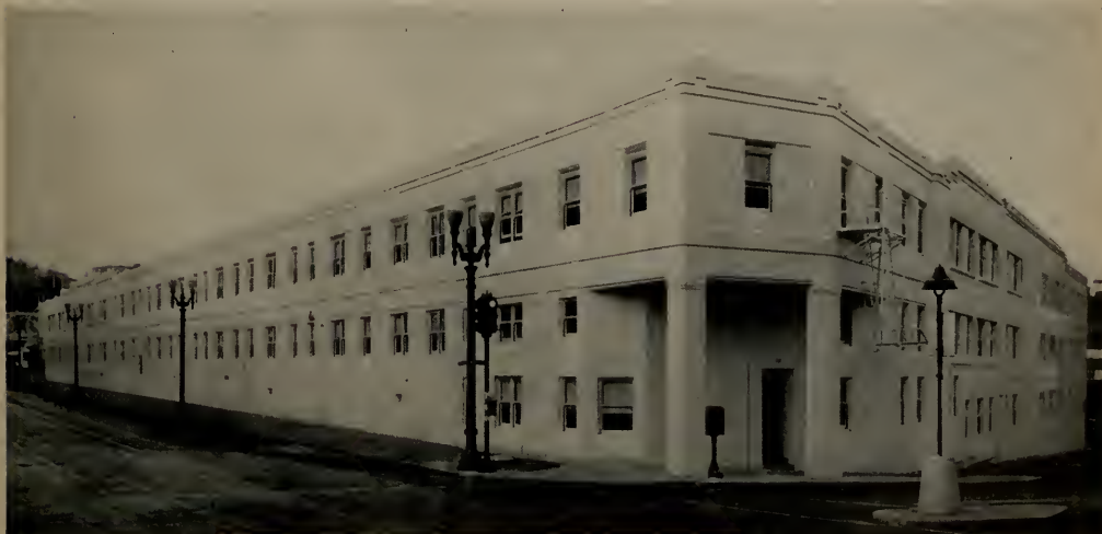
EXTERIOR VIEW OF COMPLETED STADIUM COURT APARTMENTS
