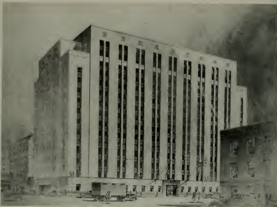
PRELIMINARY STUDY, U. S. APPRAISERS STORES BUILDING, SAN FRANCISCO The three story building in the right foreground recently collapsed under its own weight. The structure was loaded down with merchandise.
