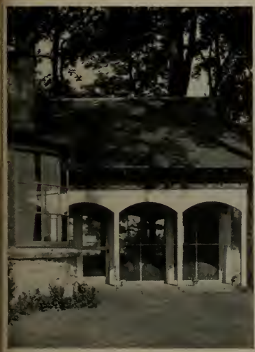
The loggia gives protected cover from garage to house and also serves to relieve the stark appearance characteristic of screened porches
