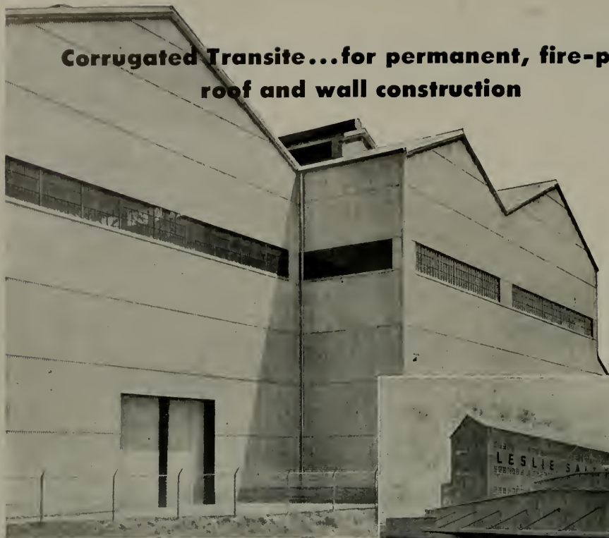
Installation by Western Asbestos Co. of Corrugated Transite for the American Forge Company, Berkeley, California
