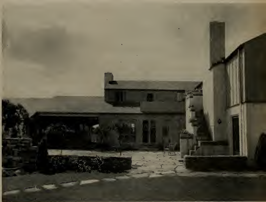
HOME AND STUDIO FOR ROY MASON, BATAVIA, N. Y. The stair winding around the chimney encourages relaxation from painting, in the large patio. Mr. Mason, noted artist, says: "It makes it a cinch to sneak the models out, when I hear my wife coming!"
