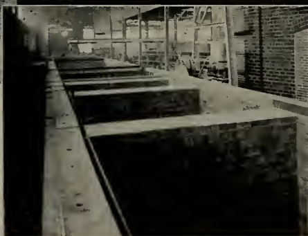
Showing how to construct a tank of Krafftile brick and Nukem jointing compound so as to resist high concentrations of almost any acid and withstand hard usage year after year.
