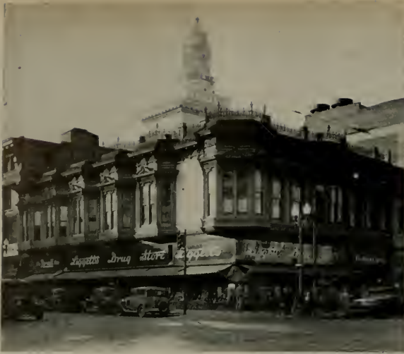
Modernization of the Delger Building called for the removal of bay windows, unadorned roof line and new exterior without making alterations of the structural elements.
