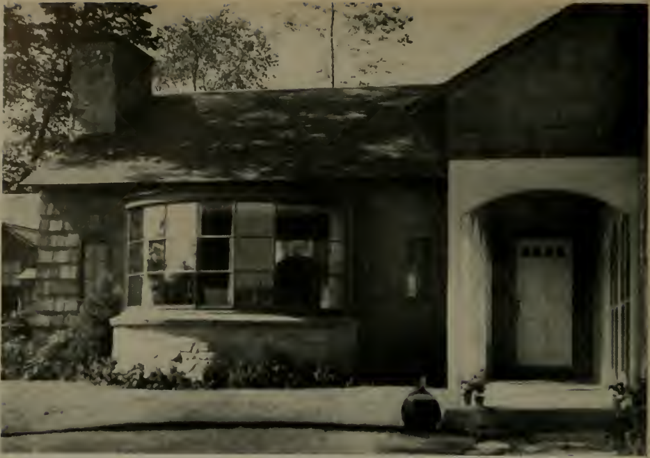
The large squares of "Thermapane" obviate any need for storm sash; they keep heat out in summer and retain it in cold weather. Roof is cantilevered to ease load on sash
