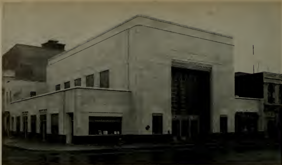
U. S. NATIONAL BANK OF PORTLAND—KLAMATH FALLS, OREGON BRANCH With Anchored Type Ceramic Veneer Material Sutton, Whitney & Aandahl, Architects
