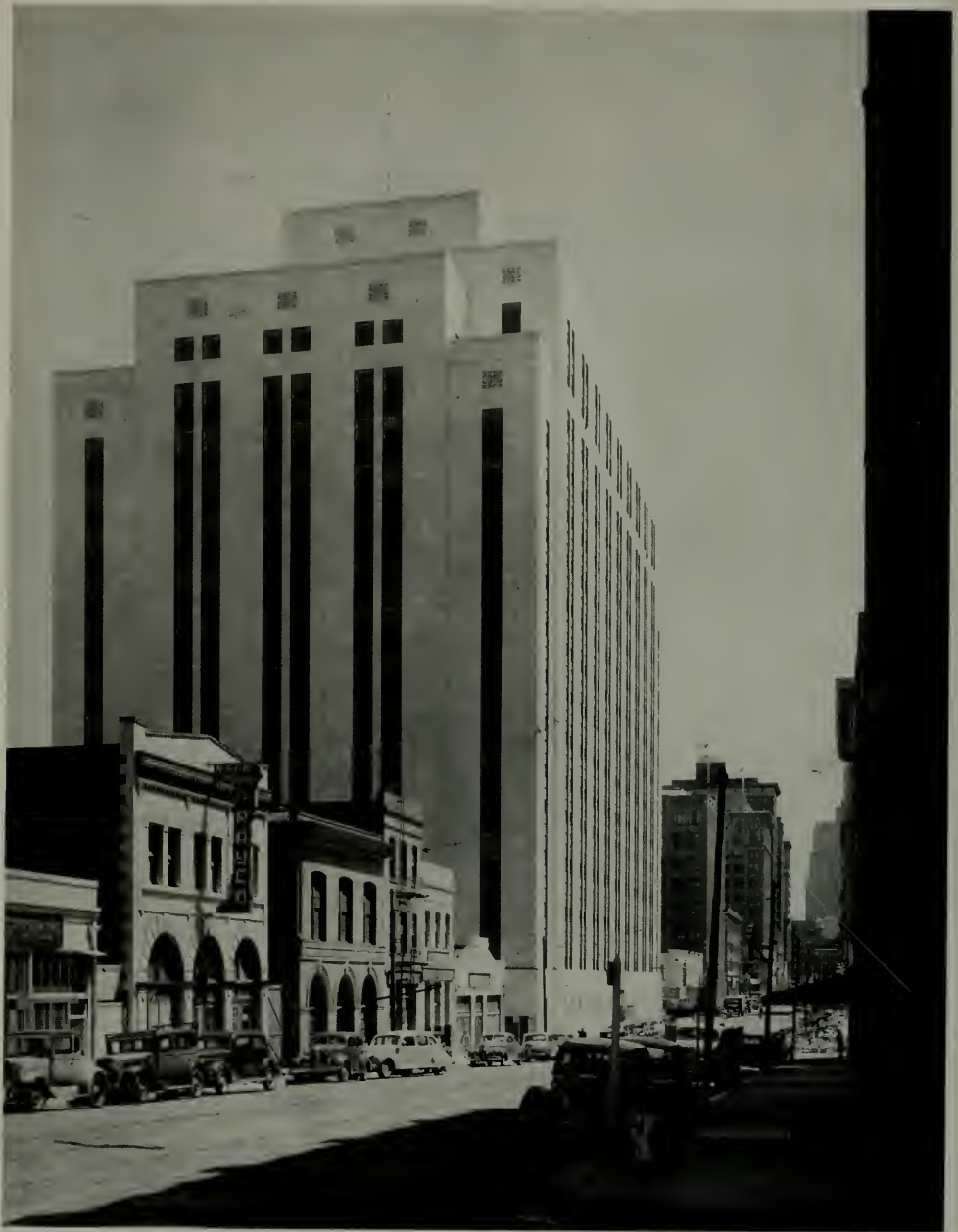
UNITED STATES APPRAISERS STORES BUILDING, SAN FRANCISCO W. E. REYNOLDS, LOUIS SIMON, GILBERT STANLEY UNDERWOOD
