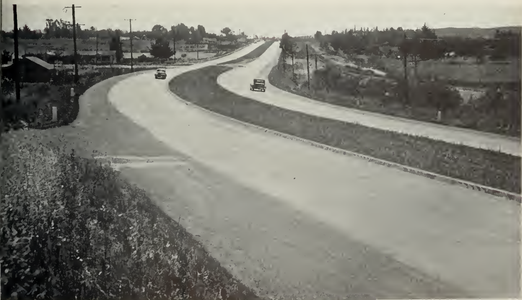
MONTEREY-CASTROVILLE-PRUNEDALE project provides highway as shown looking southerly toward Marina on 4-lane, divided Portland cement concrete pavement. Road to left is Monterey Avenue to Salinas via East Garrison of Fort Ord. (Photo courtesy Calif. Highways & Public Works.)
