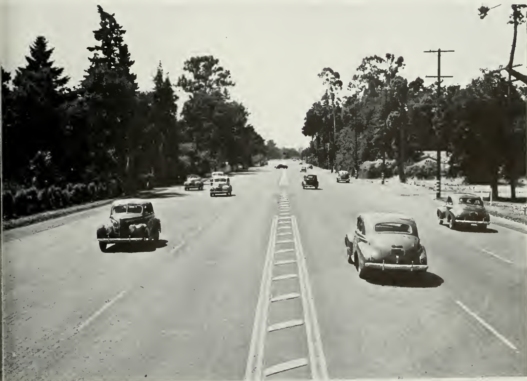
View of widened section of U. S. 101 near Atherton providing a 6-lane divided highway.
