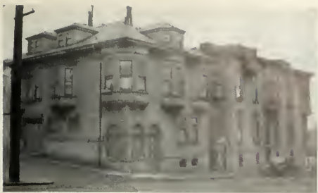
Prior to conversion . . . old, outdated.
