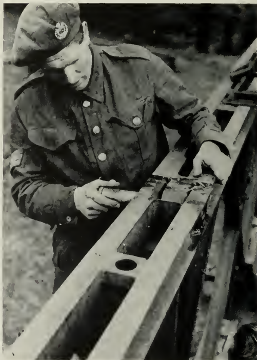
One man joins two panels with one 2-inch high-tensile steel pin.
