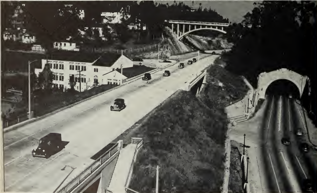
Top: Southbound traffic approaching Los Angeles on Arroyo Seco Extension and through open cut in Elysian Park—old road at left. (Note famed City Hall in background.) Bottom: Southbound traffic passing under Park Row Bridge and northbound traffic entering park tunnel. (Photo courtesy Calif. Highways & Public Works.)
