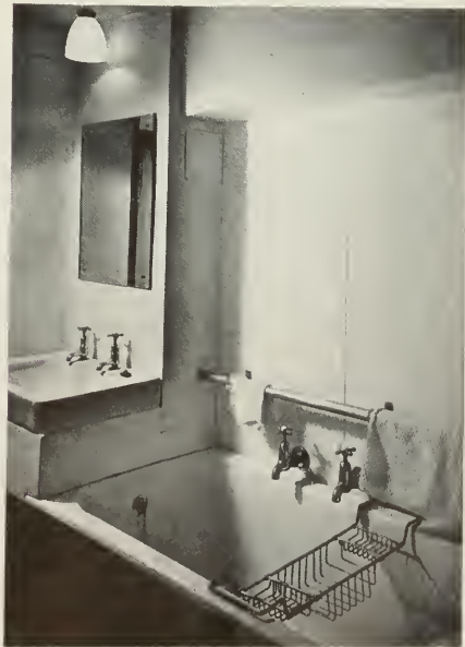
Basin, wash, towel rail and mirror are fitted in steel wall.
