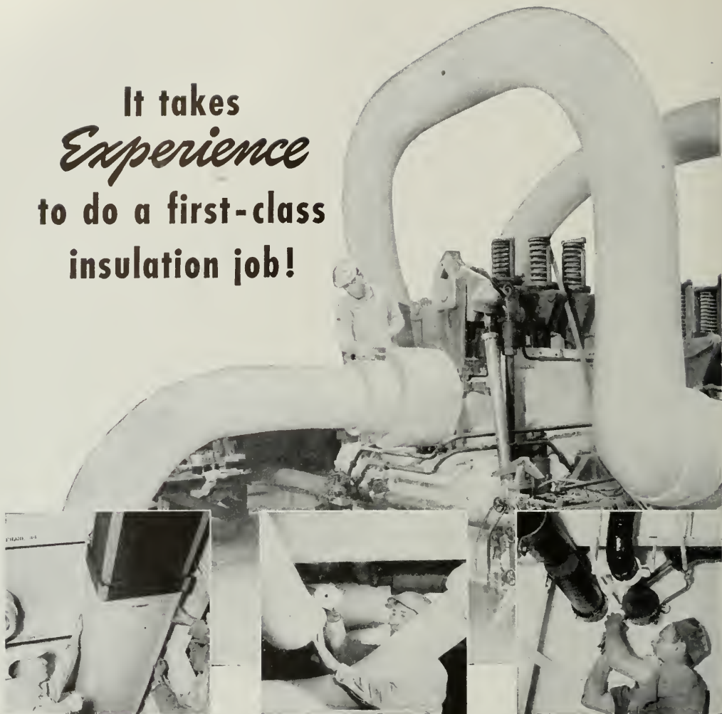
Sewing canvas over Johns-Manville BX18 insulation on a ventilating duct
