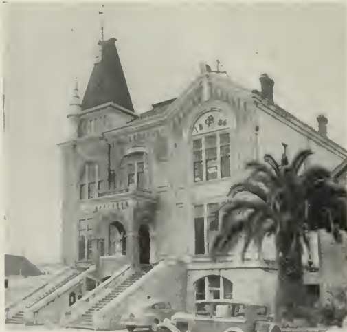
OLD CITY HALL of Petaluma, California, which is to be replaced with ultra modern building in post-war building program of city.
