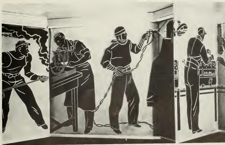
THE FIGURES in this Carrara structural glass mural stand out a quarter of an inch from a sandblasted background, although they appear to be sculptured in bas-relief.
