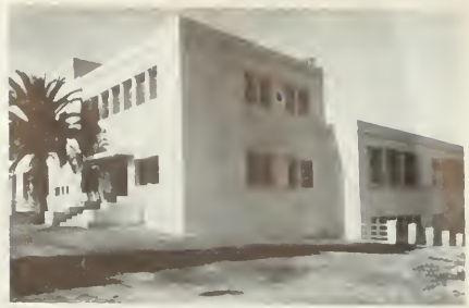
Concrete and hollow tile constructed Girls' School at Maison Carree, Algeria. Eduard Lowe, Architect
