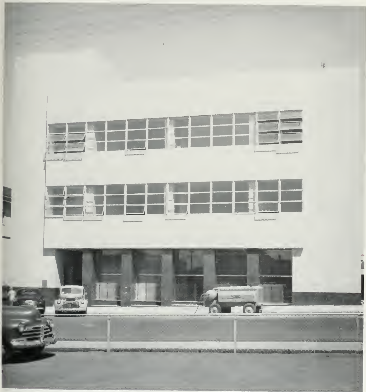
NEW BUILDING OF THE PACIFIC TELEPHONE & TELEGRAPH COMPANY—Berkeley, California MONSON BROTHERS—General Contractors
