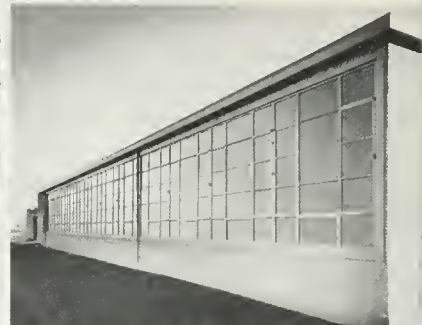
Sylvan School, Modesto Fred L. Schwartz & Wm. G. Hyberg, Architects
