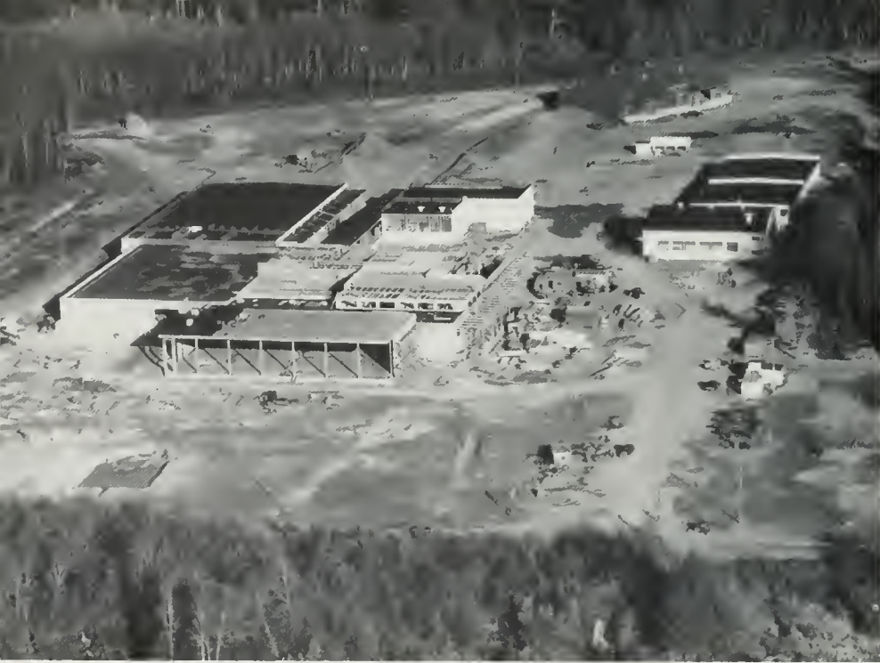
AERIAL VIEW OF THE NEW TILLAMOOK COUNTY CREAMERY ASSOCIATION PLANT
