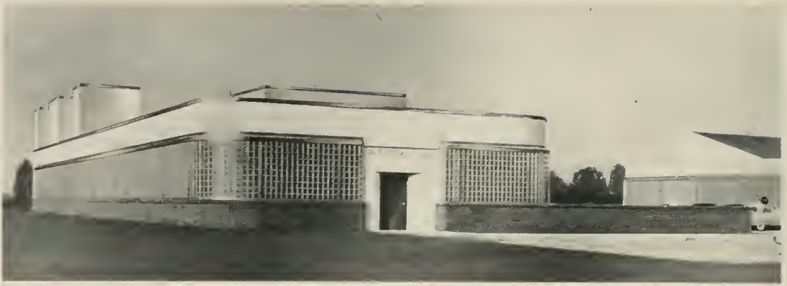
NEW Ultra Modern Research Laboratory Building — Los Angeles.
