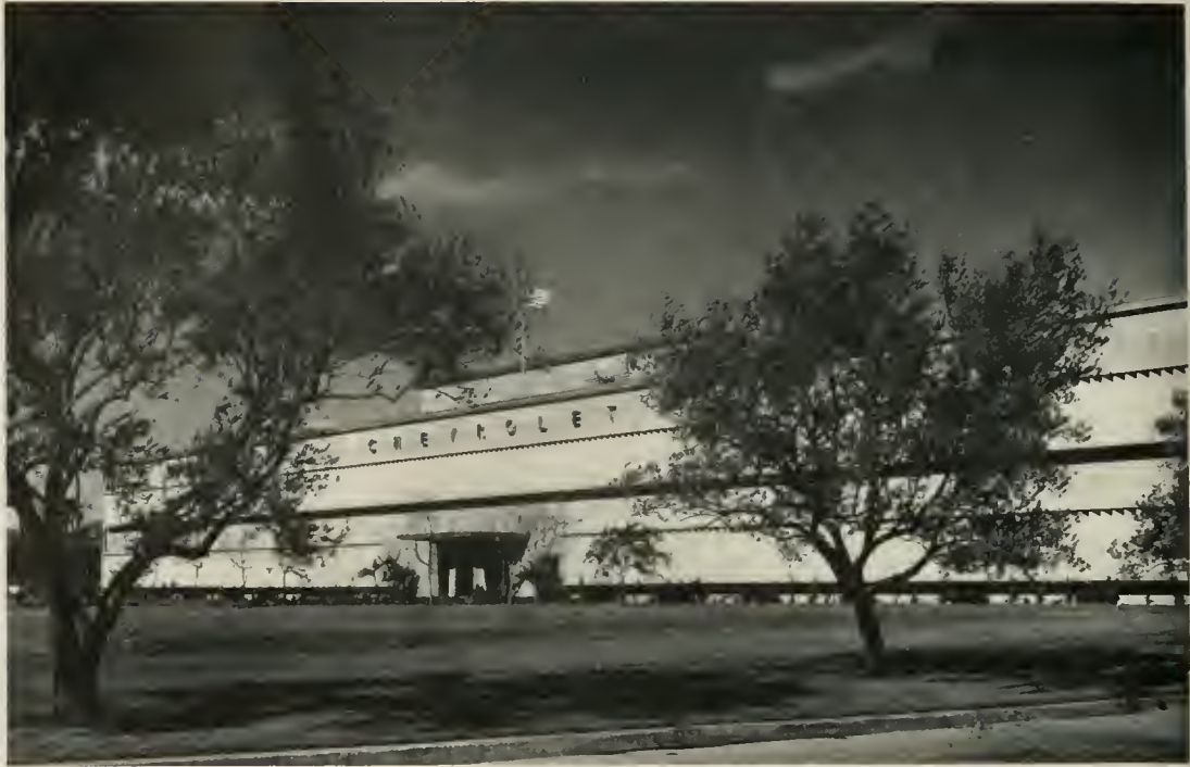
NEW CHEVROLET ASSEMBLY PLANT IN SOUTHERN CALIFORNIA.
