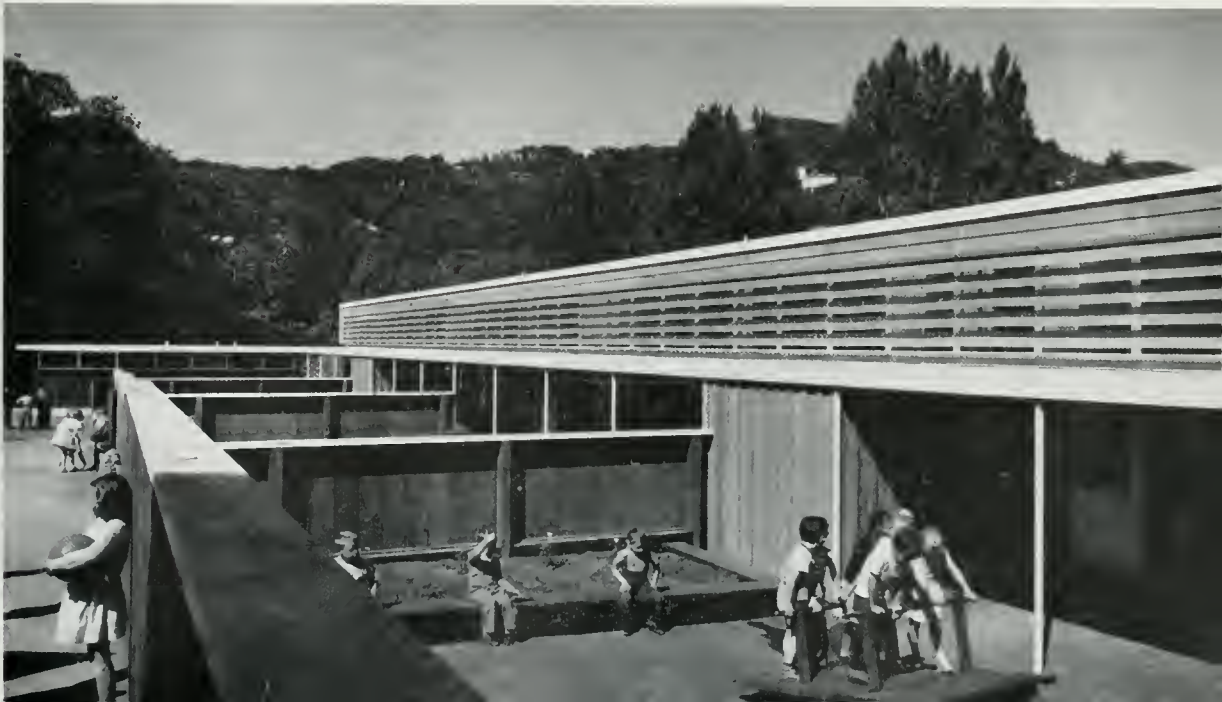
Exterior view showing installation of aluminum lighting louvers
