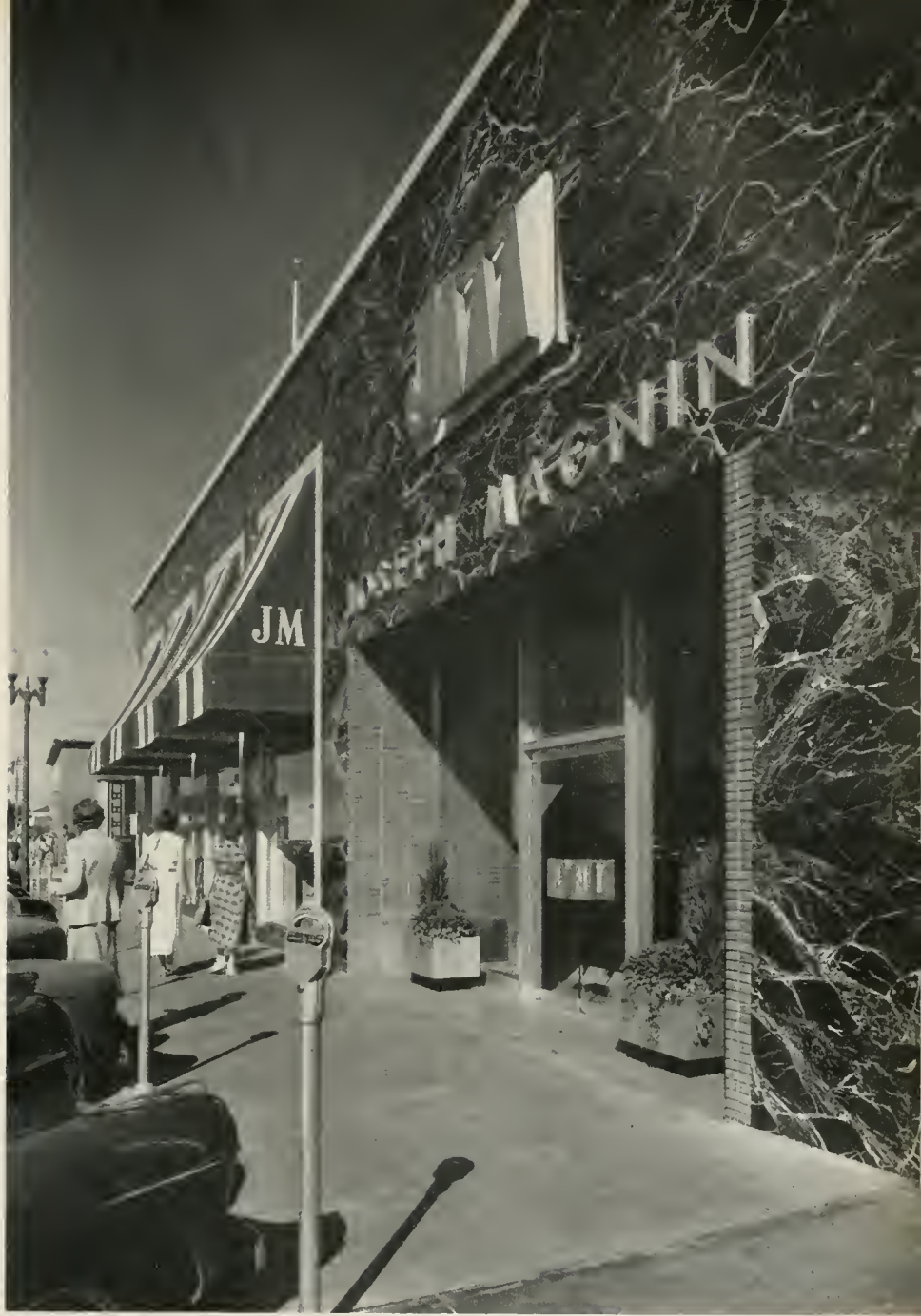
RICHNESS of the green Verde antique morble and details of street entrance set character of the store. The initials above the entry are back lighted for evening and night effect.
