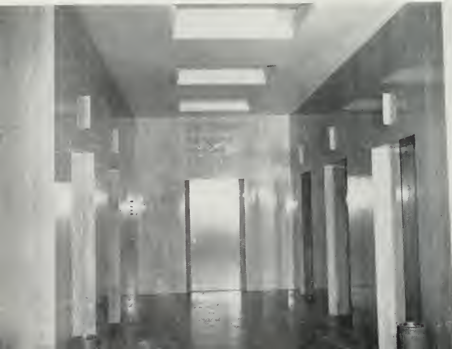
MARBLE WALLS of the main lobby entrance is indicative of marble installations throughout the 22-story annex. Elevator entrances to all floors at right and left. Indirect lighting is used and marble is used for the floor.
