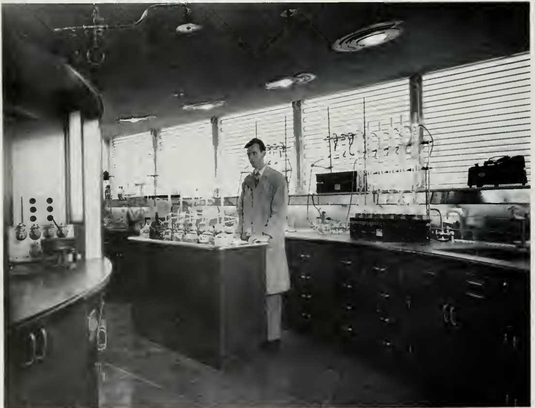
VIEW of Tower Laboratory interior showing corner of one of main floors—horizontal glass tubing making up the outer wall admits a maximum of light for work areas. Alternating with each of the square floors (as shown) are circular ones which do not extend to the outer walls of the building. The curved underside of the mezzanine-like floor above forms the ceiling (shown here) as a curving, graceful contour.
