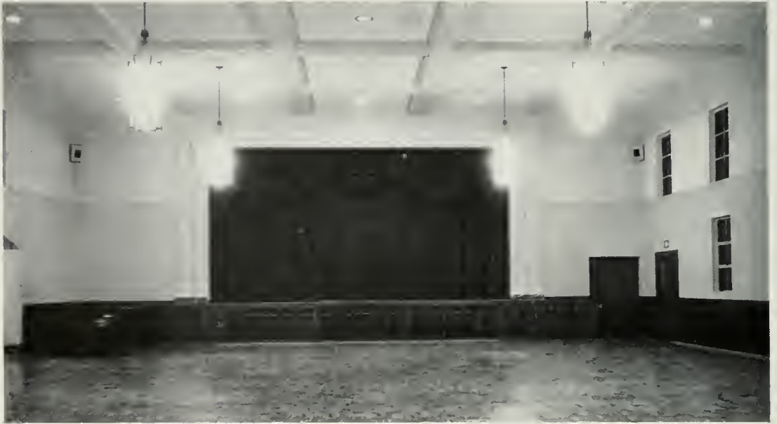
ABOVE: The spacious Recreation Hall looking towards the stage—overhead panel design permits dual lighting effects; public address system speakers are located in corners of hall near ceiling; asphalt tile floor cover.
