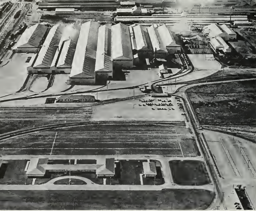
Aerial View of Entire Plant
