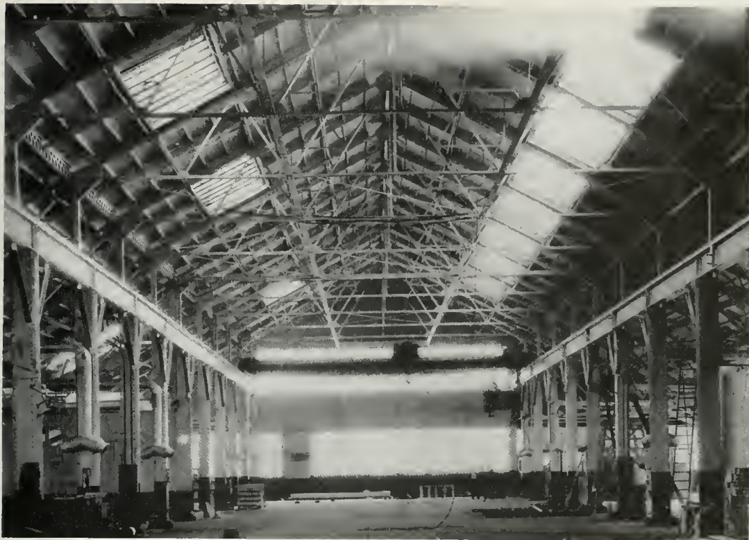
EXPOSURE TO DAMAGE BY RUST IS RIFE IN SUCH A BUILDING AS THIS
