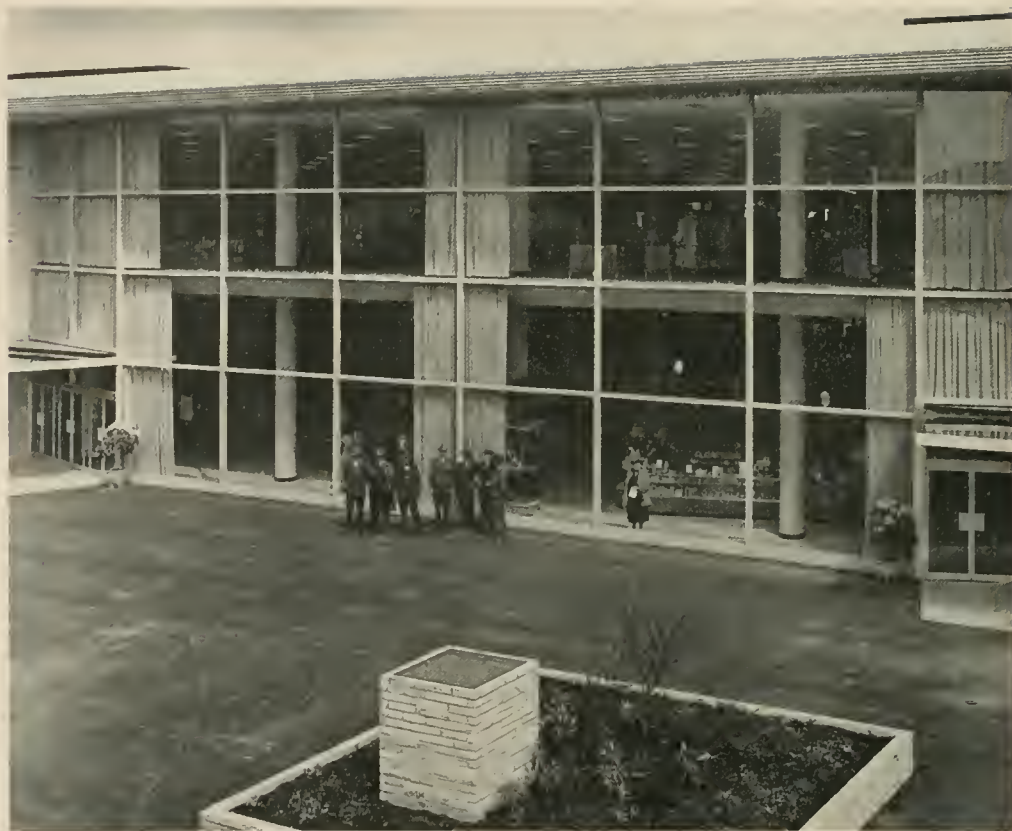
A DAYLIGHT view of the Bon Marche store entrance as seen from NORTHGATE Miracle Mall, with ventilators from underground truck passageway in the foreground landscaped for harmony with surrounding area . . . aluminum, stone and glass combine for striking front elevation of this remarkable department store.
