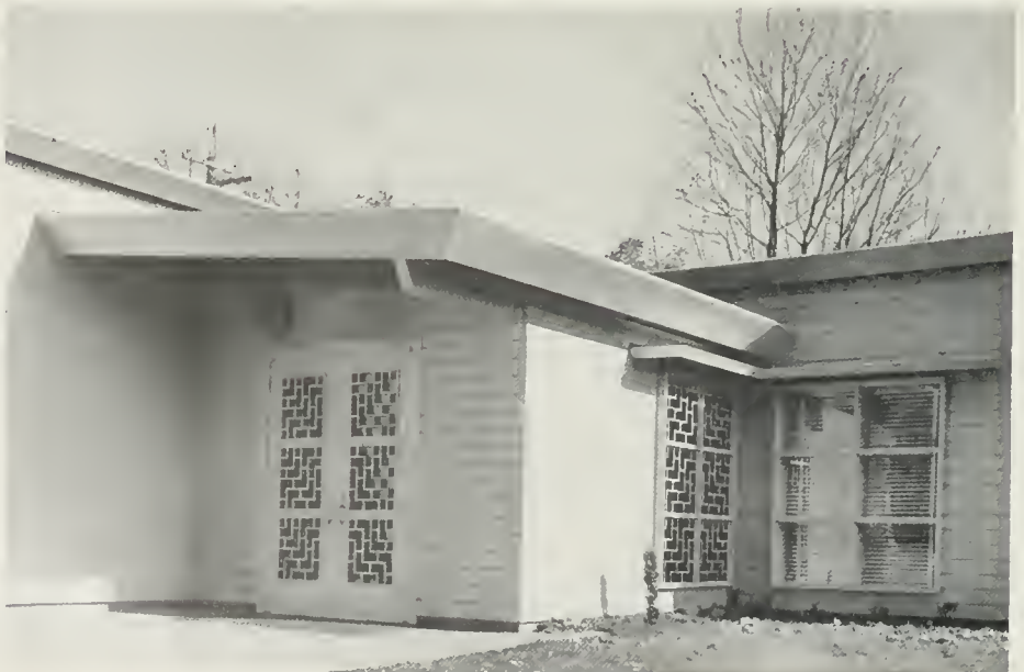
CLOSE-UP of main entrance showing detail of door and windows.
