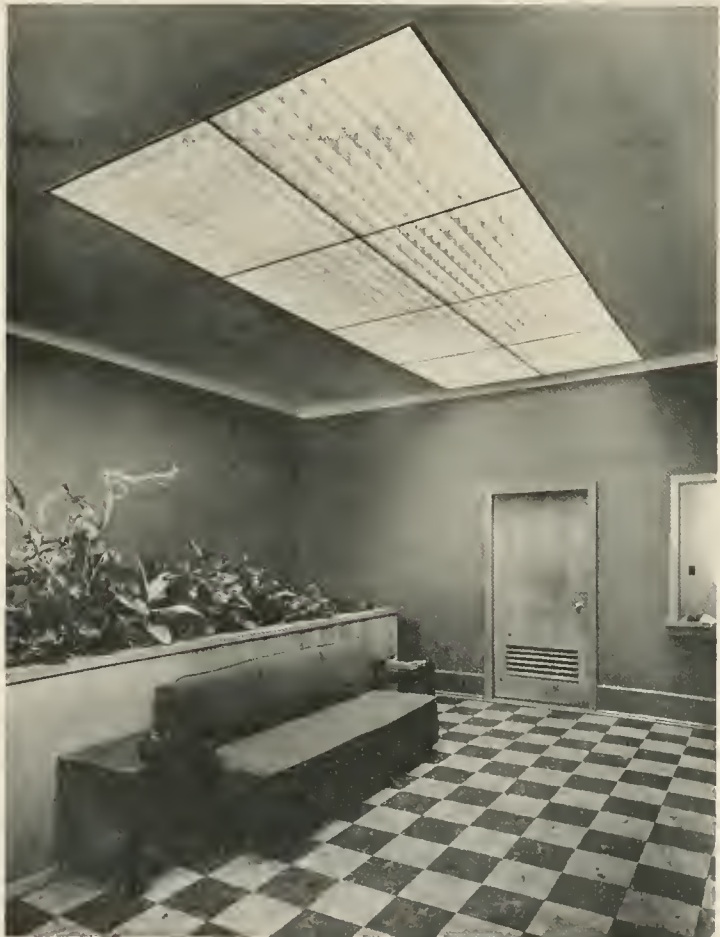
AFTER —The entire skylight area is hidden behind panel of aluminum louvered grid section set flush with ceiling. Satin finish aluminum distributes light evenly, eliminating shadows and glare.
