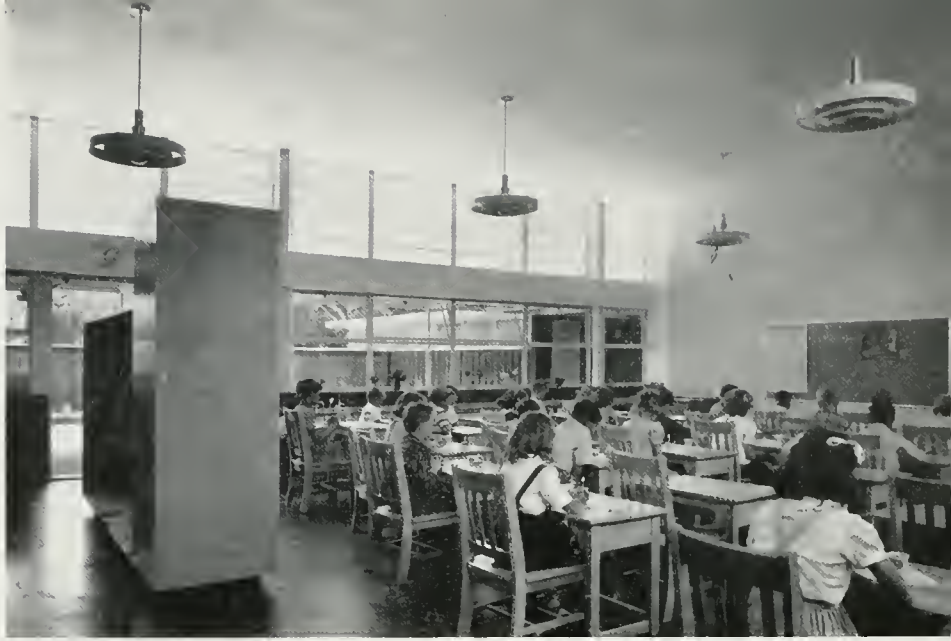
Typical schoolroom installation
