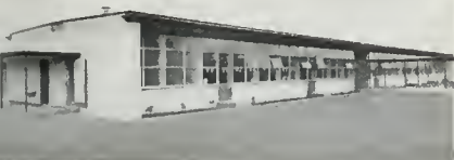
Mayfair School, Fresno Franklin & Simpson, Architects
