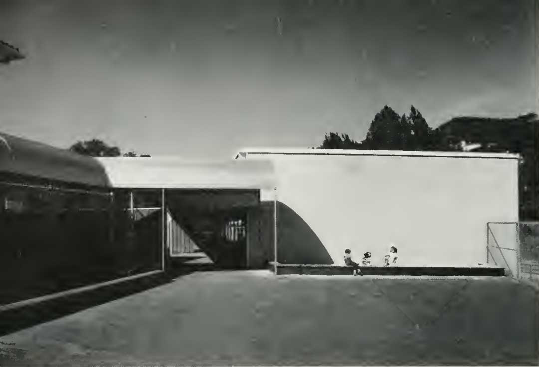
Attractive aluminum canopy connects new wing with old building.
