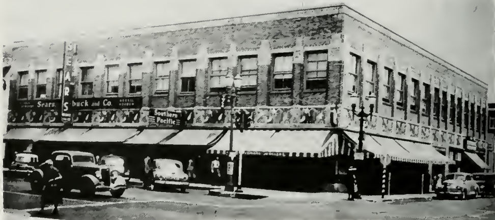
Corner Location BEFORE Start of Remodel
