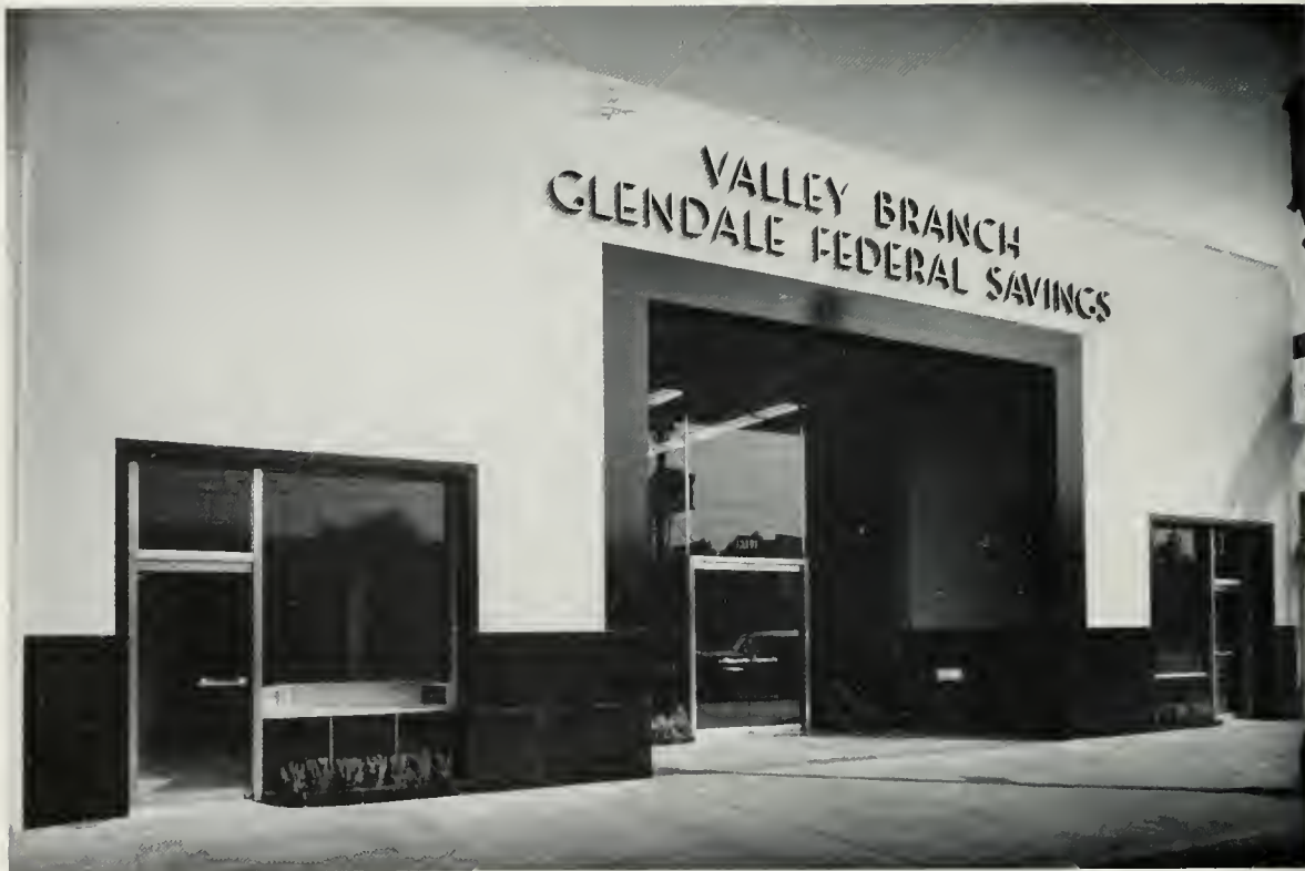
MAIN or South Facade on Ventura Boulevard
