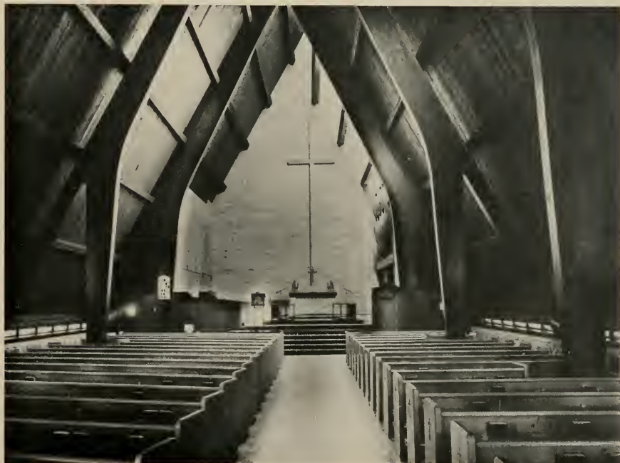
BELOW: Striking traditional design of Salem Lutheran Church at West St. Paul, Minnesota, by Architects Magney, Tussler and Setter, shows simplicity.
