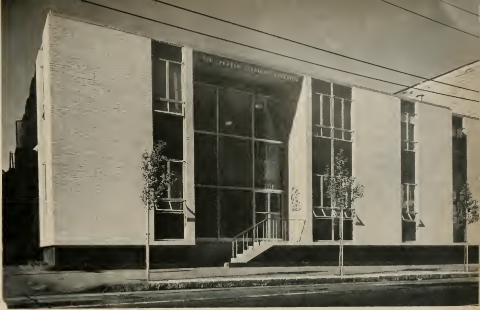
2320 SUTTER MEDICAL BUILDING . . . San Francisco
