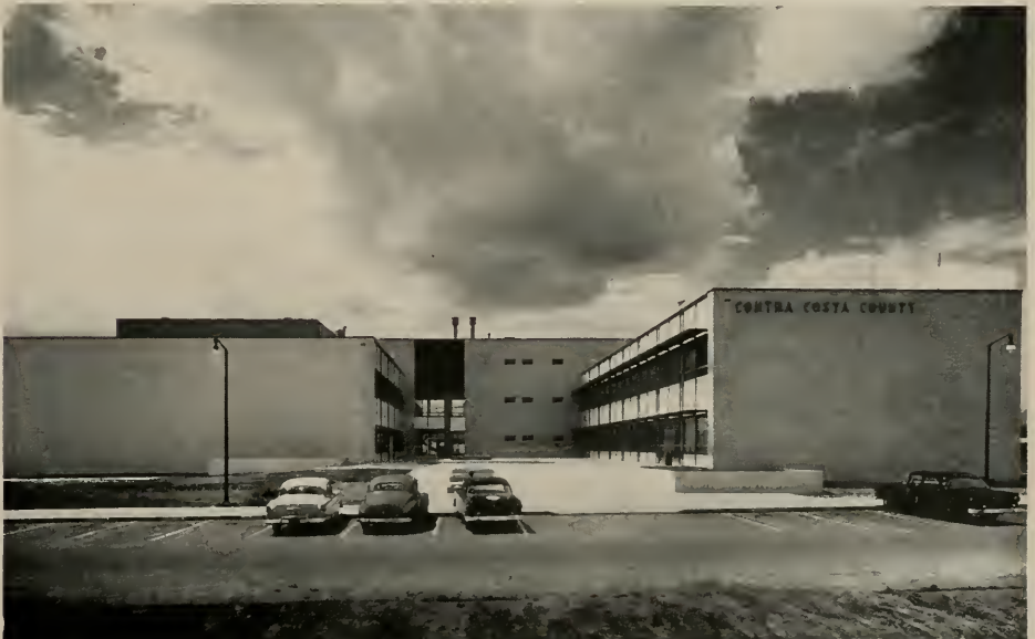
REAR PATIO COURT Elevation from parking lot. Richmond Buff brick walls, except concrete for future expansion. The patio and building area has been thoroughly landscaped.
