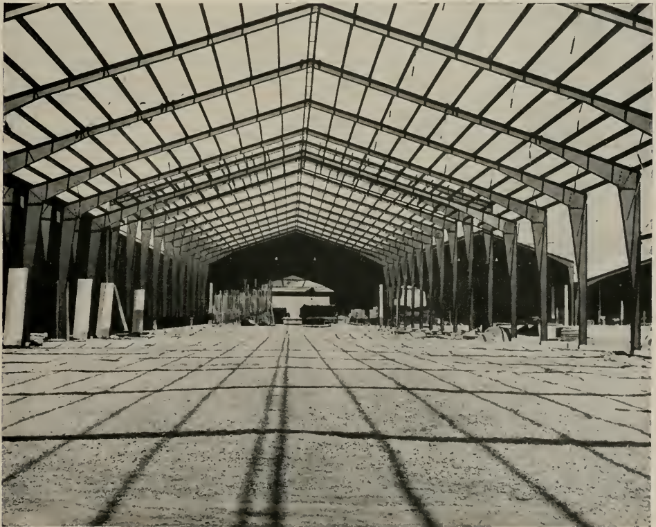
Placing steel bents
