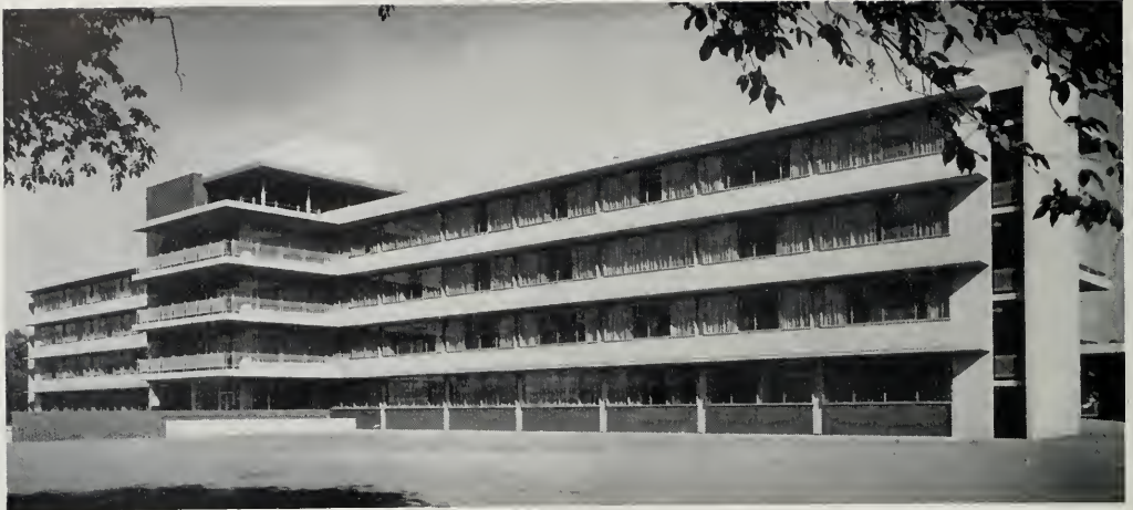
Fresno County Tuberculosis Hospital, Fresno, California. David H. Horn, A.I.A., Marshall D. Mortland, A.I.A., Associate Architects General Contractor: Midstate Construction Co. & Stolte, Inc., a joint venture
