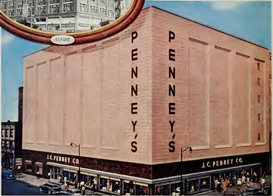
J. C. Penney Store Building, Spokane, Washington • Architects: Whitehouse & Price • Contractor & Structural Engineer: Walter G. Meyers & Son
