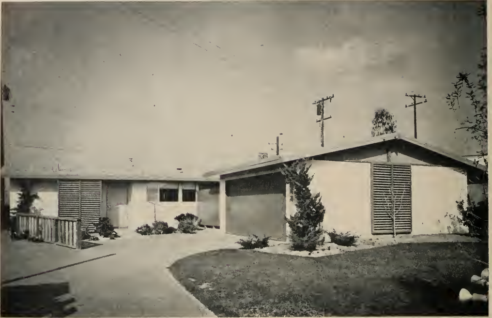
THE "TOWN and COUNTRY" HOME, designed by Architects Palmer and Krisel, AIA, for the Larwin Company, builders, Buena Park, California, and 1957 Design Merit Award Winner of the NAHB.
