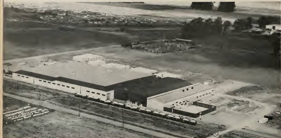
AERIAL VIEW of plants built for American Forest Products Corp'n at Newark, California. Corrugator plant at extreme right; Paper Mill at left. Designed by Raymond E. Layton & Associates.
