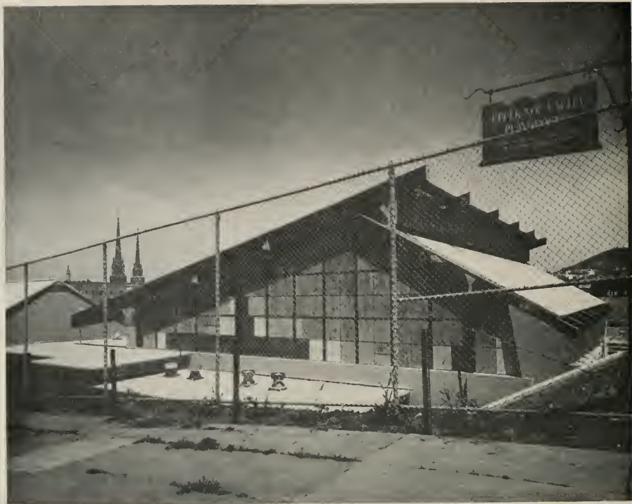
Profile showing dramatic lines of roof.
