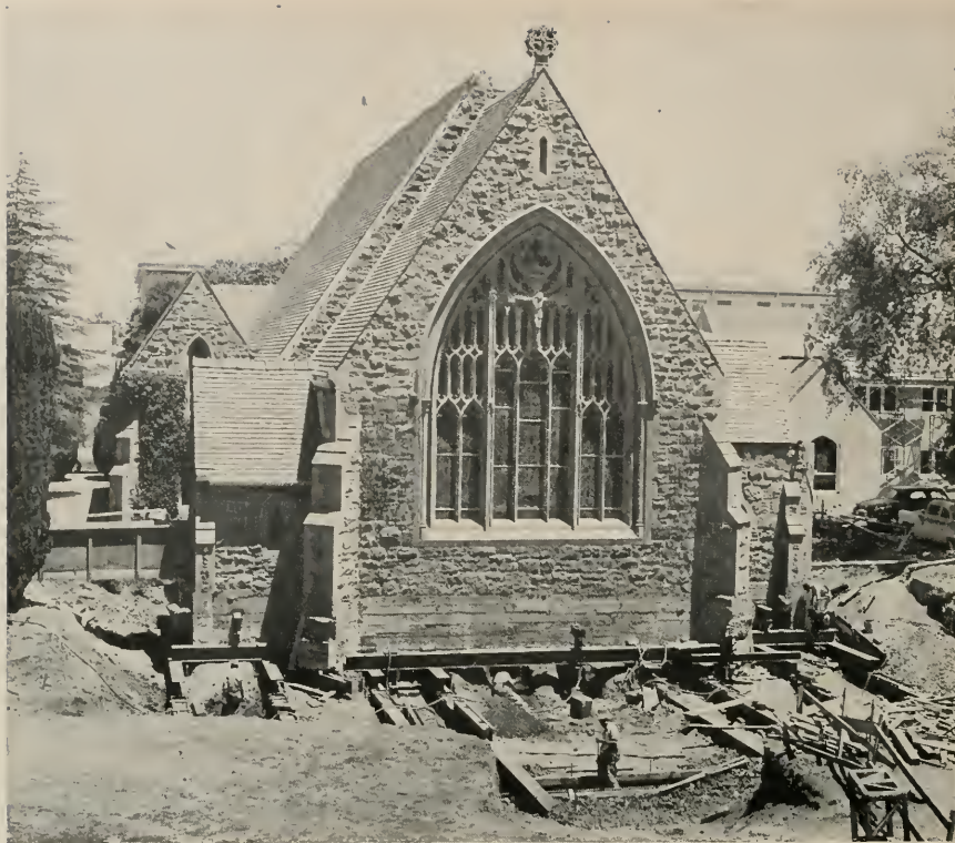
EPISCOPAL CHURCH OF ST. MATTHEW—front portion moved 30 feet.
