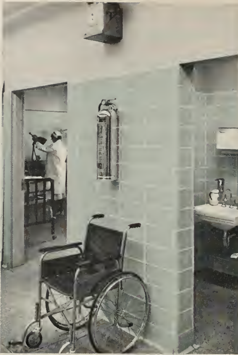
Ford Motor Company, Milpitas, California Architect: Albert Kahn, Associated Architects & Engineers Glazed structural tile by Kraftile
