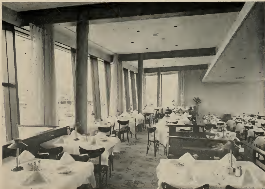
BELOW: Steel beams spanning 40 ft. of open space permit unlimited view for patrons seated in three-tier levels.
