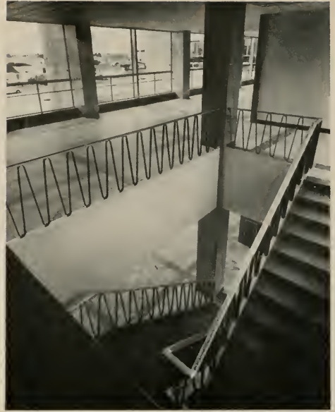
MAIN STAIR from 1st to 2nd floor is of steel with aluminum rail, with Red Verona Marble treads and risers. The lobby floor is of Verona in a field of white Columbia Marble.
