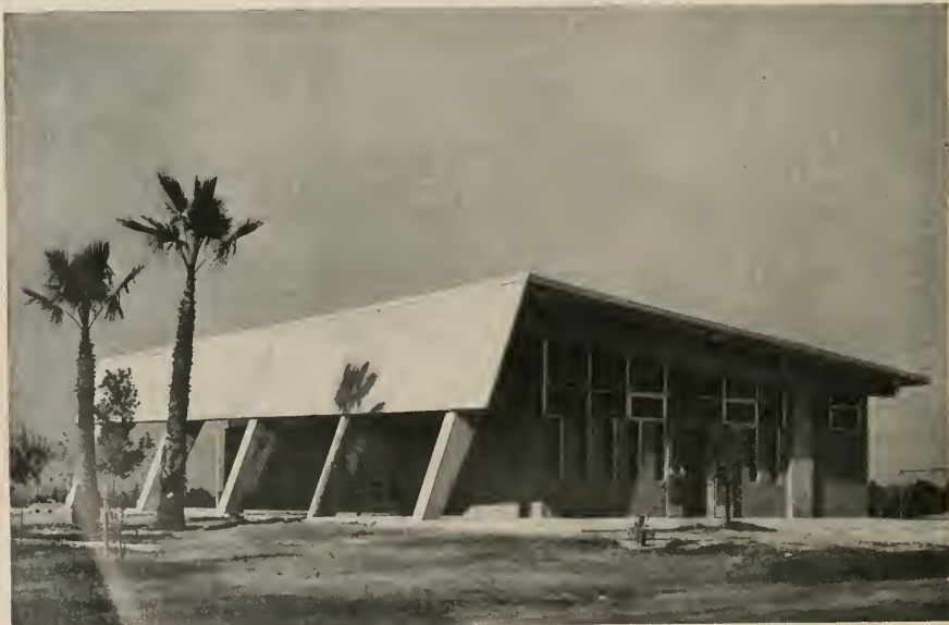
Reinforced concrete BENTS, poured on the ground, were hoisted into place; 40-ft. crane lifted 10-ton roof slabs of reinforced concrete into position; concrete-block walls then laid in place.
