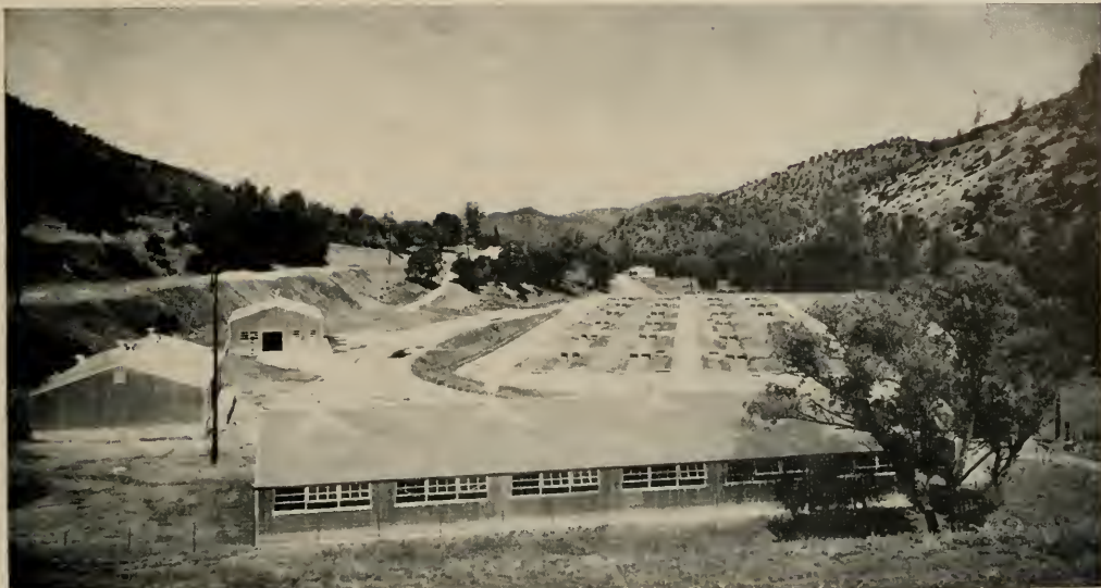
CALIFORNIA FISH & GAME —Development of the state's natural resources is shown in this large Fish Hatchery built on Mac-casin Creek, Tuolumne County, California. Work included site preparation, buildings and ponds.
