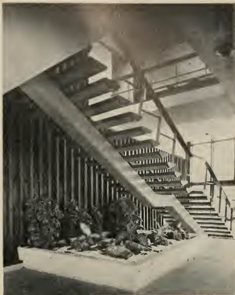
FLOATING STAIRWAY connects second floor dining area with glass enclosed foyer.
