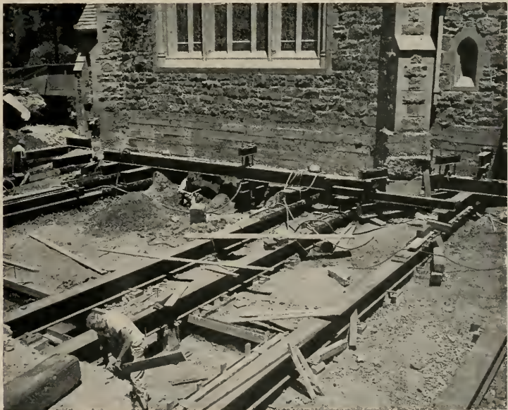
ABOVE: 400 tons of Church going for a ride at the rate of five feet per hour—for a distance of thirty feet.
