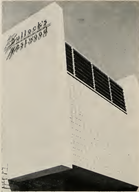
Enormous panel walls of decorative tile distinguish fashionable store—Bullock's Westwood.
