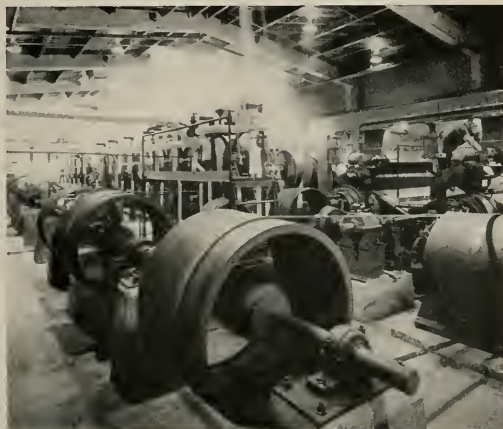
Photo shows Steam Piping and Drying Rolls, Line Shaft, Paper Mill, Newark, Calif.
