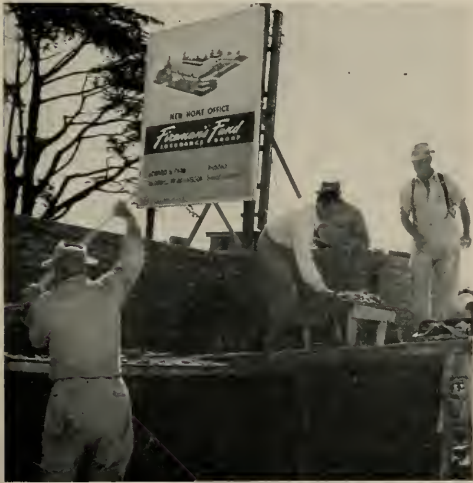
BRICK MASONS doing their part in constructing this modern building.
