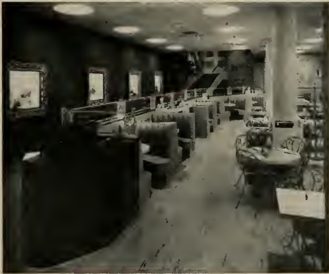
INTERIOR view of Blum's Geary Street store
