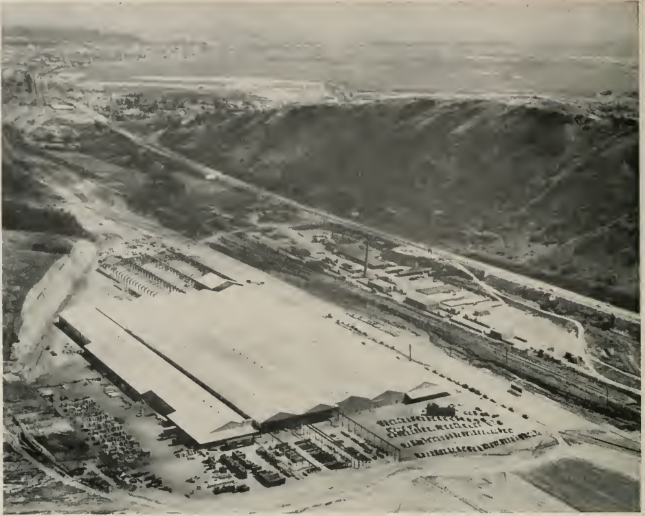
Aerial view looking south to San Diego—80% completed.
