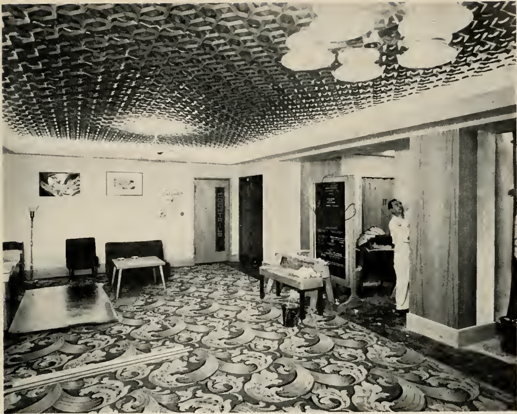
WORKMEN APPLYING FINAL TOUCHES TO REMODELING OF LOBBY
