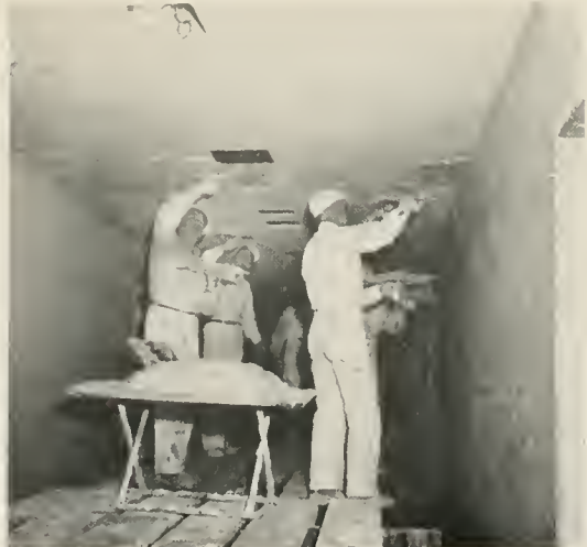
Steel stud erections on the 6th floor (left), and acoustic plaster being applied on the Main Corridor of the 5th Floor of the Peninsula Hospital.
