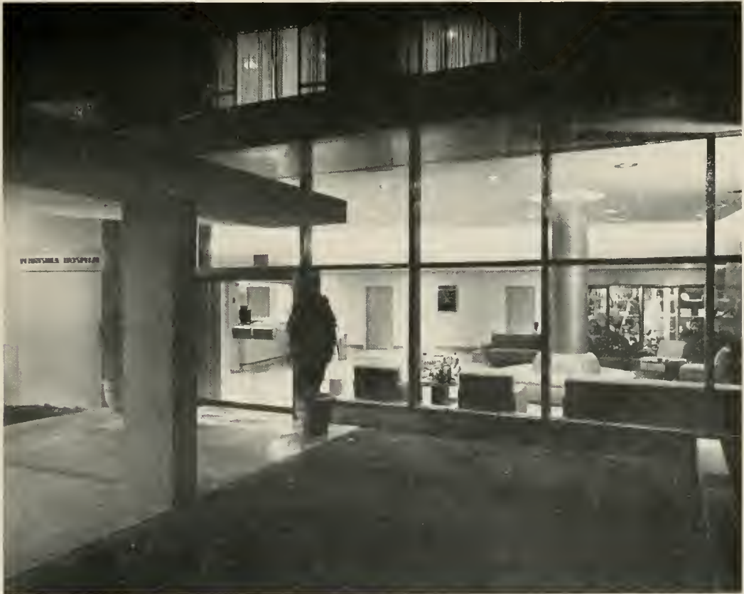
PENINSULA HOSPITAL, Burlingame, completes $4,000,000 expansion program. Original structure designed for addition of four new floors without disturbing occupants of building. (Photo courtesy Stone, Marraccini and Paterson, successors to Stone, Mulloy, Marraccini & Paterson, Architects. Smith & Moorehead, Structural Engineers.)
