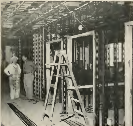
Steel stud erections on the 6th floor (left), and acoustic plaster being applied on the Main Corridor of the 5th Floor of the Peninsula Hospital.
