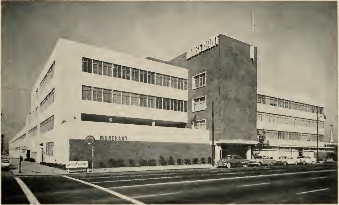
NEW PLANT of the Marchant Company, Oakland, California.
