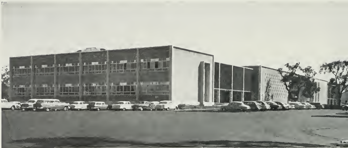
STANFORD RESEARCH INSTITUTE, Menlo Park Stanton & Stockwell, Architects
