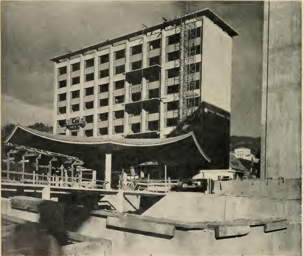
CONSTRUCTION PROGRESS VIEW of U.C. Residence Halls.
