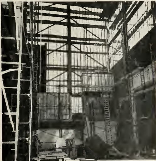
INTERIOR VIEW of light steel construction.
