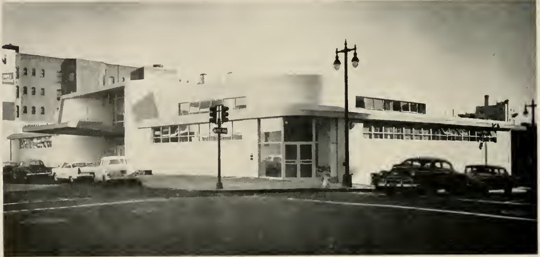
AIRLINE BUS TERMINAL
