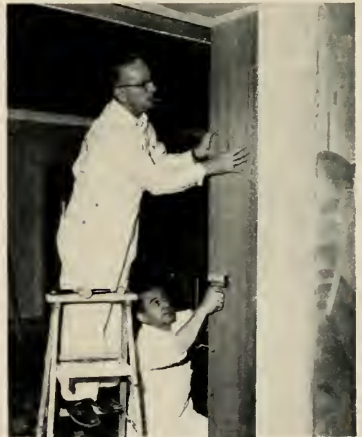
WORKMEN APPLY clear vinyl surfaced decorative panel.
