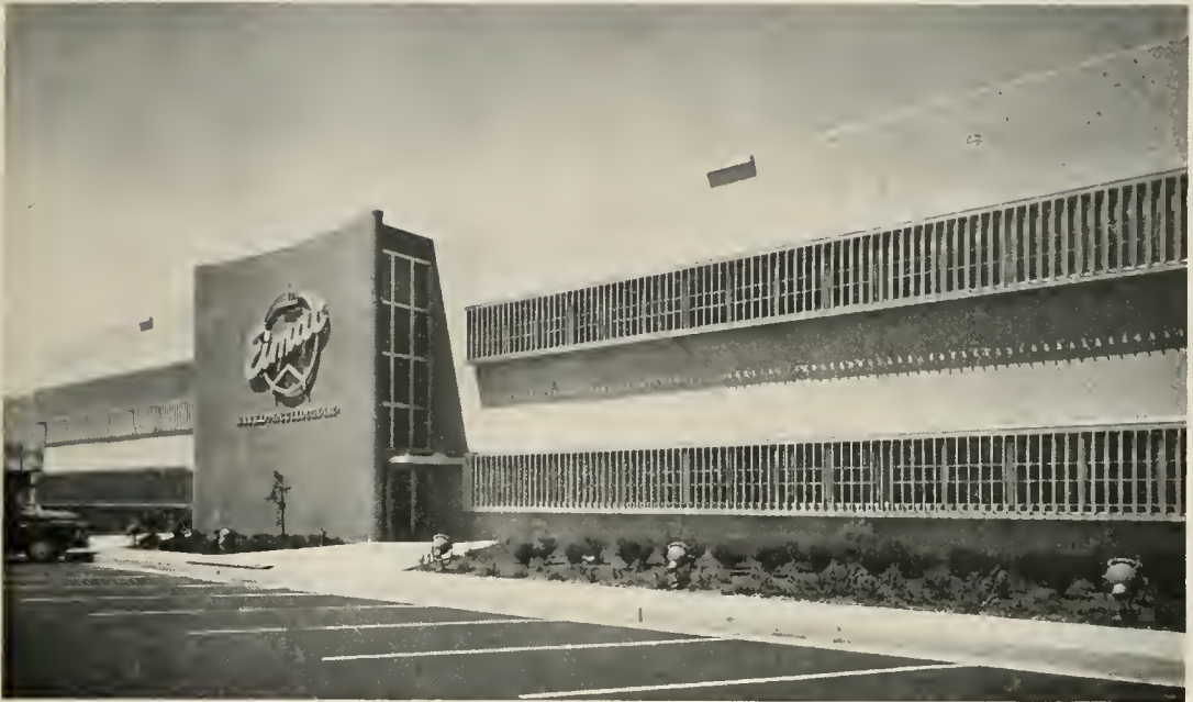
EITEL-McCULLOUGH, INC. is another addition to the rapidly expanding industrial area south of San Francisco. Exterior of 2-story office is surfaced with ceramic veneer of 3/4" square tiles applied to the slab while being poured. (Vincent G. Raney, Architect. Hall, Pregnaff & Matheu, Structural Engineers.)
