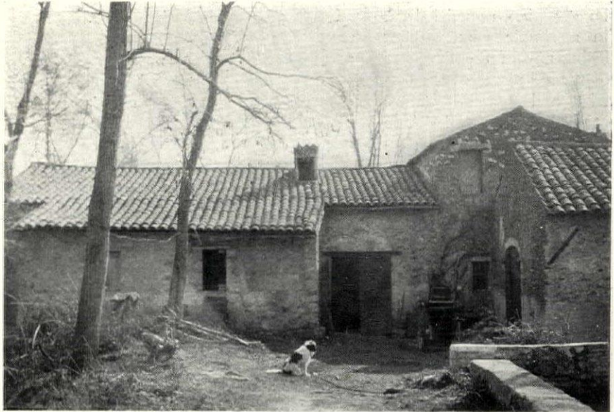
Low, Spreading Buildings of Stucco, with Tile Roofs Another view of mill at Cagnes-sur-Mer
