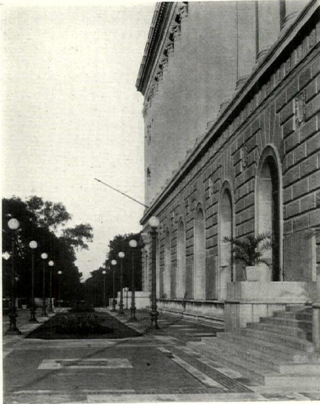
View of Terrace and Entrances
