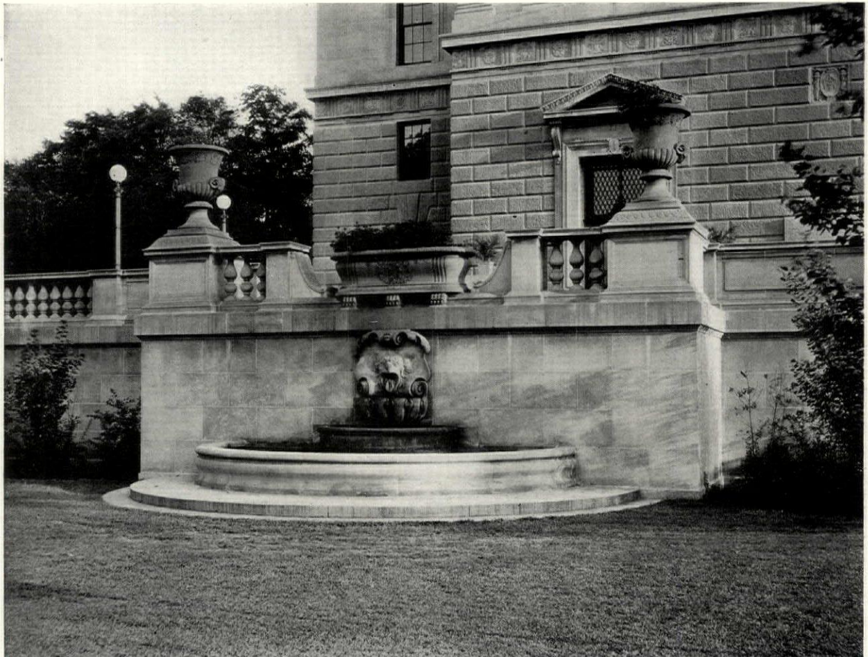
Fountain Placed Against Retaining Wall of Terrace
