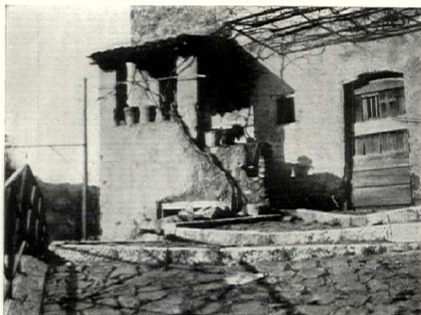
Doorway at Villeneuve-Loubet
