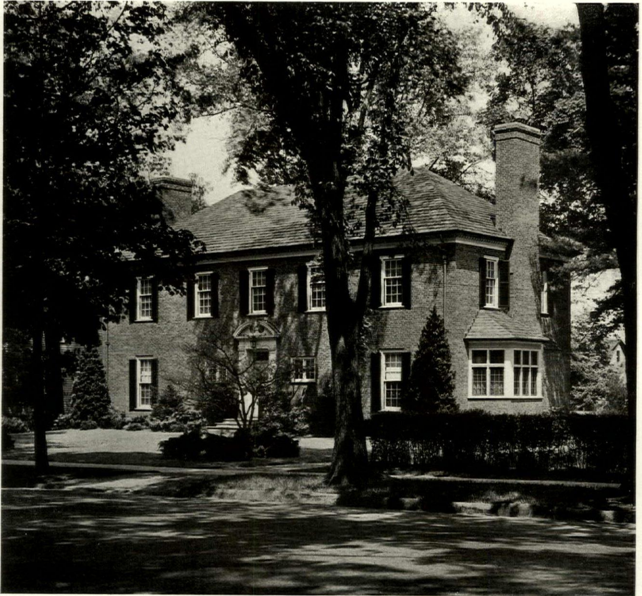
GENERAL VIEW OF HOUSE FROM STREET
