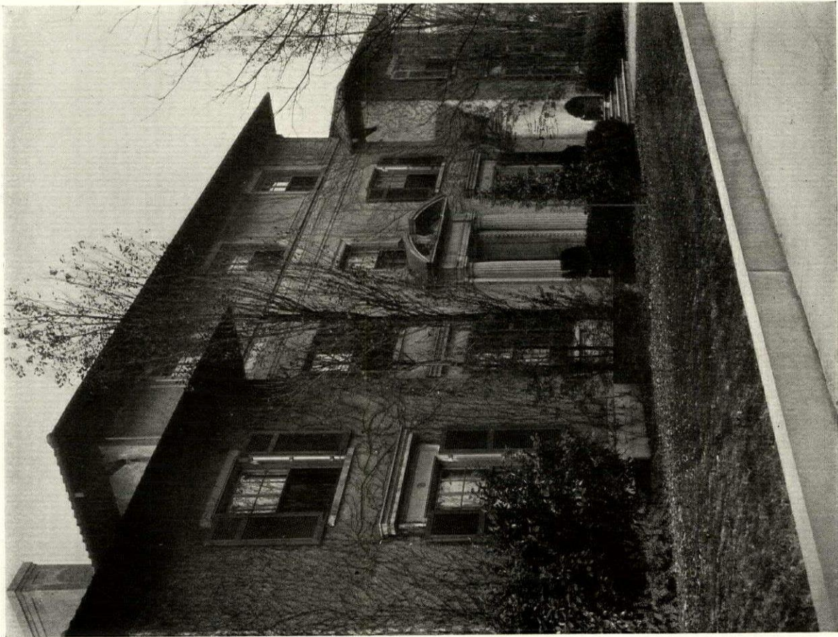
VIEW OF STREET FACADE
