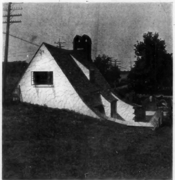
Detail of Roof and Chimney
