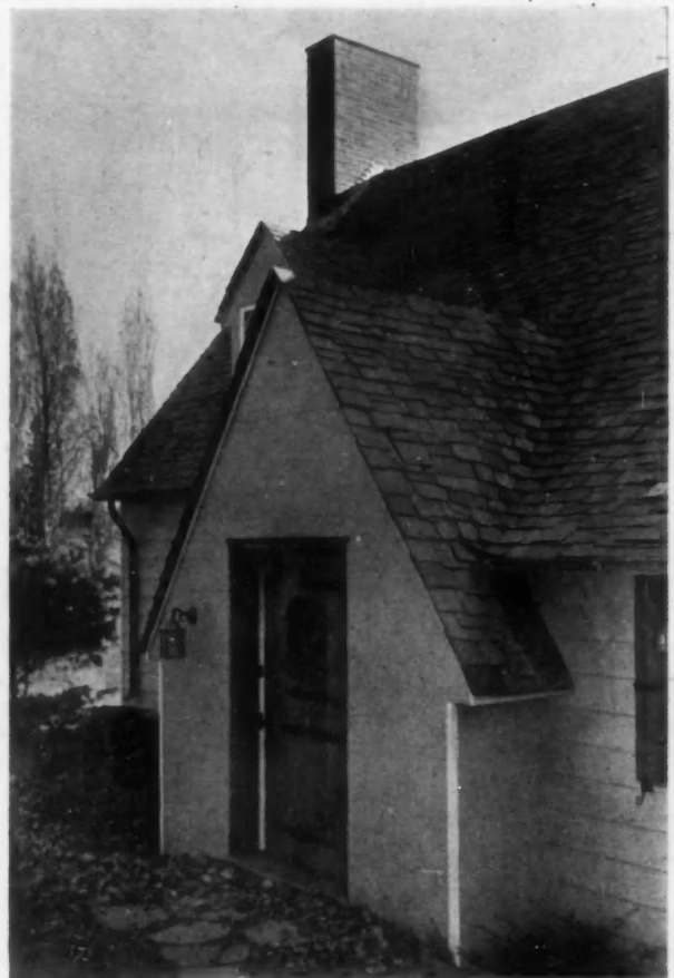
The Main Doorway
