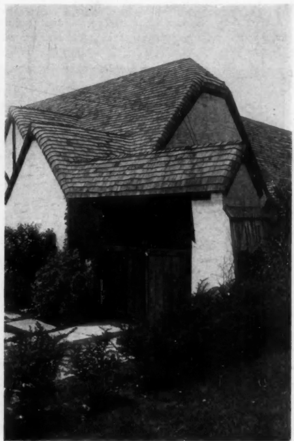
Detail of Service Entrance
