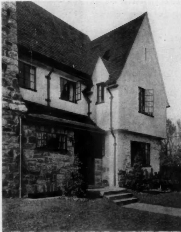
Architecture of the "Modern English" Type Makes Excellent Use of Casement Windows
