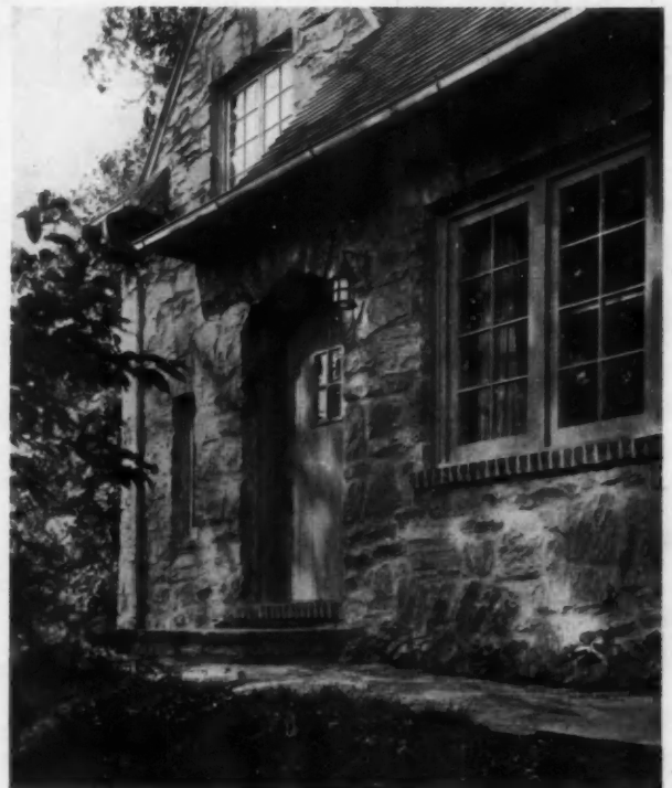
The Main Doorway
