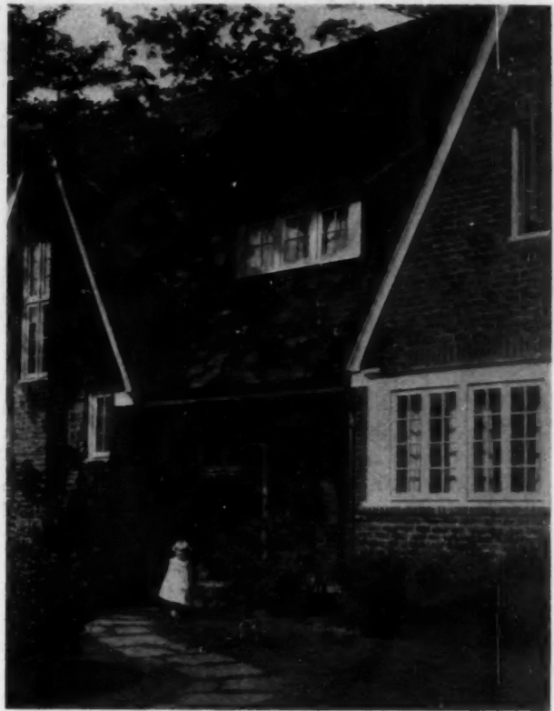
The Central Roof Pitch Was Determined by Requirements of the Second Floor Plan as Described in This Article
