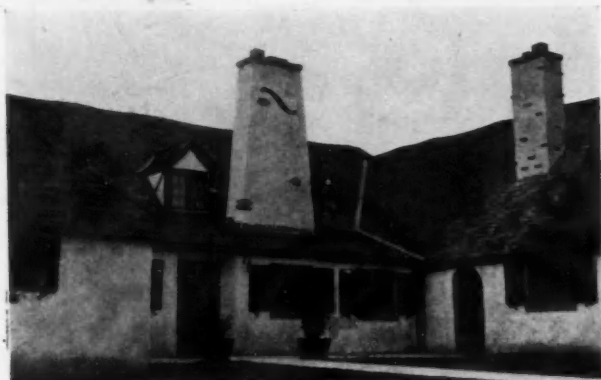
Entrance Detail, Ottawa Country Club, Ottawa, Ill. John Hannaford, Architect
