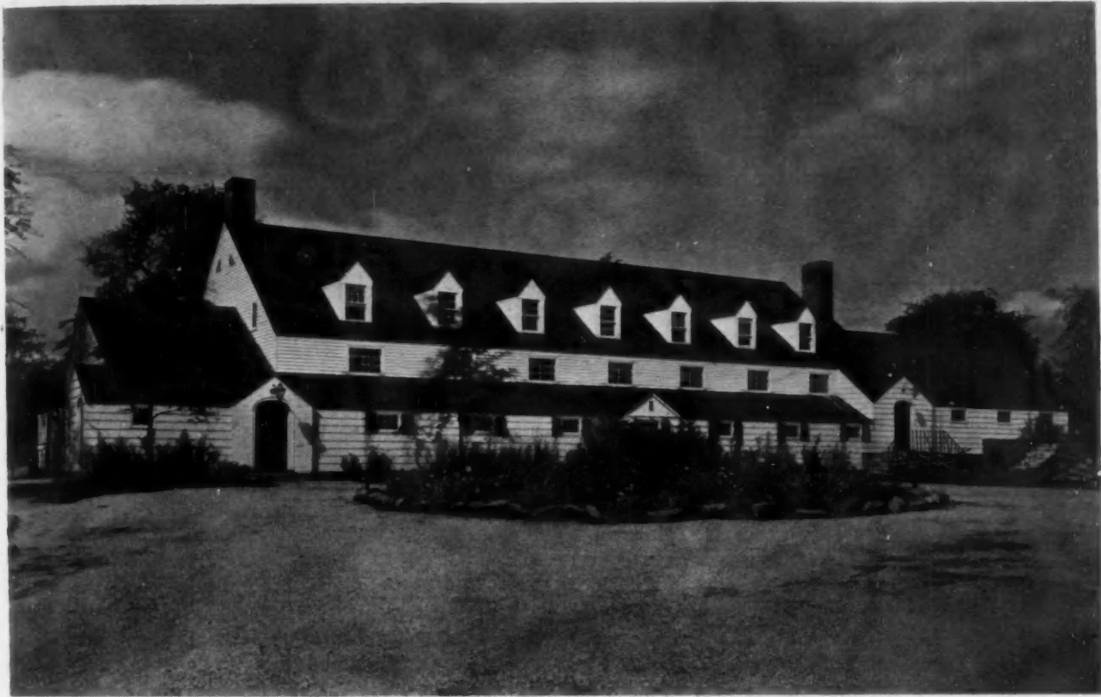
LOCKER BUILDING, NORTH HEMPSTEAD COUNTRY CLUB, PORT WASHINGTON, N. Y. WESLEY SHERWOOD BESSELL, ARCHITECT, NEW YORK
