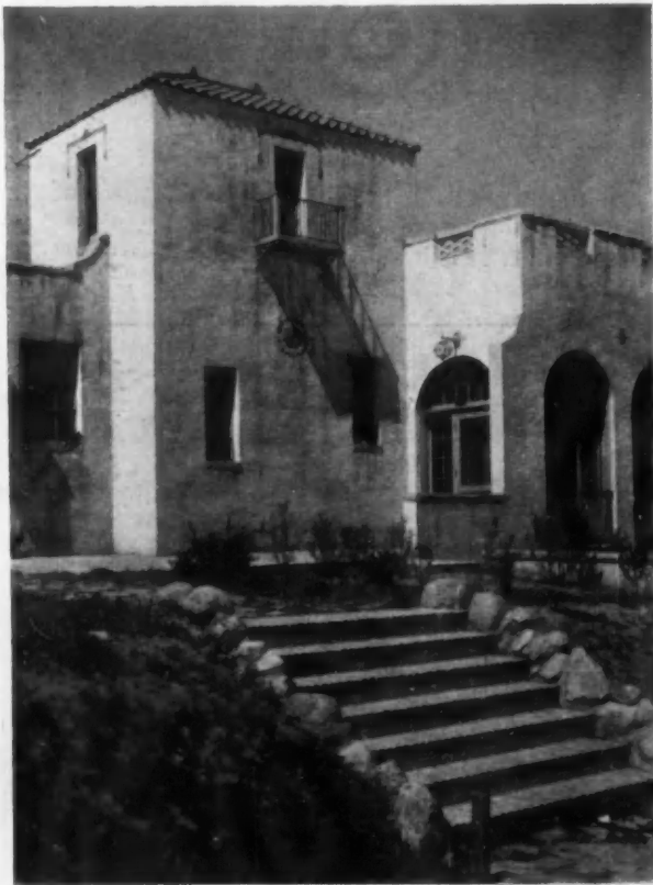
Detail of Entrance Front
