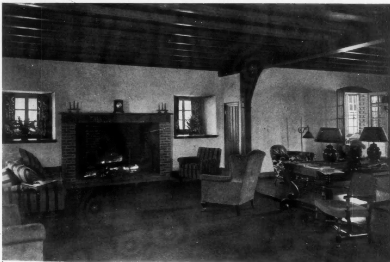
FIREPLACE IN LIVING ROOM PLAINFIELD COUNTRY CLUB, PLAINFIELD, N. J. ROGER H. BULLARD, ARCHITECT
