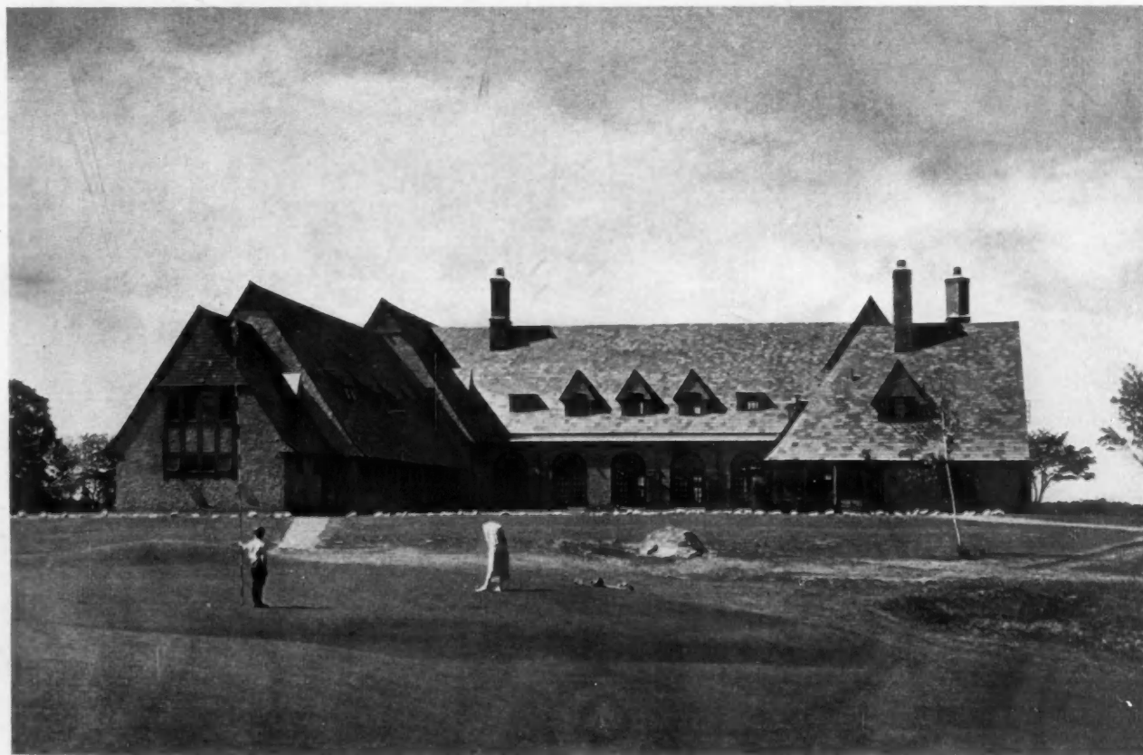
ELEVATION FACING EIGHTEENTH GREEN NORTH JERSEY COUNTRY CLUB, PATERSON, N. J. CLIFFORD C. WENDEHACK, ARCHITECT
