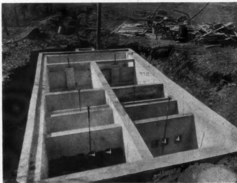
Fig. 4. A Large Type of Sewage Tank
