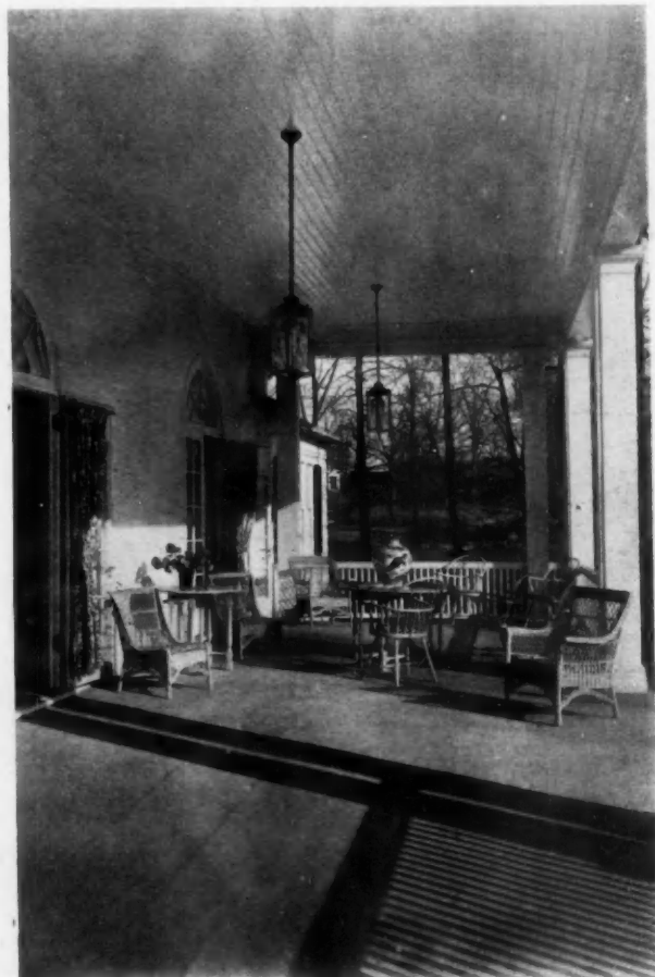
Detail of Veranda
