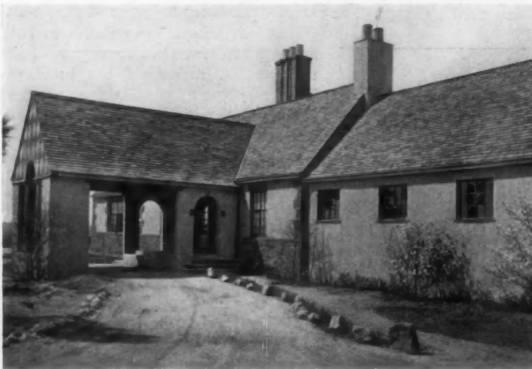
Detail of Entrance Front
