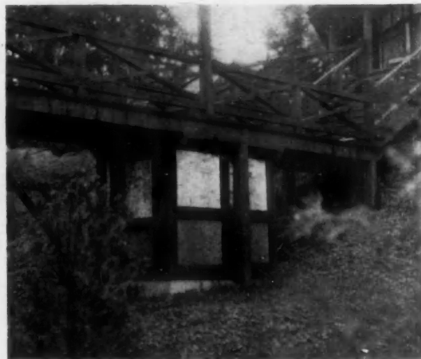
Fig. 14. Well Concealed Pump Housing
