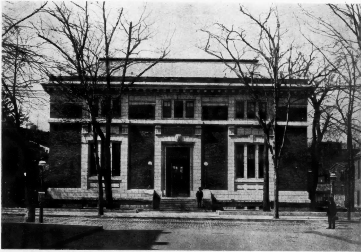
BEDFORD BRANCH, BROOKLYN PUBLIC LIBRARY LORD & HEWLETT, ARCHITECTS
