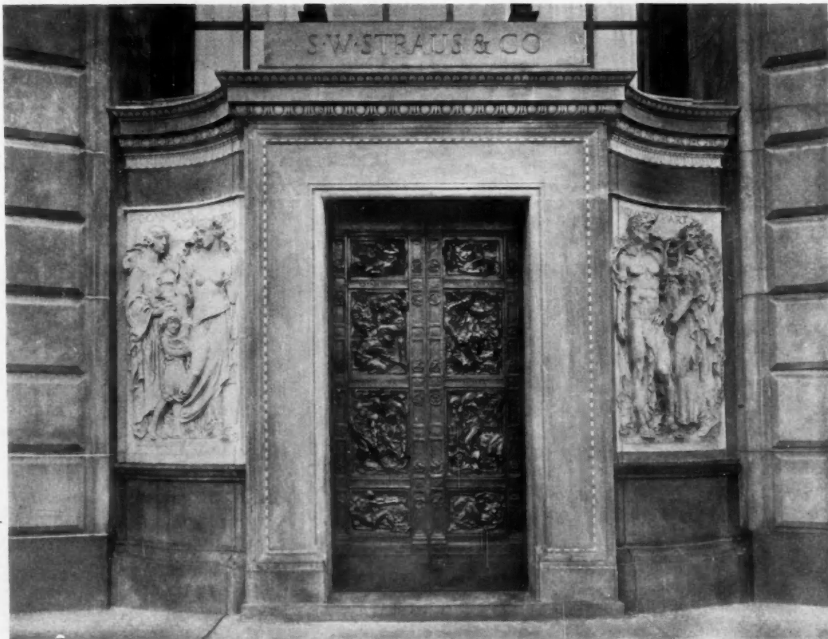
✓ Detail, Main Entrance, Straus Building, Chicago
