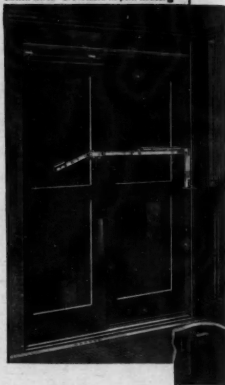
Electric Door Controller with cut-out switch in pit at bottom of elevator shaft. Pulley and weight — for controlling switch wires — are located in pent house.
