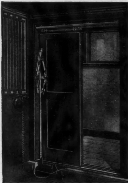
When doors are open the lock plate of the Mechanical Interlock is thrown forward and around handle of the car controller, which positively locks it, and prevents operation of the car.
