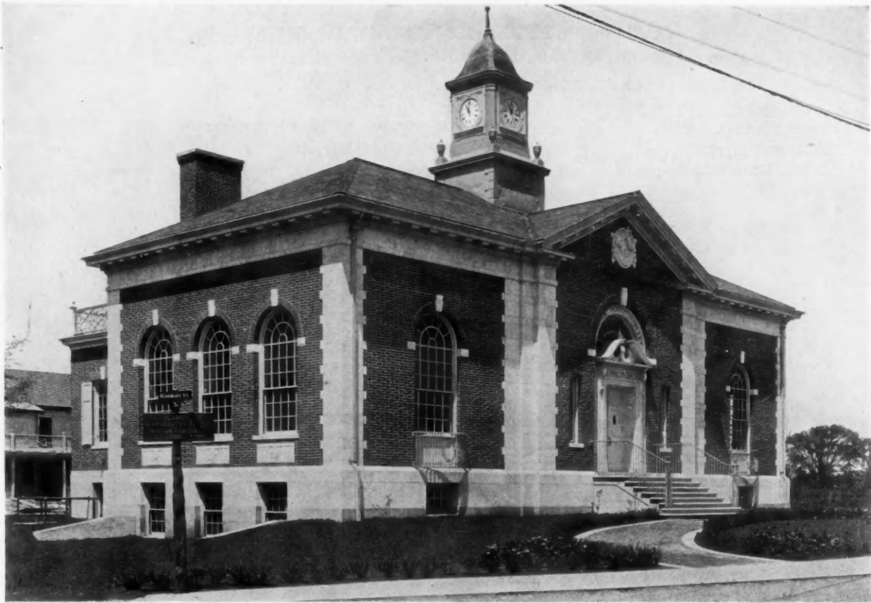
PUBLIC LIBRARY, NEEDHAM, MASS. RITCHIE, PARSONS & TAYLOR, ARCHITECTS
