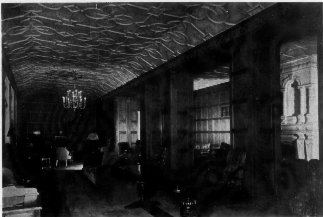
LOUNGE, LOOKING TOWARD FIREPLACE ALCOVE
