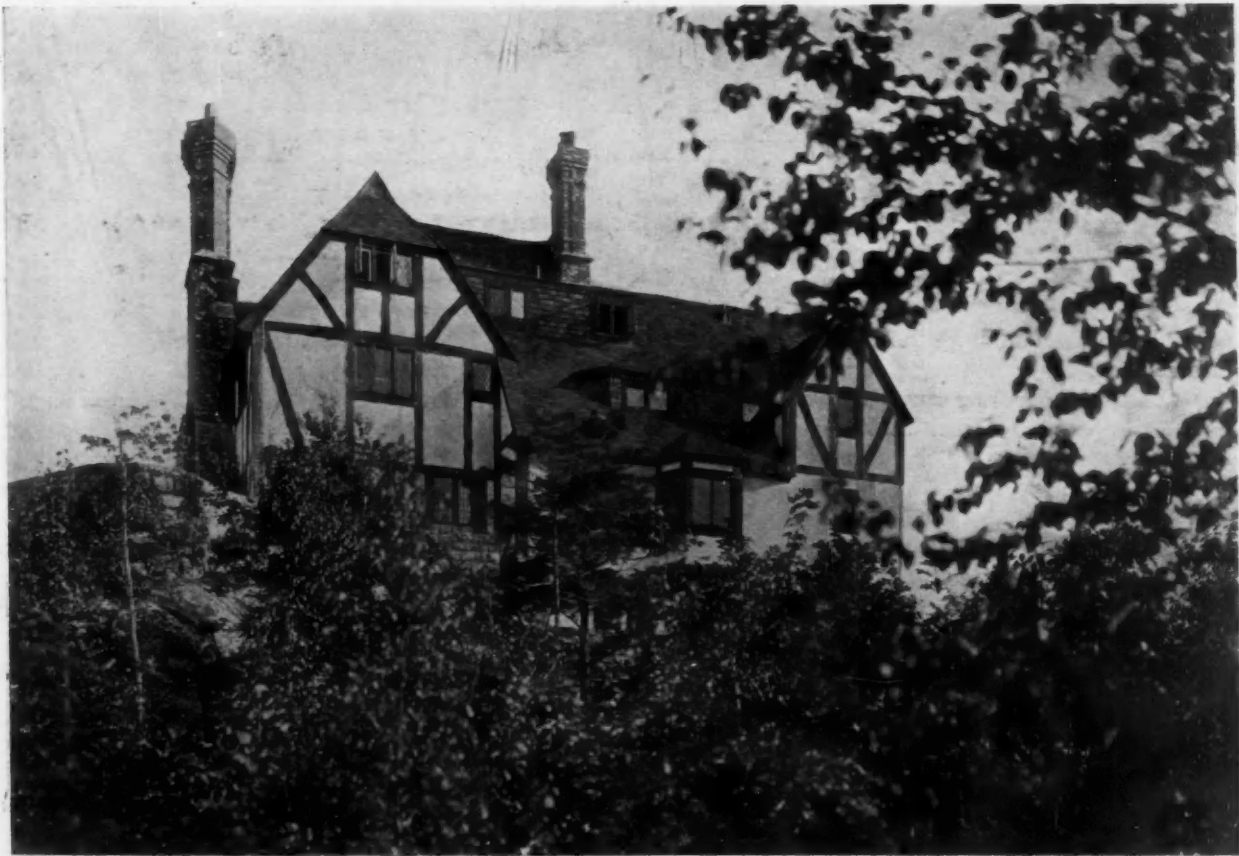
The North Side of the House Rises Above the Tree Tops
