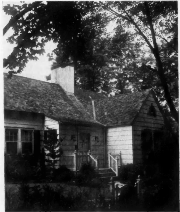
Detail of a House at Great Neck, N. Y. Patterson-King Corporation, Architects
