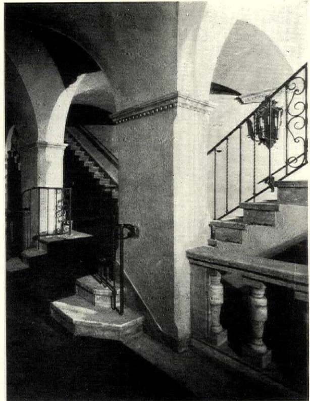
Detail, Main Stairway
