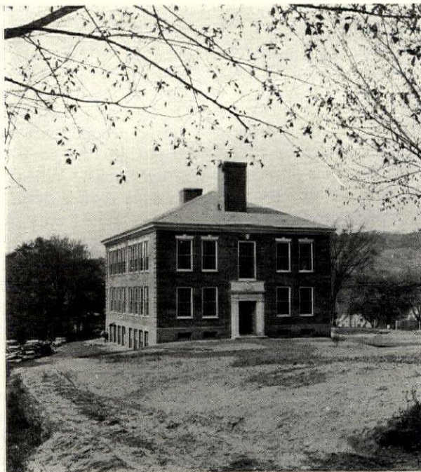
Summer Street Schoolhouse, Springfield, Vt. Brainerd & Leeds, Architects
