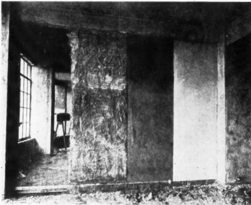
"Flagg Partition" in three stages of construction
