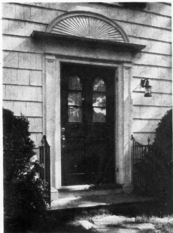
Entrance Detail, House of Ernest L. Cosgrove, Esq.
