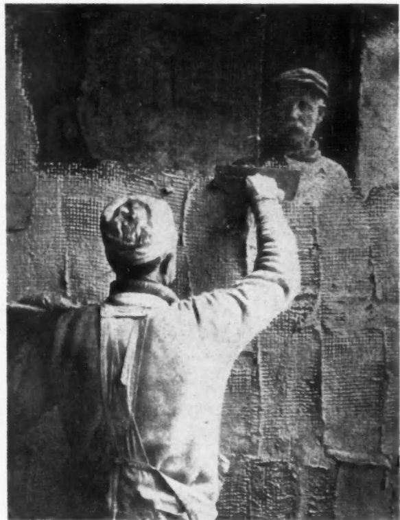
Plasterers working against each other on wire lath
