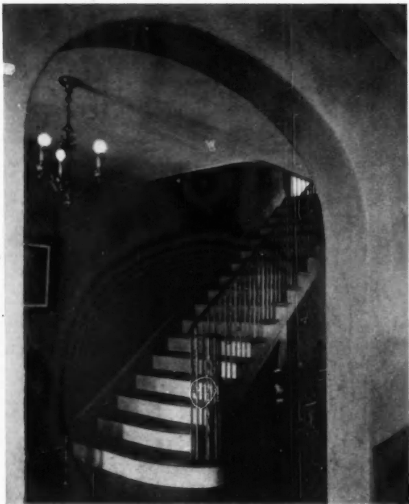
VIEW IN STAIR HALL
