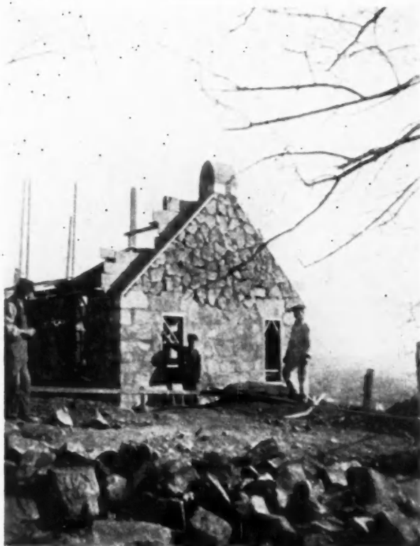
Mosaic Rubble Before and After Pointing
