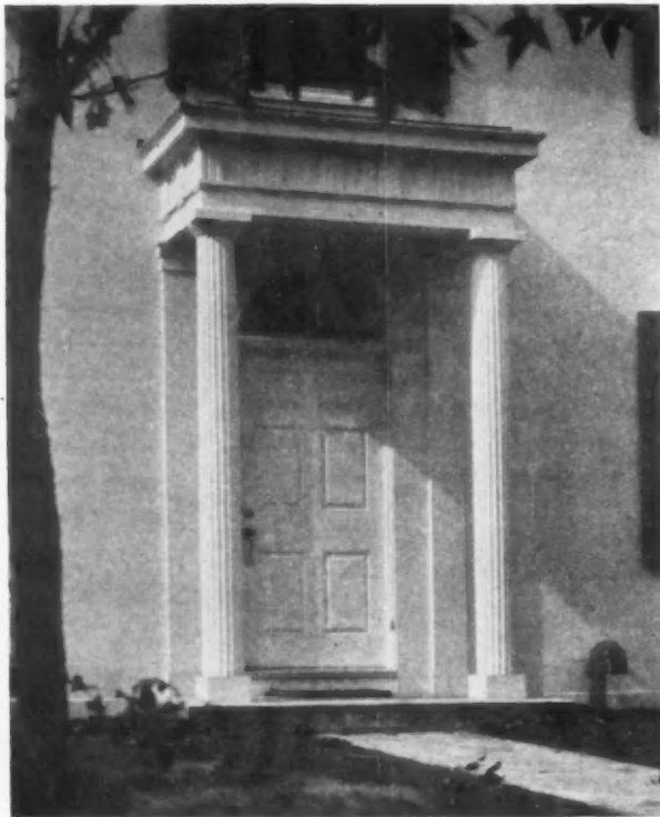
Entrance Detail, House of Dr. Francis Collins
