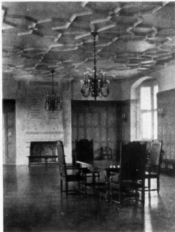
Detail, Hall, Neeley Memorial Building, Vanderbilt University Henry C. Hibbs, Architect
