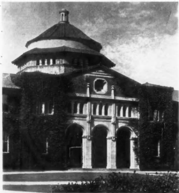
Administration Building (Southern Branch), University of California
