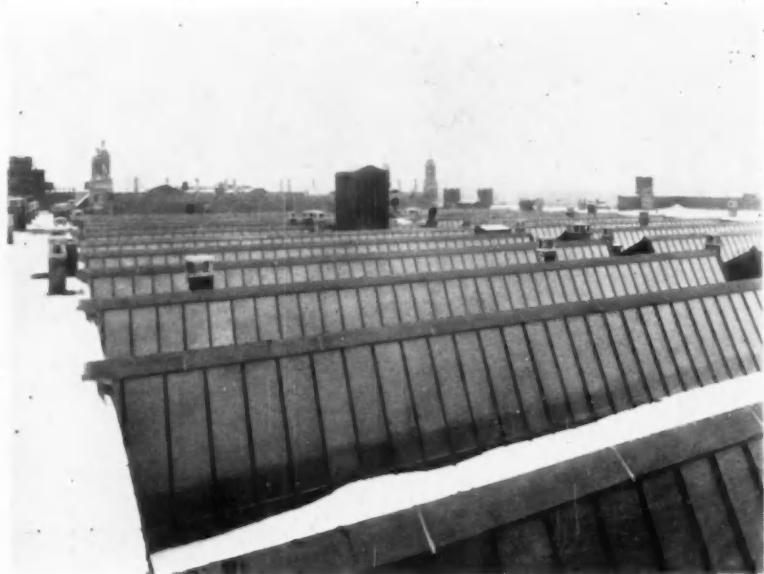
Laboratories for general student work, being the principal portion of any chemistry building, adequate provision for the best working conditions are imperative. Note the construction of these double-glazed skylights over the student laboratory at Sterling Laboratory
