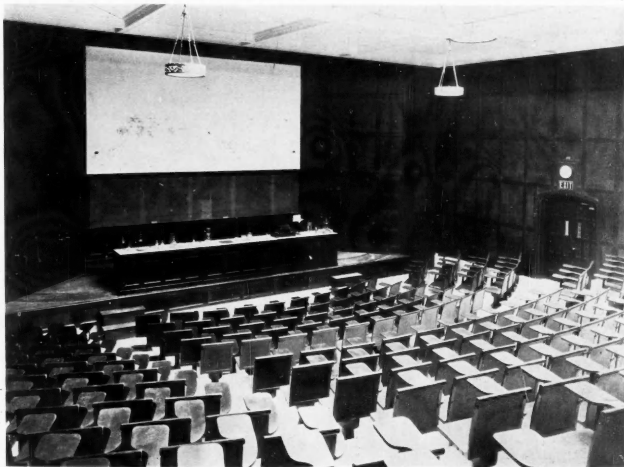
The lecture room, Sterling Chemistry Laboratory, has its lighting regulated by a skylight butterfly shutter operated from the stationary center lecture table. Movable sections of table roll on tracks to preparation room at back. Note down draft in center section of table and fume closet in blackboard
