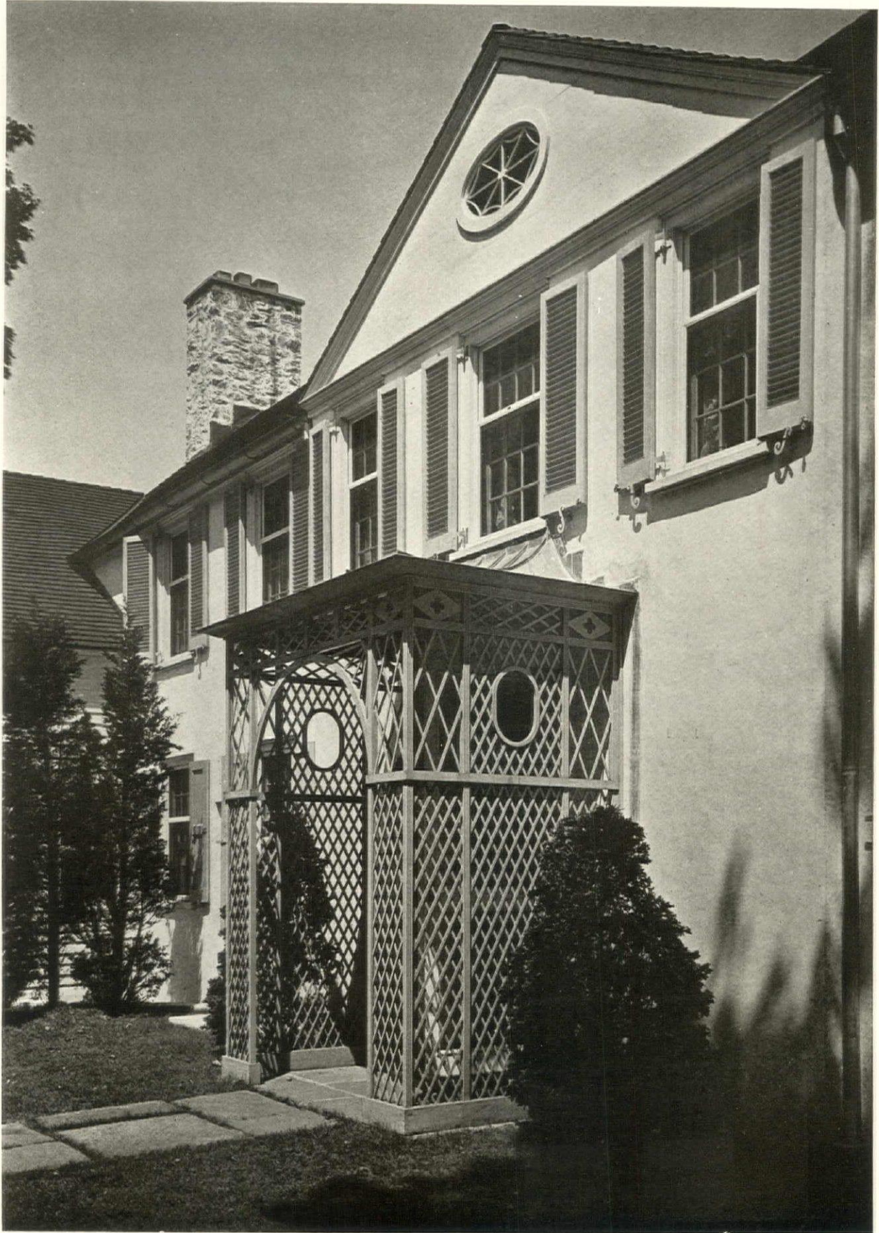
THE ENTRANCE HOUSE OF MRS. A. C. BALDWIN, BEDFORD HILLS, N. Y. BUTLER & CORSE, ARCHITECTS
