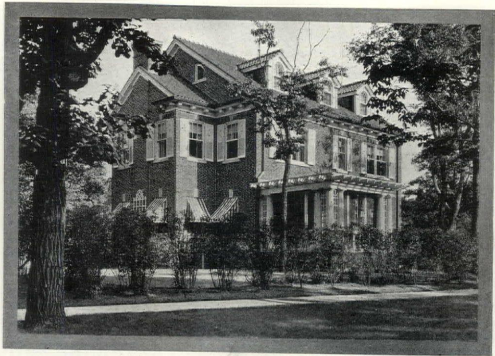
Residence of Mr. John Nyden, Architect, Evanston, Ill. C. J. McDonough Company, Heating Contractors
