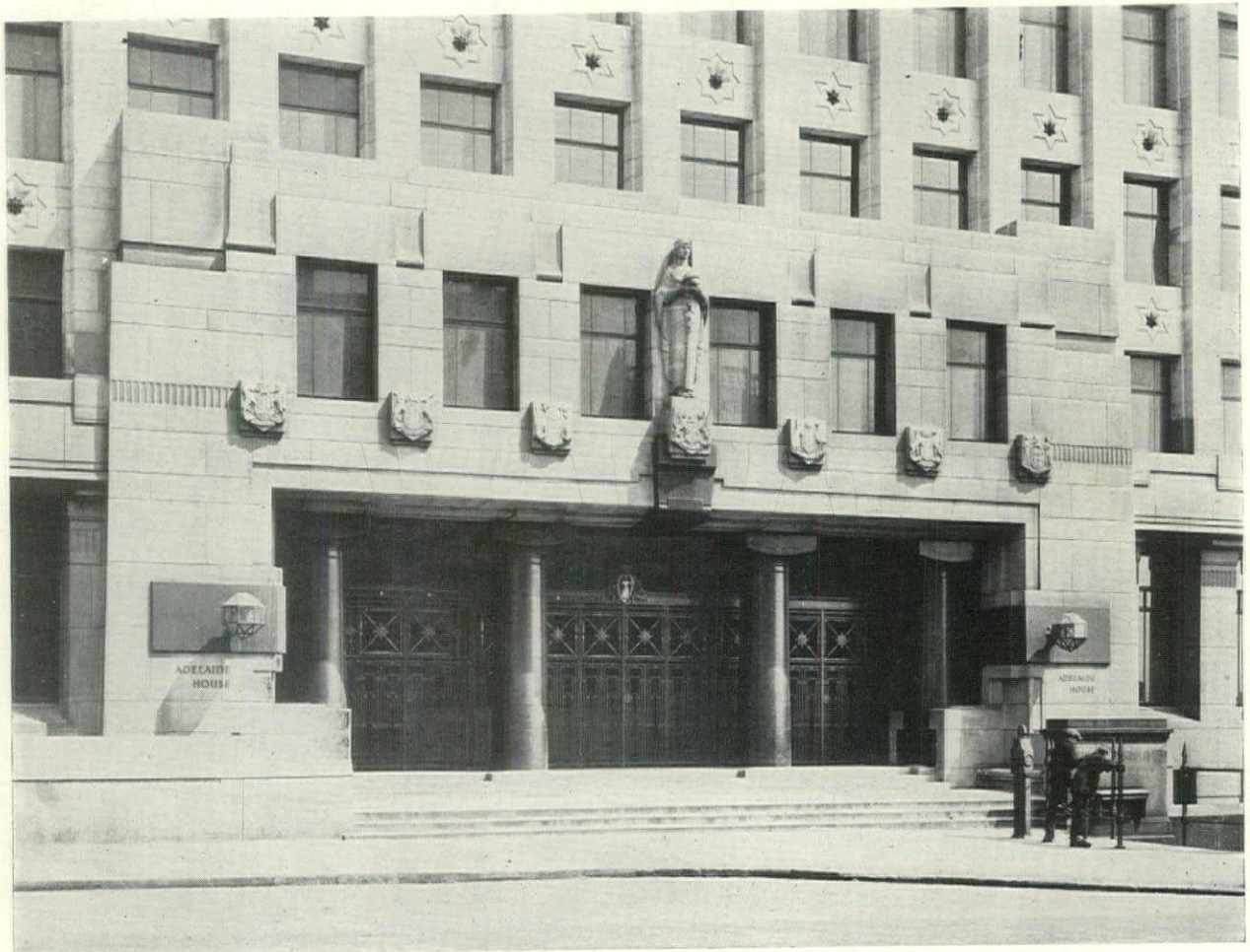
Entrance, Adelaide House
