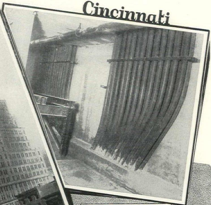
Sherarduct installation in "The Enquirer" building. Lockwood, Green & Co., Engineers.
