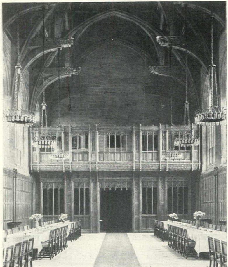
Open Timber Roofing; Graduate College, Princeton Cram & Ferguson, Architects
