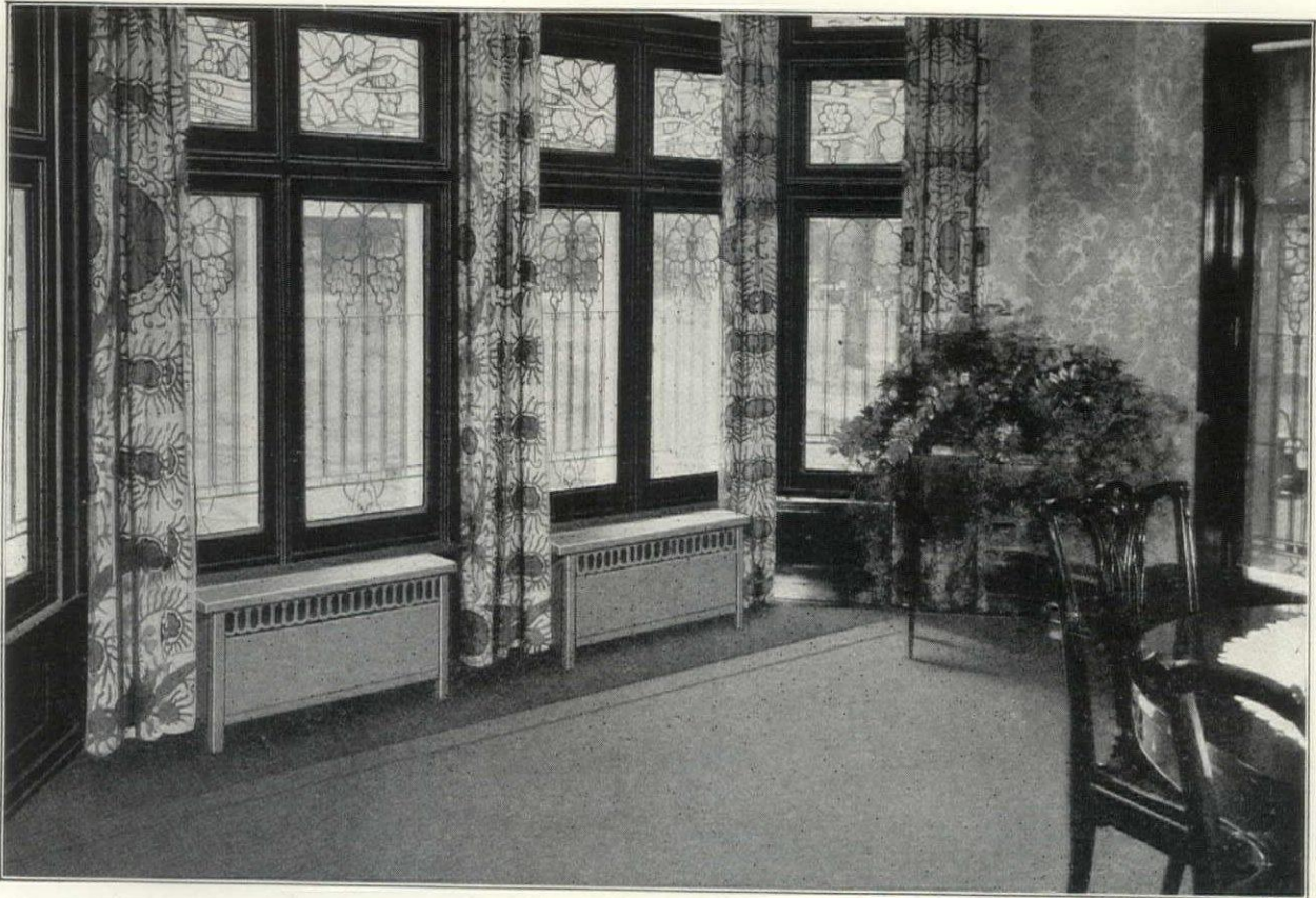
A typical installation of Visible Heat Cabinets. These cabinets are available in a wide range of sizes and styles.
