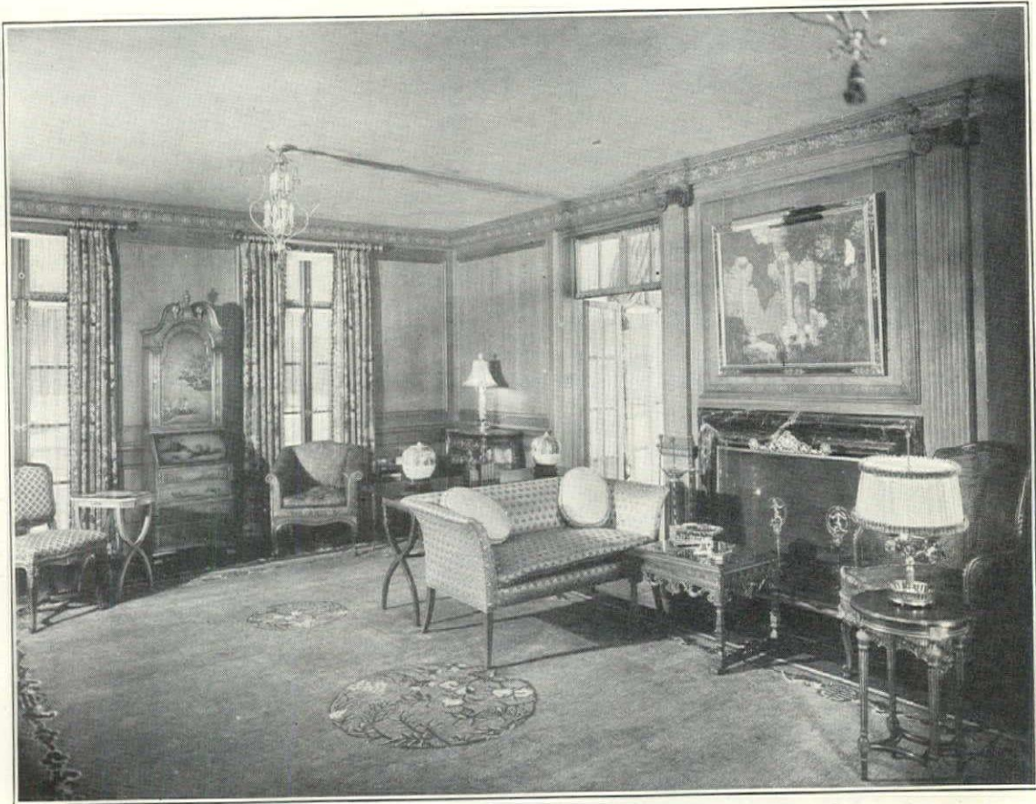
Residence of M. E. Greenebaum, Jr., Glencoe, Ill. Walnut room designed and executed by Homer Studios, Chicago
