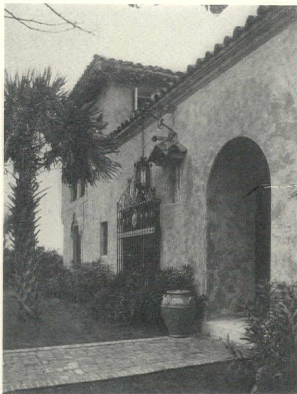
Detail, House of George Dobyne, Esq., Palm Beach Marion Sims Wyeth, Architect
