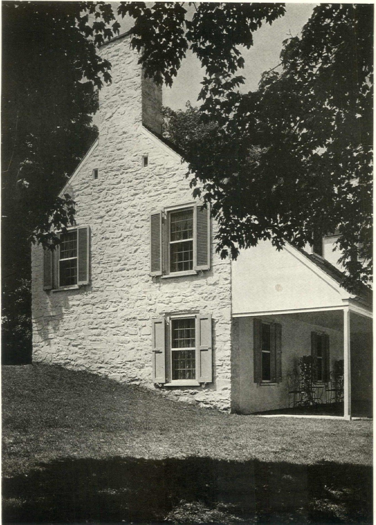
END ELEVATION FROM ORCHARD HOUSE OF MRS. A. C. BALDWIN, BEDFORD HILLS, N. Y. BUTLER & CORSE, ARCHITECTS
