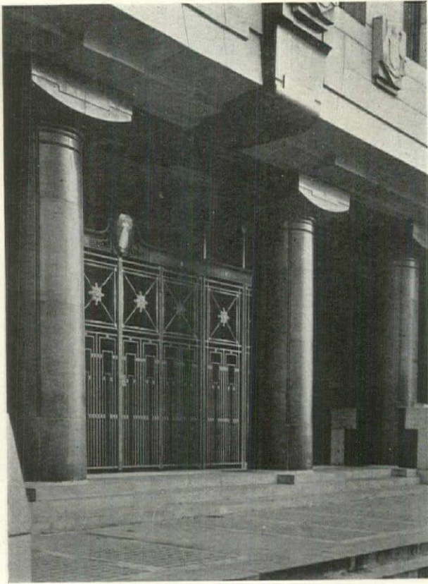
Detail of the Entrance
