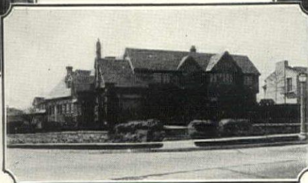
Residence of C. E. Listenwaller, Los Angeles, Calif. Architect, Arthur B. Benton, designer of the famous Mission Inn, Riverside, Calif. Contractor, R. J. Smith.
