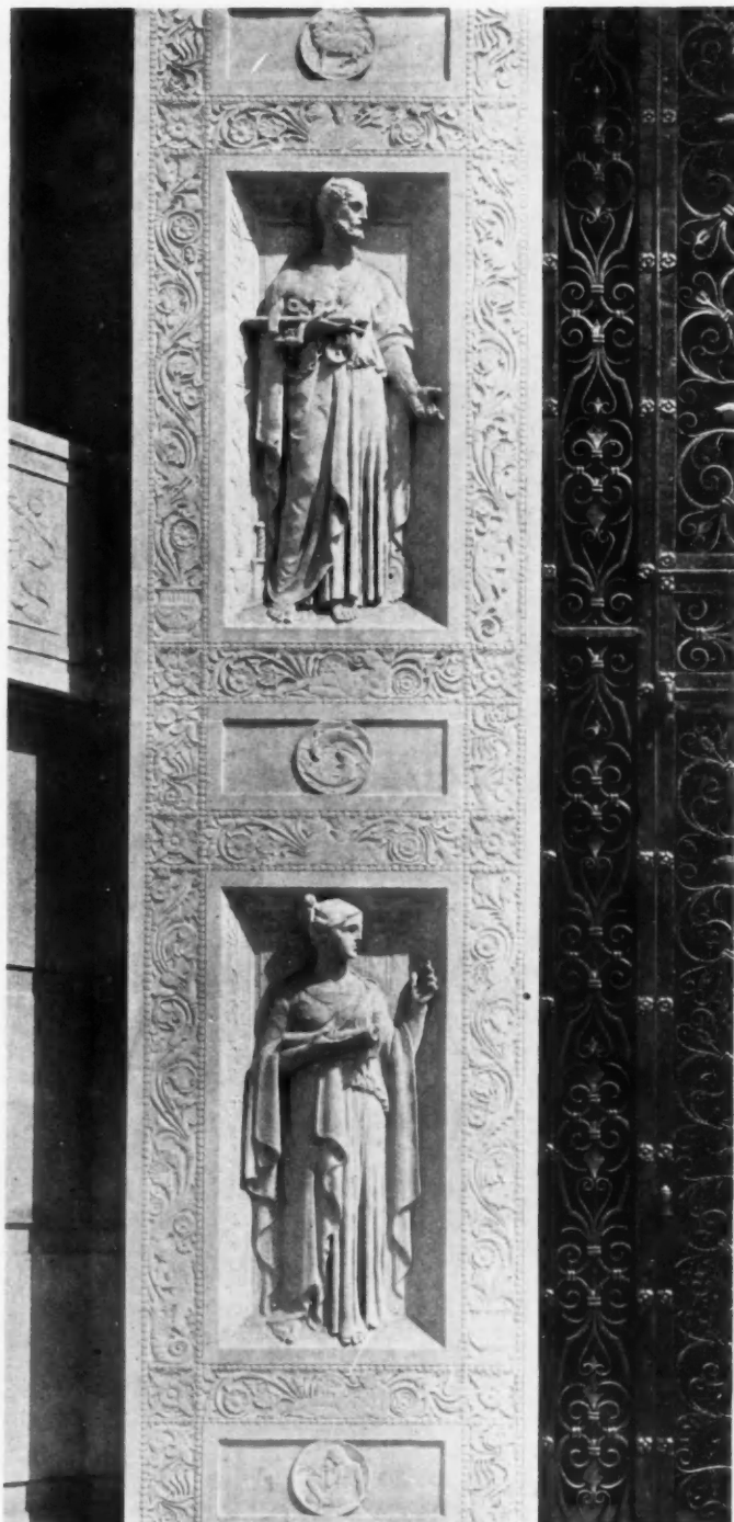
Detail of Doorway Hardware Mutual Insurance Co. Building
