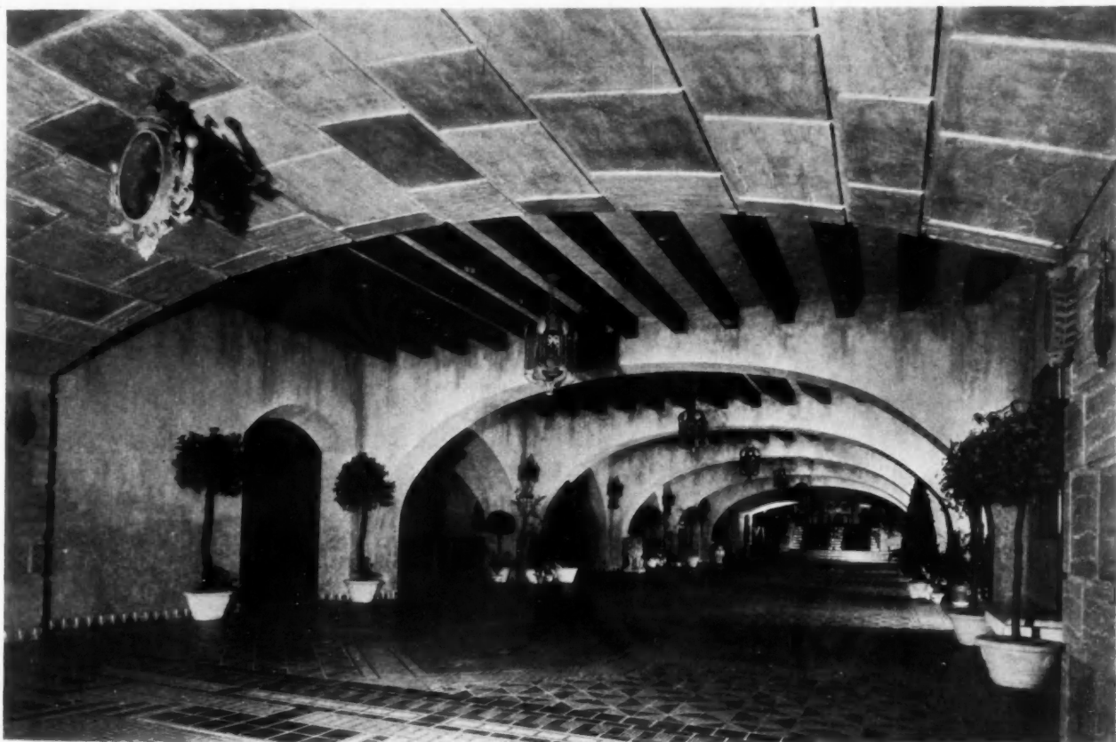
THE LOBBY ARAGON BALLROOM, CHICAGO HUSZAGH & HILL, ARCHITECTS
