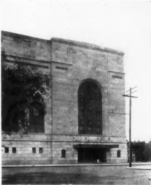
Detail, Auditorium, Minneapolis
