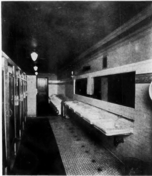
Men's Room, Public Comfort Station, Trenton, N. J. Hill & Gollner, Architects
