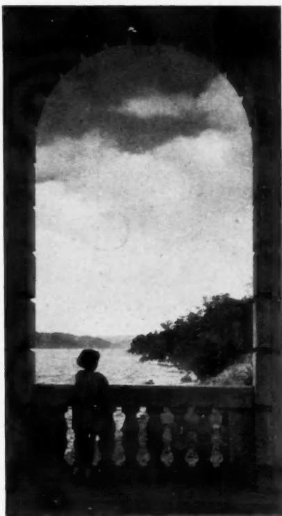
Detail, Pavilion, Kensico Dam York & Sawyer, Consulting Architects
