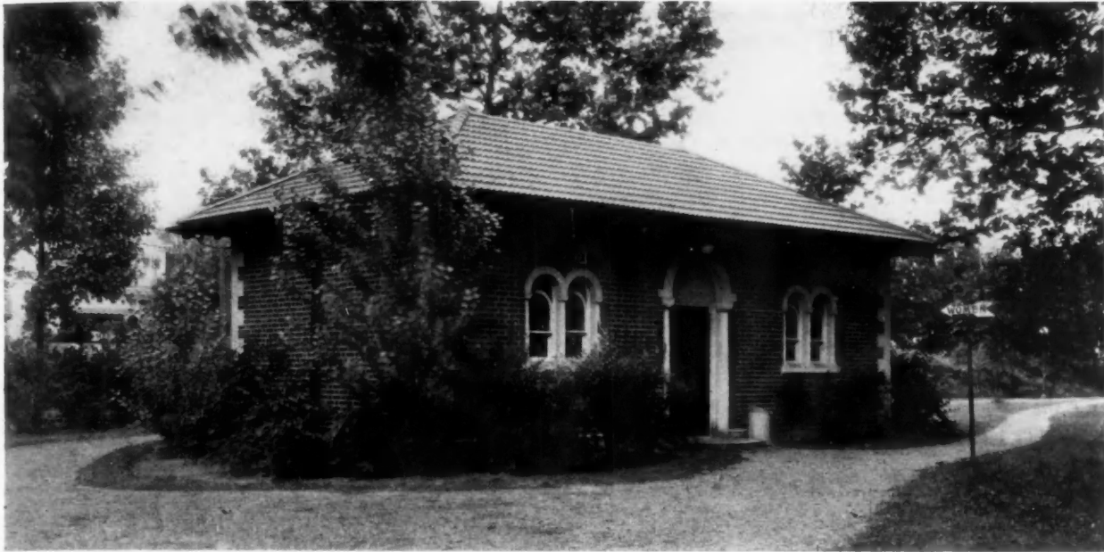
Public Comfort Station, Trenton, N. J. Hill & Gollner, Architects
