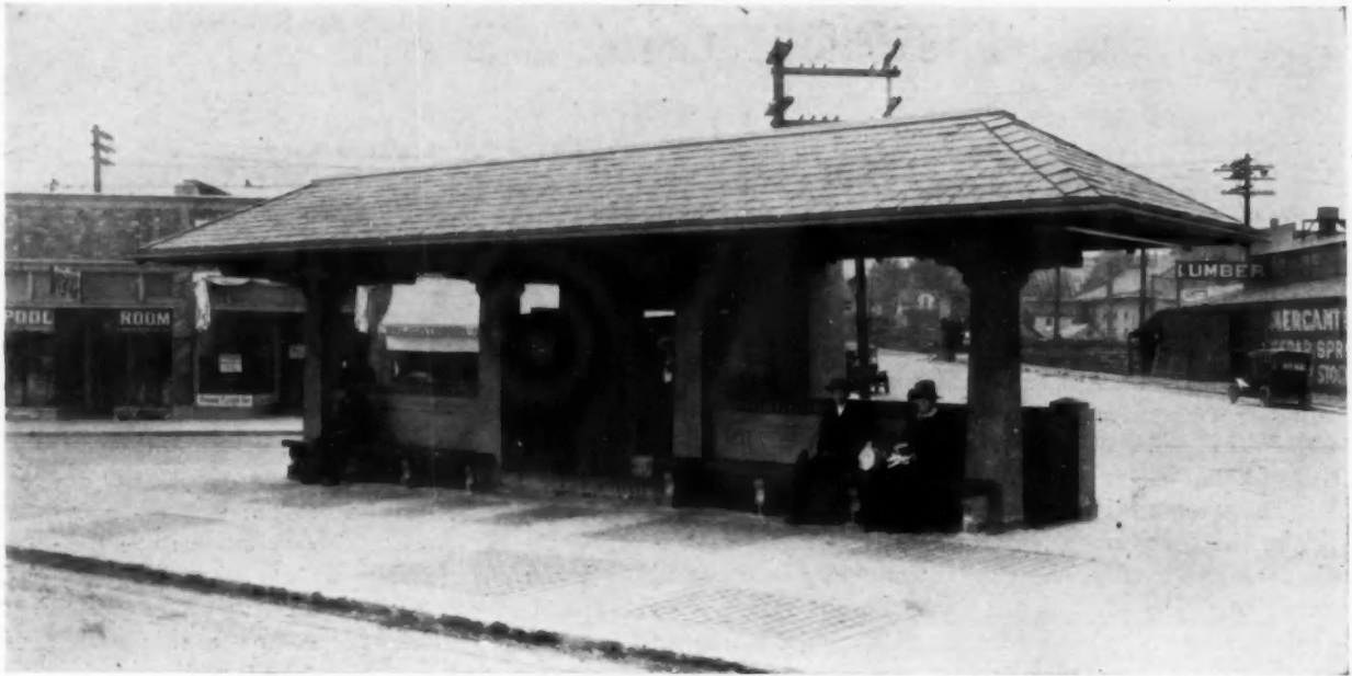
Shelter Over Entrance to Underground Comfort Station, Seattle J. Everett, Architect
