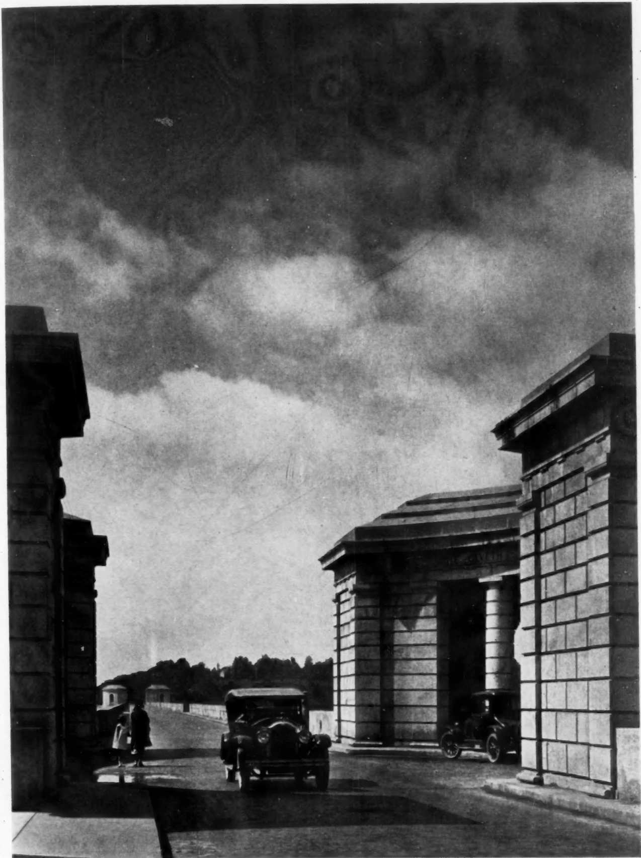
ROADWAY OVER KENSICO DAM, NEW YORK YORK & SAWYER, CONSULTING ARCHITECTS
