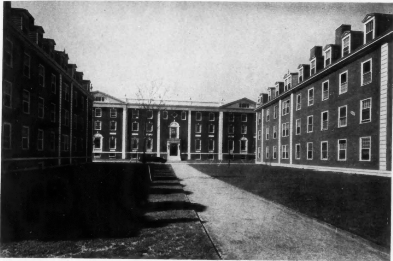
MORGAN HALL AND DORMITORIES
