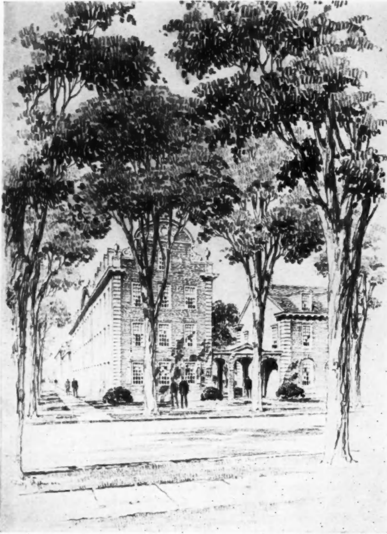
Chase Hall and Future Instructors' House
