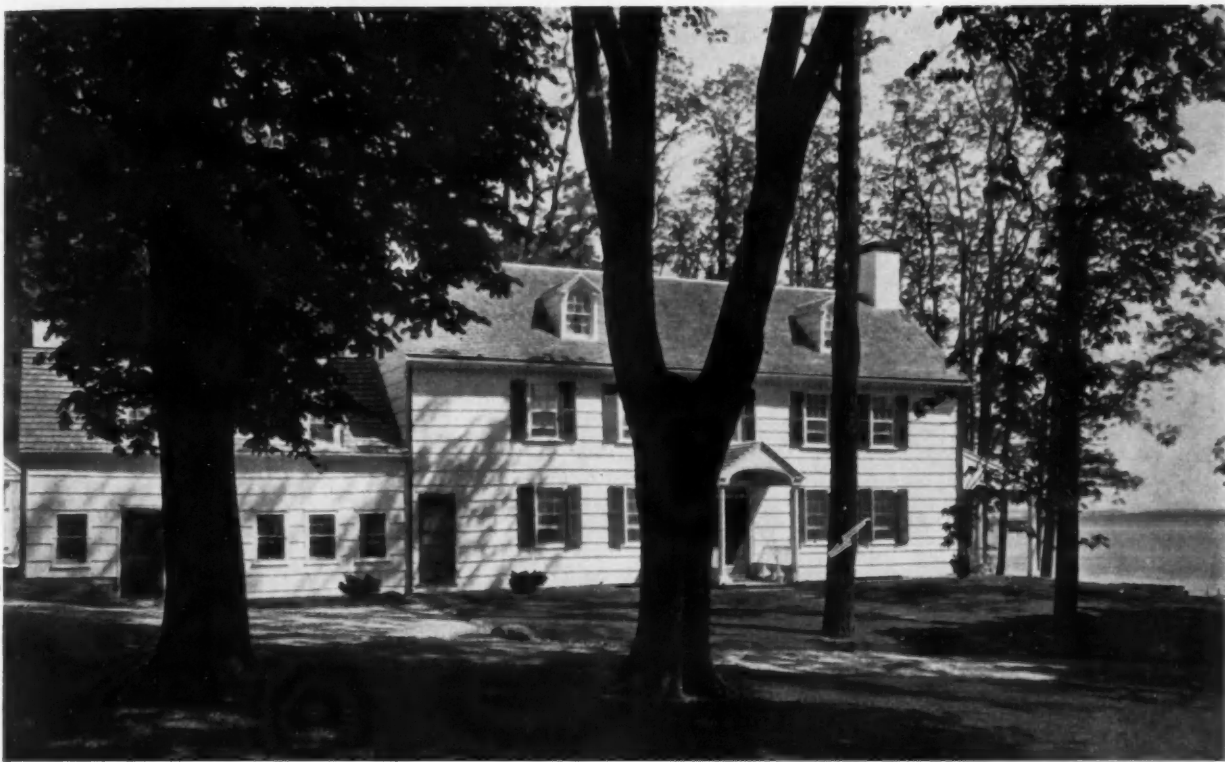
HOUSE OF WILLIAM H. DIXON, ESQ., ST. JAMES, N. Y. PEABODY, WILSON & BROWN, ARCHITECTS
