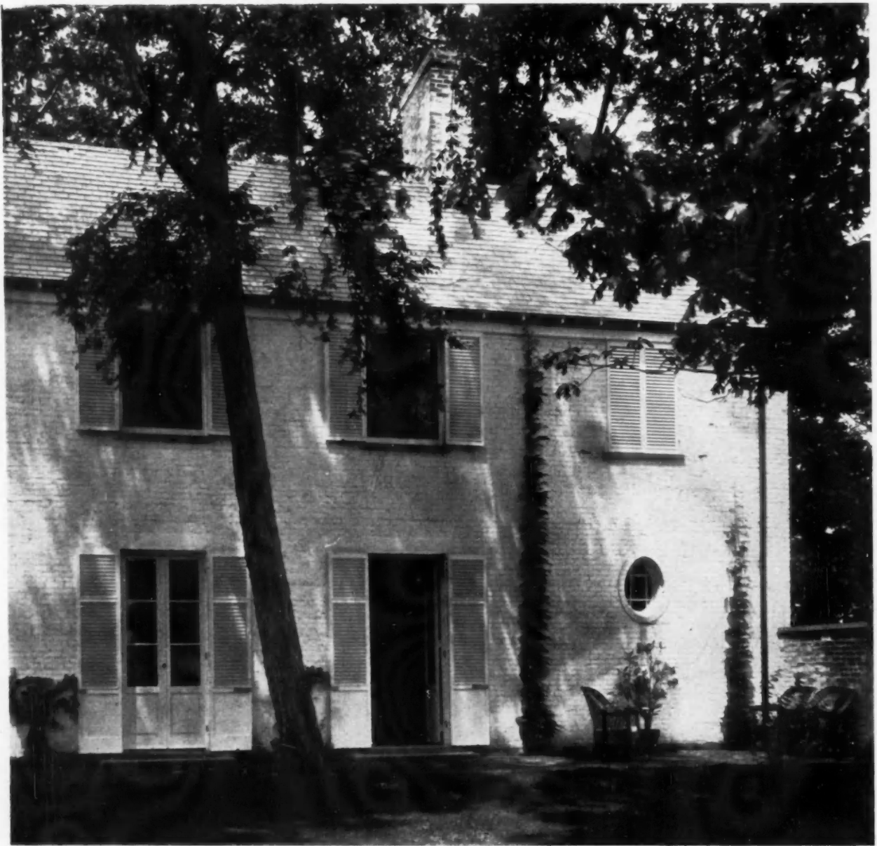
Terrace, House of Newton P. Bevin, Esq., Jamaica, N. Y. Newton P. Bevin, Architect
