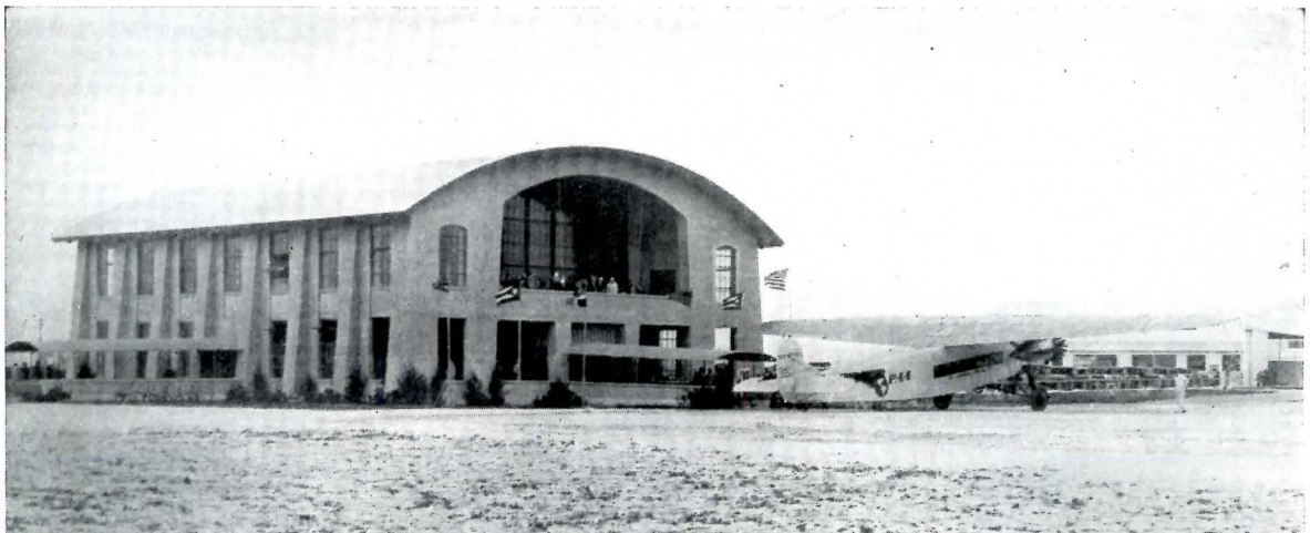
Airport Passenger Terminal of the Pan-American Airways, at Miami Delano & Aldrich, Architects
