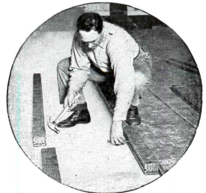
Bloxonend comes in 8 ft. lengths. The tough endgrain forms the wearing surface.
