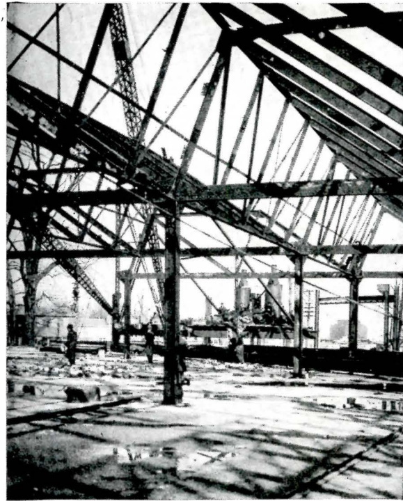
In Winter Superintendence it is Well to See that Snow Accumulations are Removed Before a Thaw Forms Puddles which an Overnight Freeze May Turn to Treacherous Sheets of Ice
