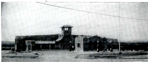
Building at the Dennison Airport, Atlantic, Mass.
