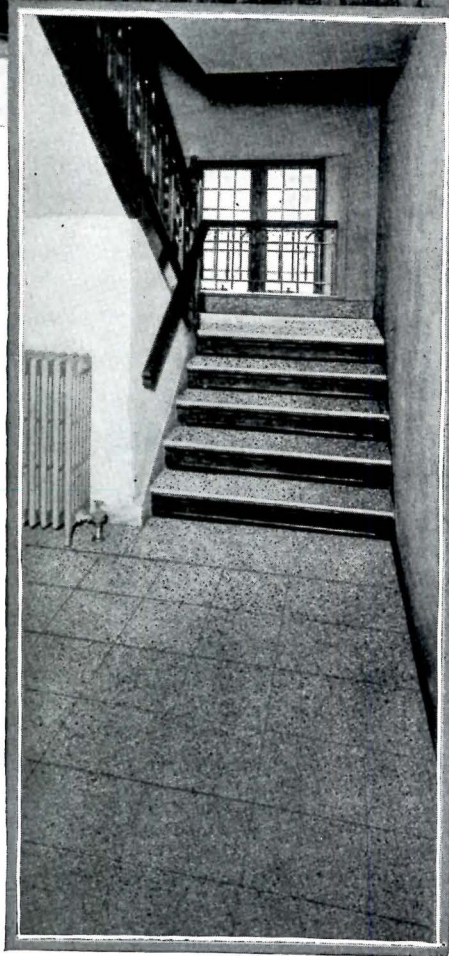
Stairway, hall and stair landings of Alberene Stone at Union Theological Seminary, New York, N. Y. ALLEN N. COLLINS, Boston, Architect
