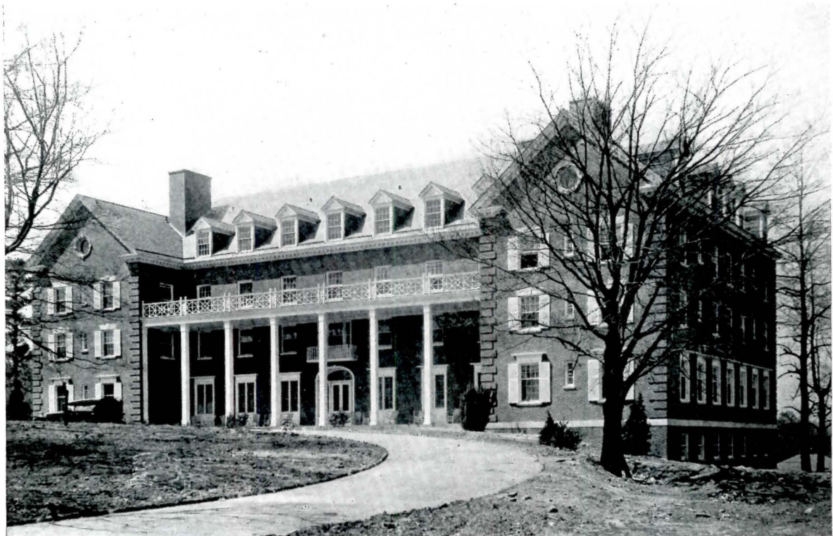
Brick Used Over Reinforced Concrete Frame, Sanitorium Near Atlanta, Ga. Hentz, Reid & Adler, Architects
