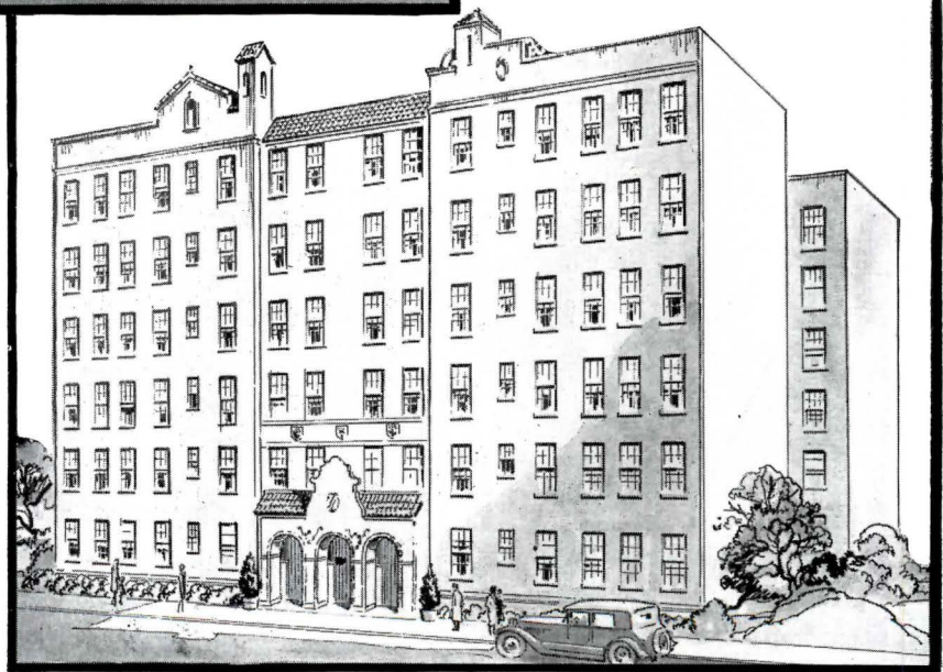
These two new apartment houses, 2101 and 2111 Myra Court, Brooklyn, N. Y. are Electrolux-equipped. Boris W. Dorfman, Architect.
