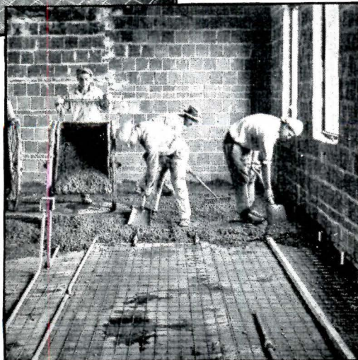
(right) Placing concrete on STEELTEX—water-tight form, correct reinforcing.
