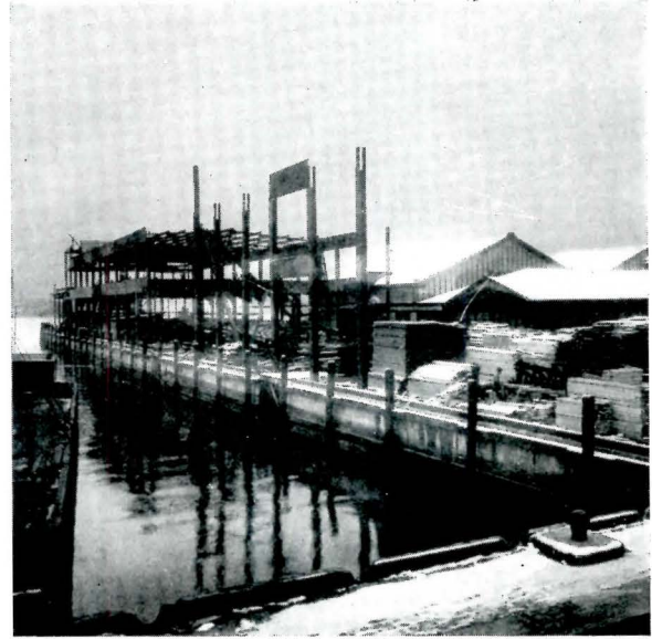
All-over Coverage Given a Municipal Pier which Was Completed on Scheduled Time Through a Winter of Record Cold and Snow. Behind the Tarpaulins, a Carefully Worked out Radiation System Provided the Requisite Heat
