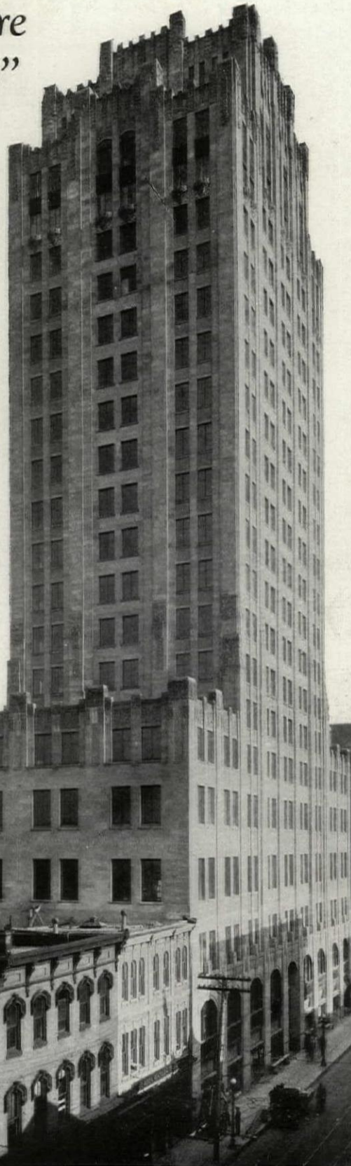
Toronto Daily Star Building, Toronto, Canada. Chapman & Oxley, Architects. Thompson-Starrett Co., Builders. First two stories Canadian granite; other 20 stories Standard Gray Indiana Limestone.
