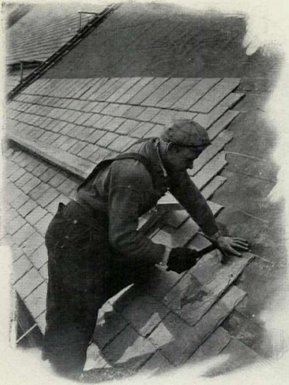
Nailing Slate directly to roof-deck of Federal Nailing Concrete Slabs on a community building.
