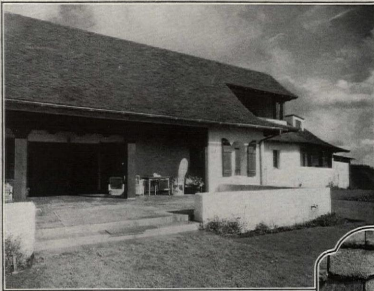
The Paul S. Winslow Residence at Honolulu, Hawaii Dickey & Wood, Architects
