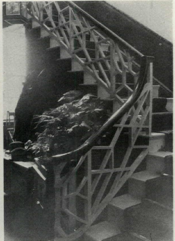
LOWER PART OF STAIRWAY
