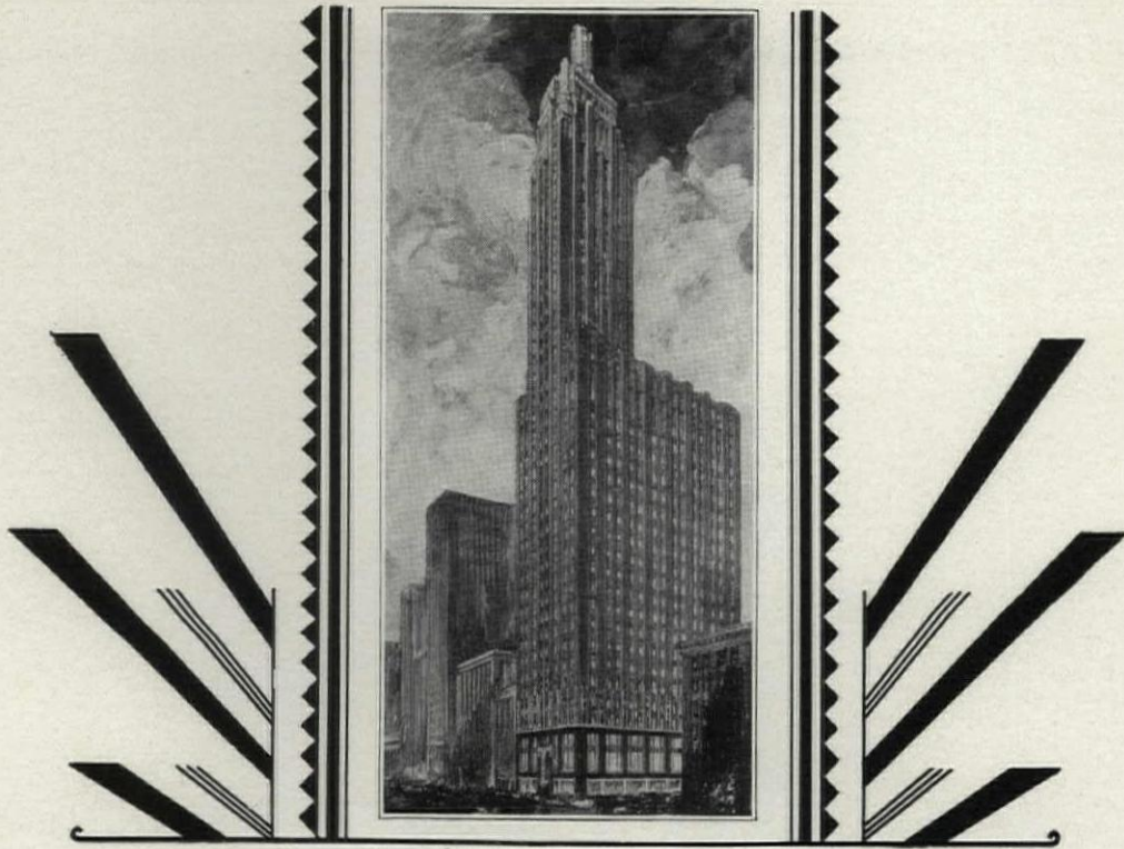
CARBIDE & CARBON BUILDING Chicago, Ill. Architects—Burnham Bros. Contractors—Paschen Bros.
