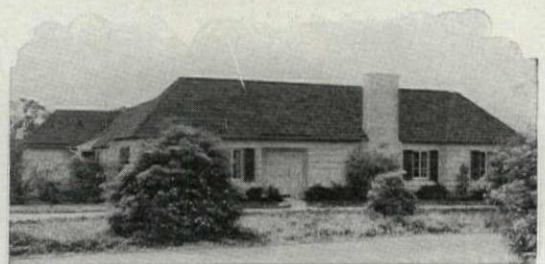
Photo by Haight Courtesy of "The American Architect" Attractive new home at Montecito, Calif. WITMER & WATSON, Architects
