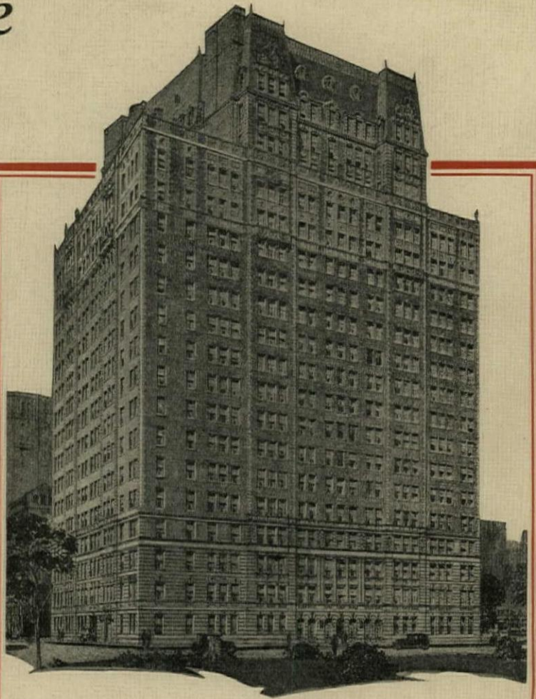
Co-operative Apartment, northwest corner Sheridan Road and Melrose Avenue, Chicago, Illinois. Architect: McNally, Quinn—10 South LaSalle Street, Chicago. Painting Contractor: Frank Gust, 7318 Ridgeland Avenue, Chicago. Material used: 1,250 gals. S-W Flattone 300 gals. Enamelastic 1,000 gals. S-W Wall Primer & Sealer 1,200 lbs. Oil Colors
