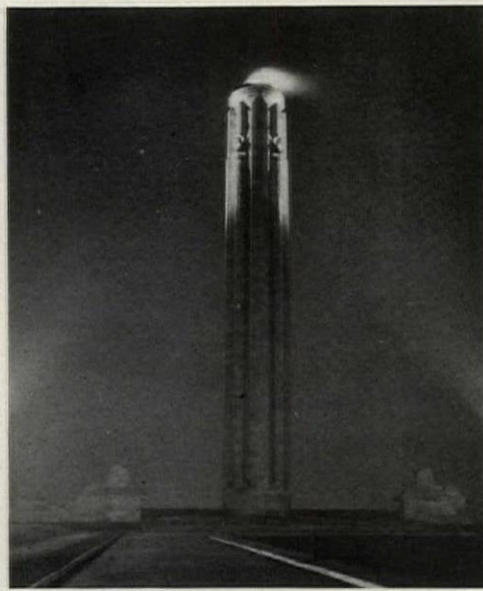
G-E searchlights are used to produce this pleasing effect of light and shadow on the Liberty Memorial at Kansas City, Mo. The units are concealed behind the cornices of the adjacent Memorial Buildings.
