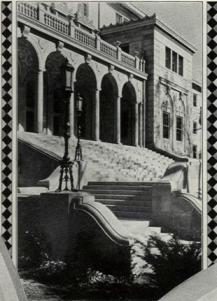
MEMORIAL UNION BUILDING, MADISON, WIS. (University of Wisconsin) Arthur Peabody, State Architect E. L. Perrault & Co., Painting Contractor
