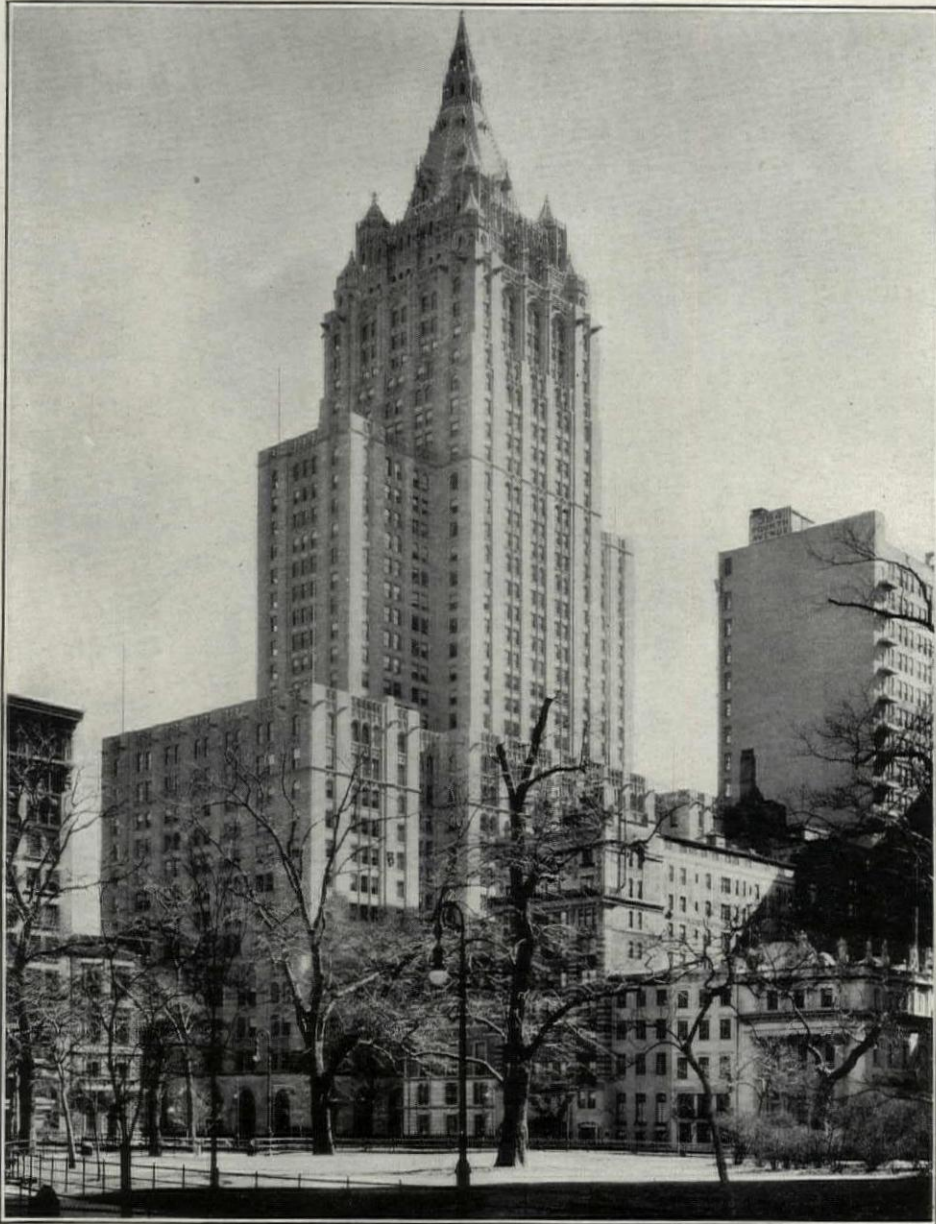
New York Life Insurance Company Building, New York City. Cass Gilbert, Architect. Starrett Bros., Inc., Builders. Built of Variegated Indiana Limestone.
