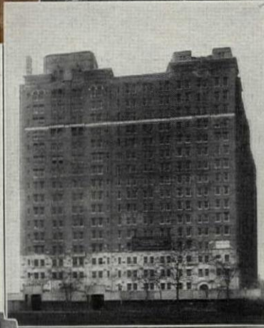
3260-70 Sheridan Road Hooper & Janisch, Architects Reliance Co., Inc., Contractors 100,000 sq. ft.—6¾", 9", 11¼" blocks
