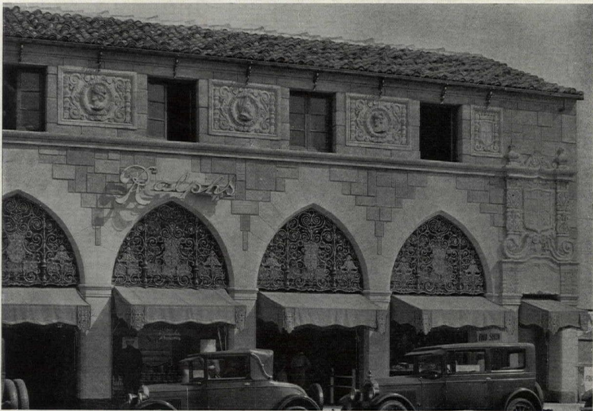
DETAIL OF SHOPS RALPHS GROCERY COMPANY BUILDING, LOS ANGELES MORGAN, WALLS & CLEMENTS, ARCHITECTS
