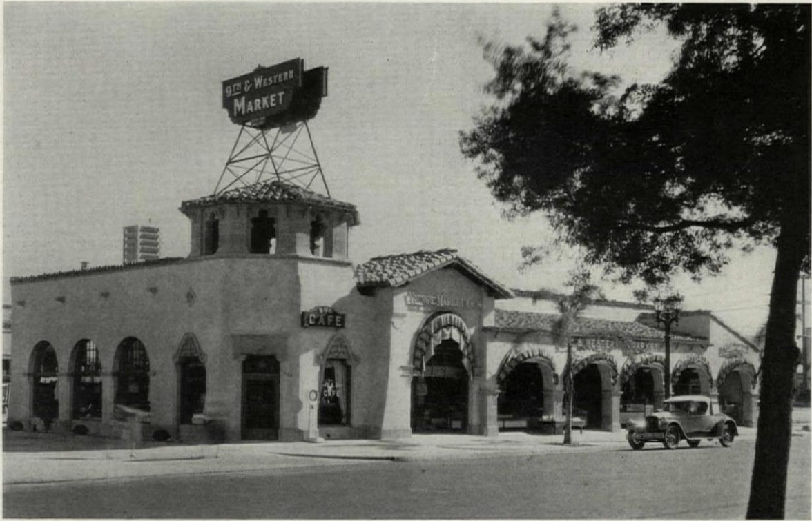
SOUTH BUILDING GROUP FOR THE BEVERLY WILSHIRE INVESTMENT COMPANY, LOS ANGELES MORGAN, WALLS & CLEMENTS, ARCHITECTS
