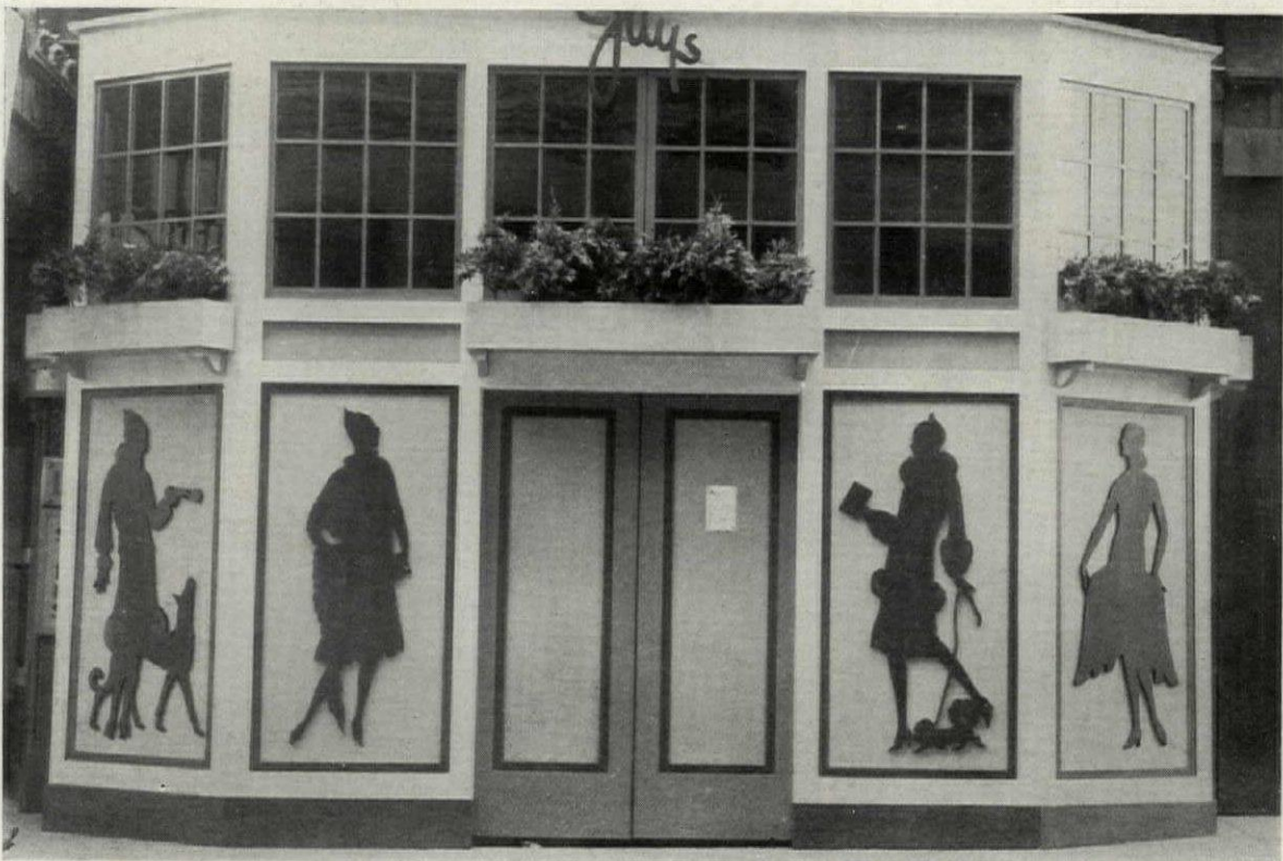
BARRICADE DURING CONSTRUCTION OF ADDITION TO JAY'S, BOSTON
