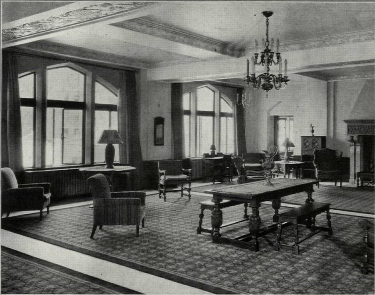
Lounge of the new Y. W. C. A. building at Cincinnati. Light, airy, cheerful. Rendigs, Panzer & Martin, Architects. F. B. & A. Ware, Associate Architects.
