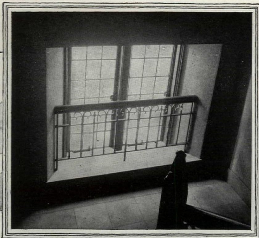
Stair landing at Union Theological Seminary, New York, N. Y. Allen N. Collins, Boston, Architect.
