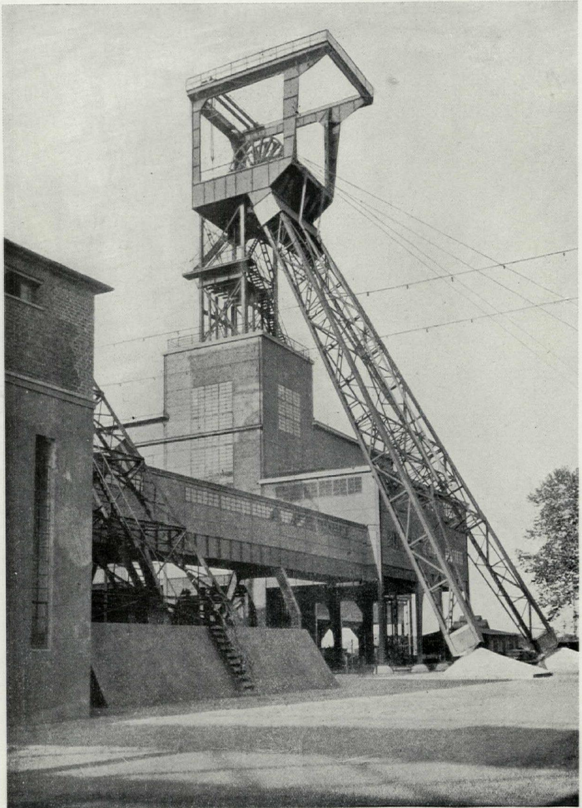
FROM PAGE 33, "ARCHITECT VS. ENGINEER." PROPER INCORPORATION OF OPEN STEEL SUPERSTRUCTURES IN THE BUILDING SCHEME THROUGH TOWER BASES
