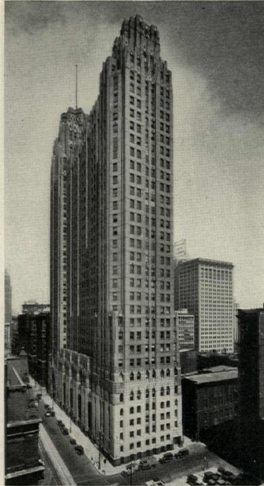
The Union Trust Building, Detroit; Smith, Hinchman & Grylls; Donaldson & Meier, Architects
