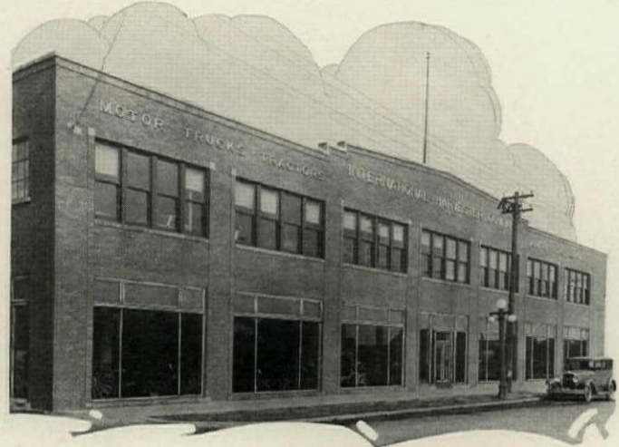
International Harvester Co., St. Cloud, Minn., an industrial building with many large display windows safely set in Brasco construction
