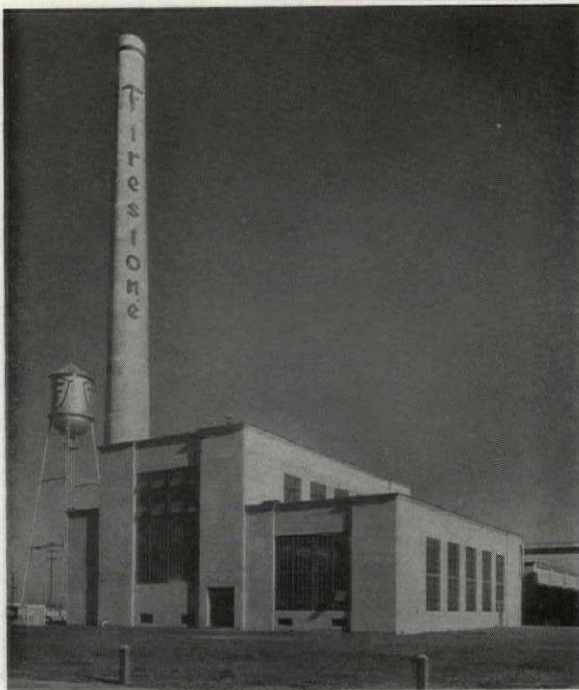
Courtesy of Stone & Webster Engineering Corporation BOILER PLANT, FIRESTONE TIRE & RUBBER CO., LOS ANGELES
