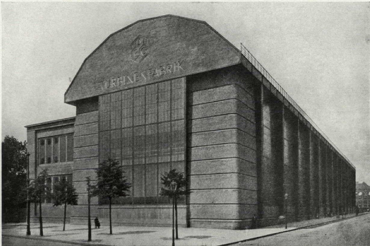
TURBINEN HALLE, A. E. G. COMPANY, BERLIN PETER BEHRENS, ARCHITECT
