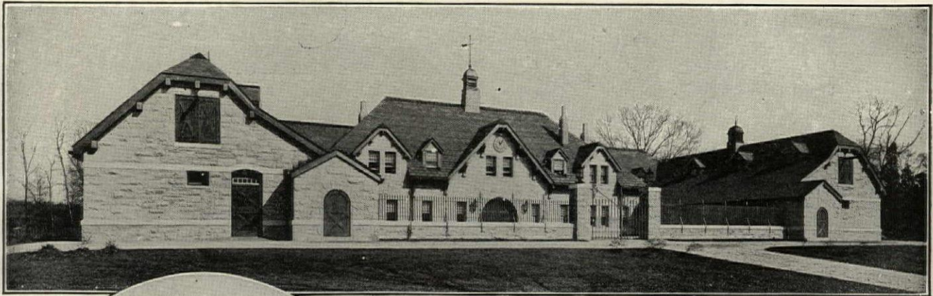
STABLES OF WM. ZIEGLER, JR., NOROTON, CONN., H. P. KNOWLES, ARCHITECT
