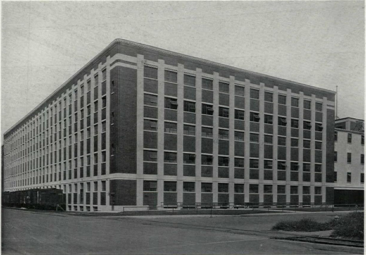
Warehouse, Mishawaka Woolen Mills Company, Mishawaka, Ind. Albert Kahn, Inc., Architects and Engineers
