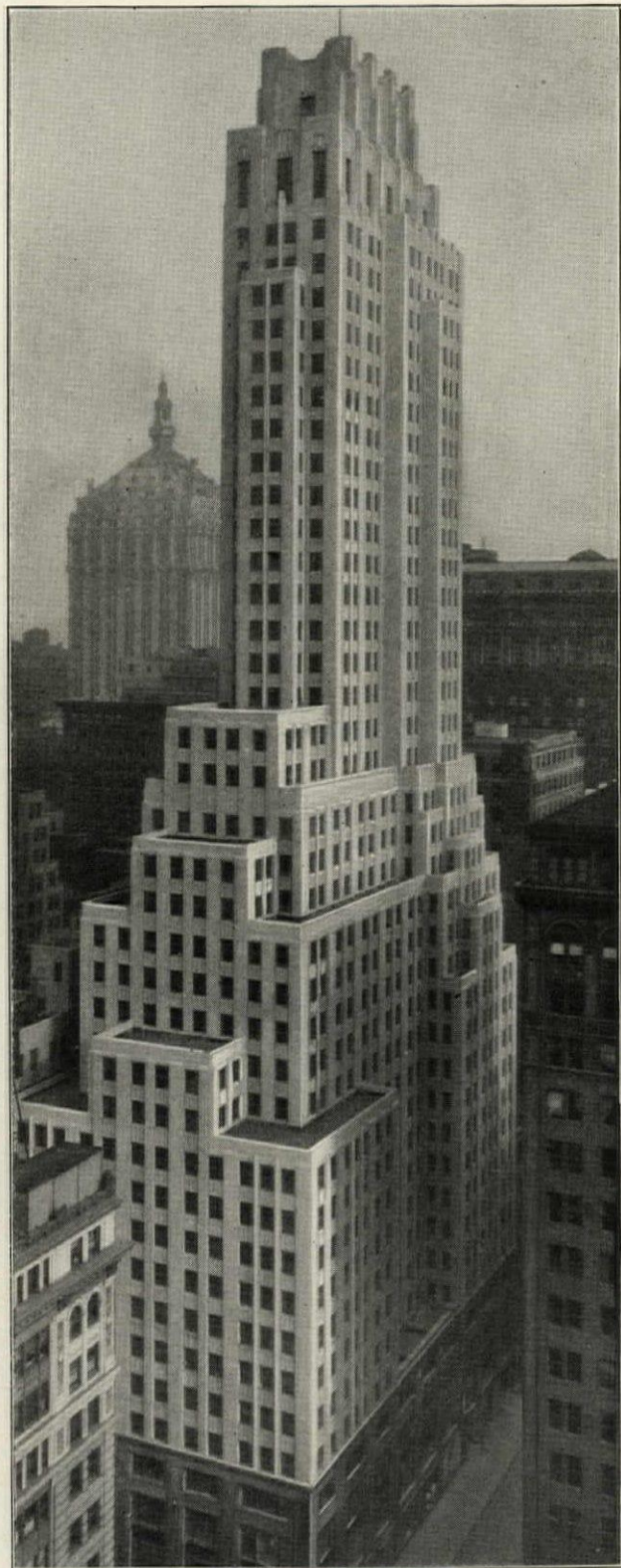
LEFCOURT NATIONAL BUILDING, NEW YORK CITY Management of A. E. Lefcourt Realty Holdings Architect: Shreve & Lamb
