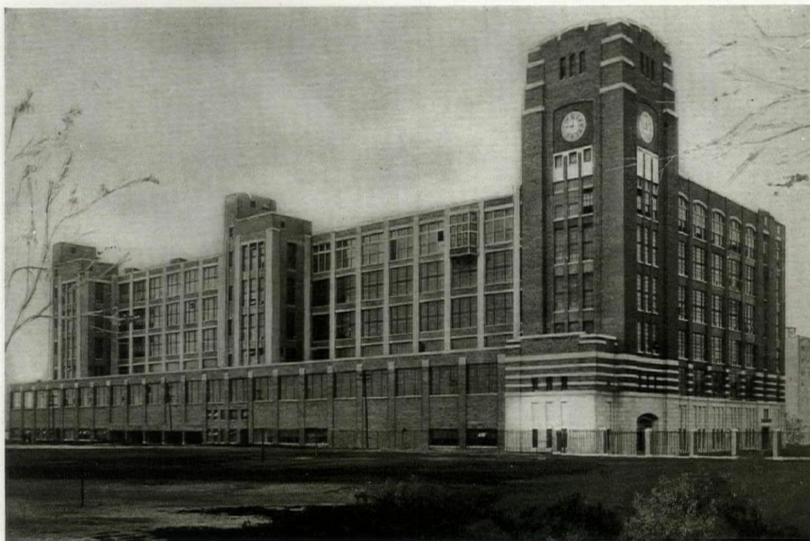
BUILDING FOR W. F. SCHRAFFT & SONS, BOSTON DESIGNED BY LOCKWOOD GREENE ENGINEERS, INC.
