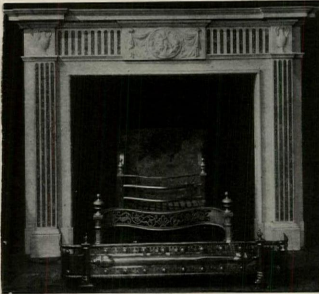
Finely carved statuary marble mantel with brocatelle inlay. Shelf 6' 0" x 4' 8", opening 3' 8½" x 3' 5½" high.
