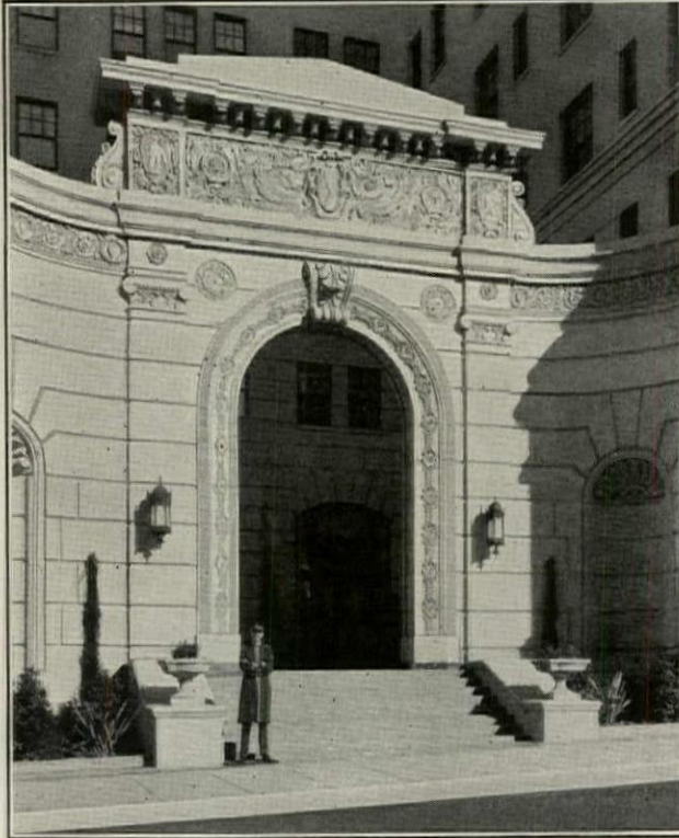
The entrance to the Arcady Apartments in Los Angeles, is a striking example of the ornamental beauty attainable in monolithic concrete. Walker and Eisen, Architects, Los Angeles.
