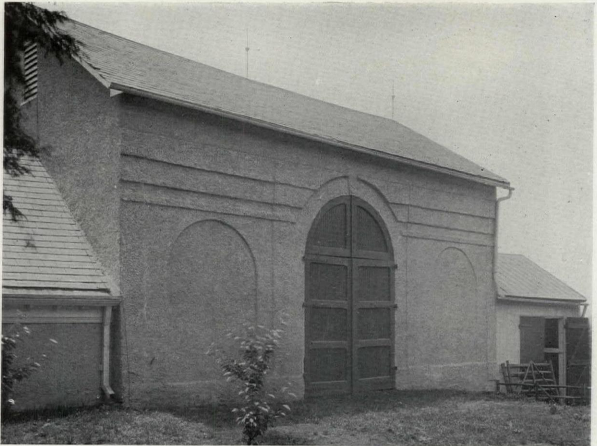
North Front of Barn, Unaltered "Kenwood," Bethayres, Pa.
