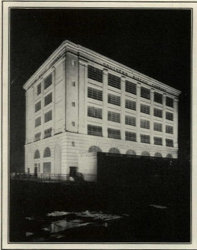
This modern factory building, the plant of the Southern Biscuit Works at Richmond, Va., demonstrates the combination of true beauty with the purely practical in reinforced concrete construction. The picture at the left shows also how splendidly a concrete exterior lends itself to flood lighting. Francisco and Jacobus, Architects, New York City.
