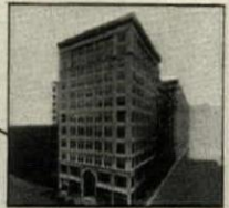
Bedell Building, Portland, Ore.
