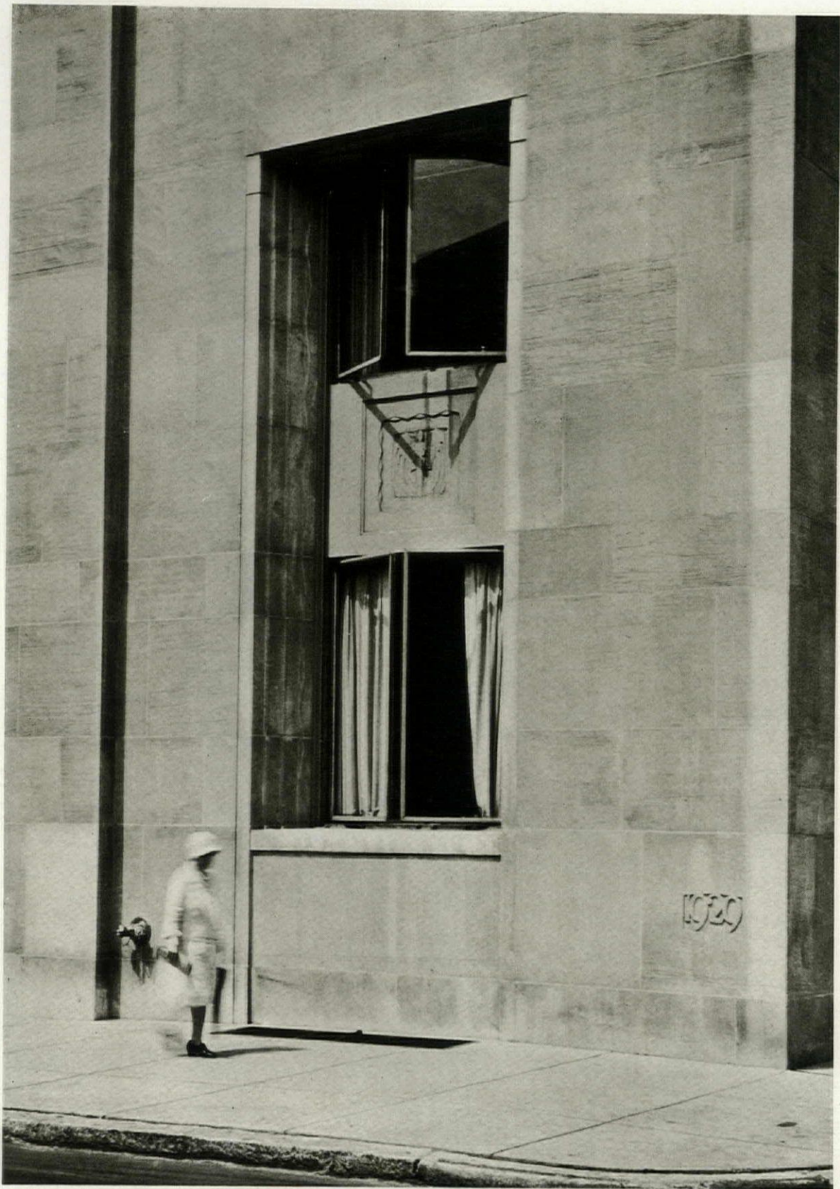
DETAIL, FRONT ELEVATION BUILDING FOR N. W. AYER & SON, INC., PHILADELPHIA RALPH B. BENCKER, ARCHITECT
