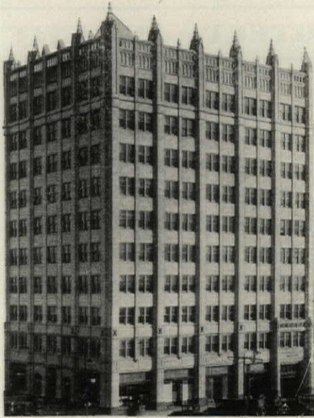
Owners of the National Reserve Life Insurance Company Building, Topeka, Kansas, need not worry about their heating and ventilating ducts for years to come. All sheet metal parts are of ARMCO Ingot Iron, the iron that fights rust and corrosion. Architect: Ralph E. Scamell, Topeka. Sheet Metal Contractor: George Warren Sheet Metal Works, Topeka.
