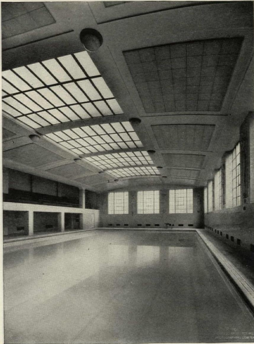
Johns-Manville Sanacoustic Tiles installed as ceiling of Girls' Swimming Pool, Oak Park and River Forest Township High School, Oak Park, Ill. Childs & Smith, Architects, Chicago, Ill.
