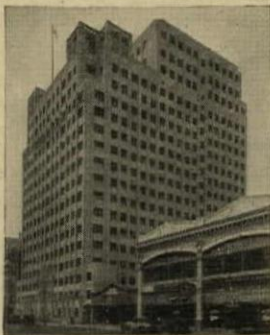
The Hahnemann Hospital, Philadelphia, Pa., where Monel Metal American-Perry Laundry Machines have been installed.
