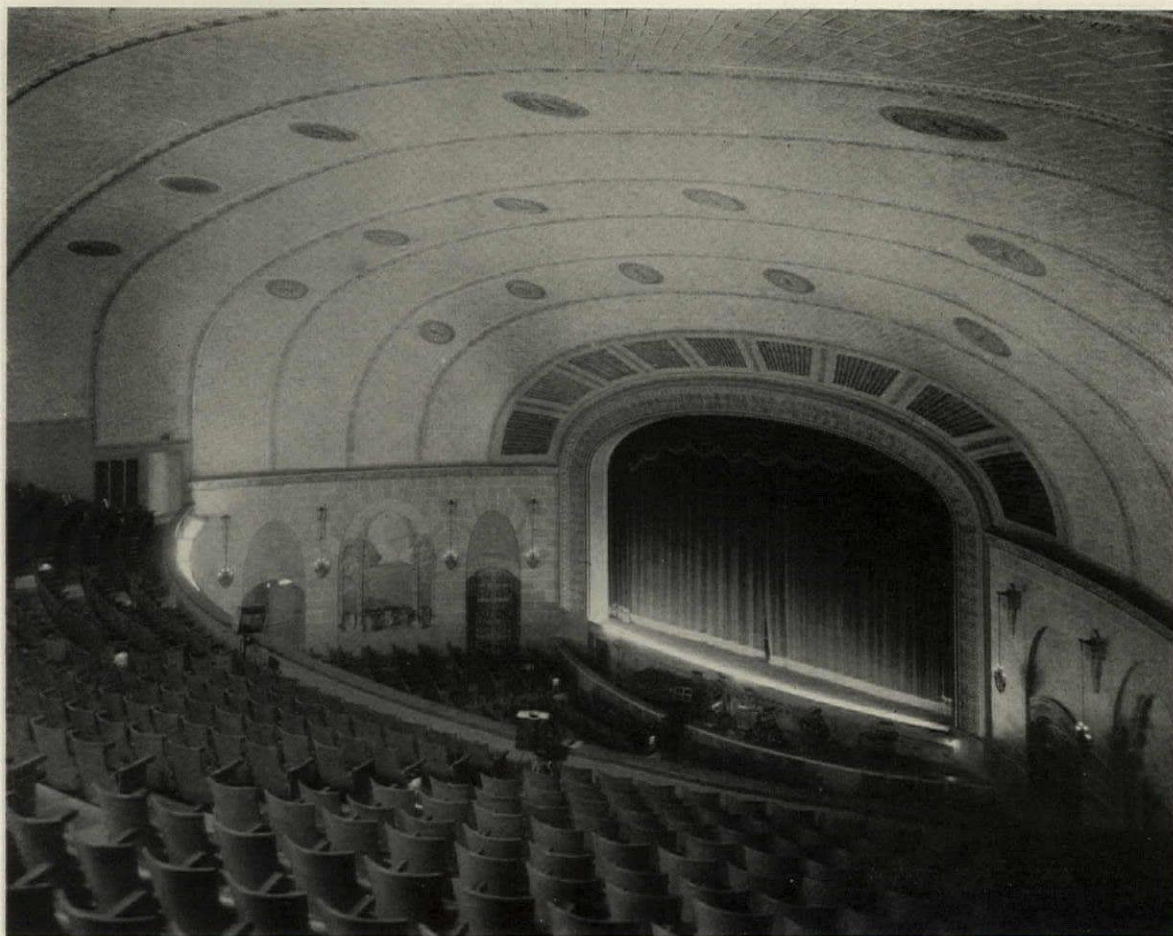
Theater with Ceiling Curvature which Would Produce Echoes, Corrected by Using Absorbent Tile Vaulting
