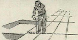
Tying the reinforcement
