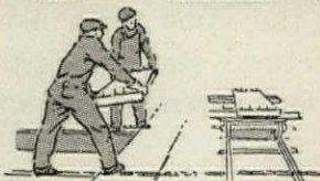
Laying a Gypsteel slab
