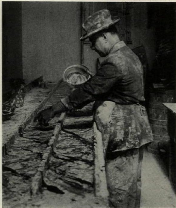
Various Colored Cements are Distributed to Give the Effect of Mottled Backgrounds
