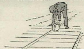
Grouting the joints between slabs
