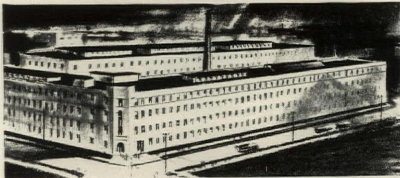
St. Louis Ave. Plant International Shoe Company , St. Louis Mo. Constructed by International Shoe Co., Eng. Dept. Barrett Roofed by Swift Roofing Co., St. Louis, Mo.
