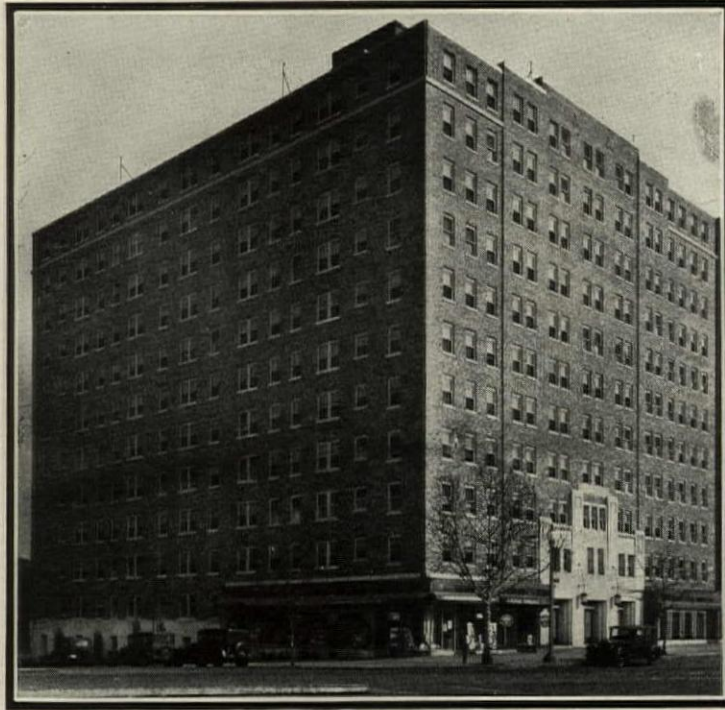
In the Park Lane Apartments, Frigidaire adds to the comfort, health and satisfaction of tenants in 276 suites. This is one of the largest and most popular apartment buildings in the city.
