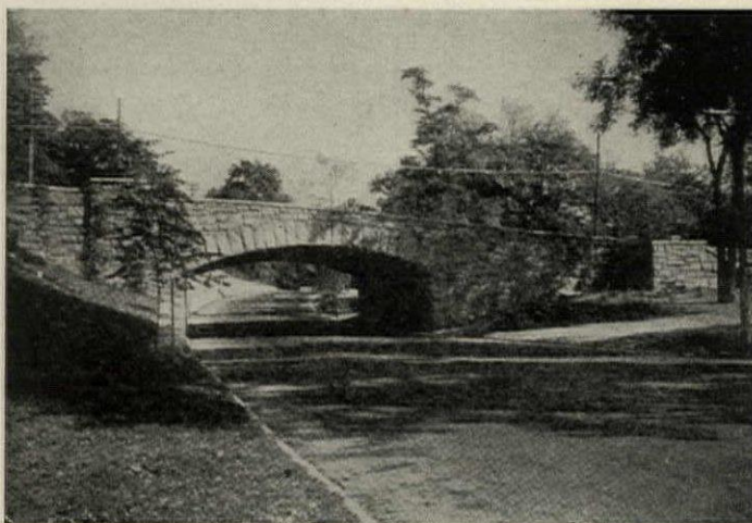
A Grade Separation, Tuckahoe Road, Bronx River Parkway, New York
