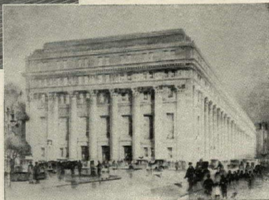
The stately Mitsui Bank, Tokyo, Japan, atop which is a Carey Built-up Roof.
